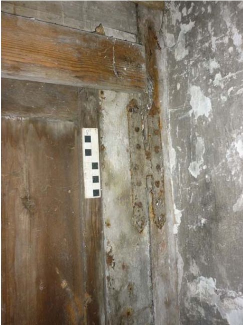
Plate 25 (left): Hinge detail on the door to the east side of the north internal elevation of Room 2
