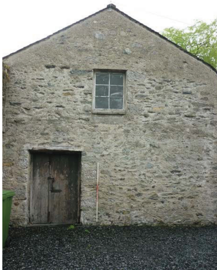
Plate 15: West external elevation
