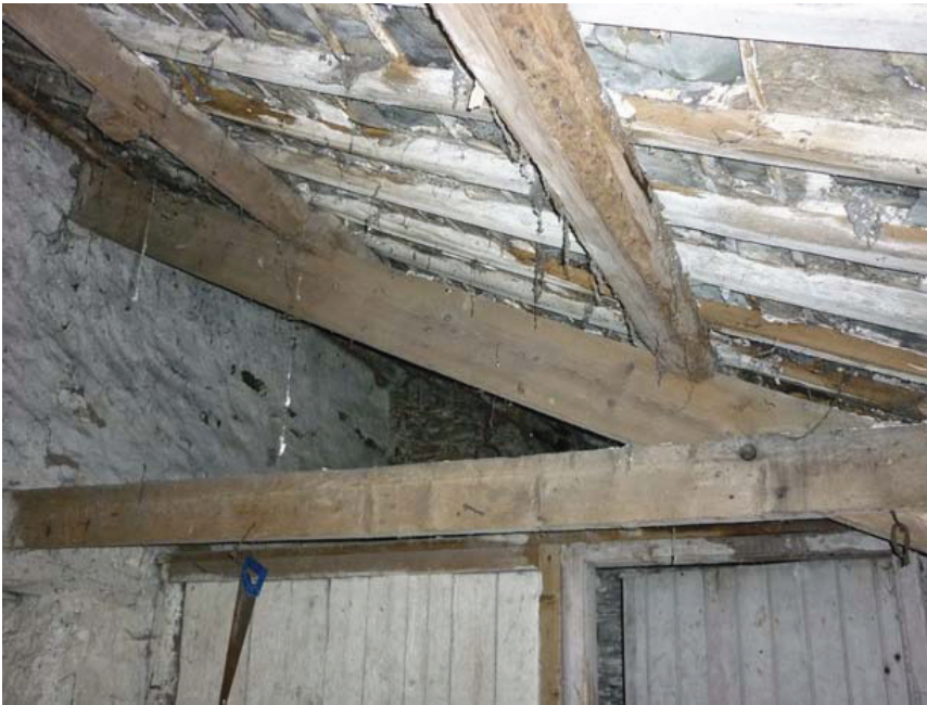
Plate 18 (left): Half truss in Room 1
