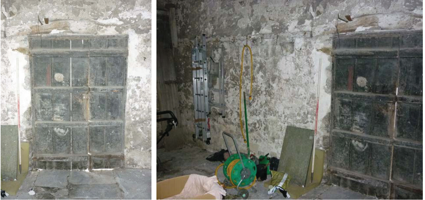
Plate 29 (left): Double plank and batten door on the north side of the west internal elevation of Room 2
