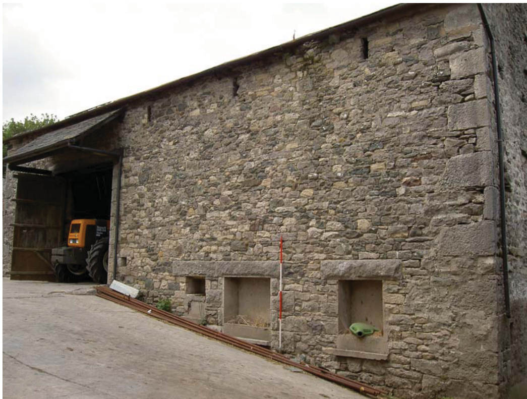
Plate 6: The inserted and blocked windows on the east side of the south external elevation, looking north-west
