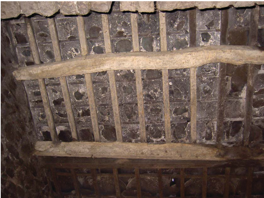
Plate 13: Roof of porch on the north side of the barn showing the hand-finished timbers, looking up
