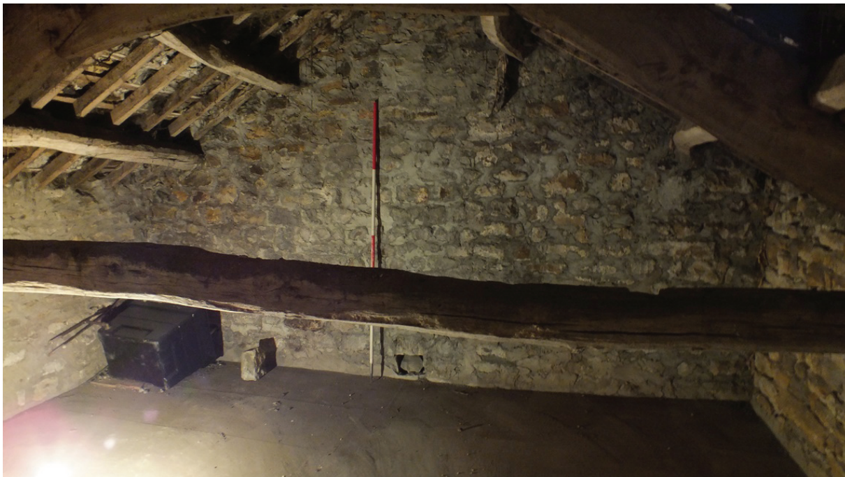
Plate 28: South-west elevation (F1)
