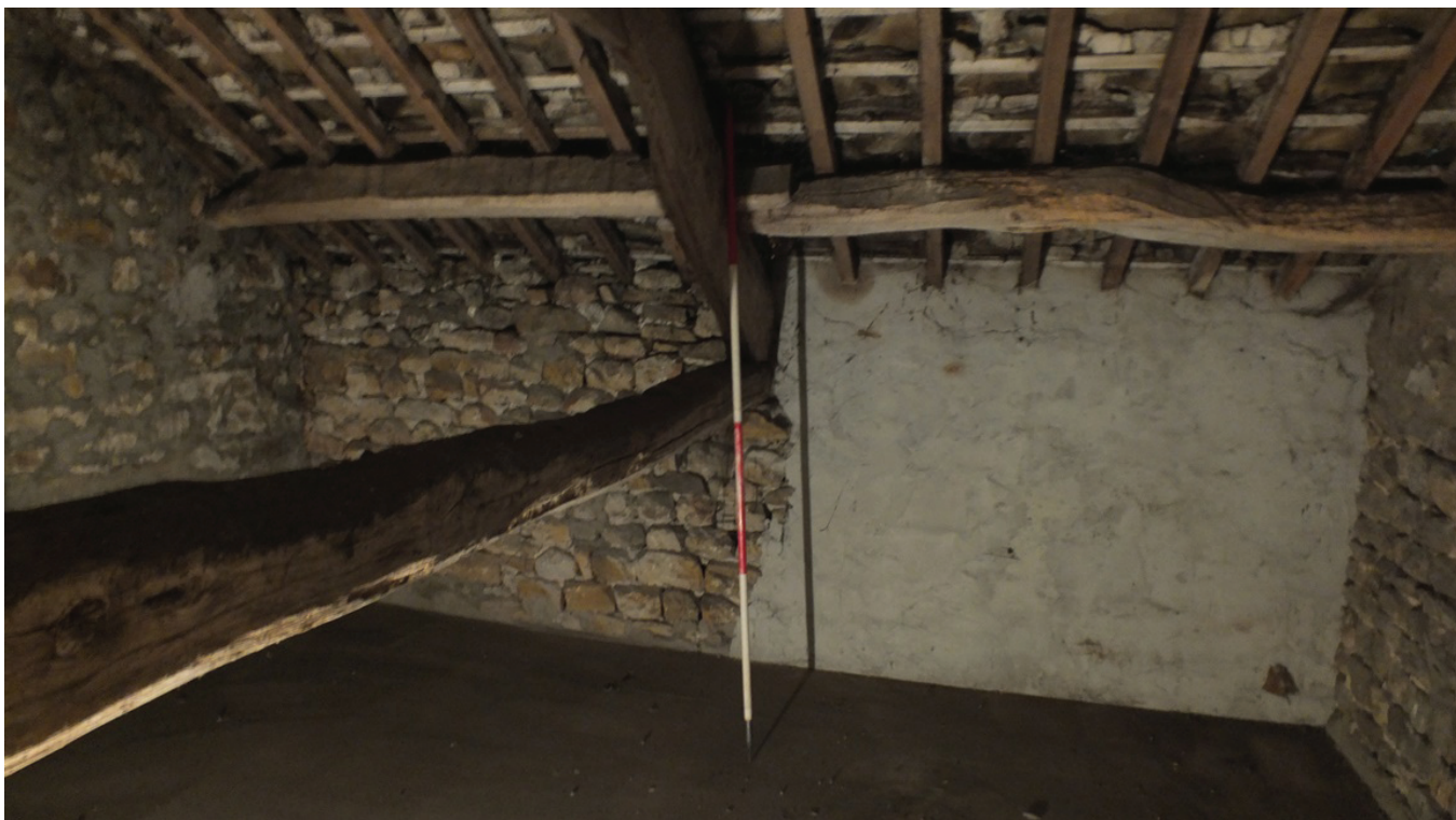
Plate 31: North-west elevation (F1)
