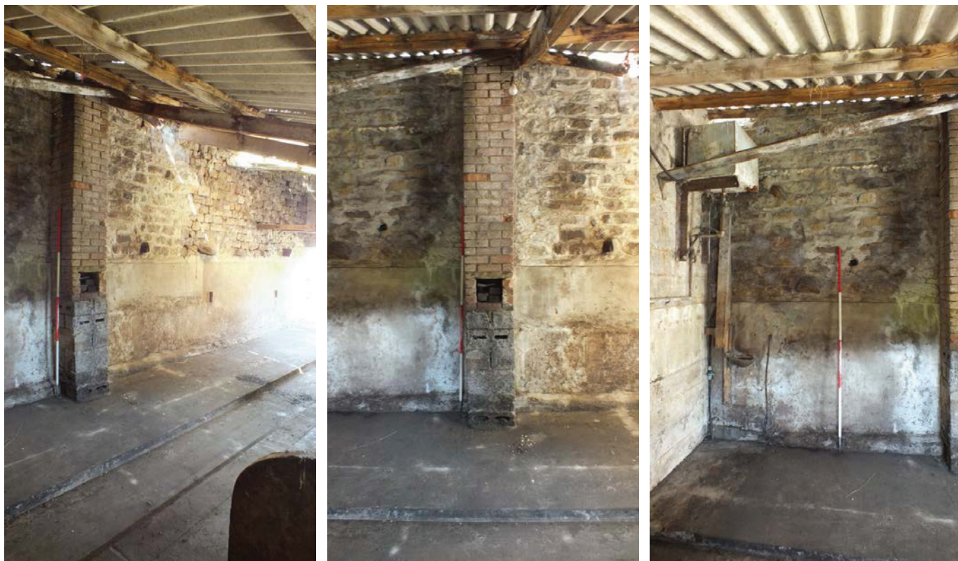
Plate 22 (left): North-east end of the north-west elevation (G2)
