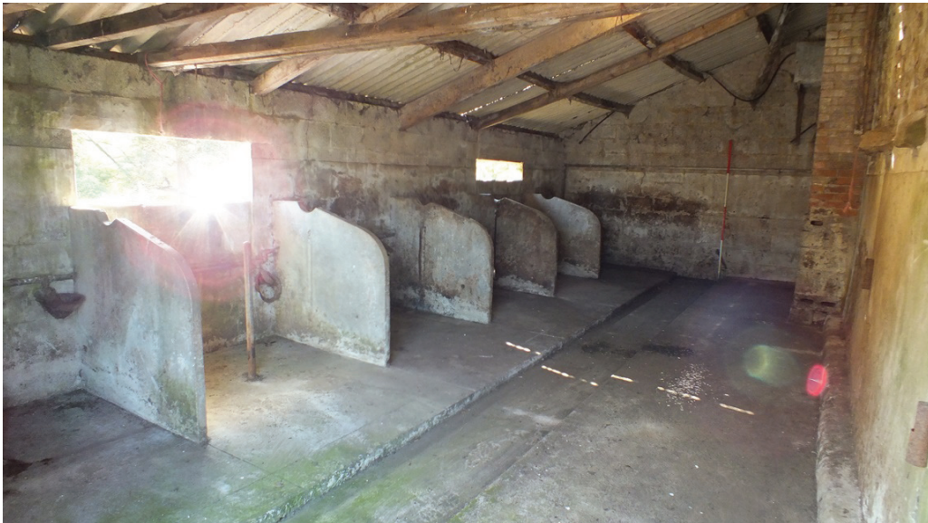
Plate 20: Stalls along the south-east elevation of G2
