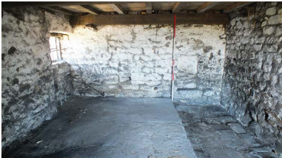
Plate 16: South-east elevation of G1
