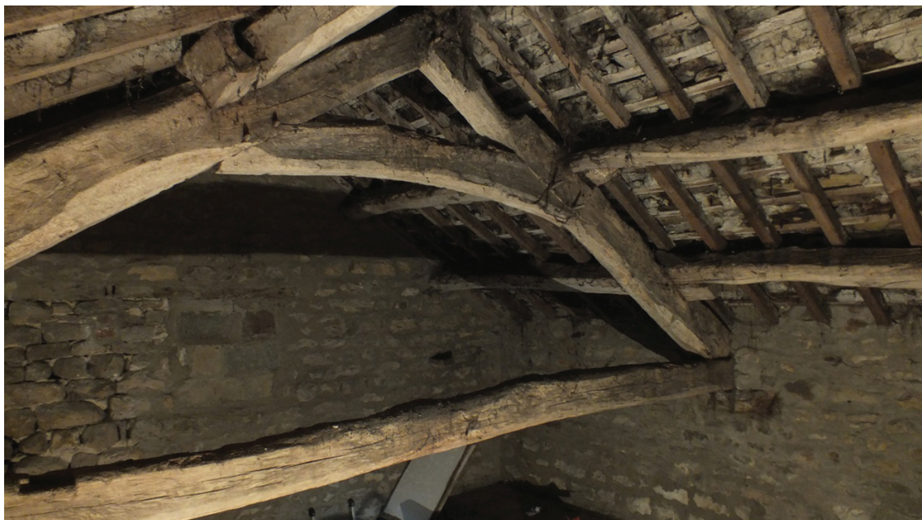
Plate 32: South-west side of the truss (F1)
