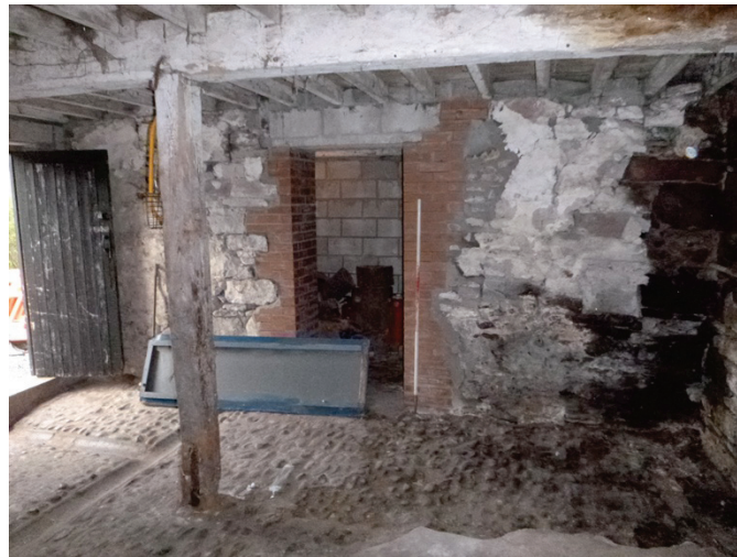
Plate 27: West elevation, Room G3, viewed from the east
