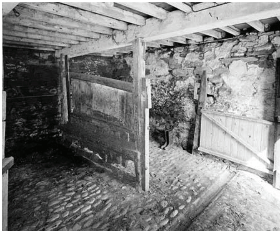
Plate 11: Photograph of the ground floor of the building in 1992 (Historic England 2014)
