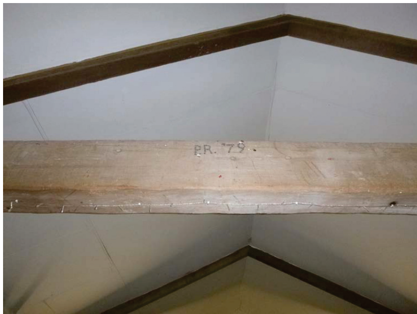
Plate 42: Text on truss in Room F1, viewed from the west
