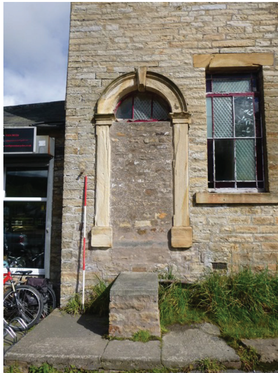
Plate 52: Blocked doorway at the west end of the south external elevation, viewed from the south
