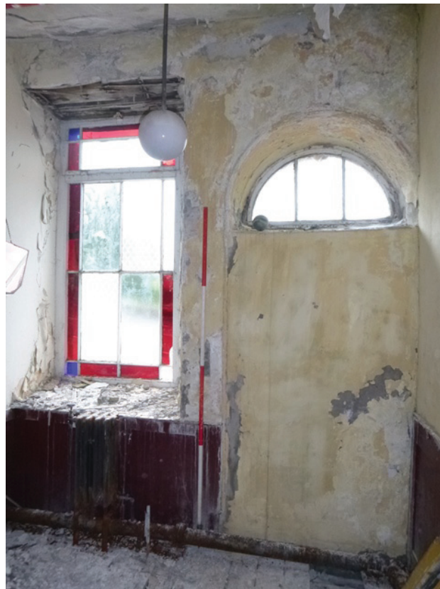
Plate 81: Window and blocked doorway in the south elevation, ground floor Room 4, viewed from the north
