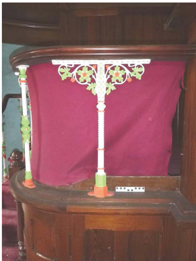
Plate 65 (left): Detail of the iron brackets supporting the pulpit rail, ground floor Room 2, viewed from the north
