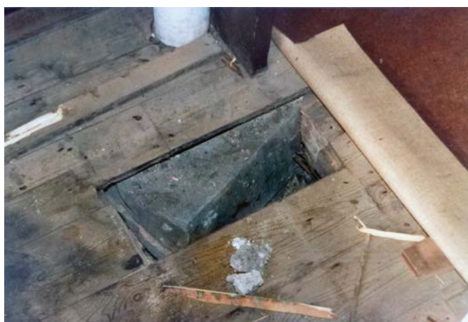
Plate 28: Cast iron column base, 1986 (CAC(C) DFCM/10/237 1986)
