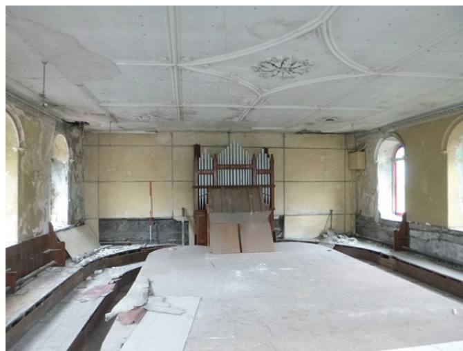
Plate 91: The west elevation in first floor Room 1, viewed from the east
