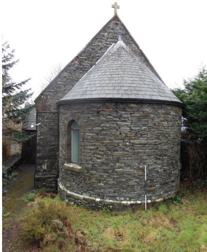
Plate 5: East external elevation, viewed from the east
