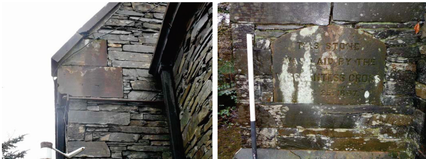
Plate 6 (left): Kneeler with tie rod running across, south side of east external elevation, viewed from the east
