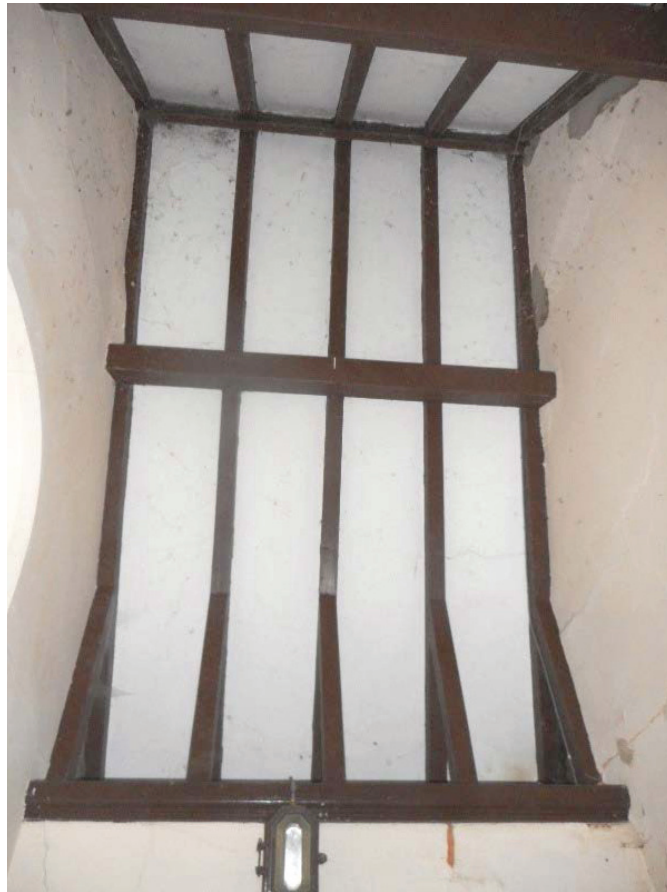
Plate 31: Roof in Room 3
