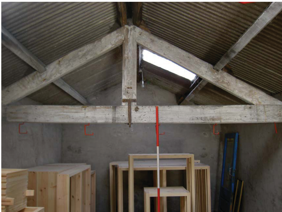
Plate 8: Detail of roof structure
