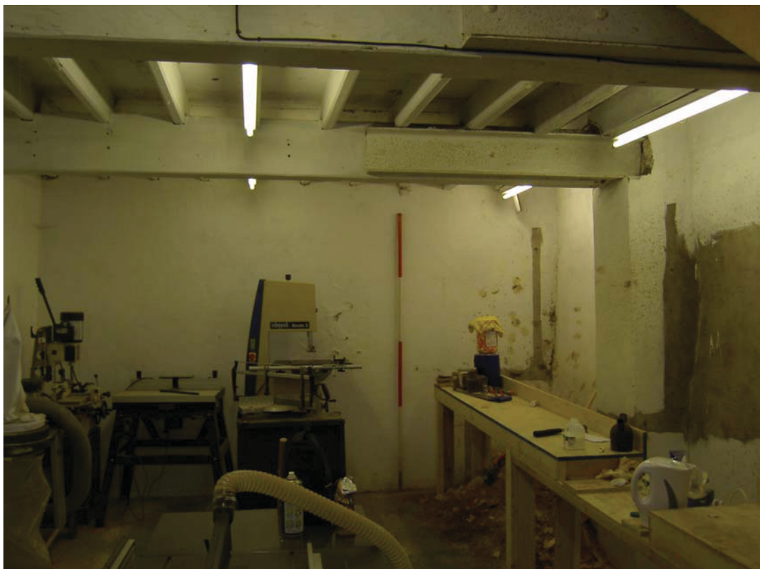
Plate 10: Detail of first floor beam repair
