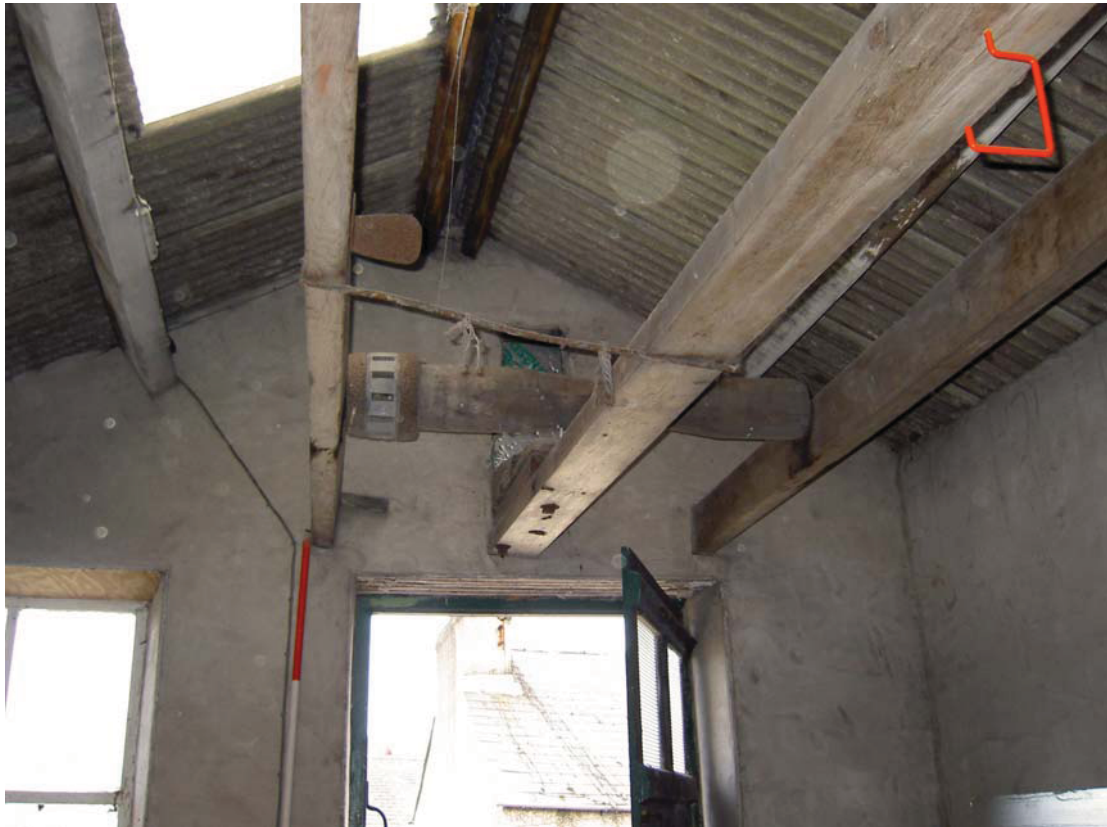
Plate 9: Hoist mechanism on second floor
