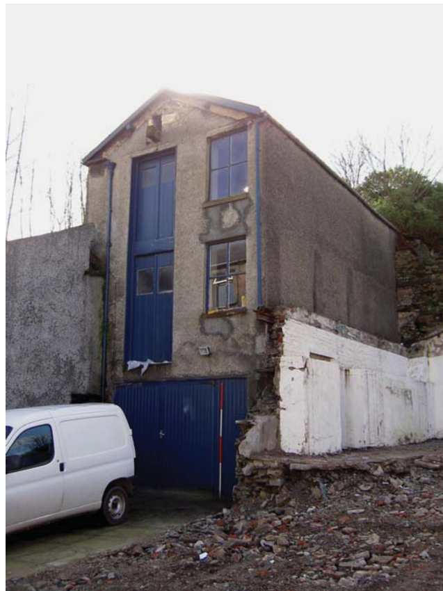
Plate 6: External north-east elevation, from the north
