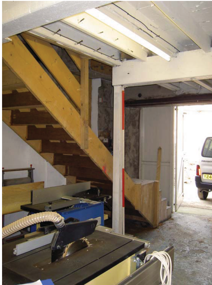
Plate 11: Cut beam and post support to accommodate modern stairway
