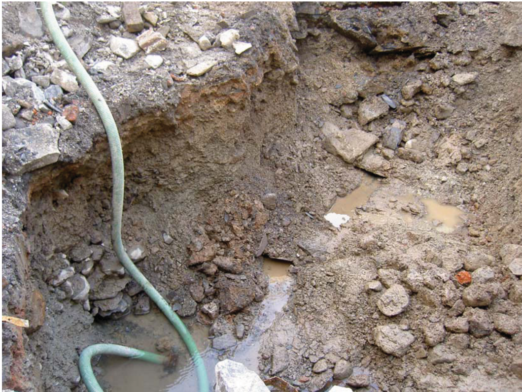
Plate 12: Culvert in Trench 1
