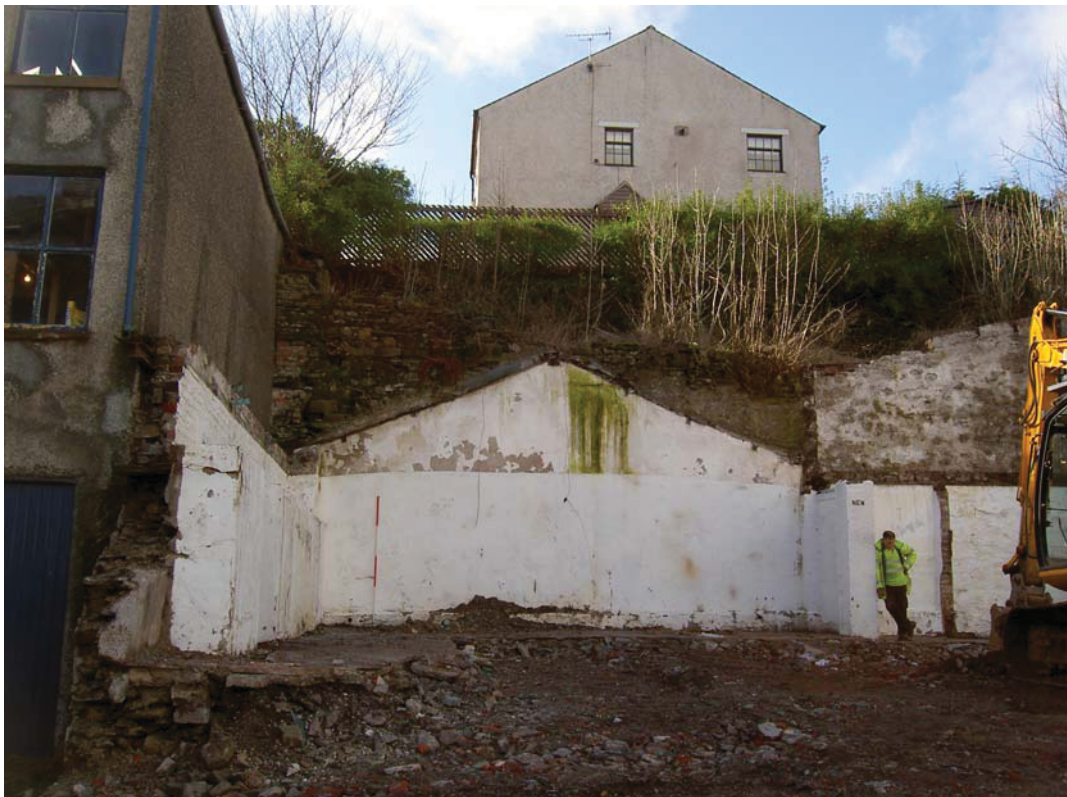
Plate 15: Current retaining wall to rear of plot indicating landscaping of site
