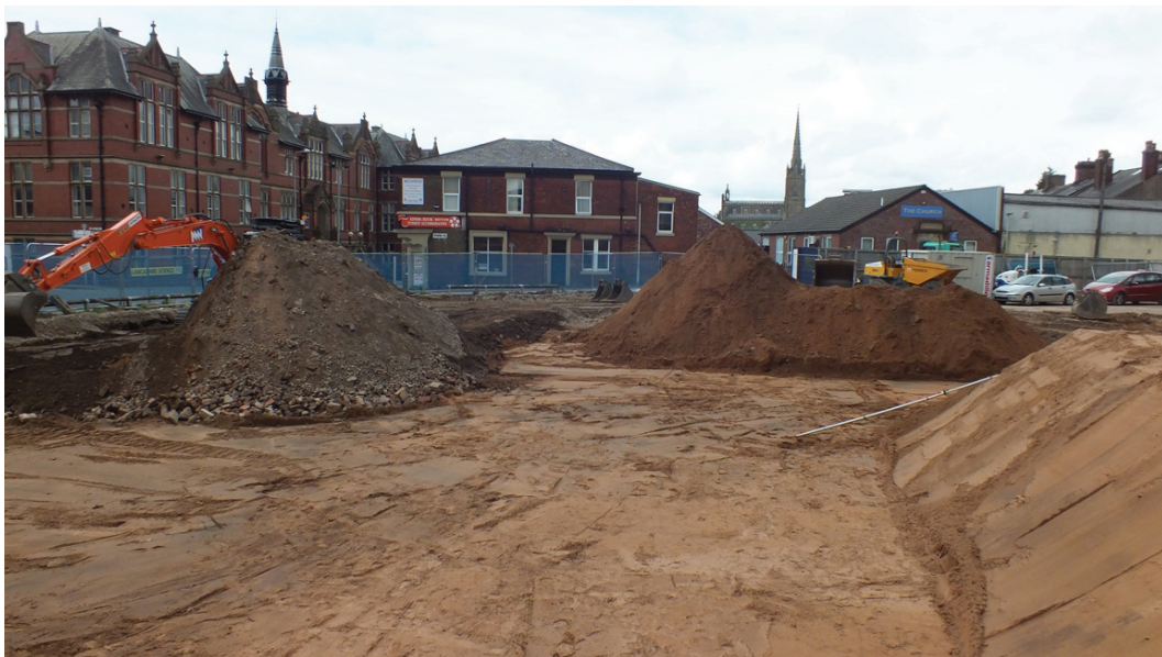
Plate 8: Site viewed from the south-east
