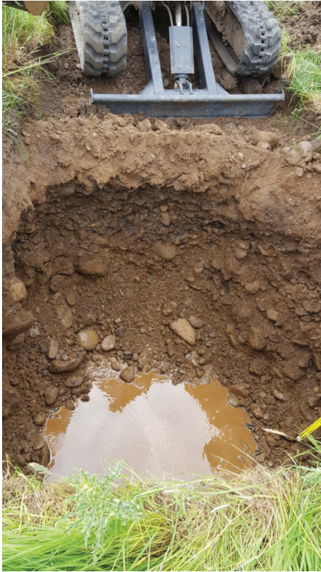
Plate 14 (left): The partially-excavated trench for the septic tank (photograph: J. Beaty)
