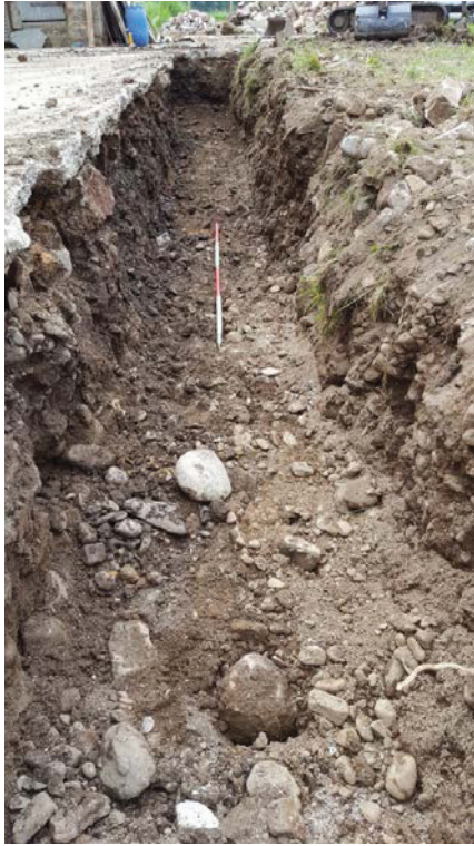
Plate 10 (left): The western section of the foundation trench for the extension on the western side of the barn. The scale measures 2m in length (photograph: J. Beaty)
