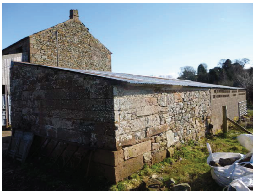
Plate 3: Building to the south showing extant original fabric (photograph: J. Parsons)
