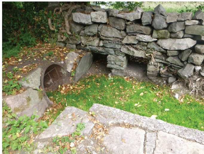
Plate 19: Structure against the south end of the western boundary, presumed to be part of the leat, showing the iron 'pipe' and leat
