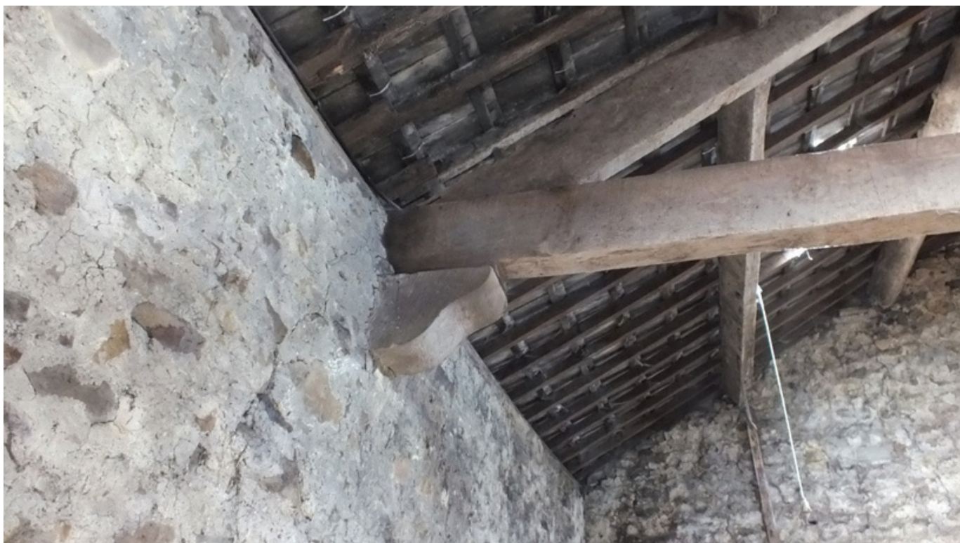
Plate 20: Scrolled corbel below the north end of the truss in G1
