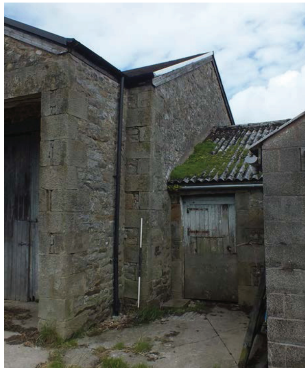
Plate 8: The east external elevation
