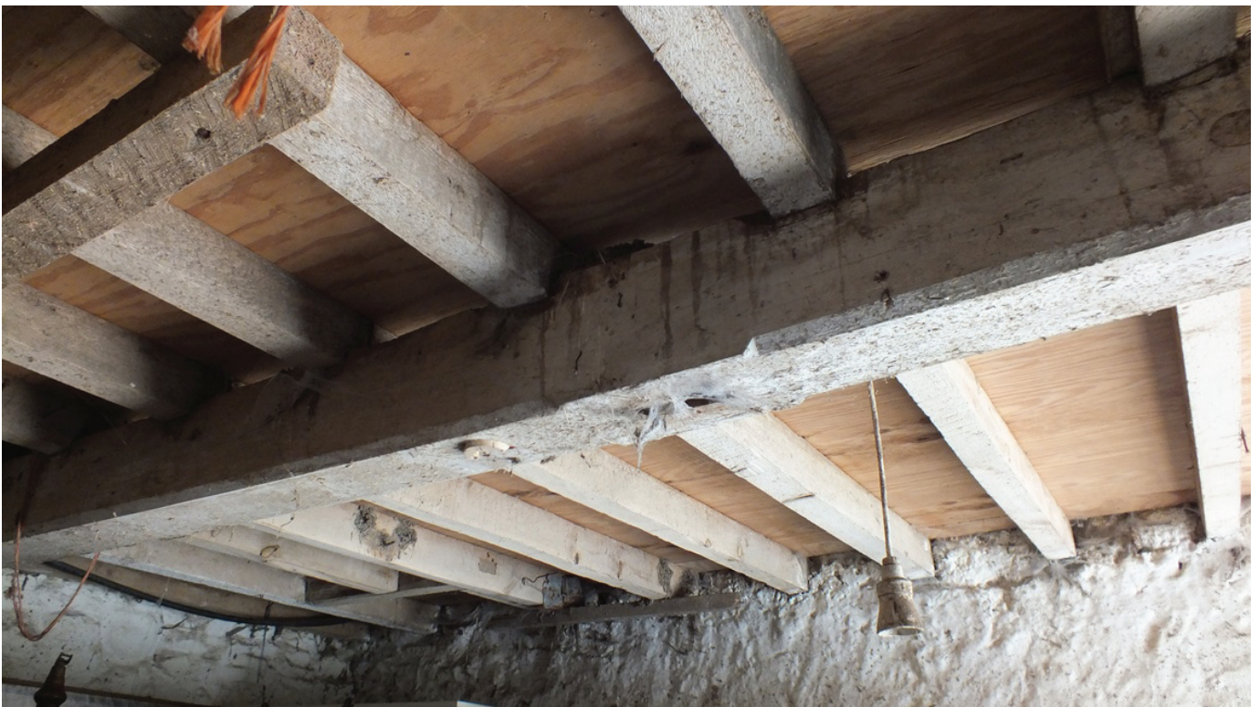
Plate 27: Detail of the chamfered beam and slot in G3
