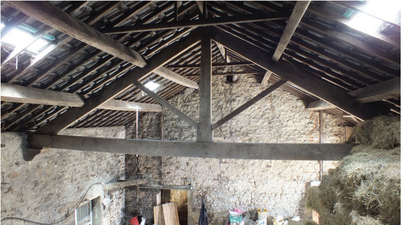
Plate 19: Truss in G1
