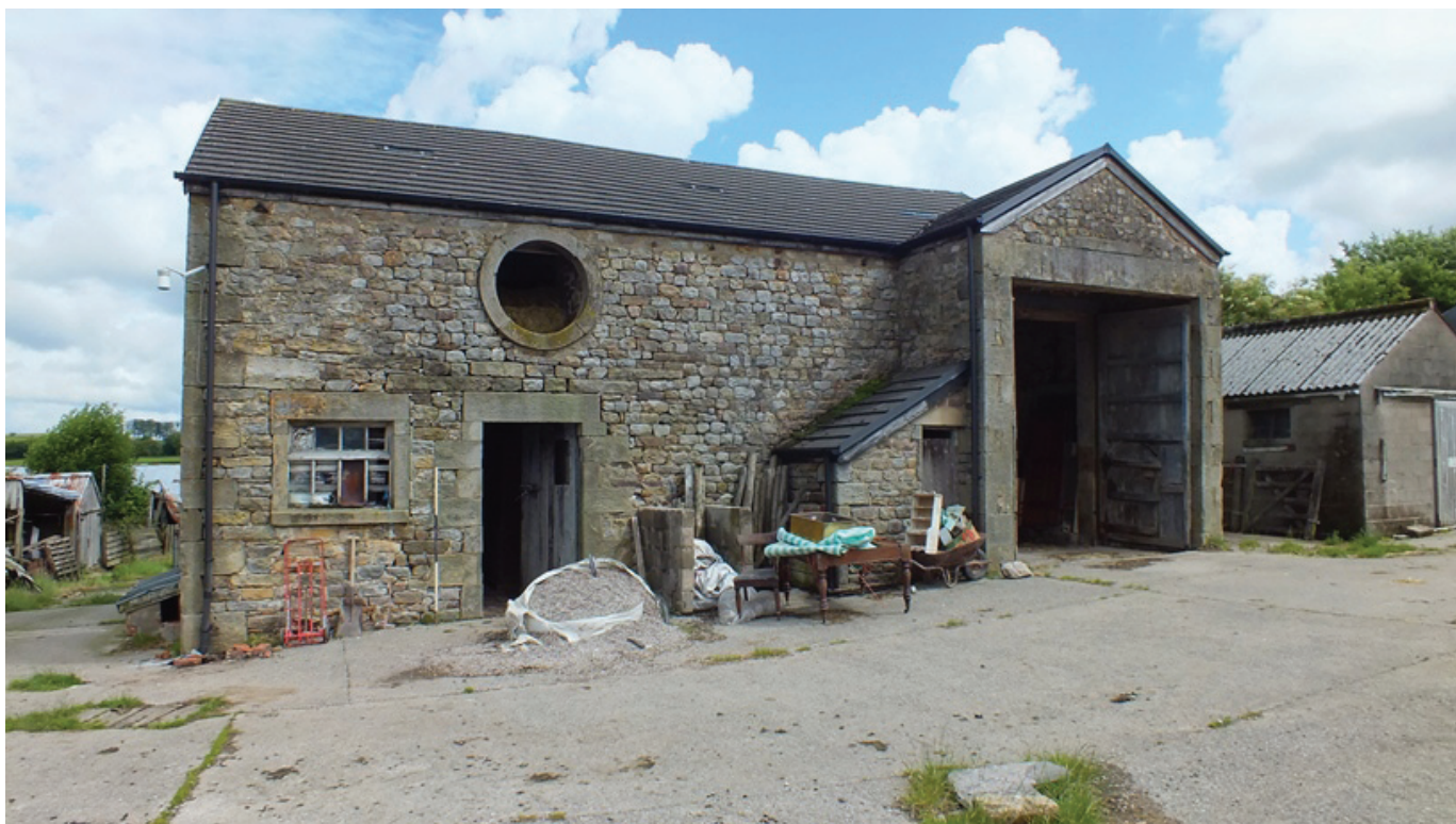
Plate 10: General view of the south external elevation
