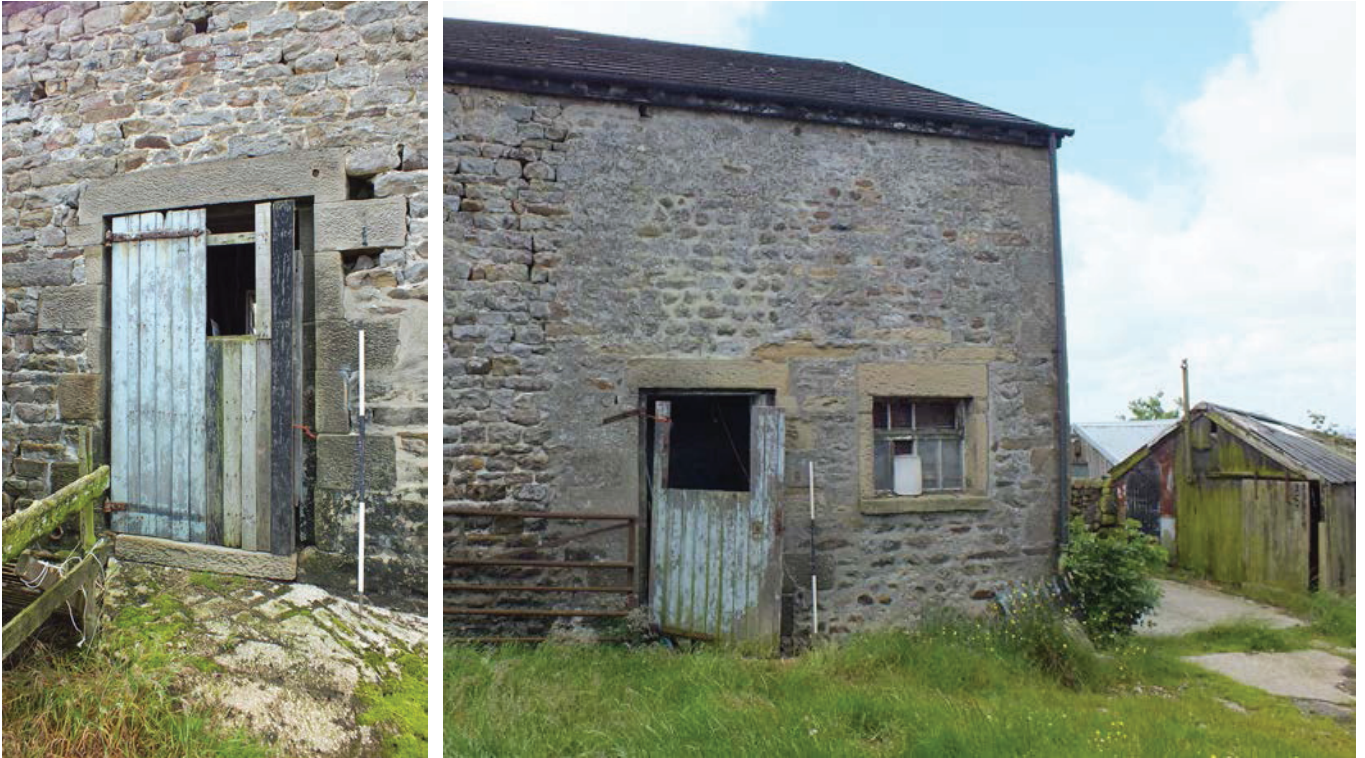
Plate 6 (left): Doorway at the east end of the north external elevation
