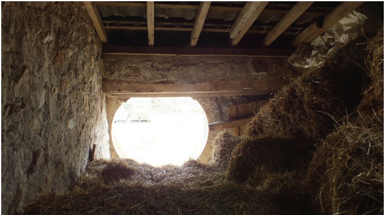
Plate 33: Pitching window in the south elevation of F1
