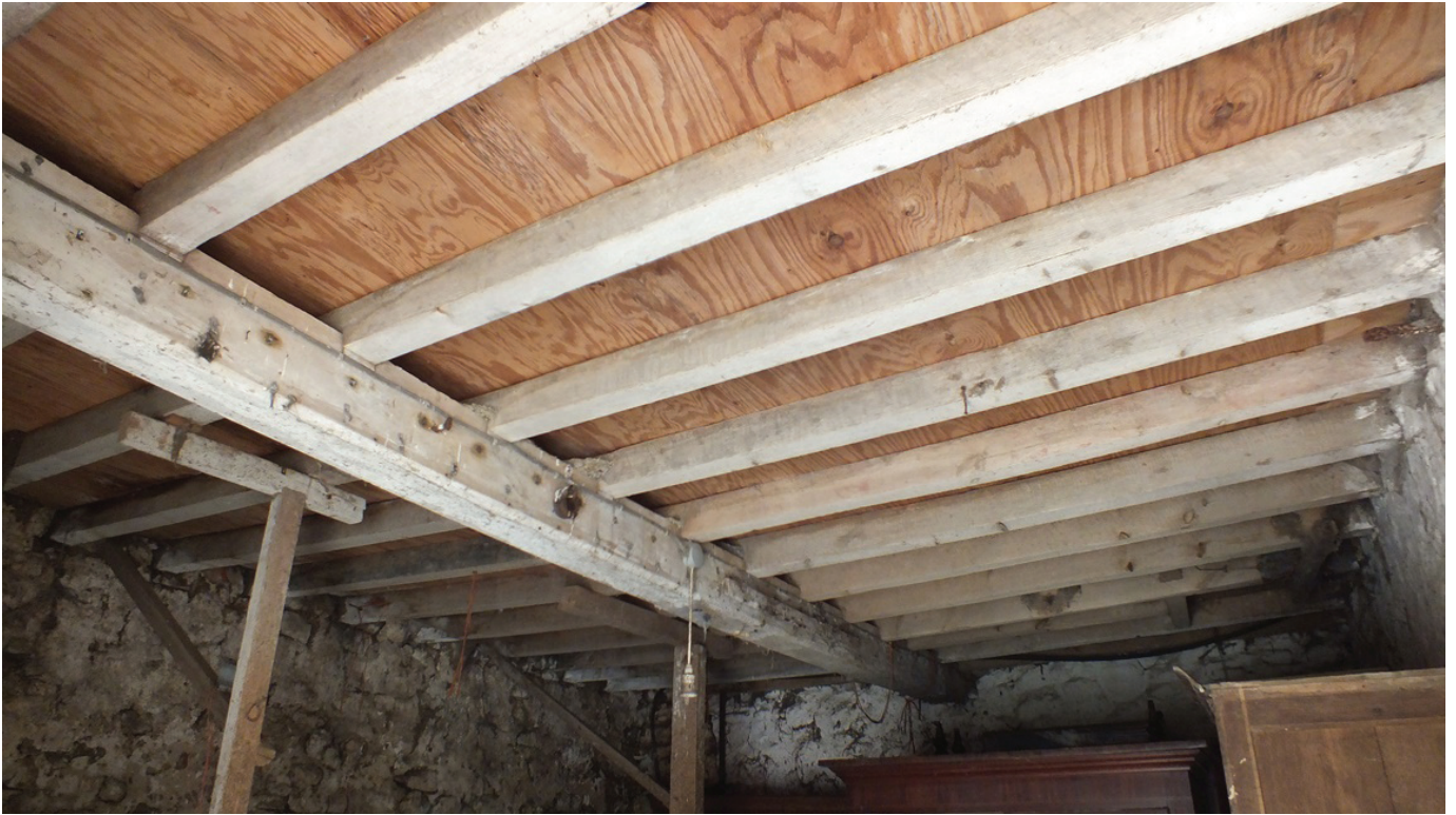
Plate 26: Beam across the ceiling in G3
