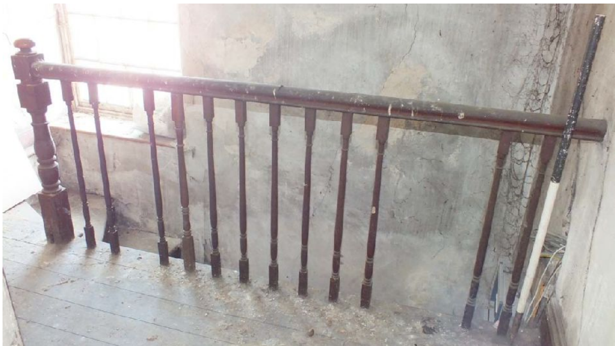
Plate 114: Detail of the stair rail on the second floor
