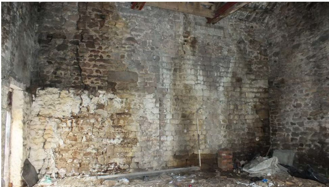
Plate 59: West elevation of the barn
