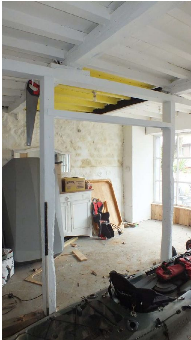
Plate 26: Timber posts supporting the joists in G1
