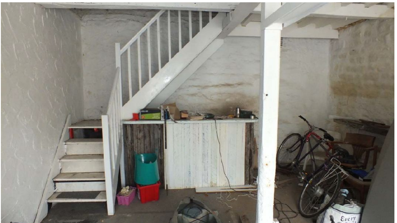
Plate 28: The west elevation of G1
