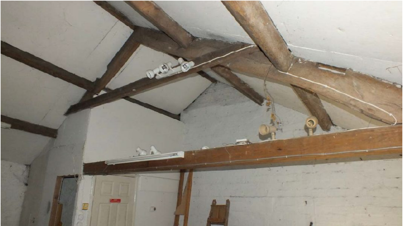
Plate 70: Truss in the disused shop (F1)
