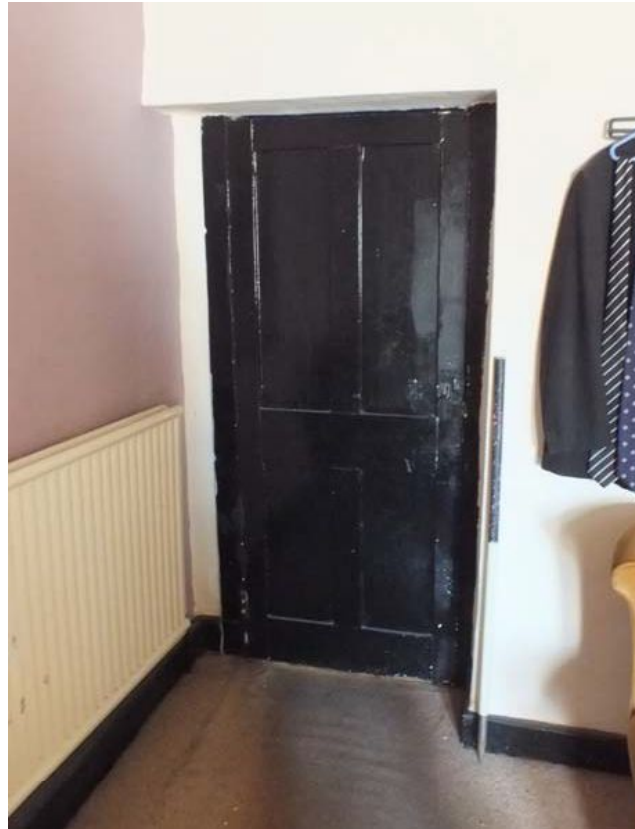
Plate 86: Detail of the raised and fielded panel door in F6
