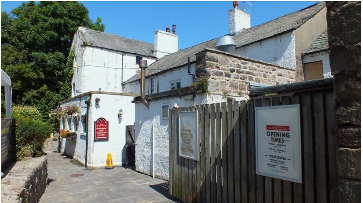
Plate 20: Flat-roofed extensions to the rear of the Royal Hotel
