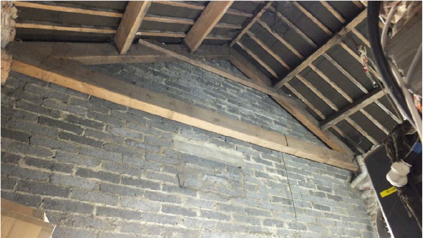
Plate 72: Truss visible on north side of F2
