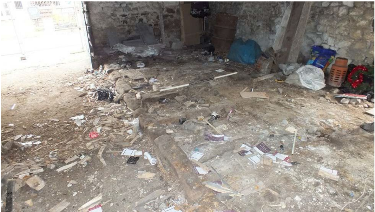
Plate 55: Raised floor on the south side of the barn
