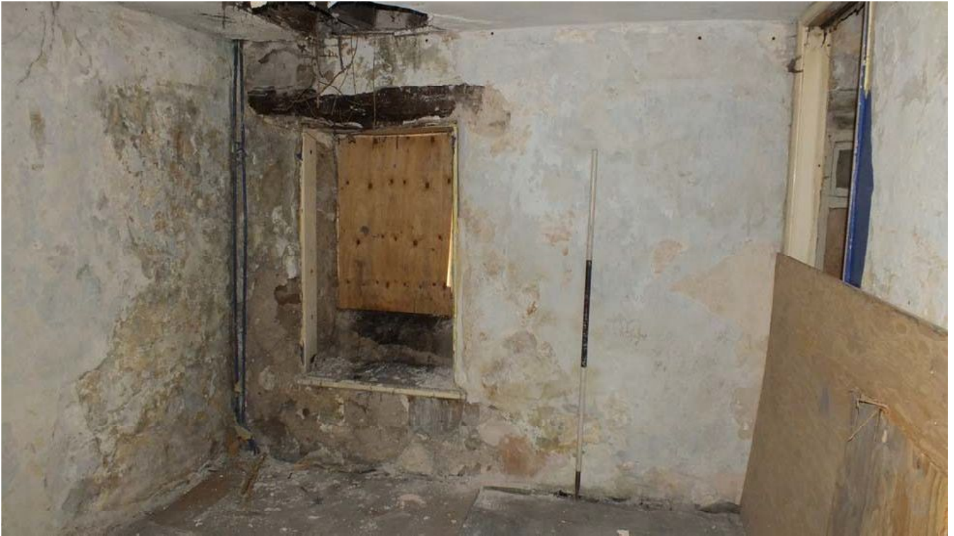
Plate 105: Window in the west elevation of Room F12
