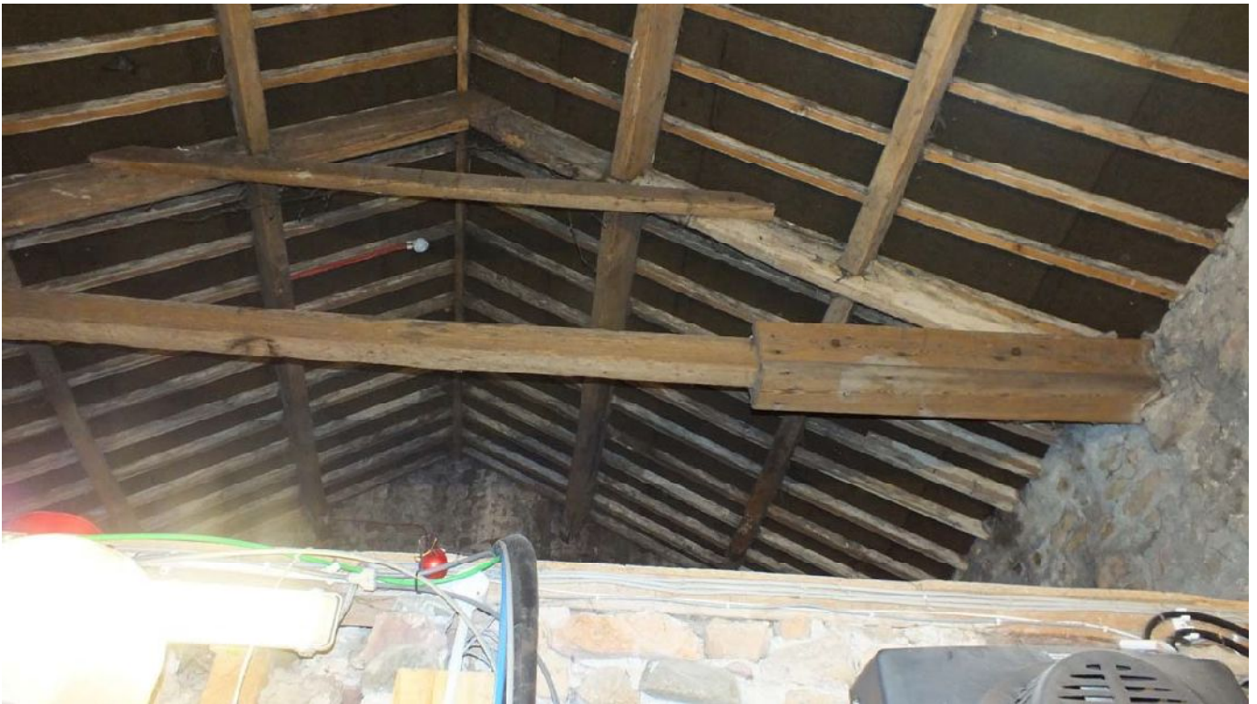
Plate 73: West end of truss visible on south side of F3
