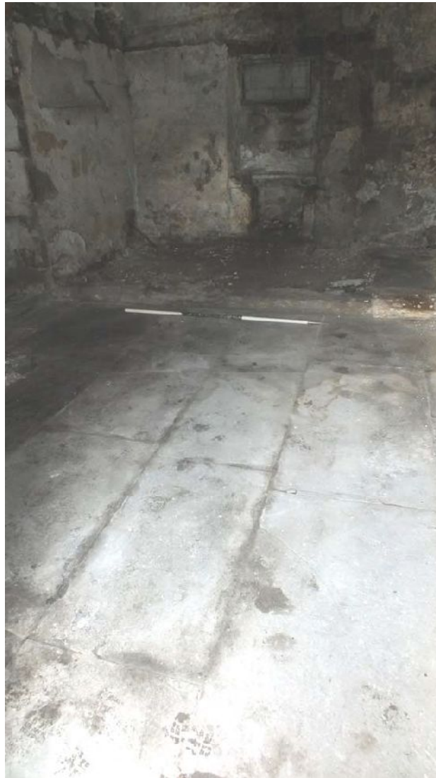
Plate 60: Flag floor in Room G14
