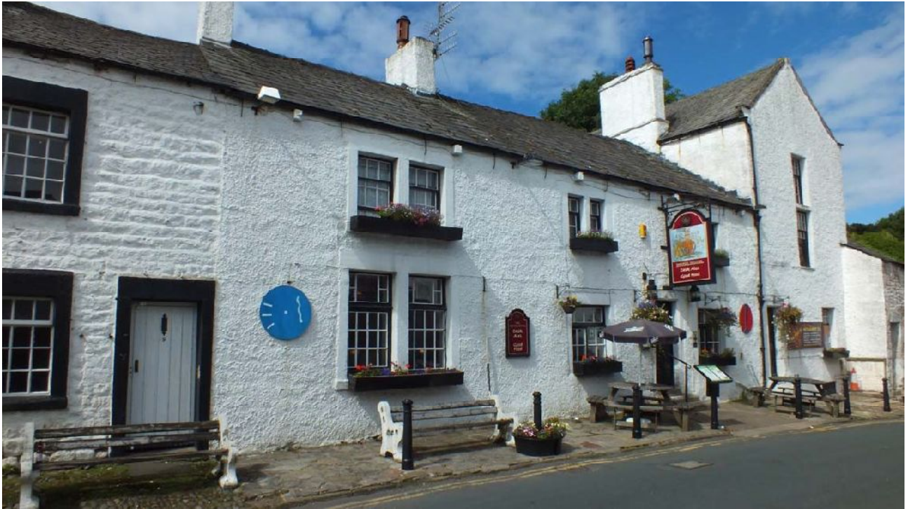
Plate 11: The east external elevation of the main building of the Royal Hotel
