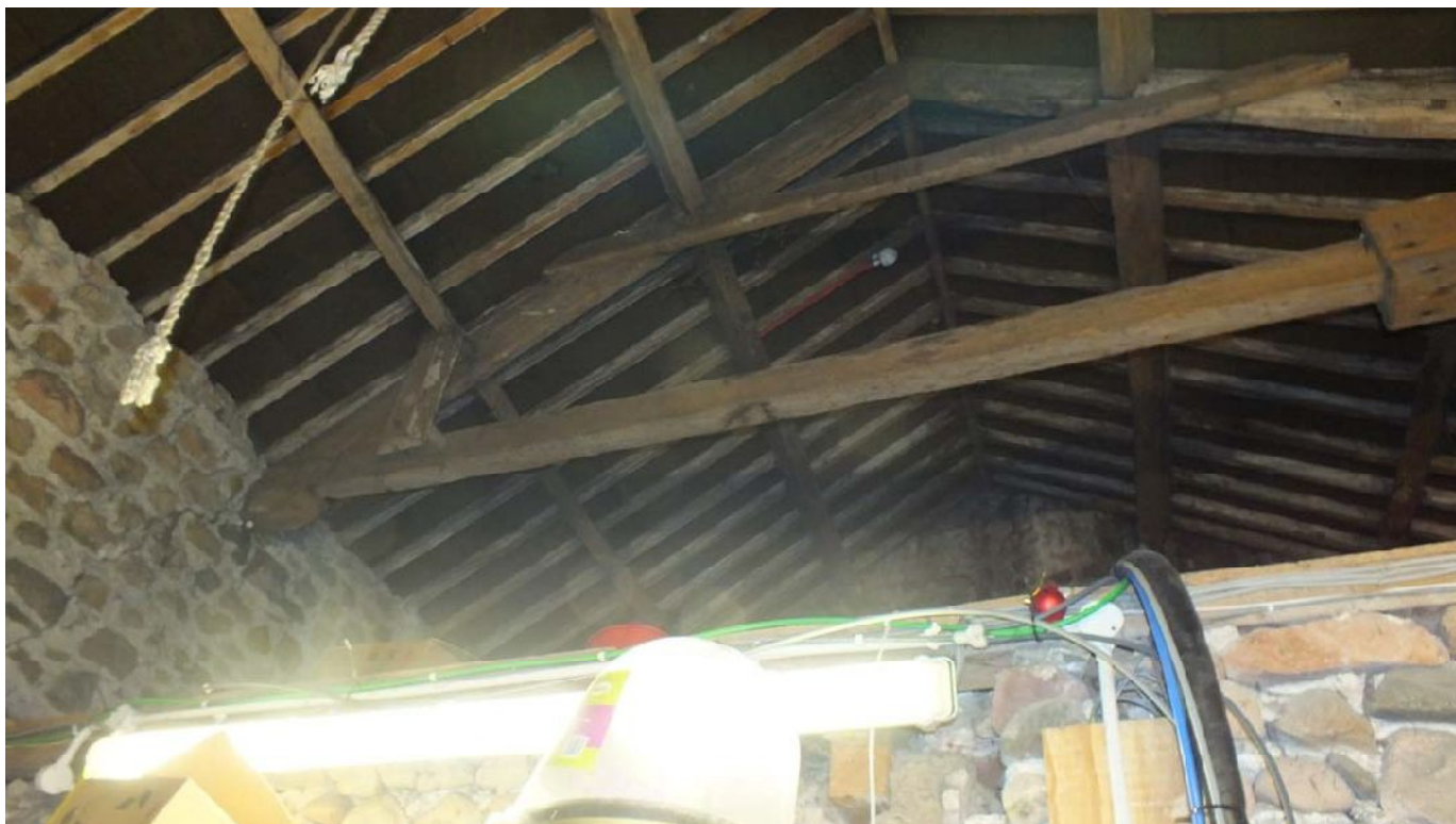
Plate 74: East end of truss visible on south side of F3
