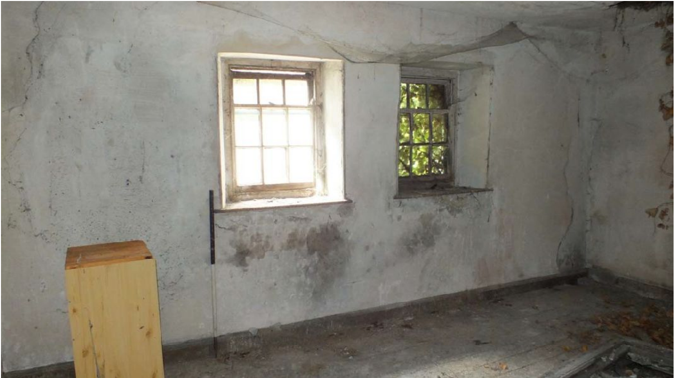
Plate 112: Windows in the west elevation of S1
