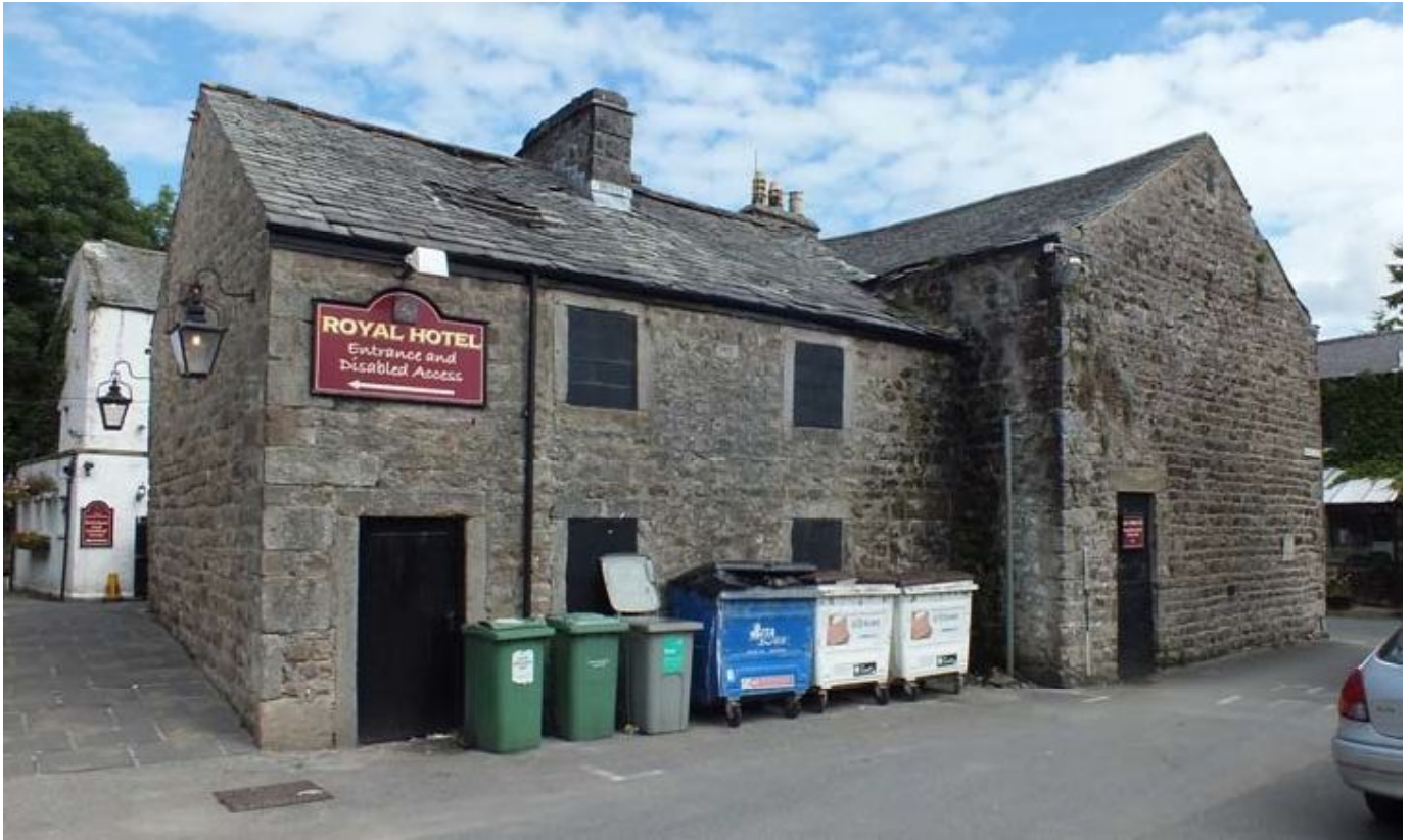
Plate 16: South external elevation viewed from the carpark
