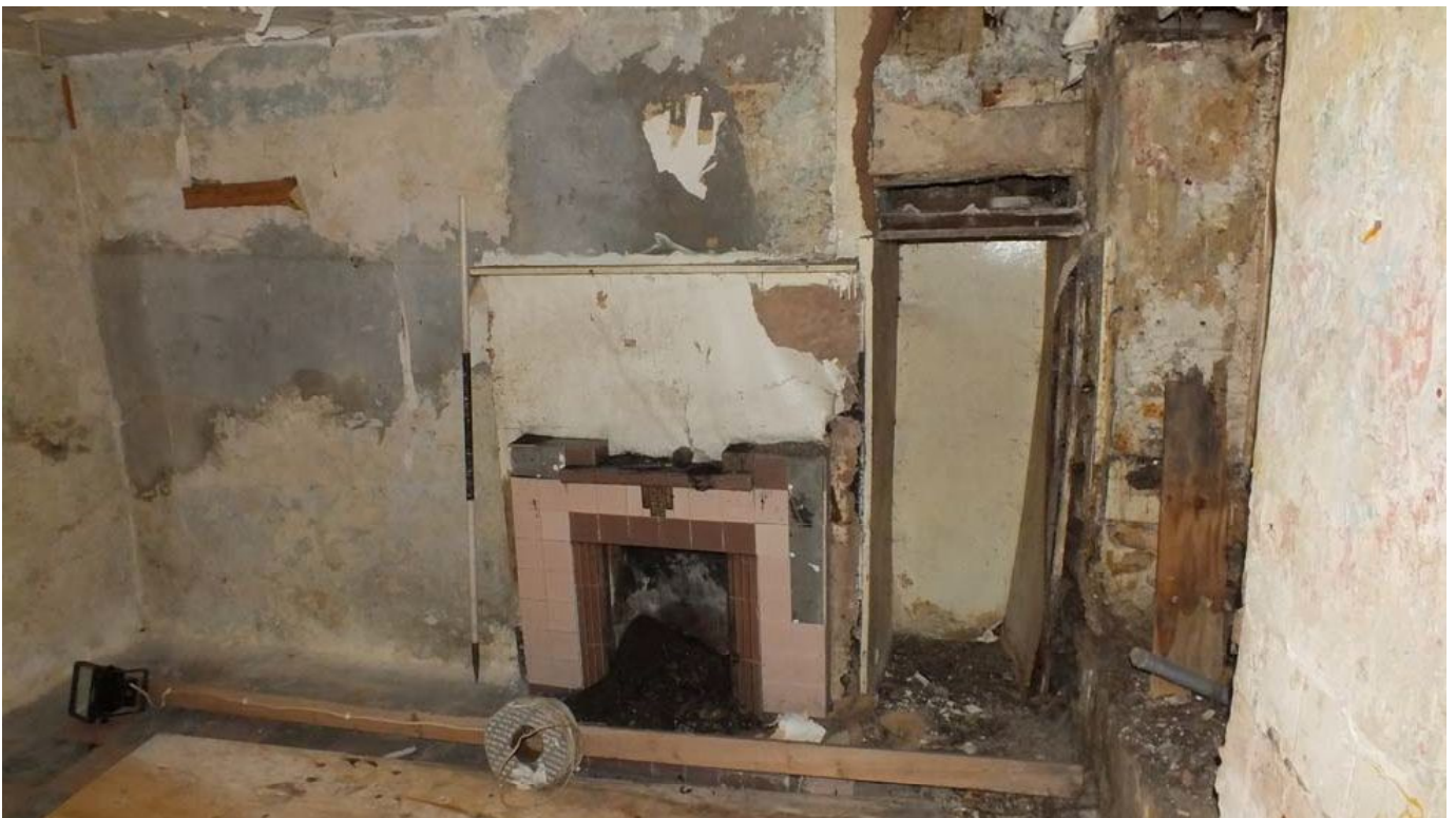
Plate 53: Fireplace and alcove, south elevation of Room G13
