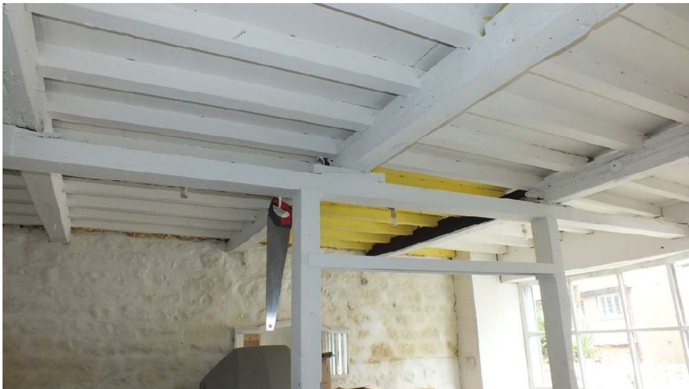
Plate 25: The ceiling of the disused shop (G1)
