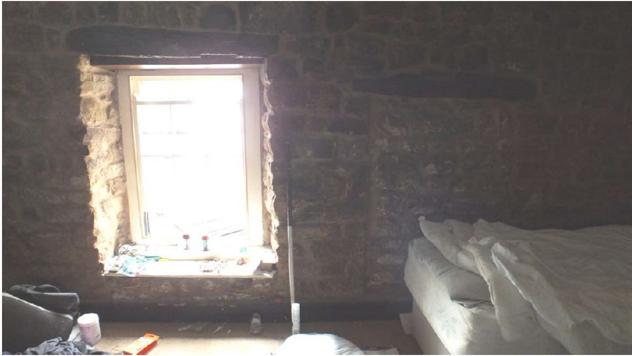
Plate 96: Sash window and blocked window in the west elevation of F10
