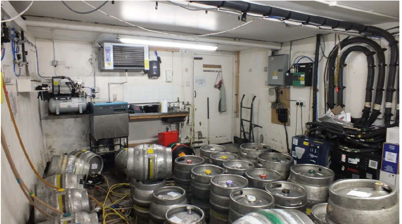
Plate 31: East elevation of G3
