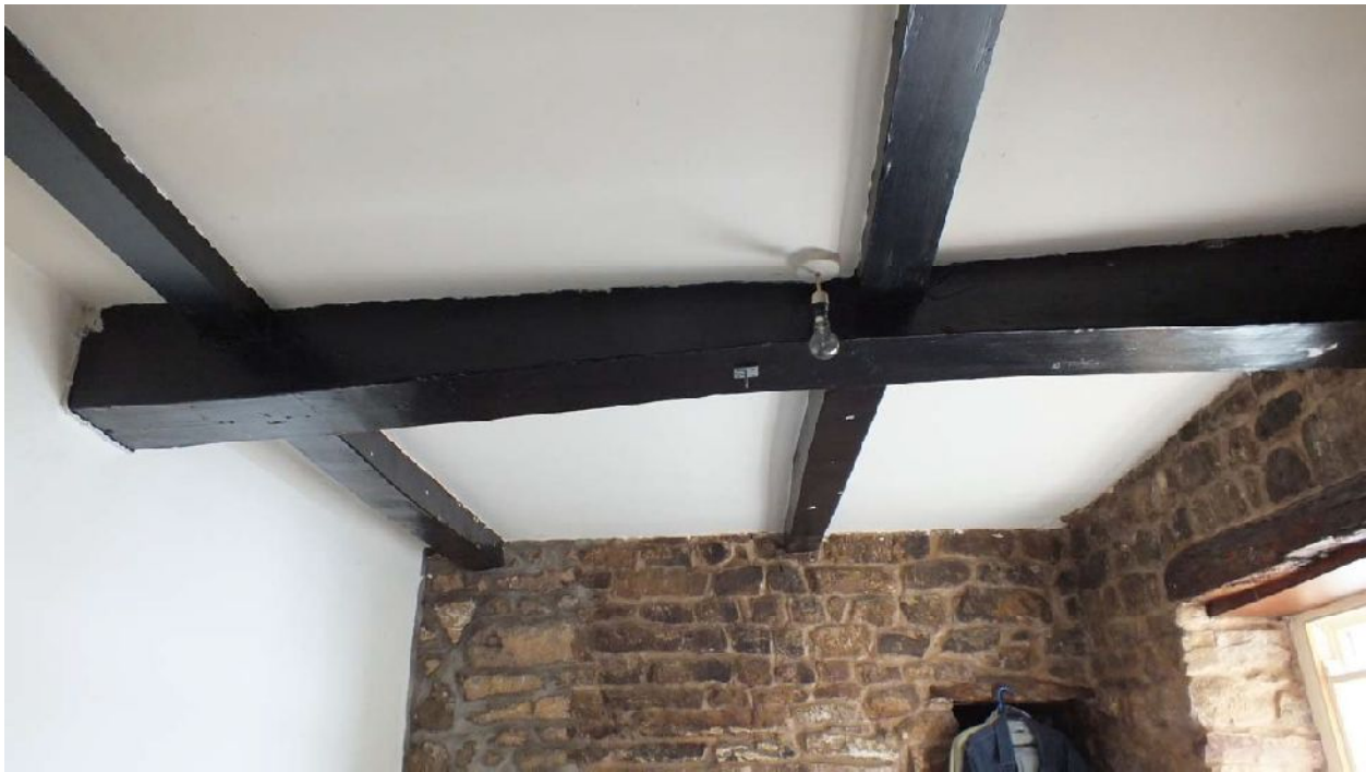
Plate 94: Beams across the ceiling in F10
