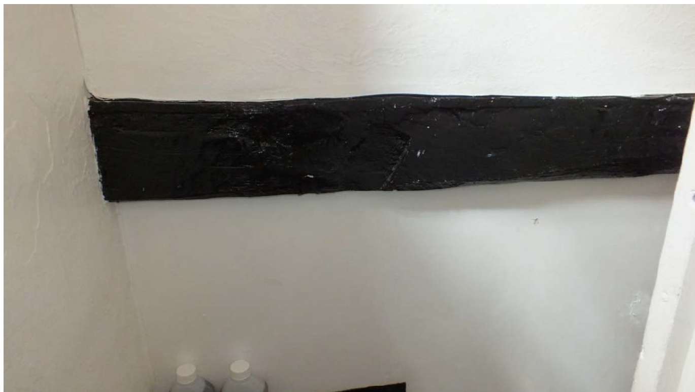
Plate 103: Reused cruck in the north wall of the stairs
