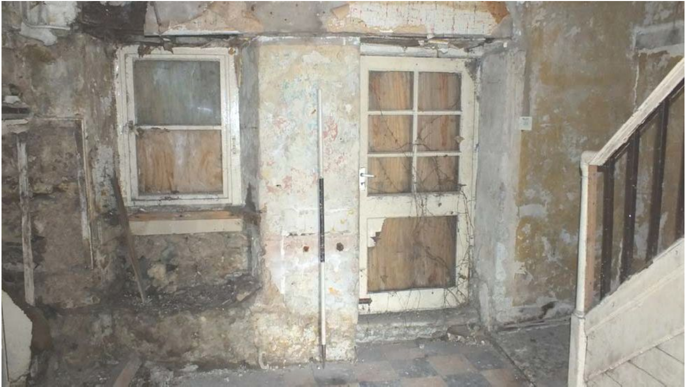
Plate 54: Window and doorway, west elevation, Room G13
