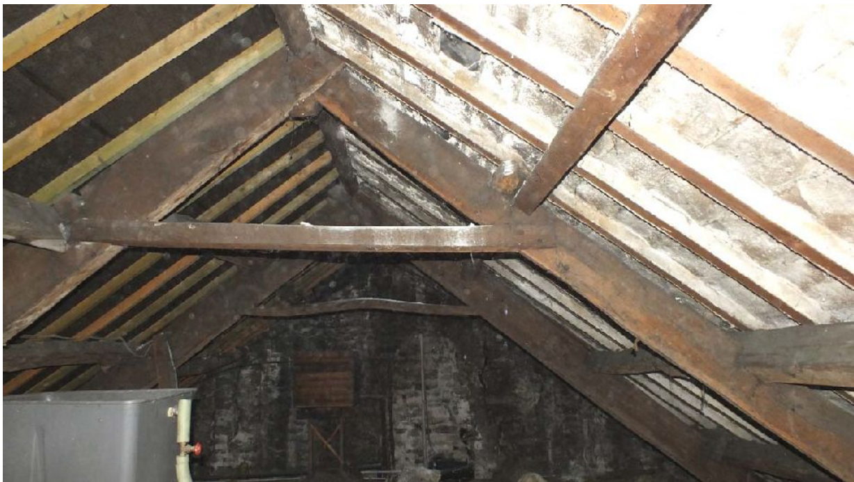
Plate 109: Trusses in the main part of the roof space
