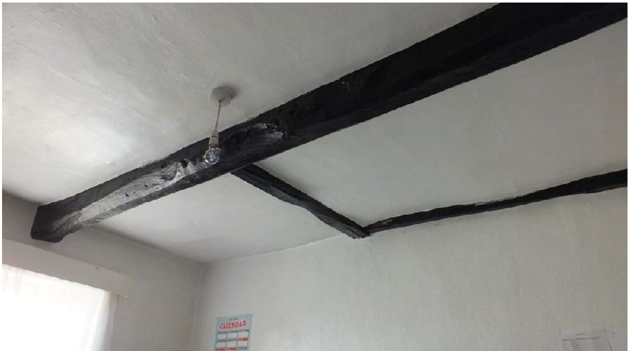
Plate 87: Beams across the ceiling in F7
