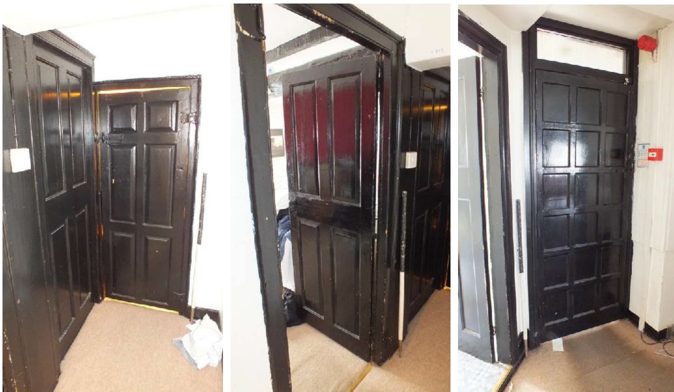
Plate 100 (left): Cupboard door and redundant door at the end of F11
