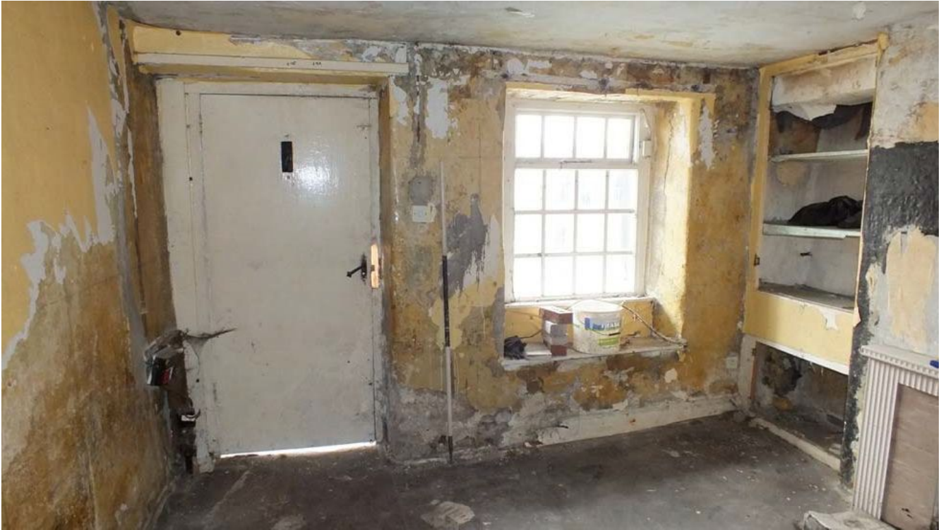
Plate 50: East elevation in Room G12
