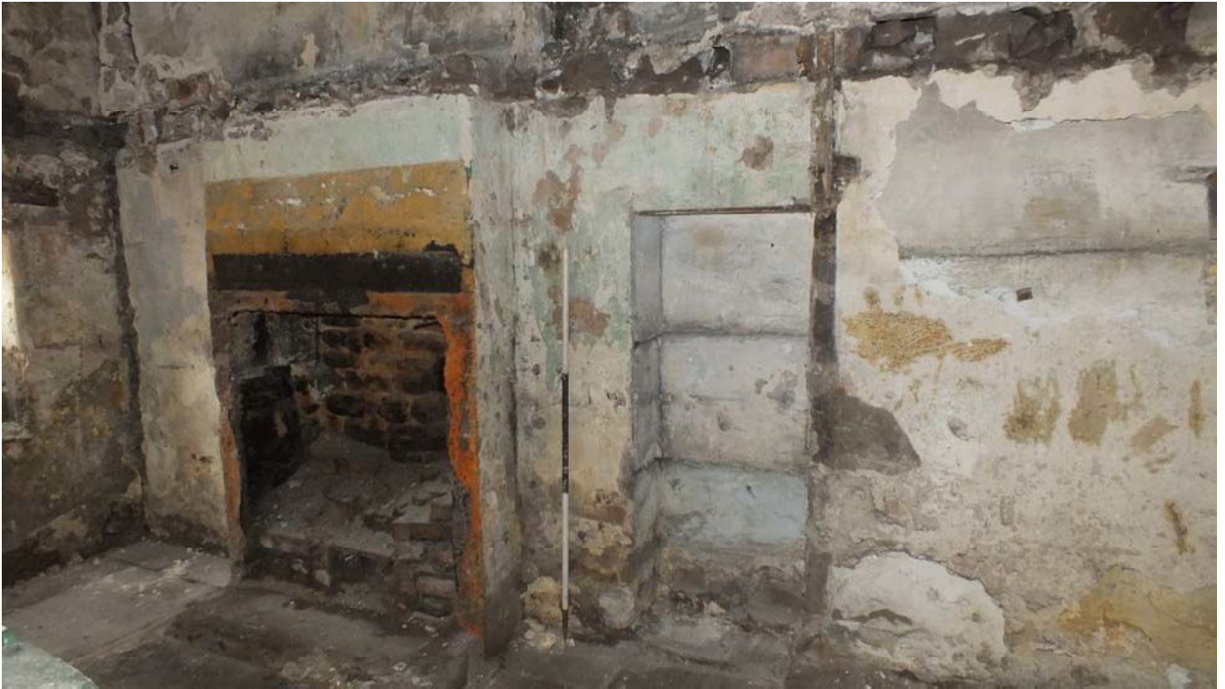
Plate 66: Fireplace and alcove, west elevation, Room G14
