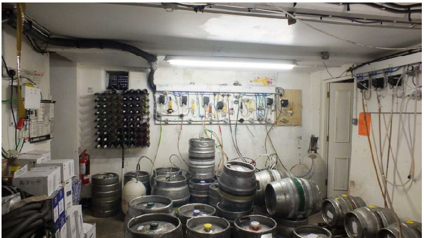
Plate 34: West elevation of G3
