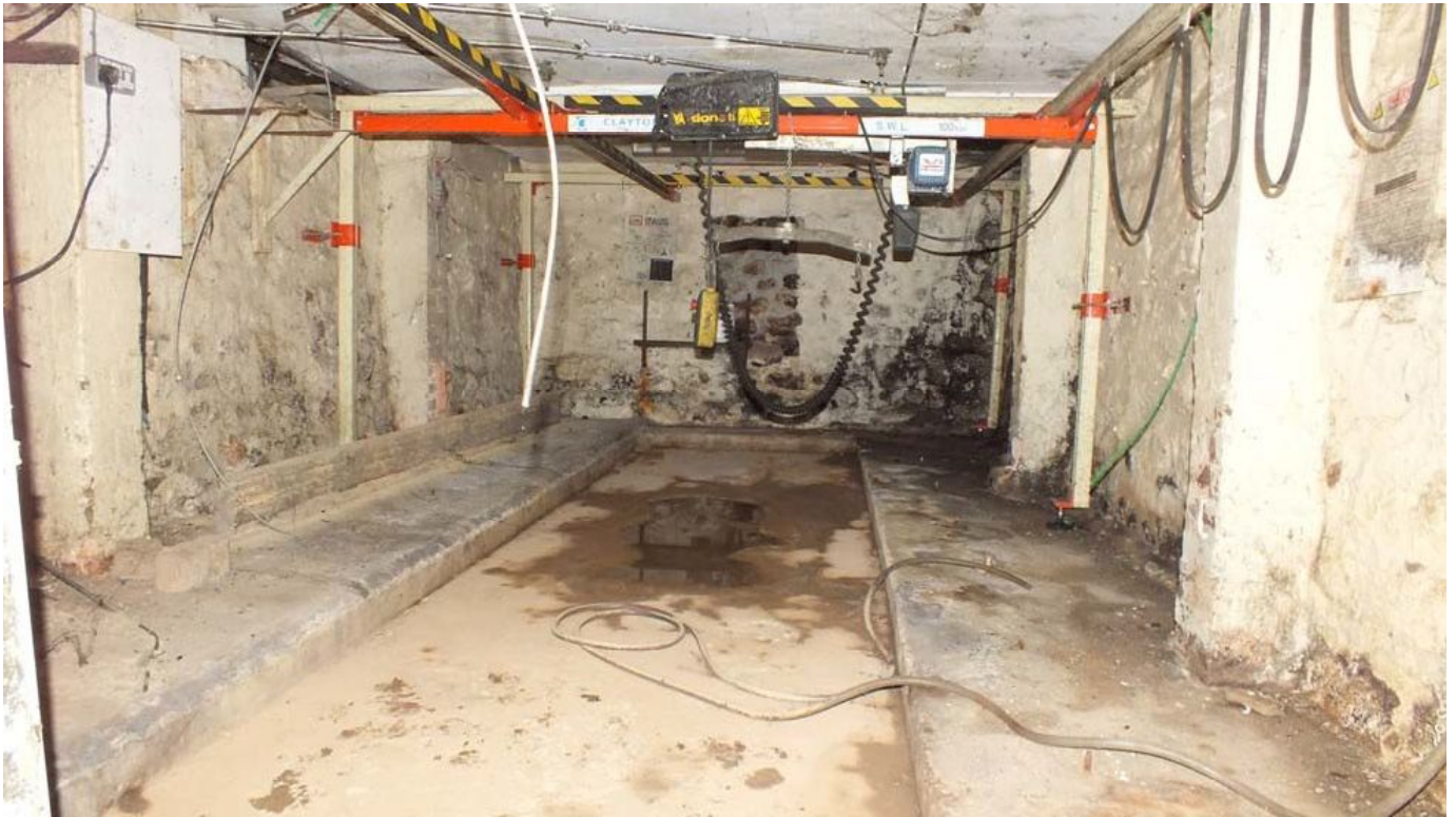
Plate 117: The west end of the cellar below Room G4
