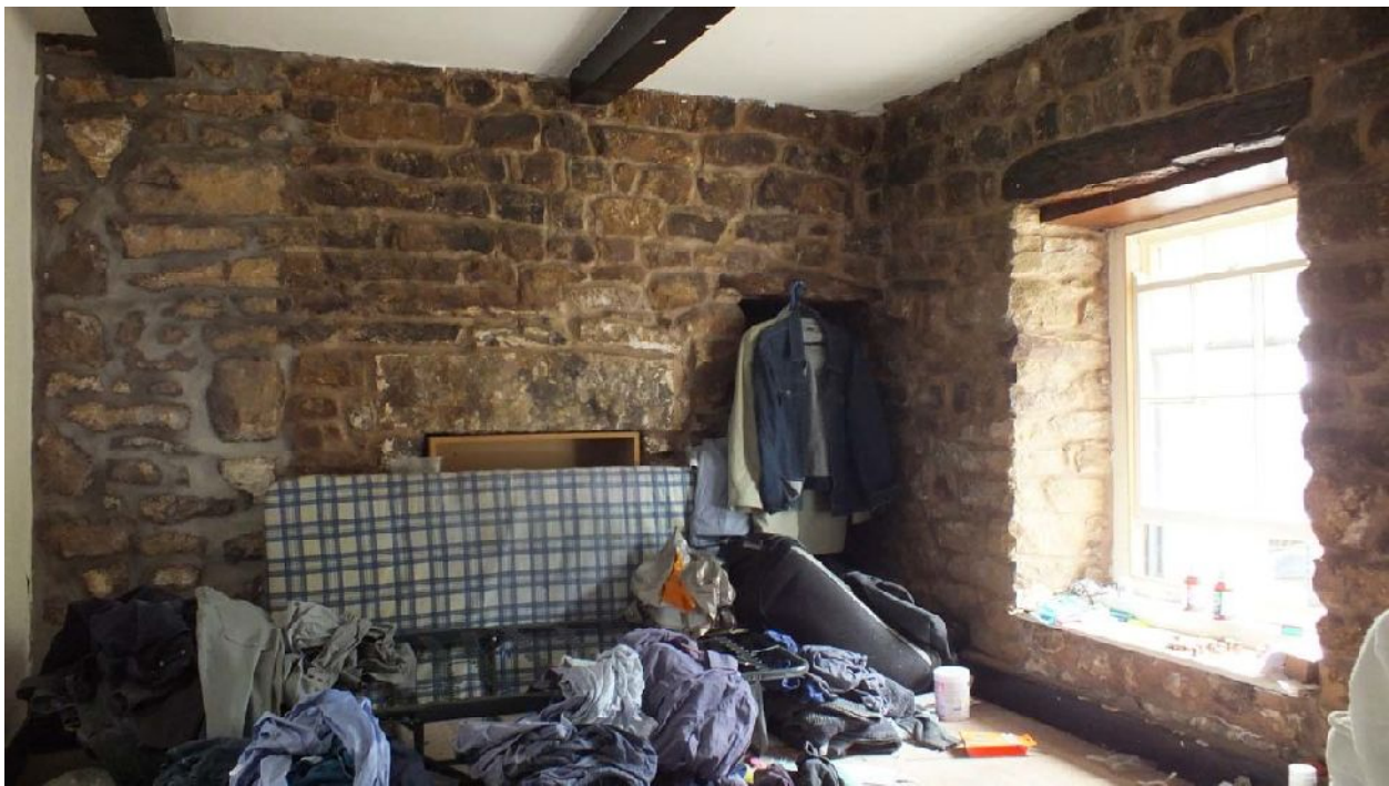
Plate 95: The south and west elevations of F10
