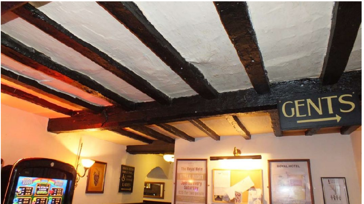
Plate 37: Beams in the ceiling at the north end of G5
