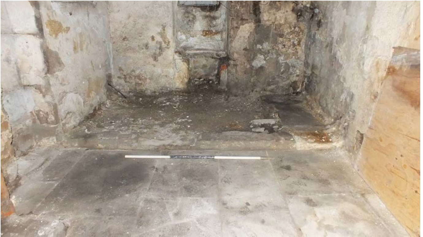
Plate 61: Raised floor on the north side of Room G14
