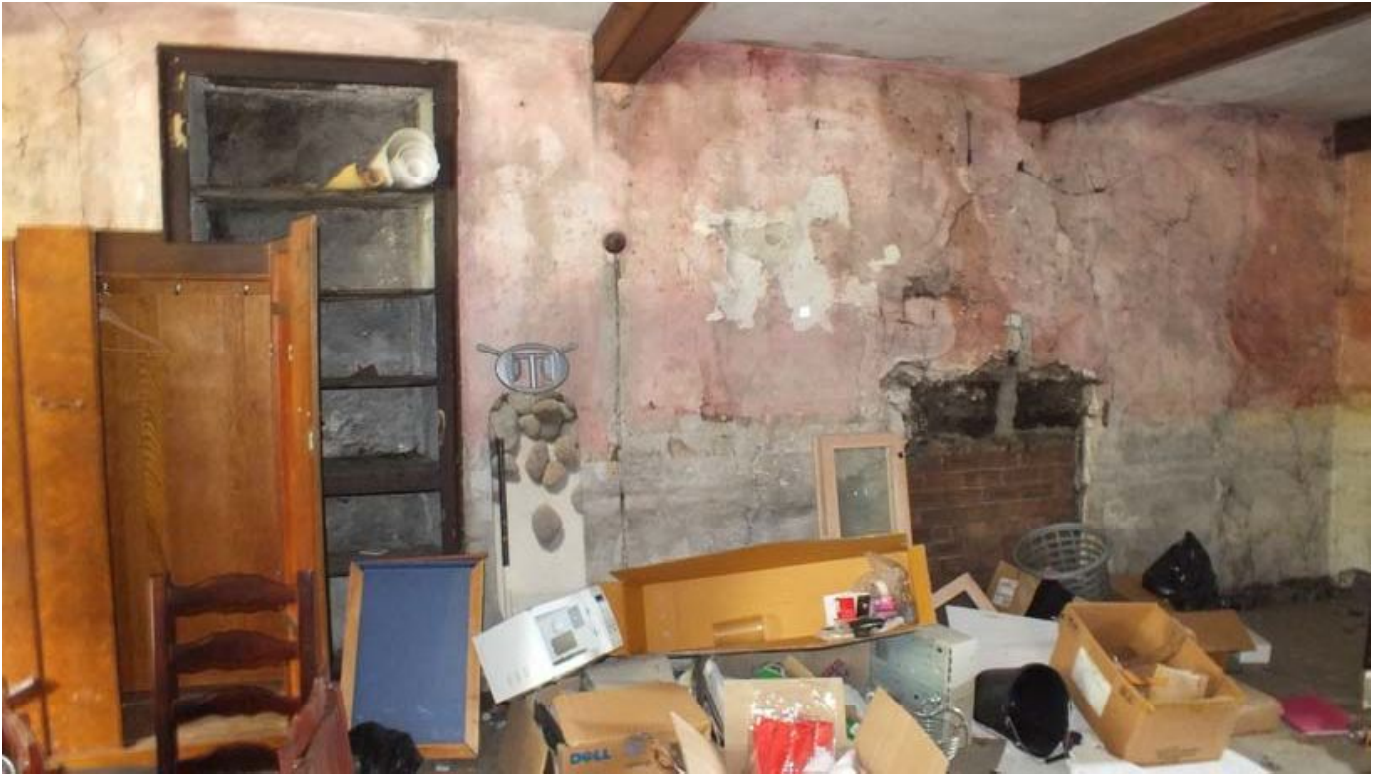
Plate 77: The north end of the west elevation of F4
