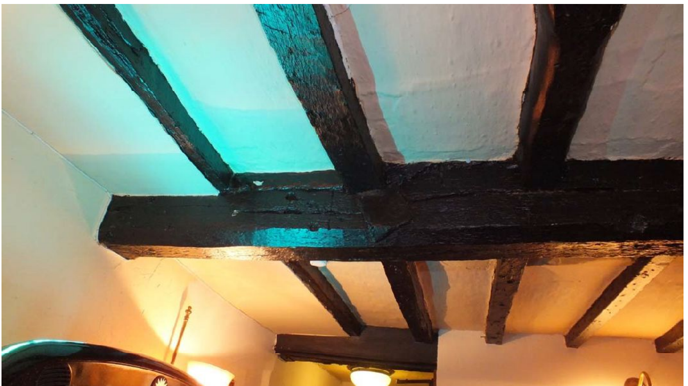
Plate 38: Detail of reused beams in the ceiling of G5
