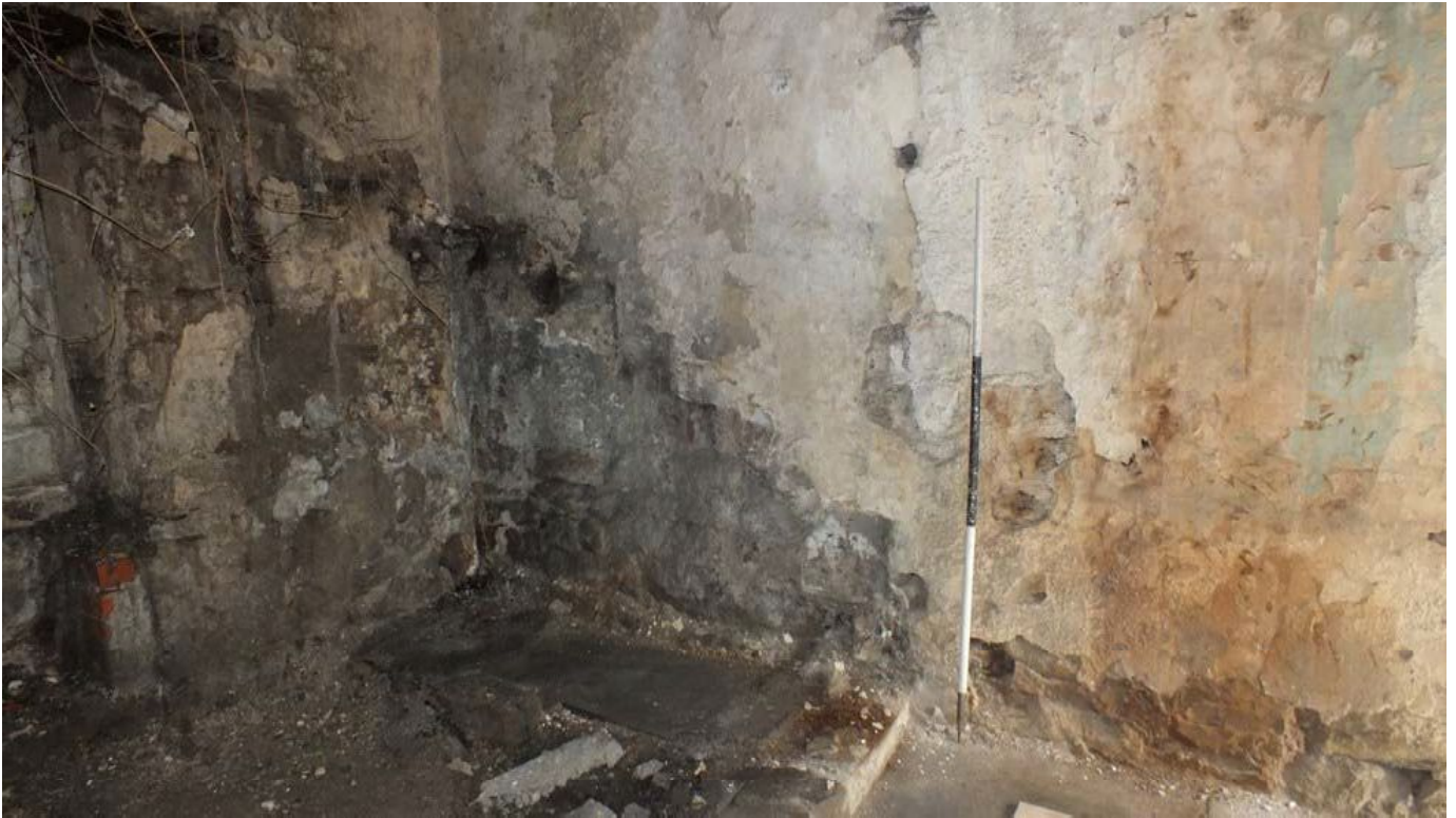
Plate 63: Scar of former staircase in the north-east corner of Room G14
