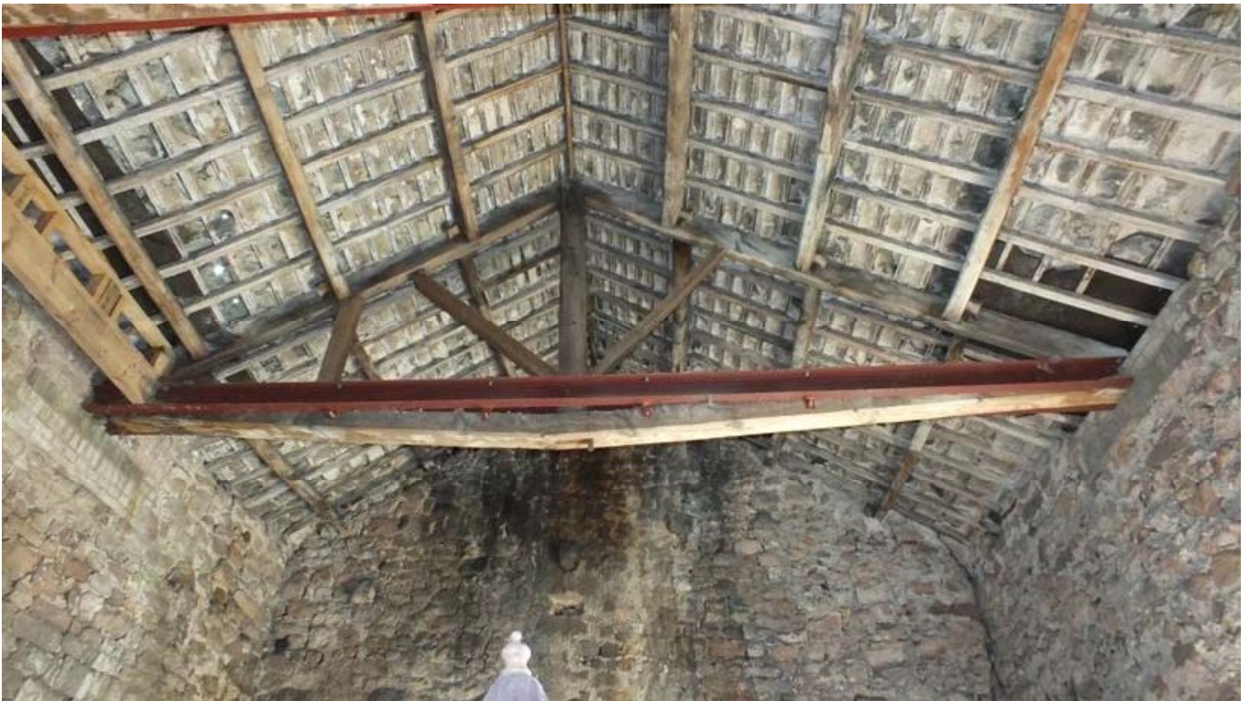
Plate 110: Truss in the barn
