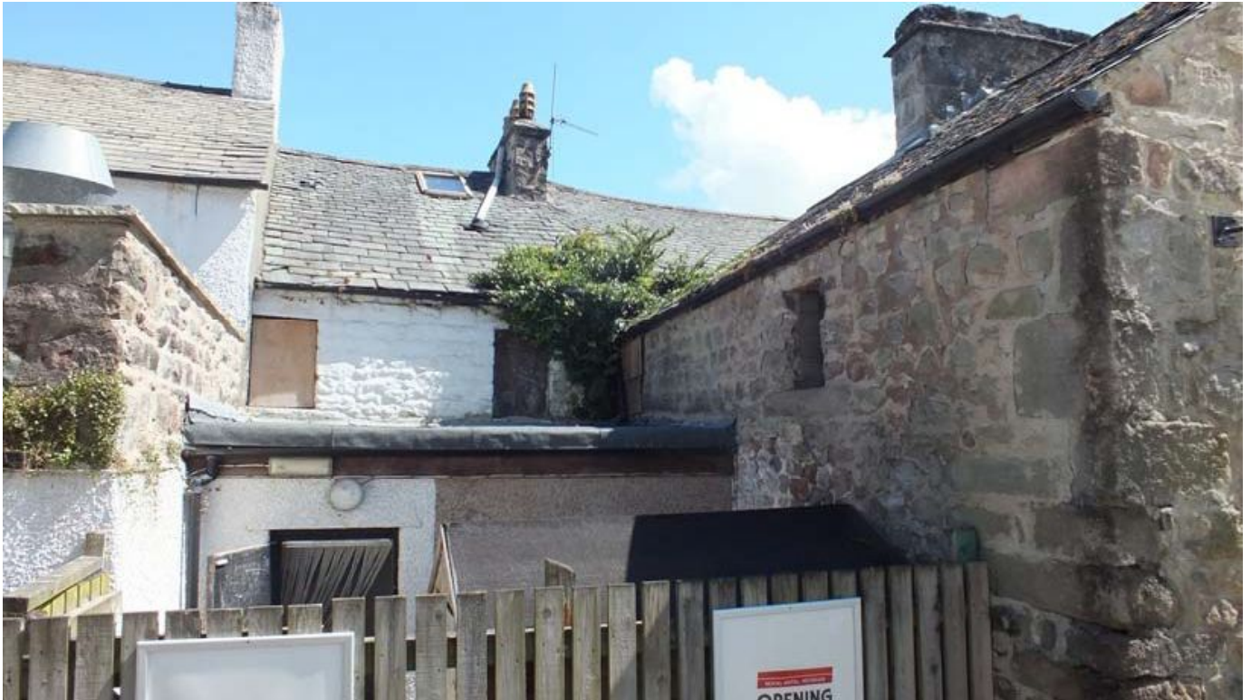
Plate 19: The rear of the cottage (2) facing onto Main Street
