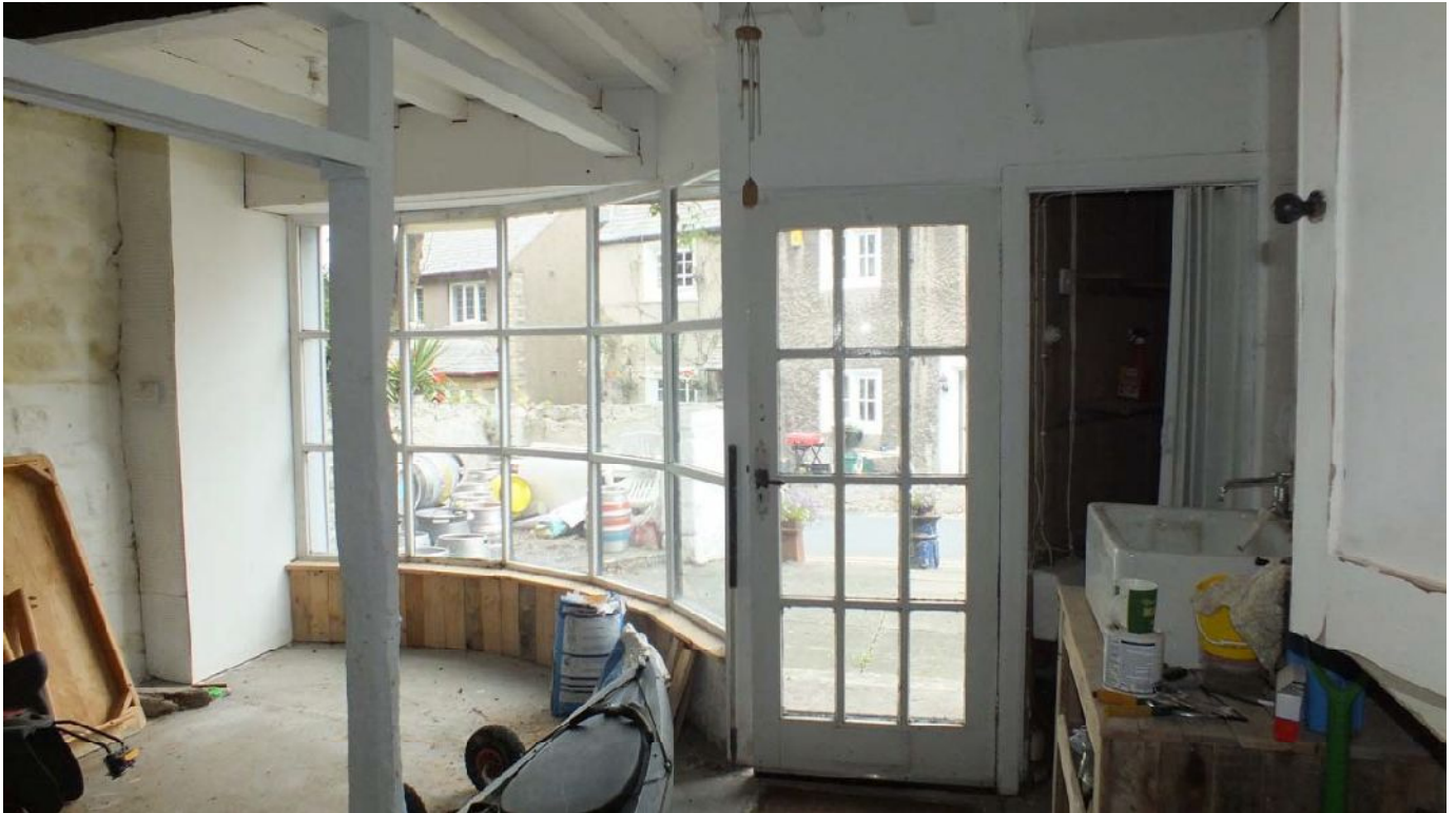
Plate 27: The east elevation of G1
