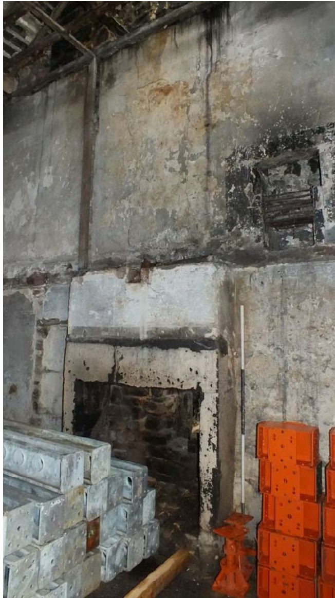
Plate 69: East elevation, Room G15
