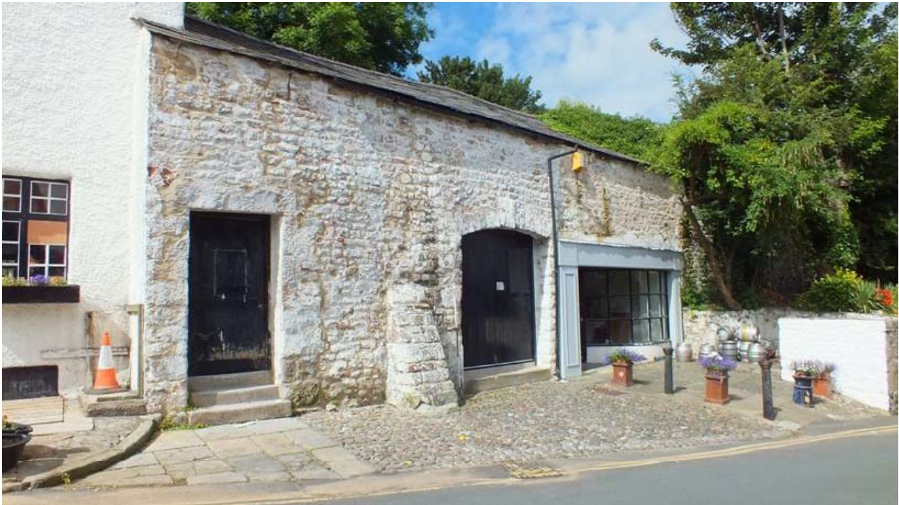
Plate 7: The north end of the east external elevation
