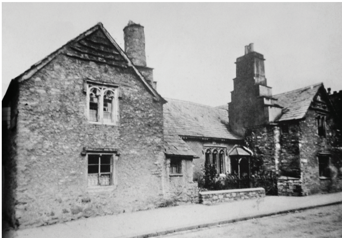
Plate 19: Early photograph (reproduced from Nicholls and Hughes 2006, 53)
