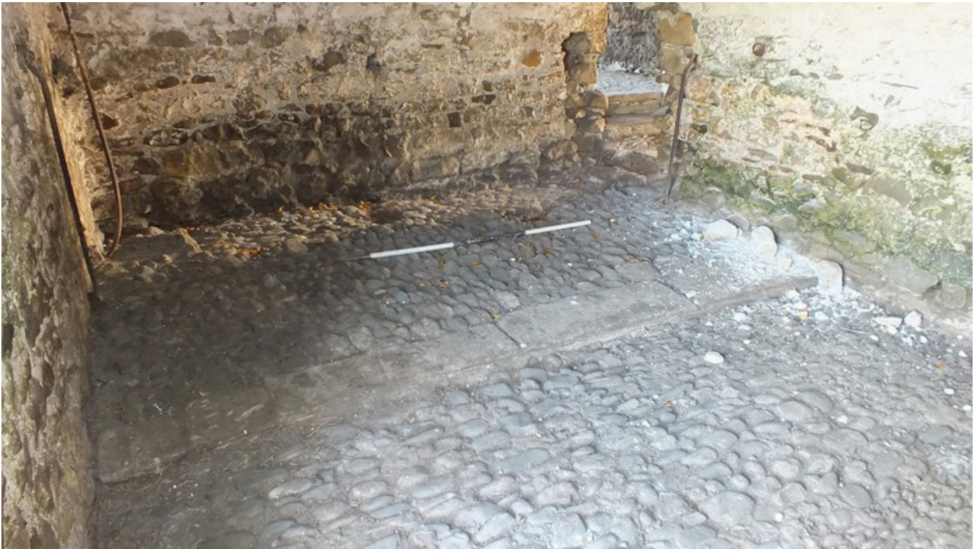
Plate 33: The floor on the east side of Room G3, viewed from the north-west
