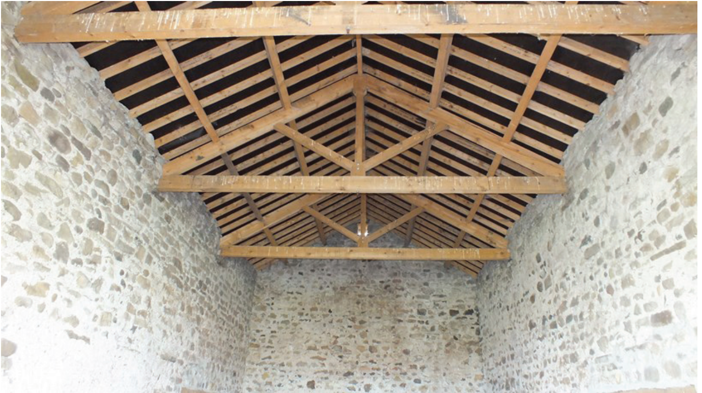
Plate 28: The roof trusses in Room G2, viewed from the north
