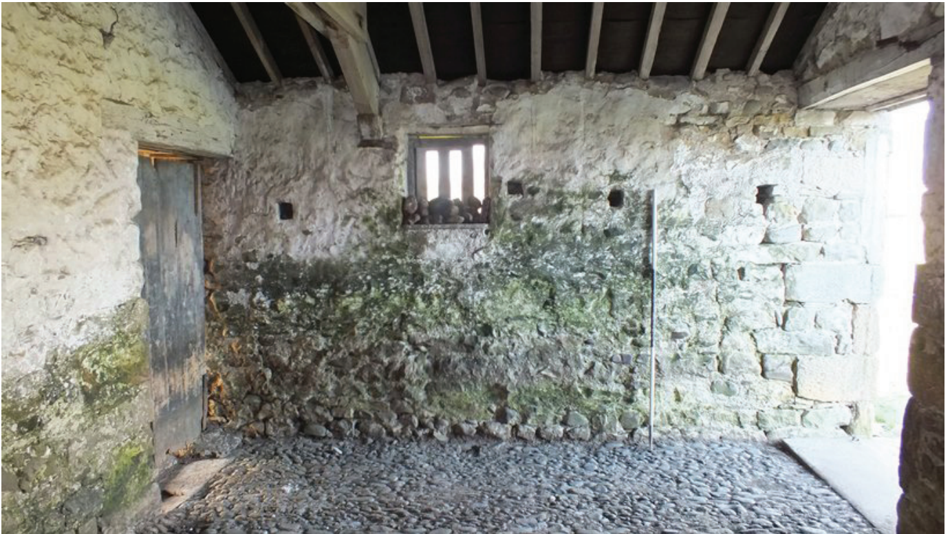
Plate 39: The west internal elevation of Room G3, viewed from the east
