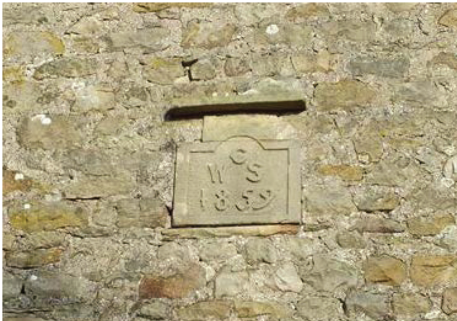
Plate 16: The datestone in the south external elevation, viewed from the south
