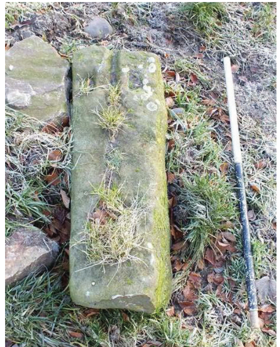
Plate 7 (left): Chamfered lintel re-used in the boundary wall to the south-east of the building, viewed from the west
