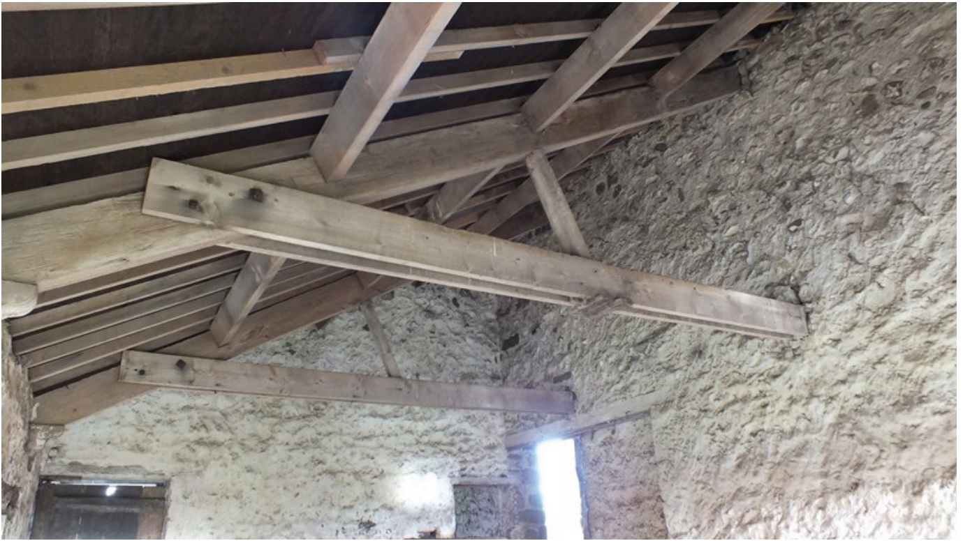
Plate 42: Trusses in Room G4, viewed from the south-west
