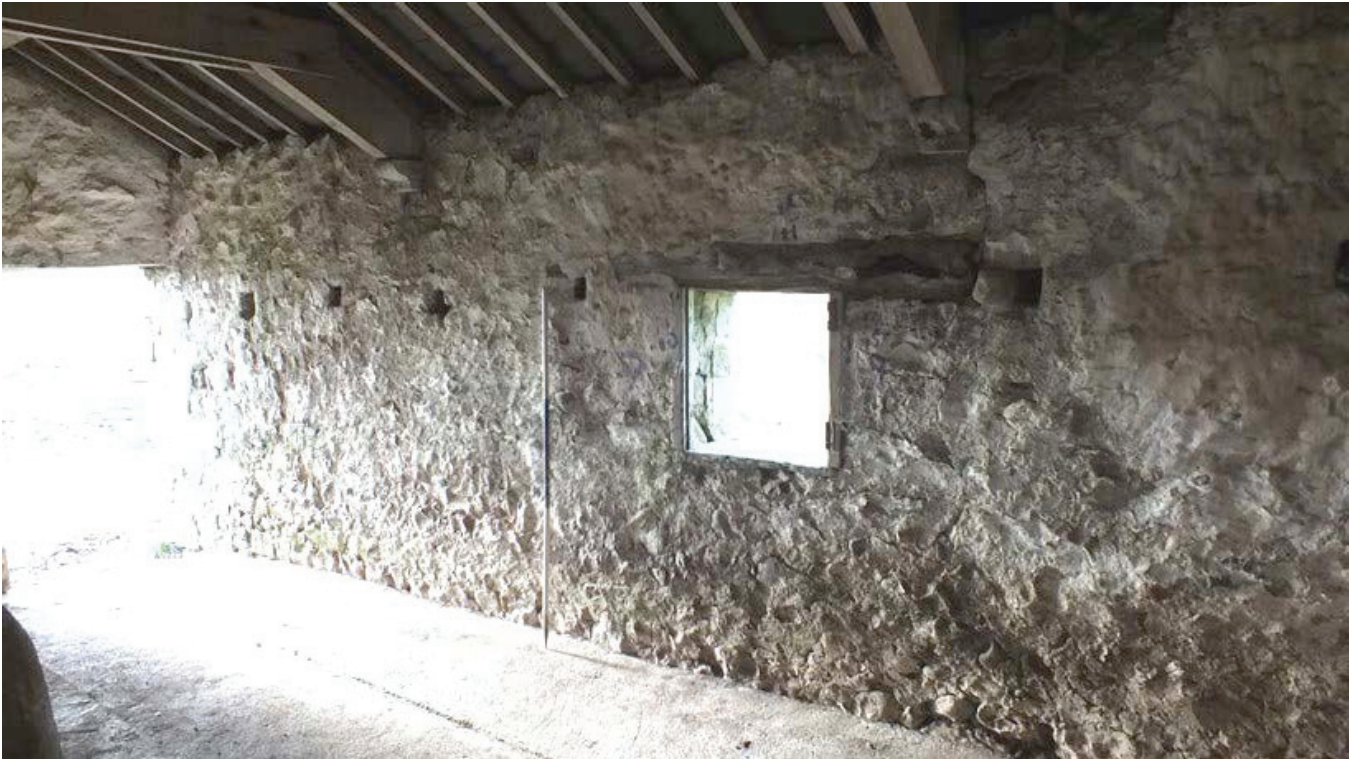
Plate 48: The west internal elevation of Room G4, viewed from the north-east
