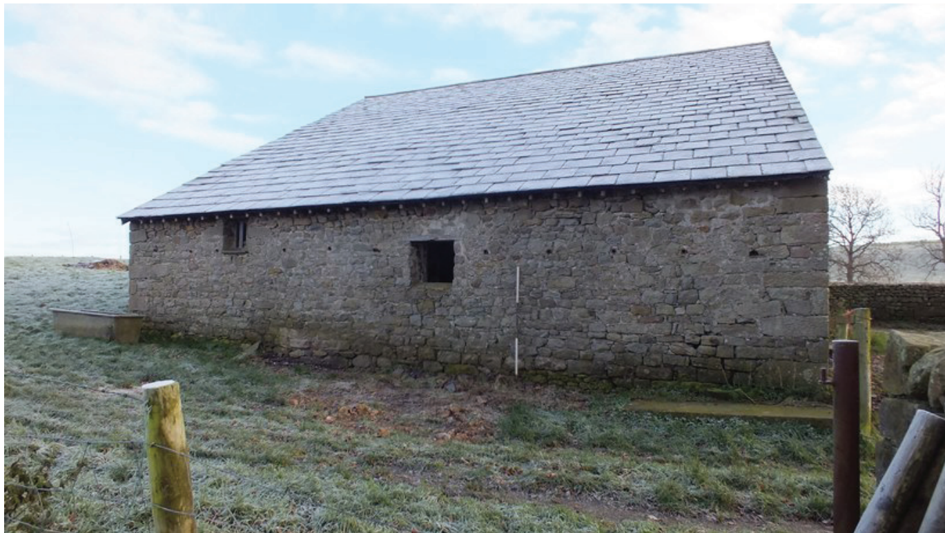
Plate 17: The west external elevation, viewed from the south-west
