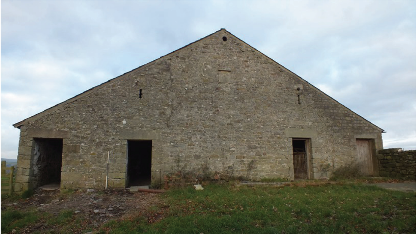
Plate 15: The south external elevation, viewed from the south
