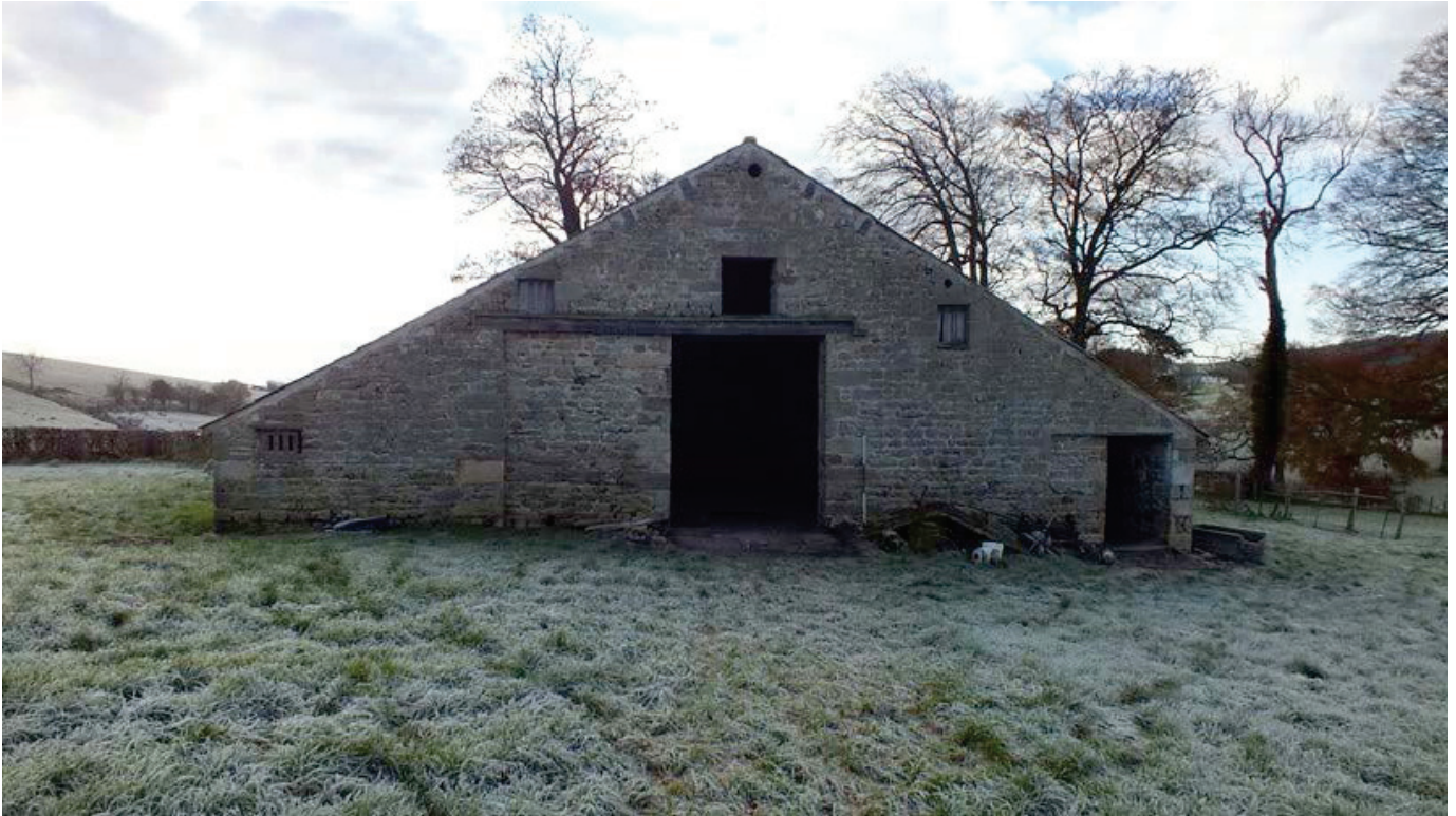
Plate 9: The north external elevation, viewed from the north
