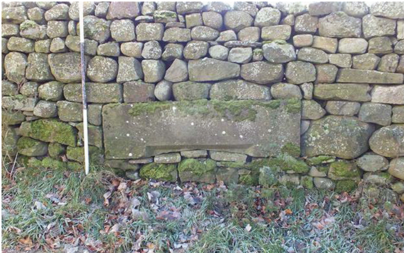
Plate 7 (left): Chamfered lintel re-used in the boundary wall to the south-east of the building, viewed from the west
