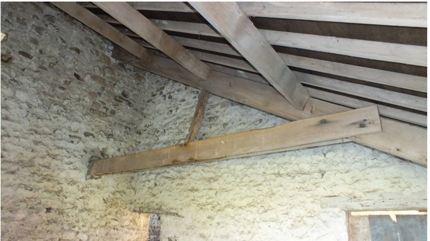
Plate 34: Truss in Room G3
