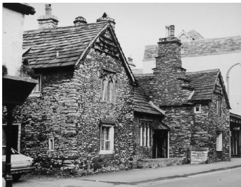
Plate 24: Photograph of the Castle Dairy taken from the south (CAC(K) WDX 1248 c1960s)
