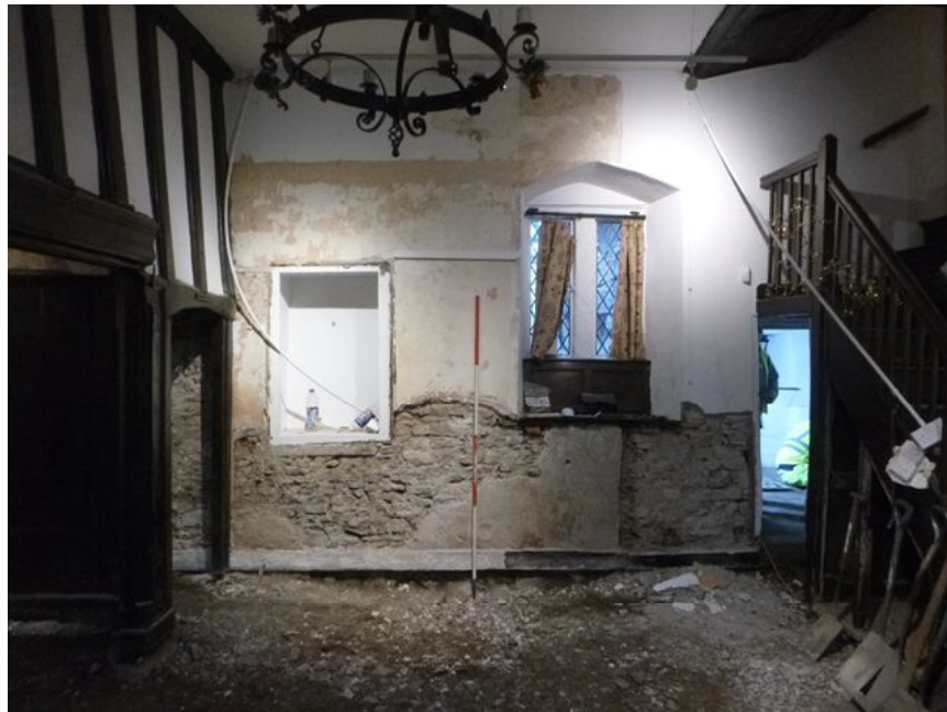
Plate 36 (left): Plaster removed along the side of the corridor in G2
