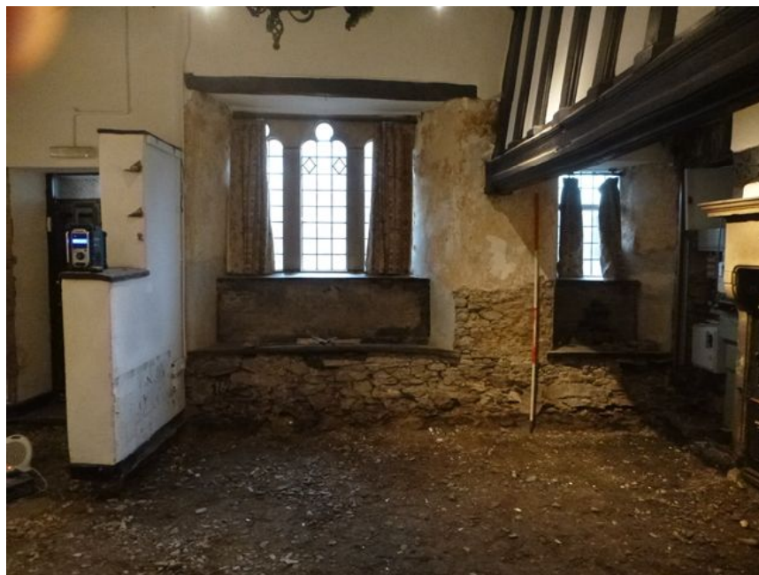
Plate 38: Areas of plaster removed from the south-east elevation of G2
