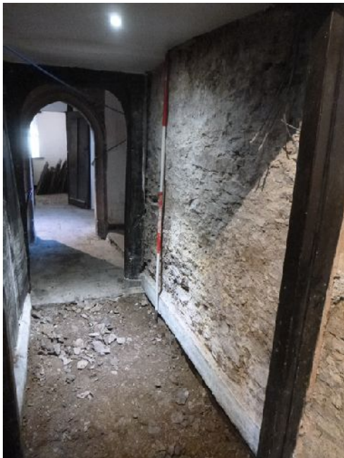
Plate 36 (left): Plaster removed along the side of the corridor in G2
