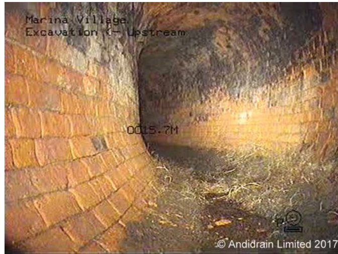
Plate 17: General view inside the flue
