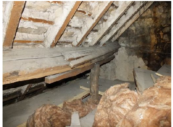
Plate 14 (left): The north-east end of the north-west purlin showing empty slots, viewed from the west
