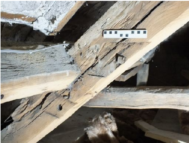
Plate 18 (left): Detail of the empty slots at the south-east end of the truss, viewed from the north-east
