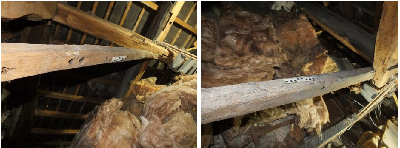
Plate 22 (left): The underside of the collar showing empty peg holes, viewed from the south-east
