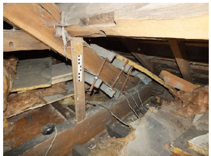
Plate 20 (left): Detail of the empty slot at the north-west end of the truss, viewed from the north-east
