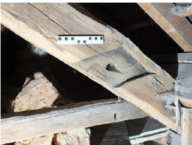
Plate 20 (left): Detail of the empty slot at the north-west end of the truss, viewed from the north-east
