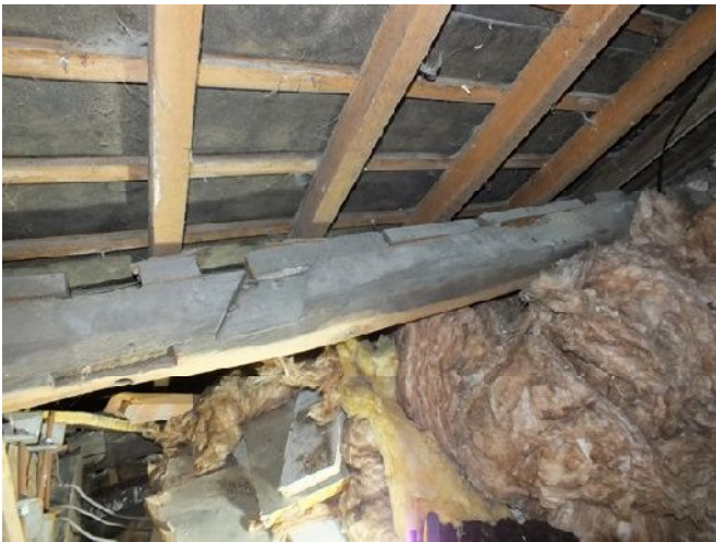
Plate 14 (left): The north-east end of the north-west purlin showing empty slots, viewed from the west
