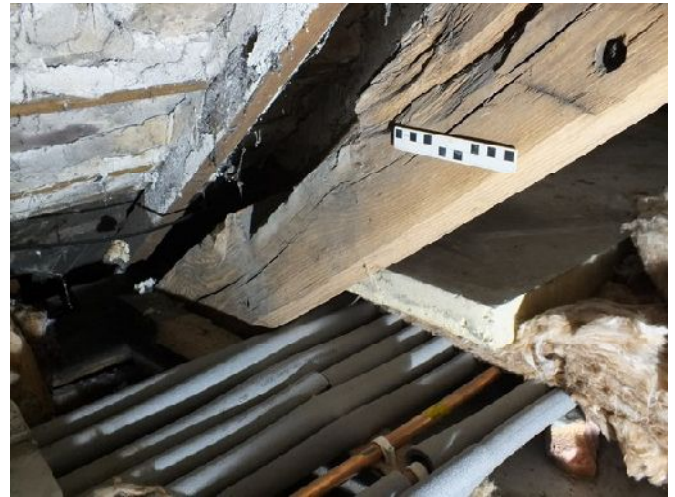
Plate 18 (left): Detail of the empty slots at the south-east end of the truss, viewed from the north-east
