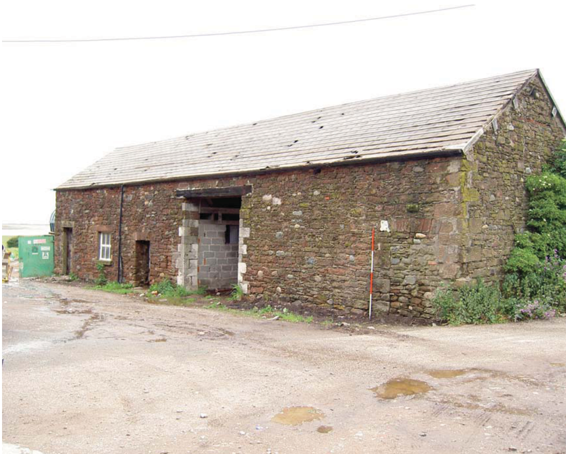
Plate 6: Building 2, from the south
