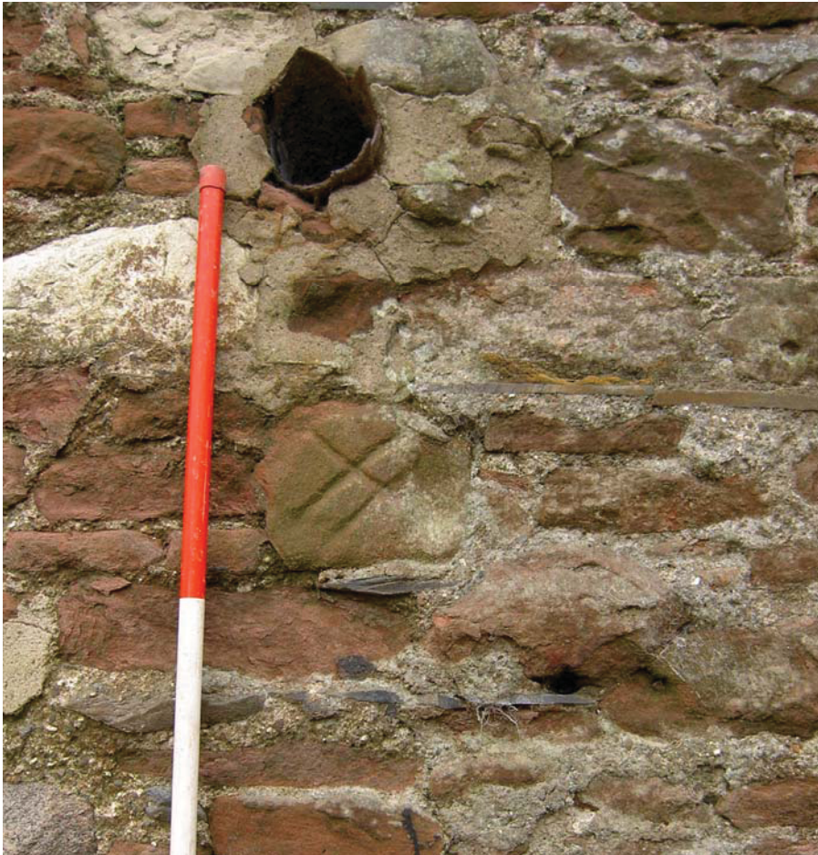
Plate 13: Marked stone in the north-north-east elevation of Building 5
