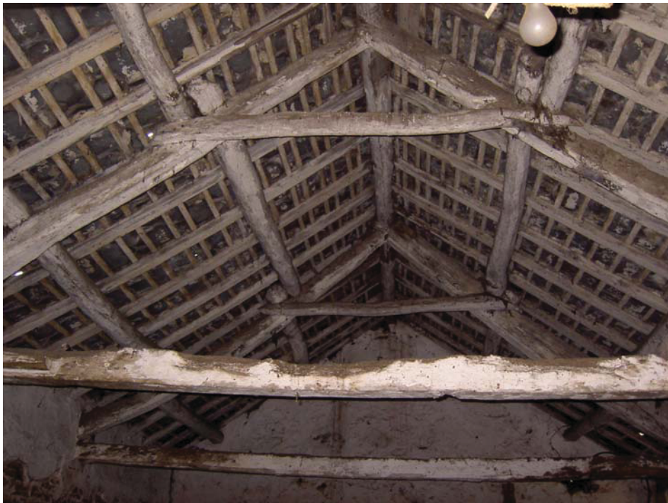
Plate 14: Collared trusses in south-east end of Building 1, looking south-east
