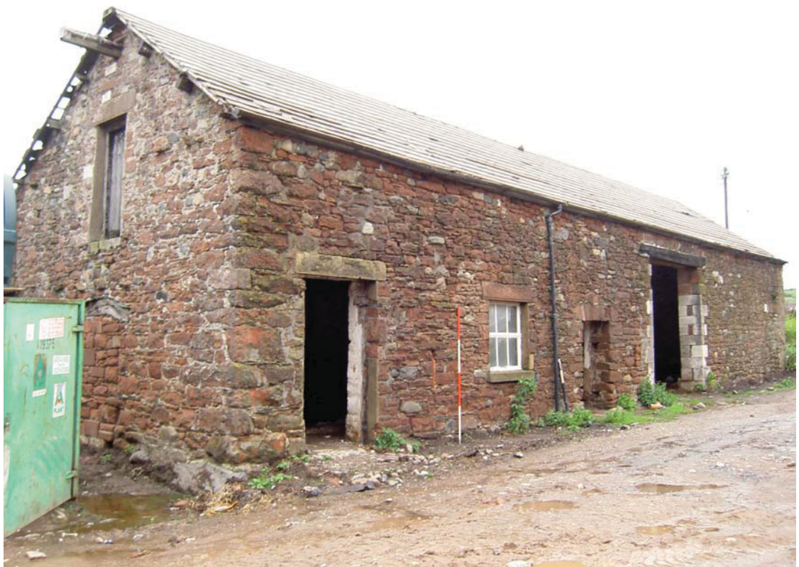
Plate 10: Building 2, from the west
