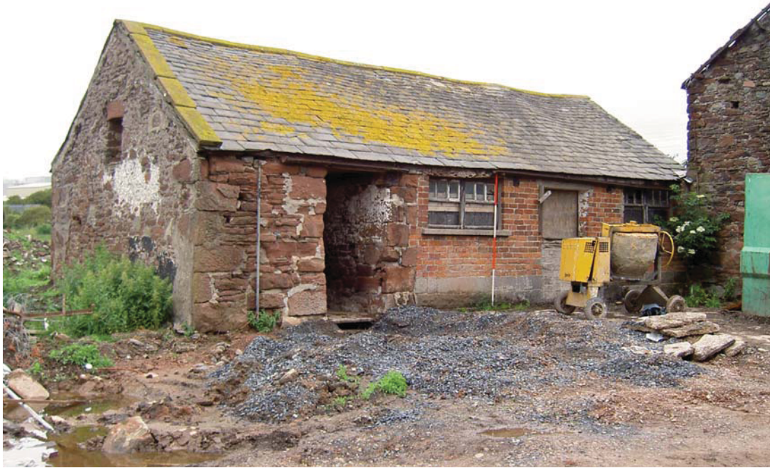
Plate 5: Building 1, from the west
