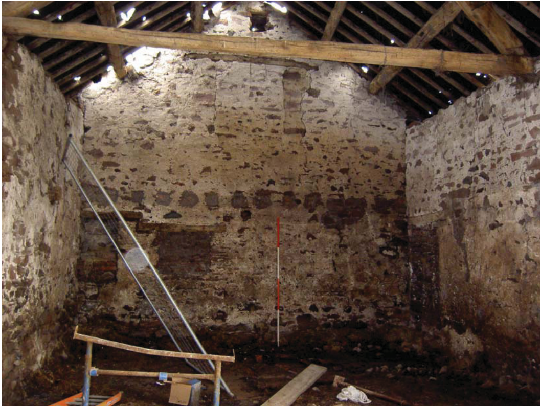
Plate 15: Evidence of half loft and blocking in south-east end of Building 2
