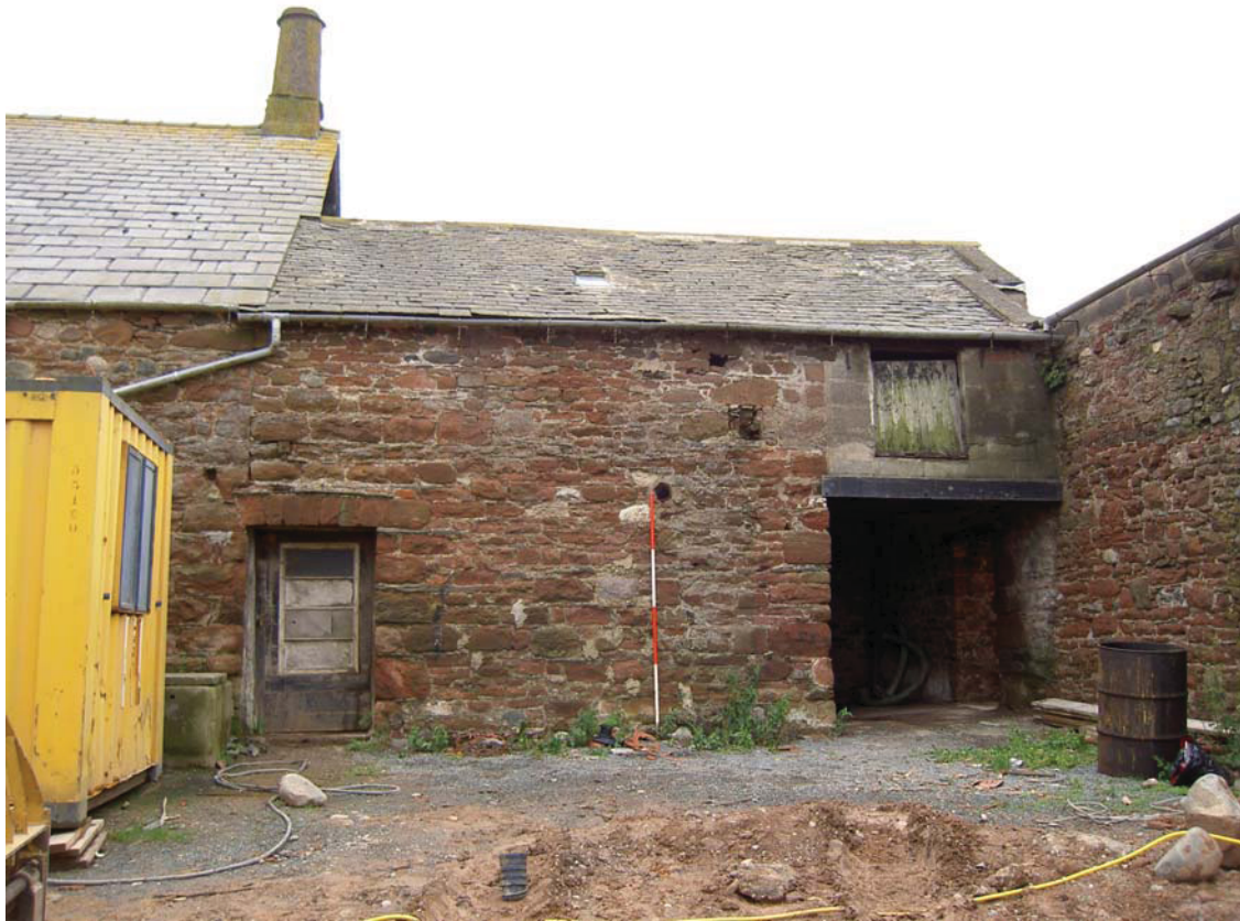
Plate 9: Building 5, north-north-east elevation
