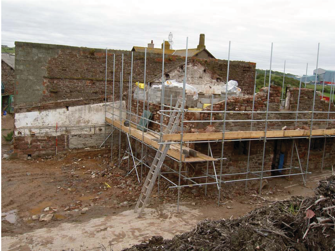
Plate 7: Building 3 and west elevation of Building 4, from the north-west
