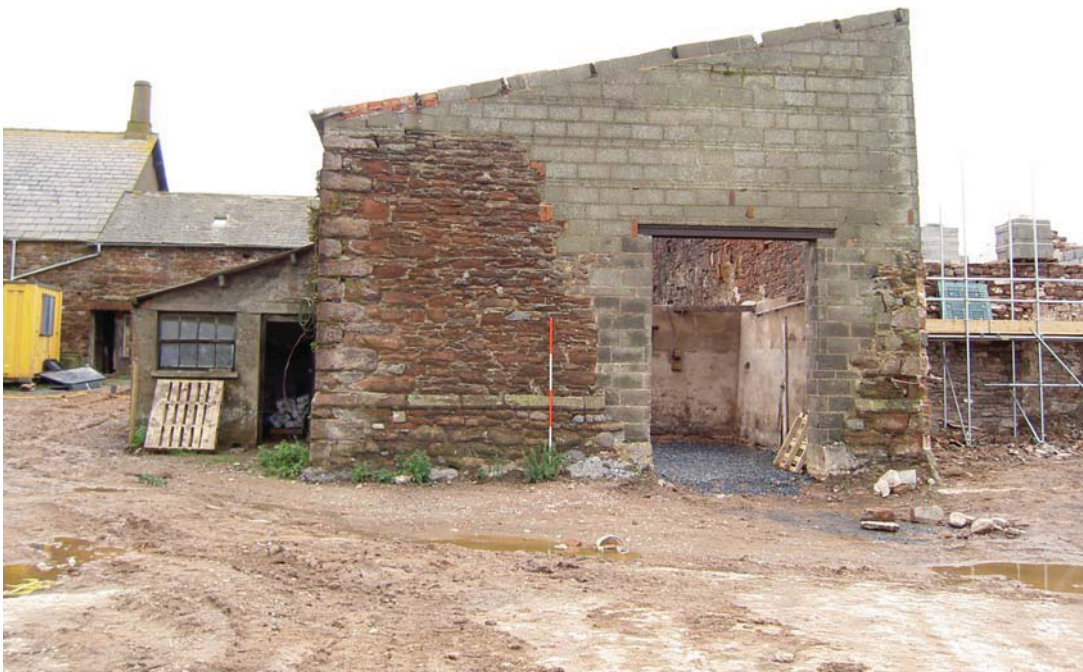
Plate 12: Building 4 from the north-north-east showing plinth
