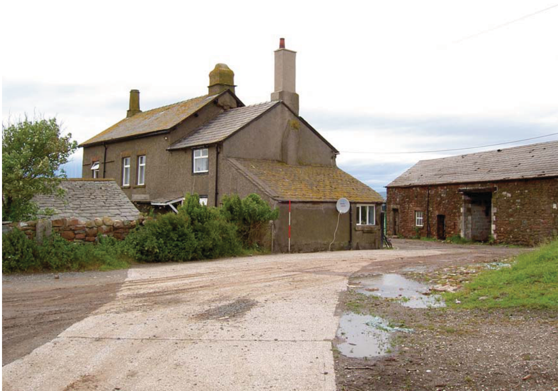
Plate 21: View of the Building 2 in relation to the farmhouse, from the south
