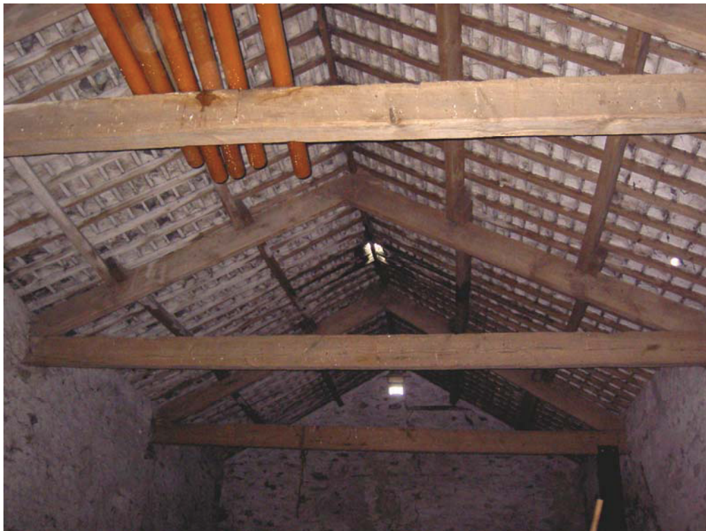
Plate 28: Roof trusses in ground floor threshing area of Building 4
