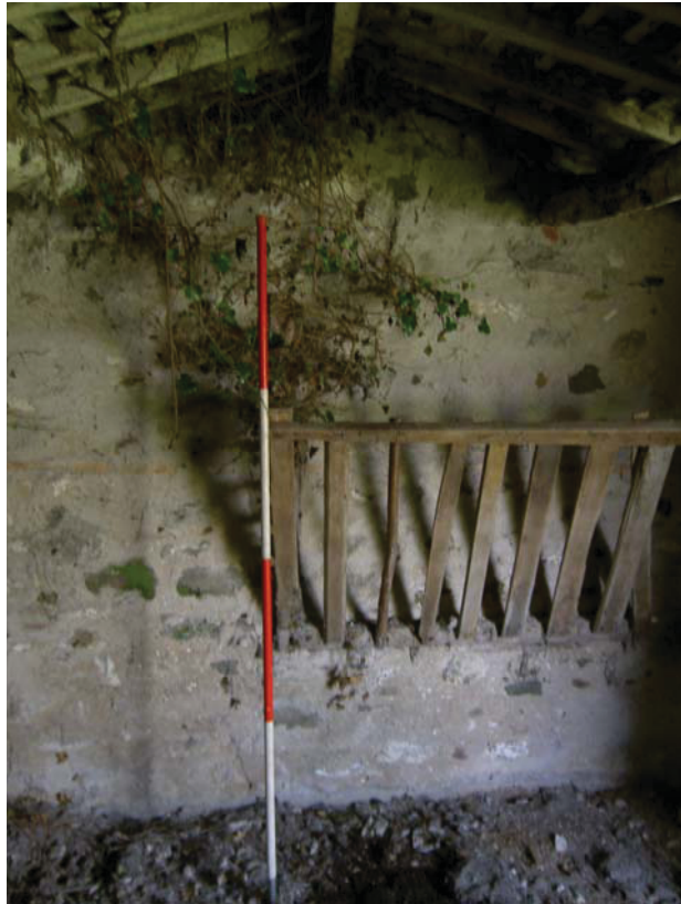
Plate 25: Interior north elevation of Building 2, showing row of orange ceramic tiles
