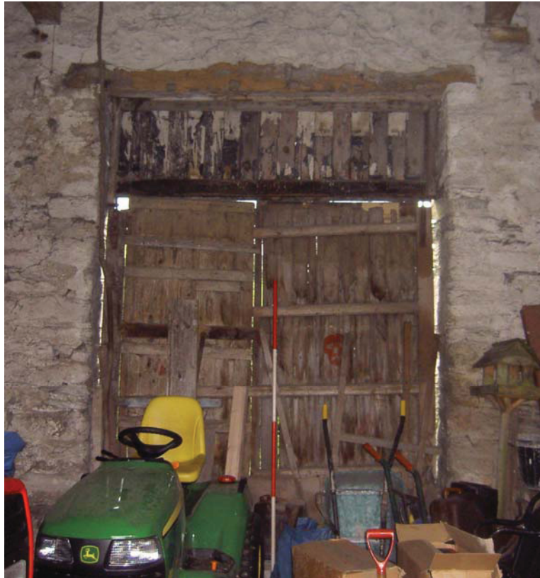
Plate 27: Northern door to ground floor of Building 4
