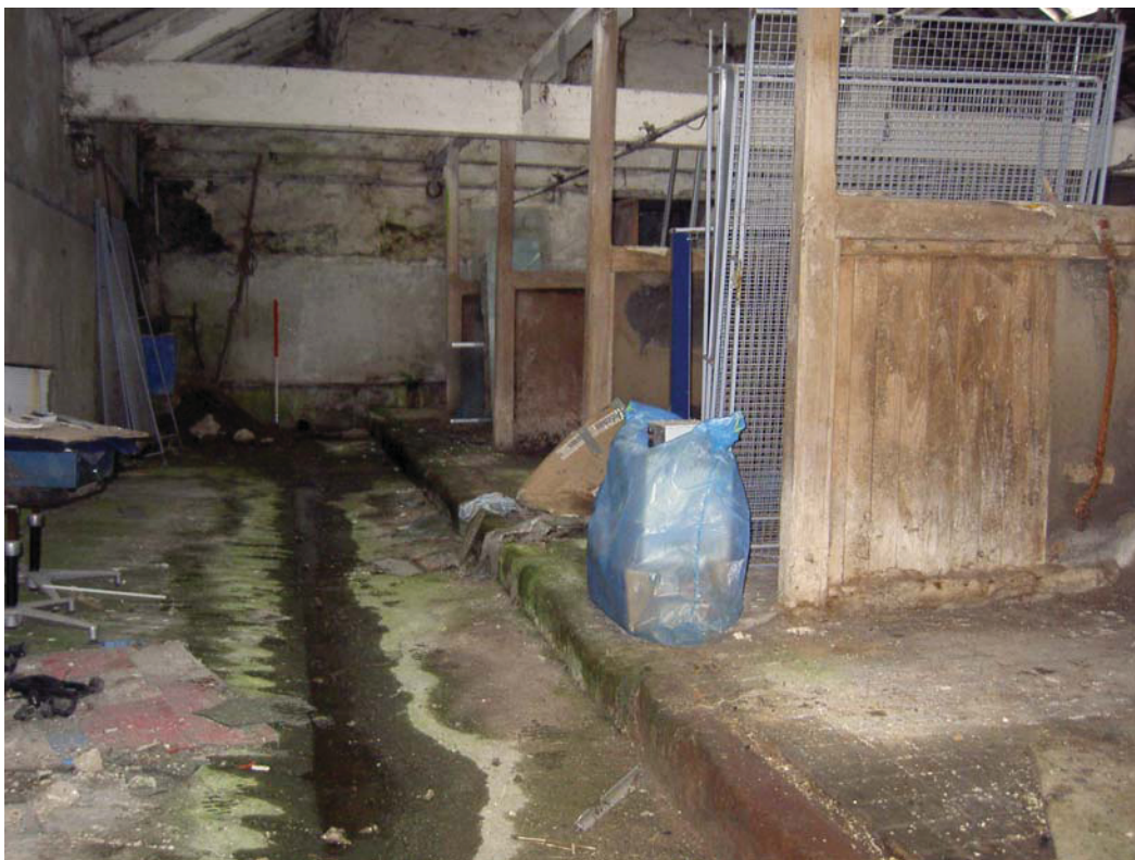
Plate 32: Western stalls in Building 5, showing stone and plank partitions
