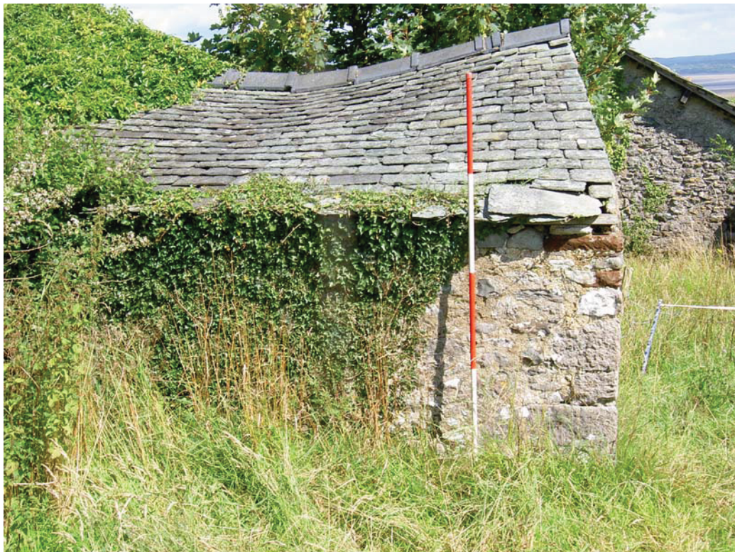
Plate 20: West elevation of Building 3
