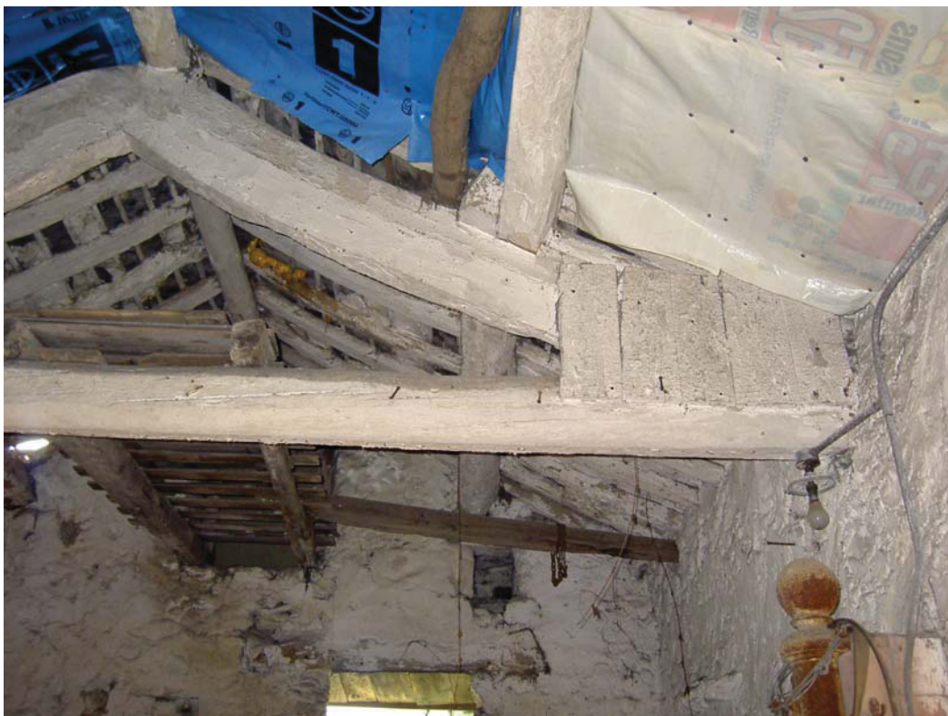
Plate 24: Internal west elevation of Building 2, showing 'ladder'
