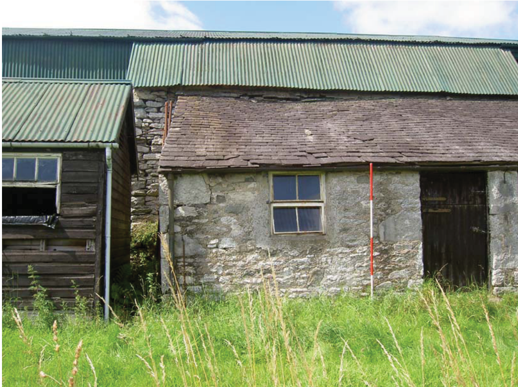
Plate 13: Southern part of Building 1, from east
