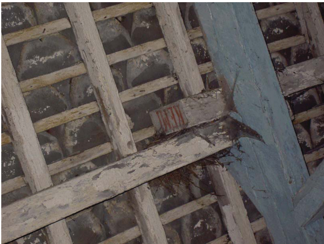
Plate 34: Marked purlin in roof of Building 5
