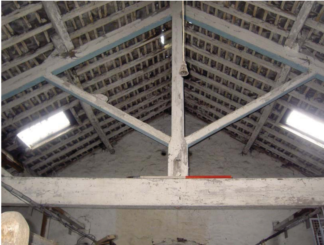
Plate 33: Roof truss in Building 5, from south
