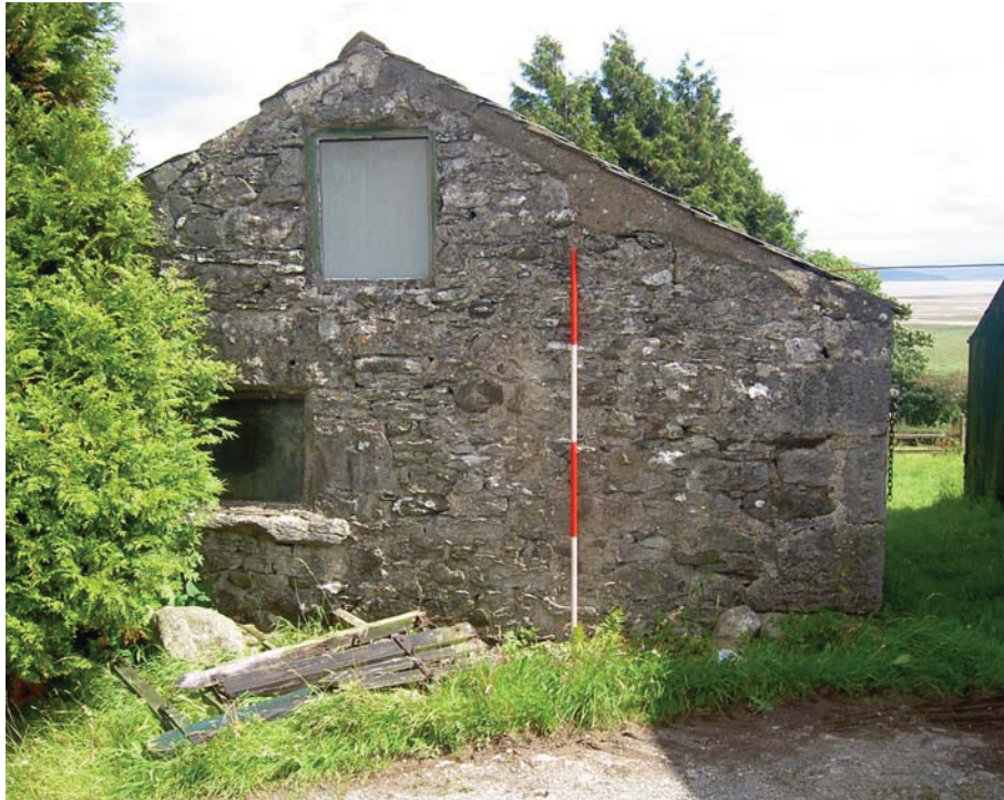
Plate 17: West elevation of Building 2
