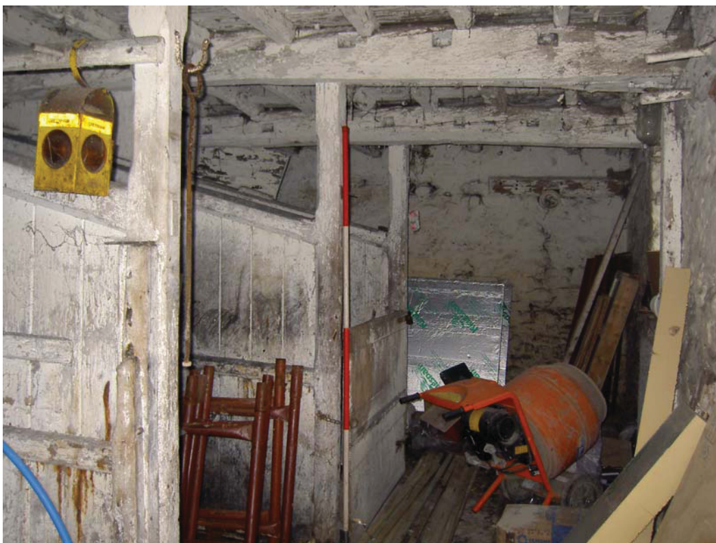
Plate 30: Stalls in eastern shippon, lower ground floor of Building 4
