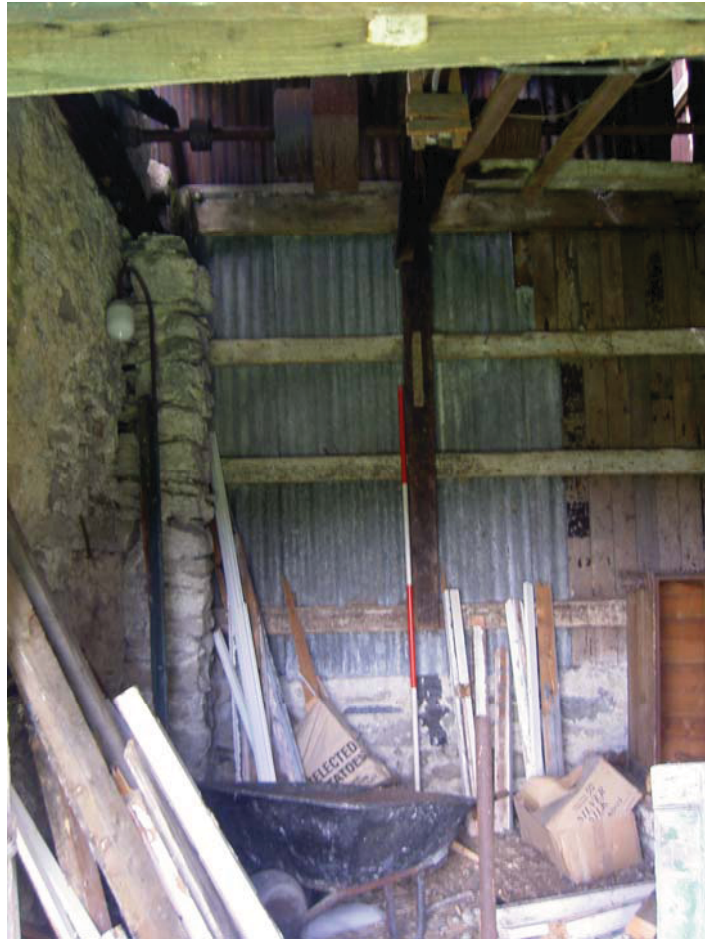
Plate 15: Interior of outshut at north of Building 1, from east
