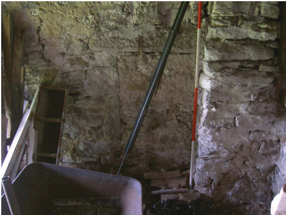
Plate 16: Blocked doorway in north elevation of Building 1, from north
