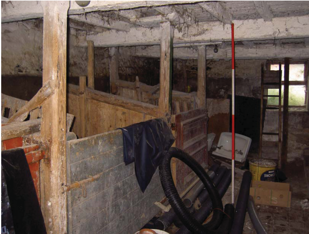
Plate 31: Stalls in western shippon, lower ground floor of Building 4
