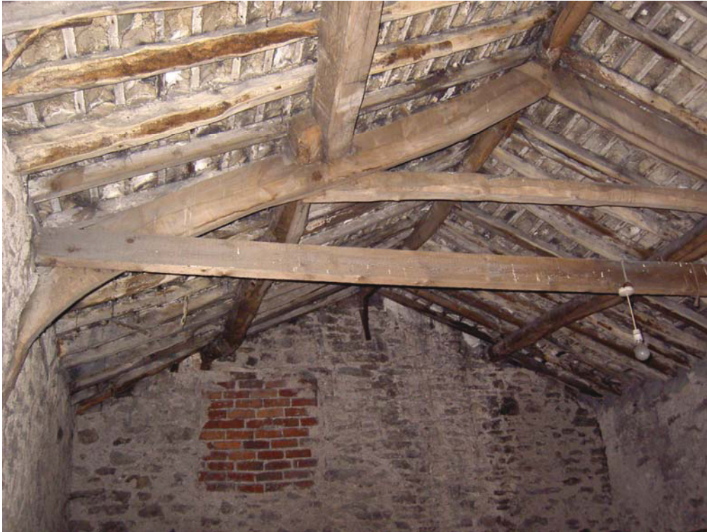
Plate 15: General view of south face of truss, first floor Building 2
