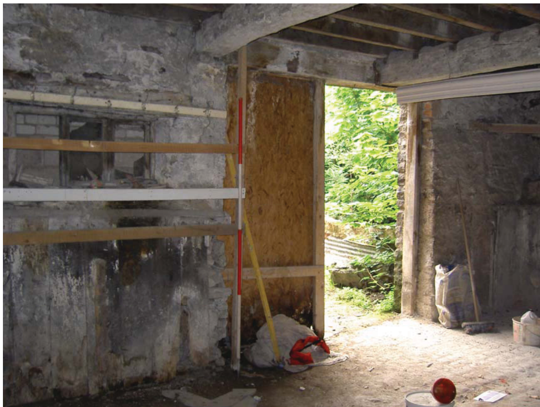
Plate 14: Doorway in south-east side of ground floor, Building 2
