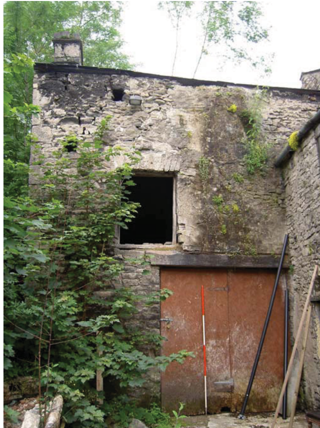
Plate 11: The east external elevation of Building 2
