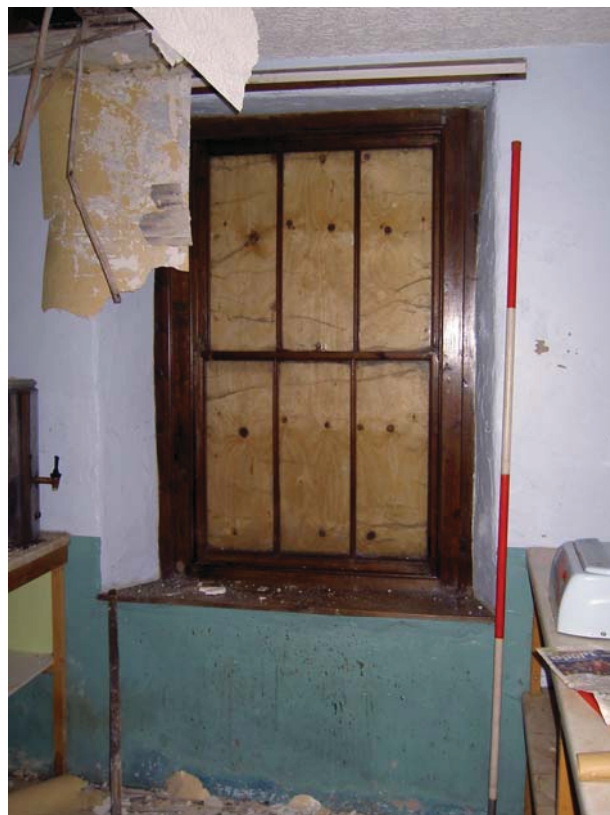
Plate 42: Sliding sash window in ground floor Room 7
