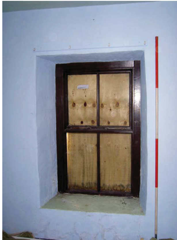
Plate 55: Typical modern window, first floor Room 7
