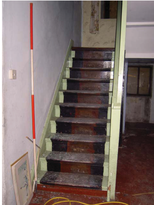
Plate 41: Stairs in ground floor Room 6
