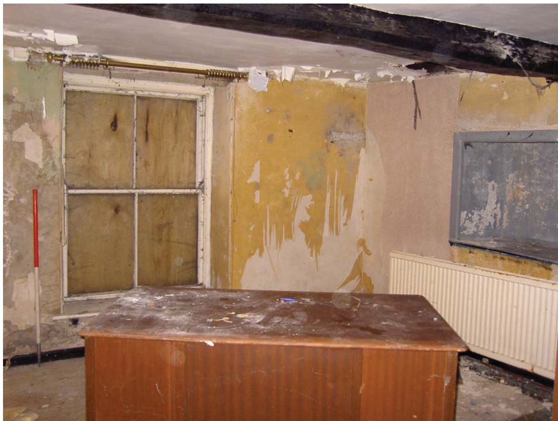
Plate 40: General view of ground floor Room 4
