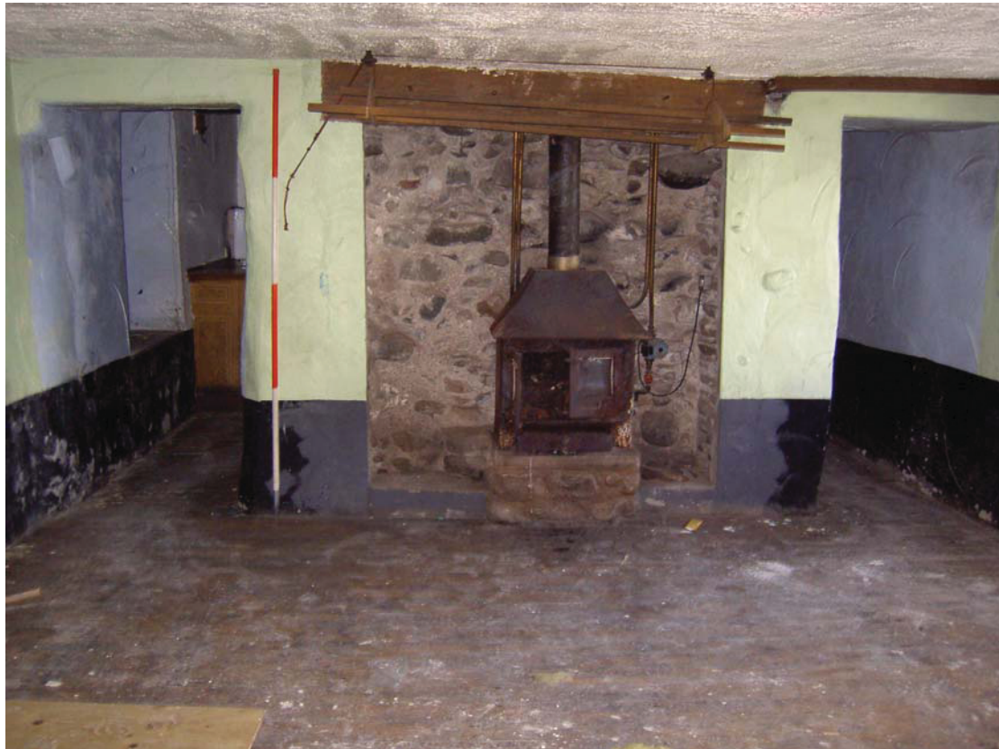
Plate 47: Enlarged fireplace in ground floor Room 9
