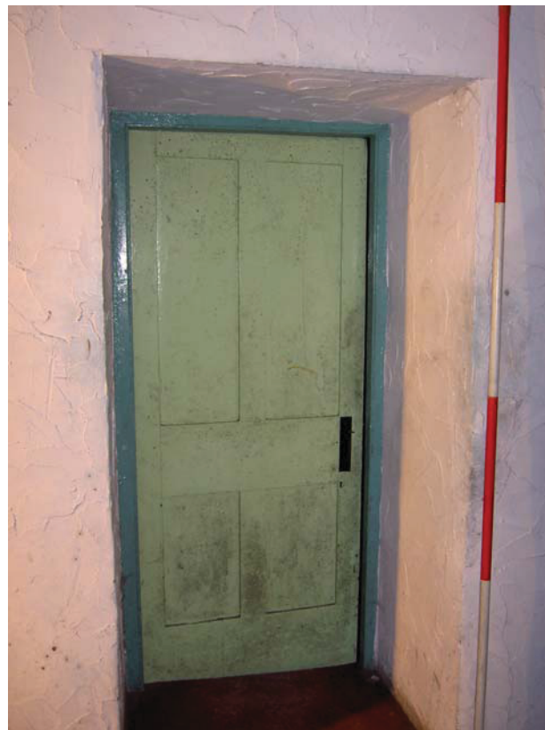
Plate 44: Typical four-panel door leading into ground floor Room 7
