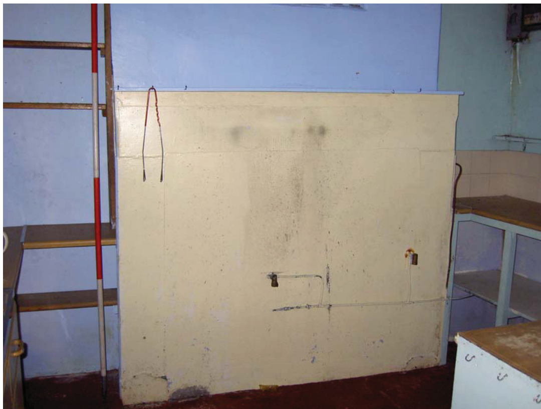
Plate 38: The large fireplace in ground floor Room 1
