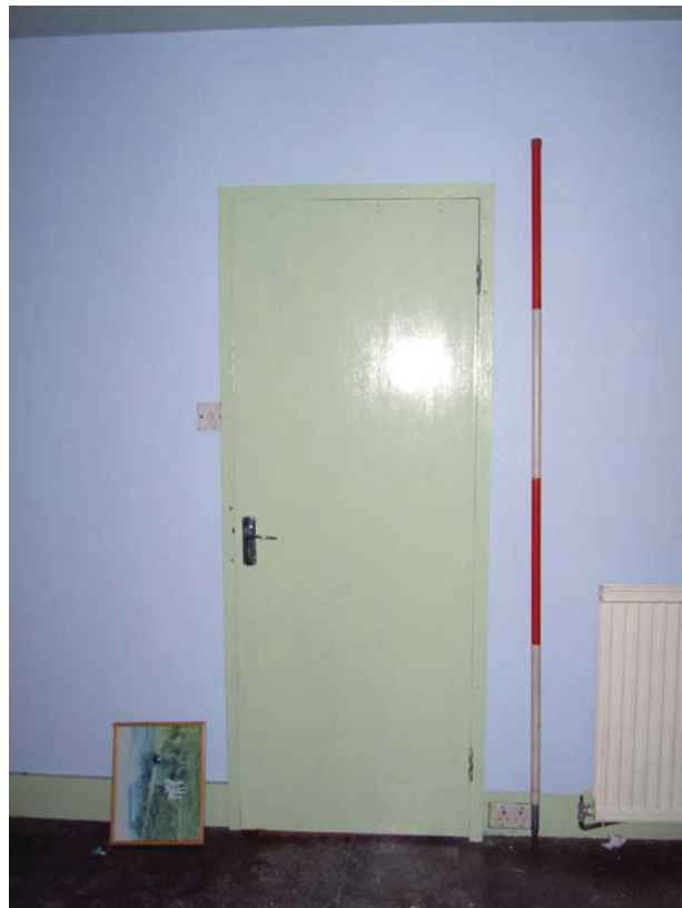
Plate 54: Typical modern plywood door, first floor Room 7
