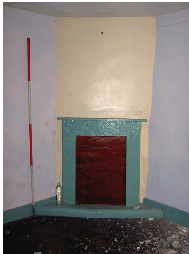
Plate 52: Fireplace in first floor Room 4
