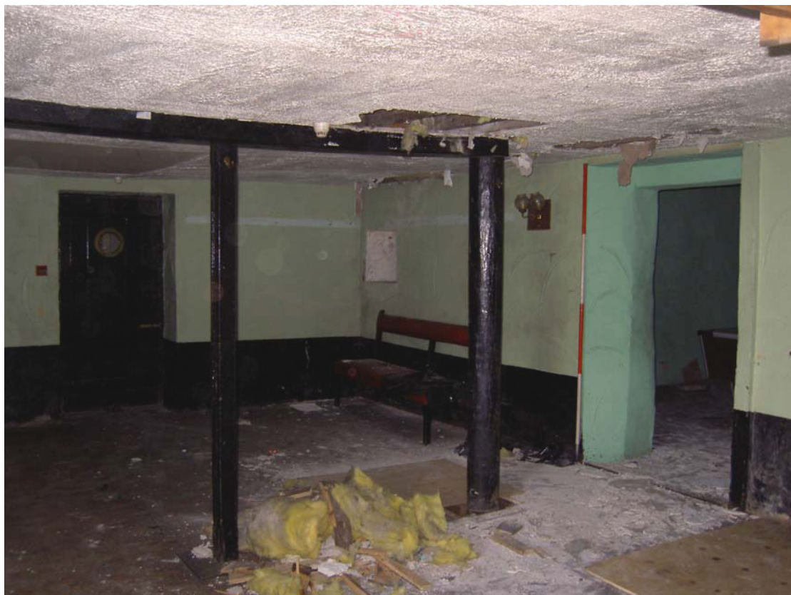
Plate 46: Inserted beam and posts in ground floor Room 9
