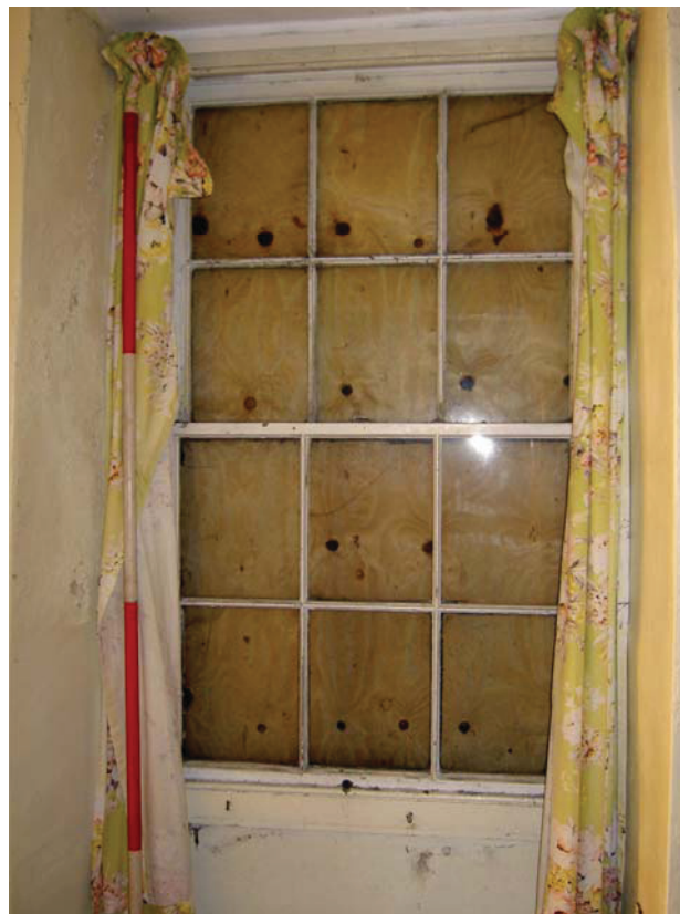
Plate 50: Typical sliding sash window, first floor Room 2
