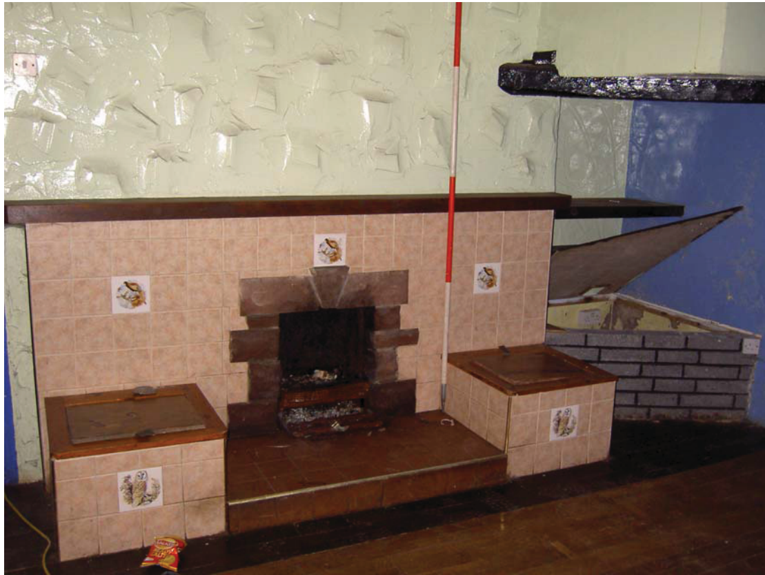
Plate 39: The modern fireplace in ground floor Room 3
