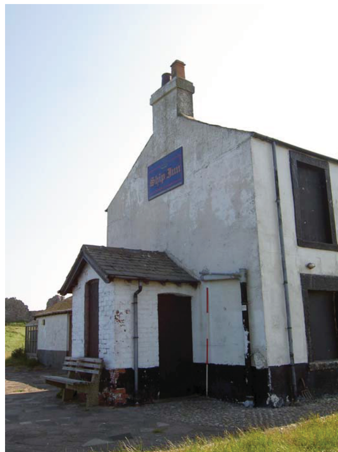
Plate 36: The east external elevation
