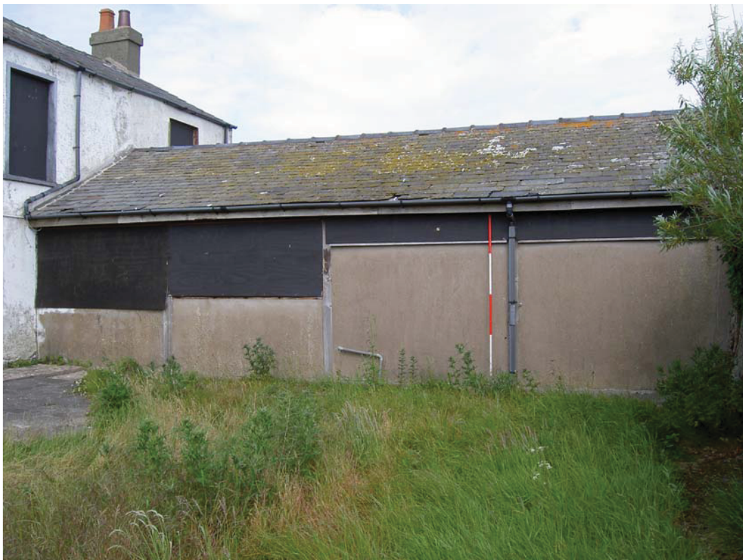
Plate 32: The west external elevation of the pool room
