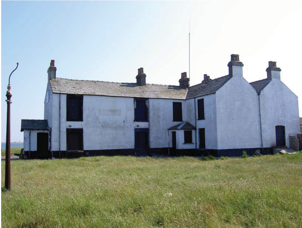
Plate 29: The north external elevation of the building
