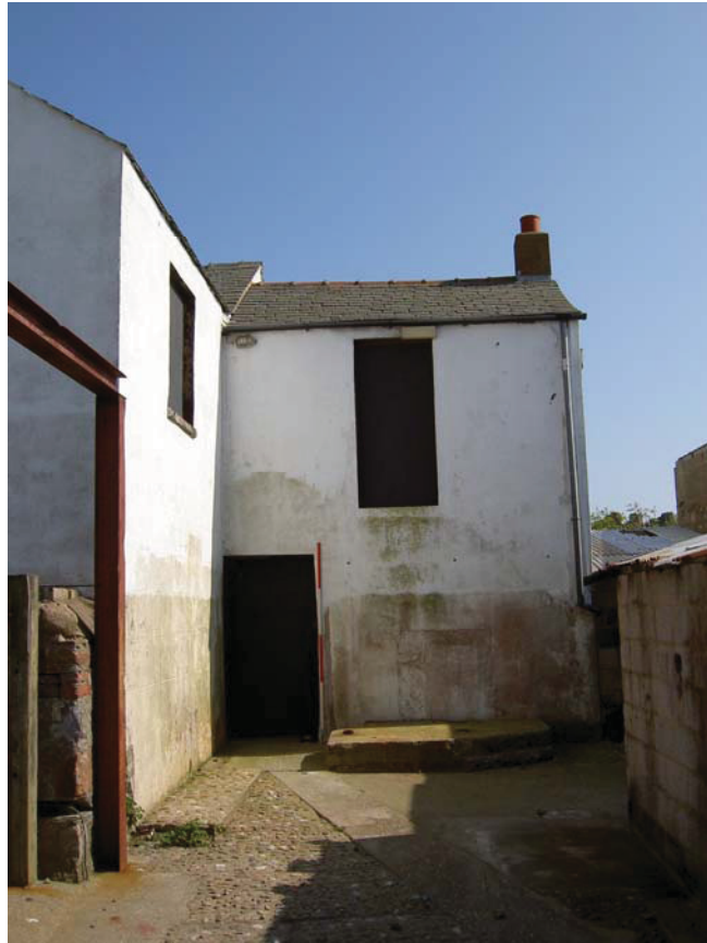
Plate 31: The west end of the north elevation of the building
