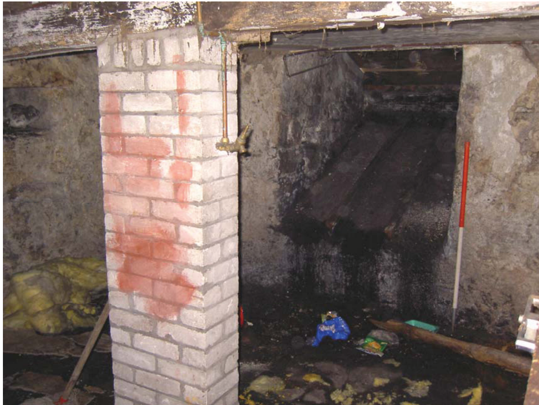
Plate 37: General view of cellar Room 1 showing the brick column supporting the ceiling and the barrel hatch
