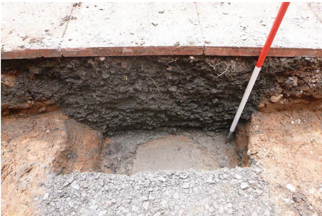
Plate 26: Concrete 108 at the base of feature 105, viewed from the north-east
