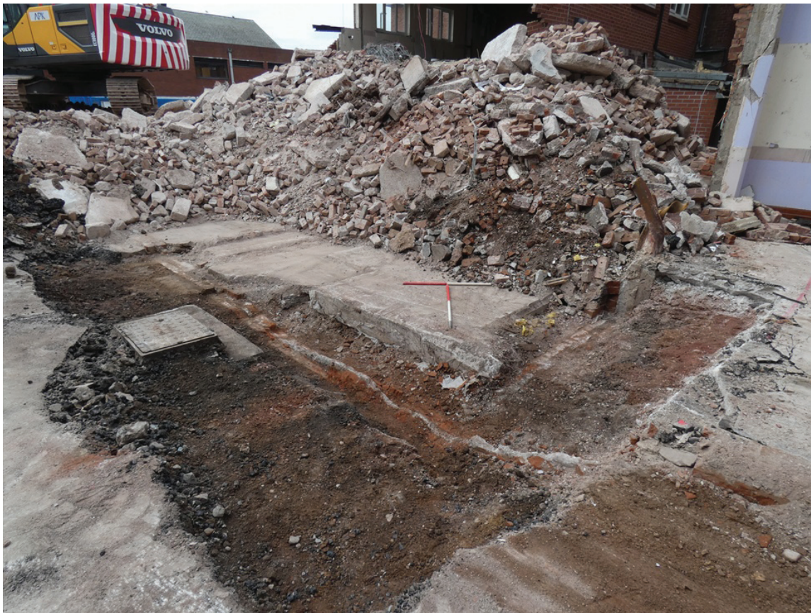
Plate 36 Trench 3, viewed from the east
