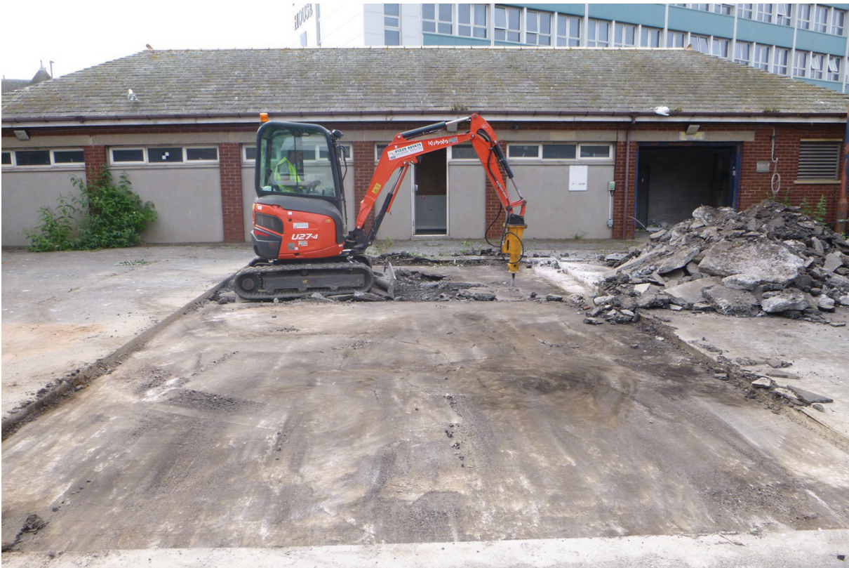
Plate 29: Removing concrete surface 202 , viewed from the north-west
