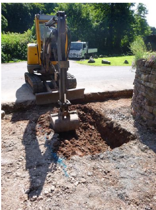
Plate 3: Working shot, south pit, viewed from the west
