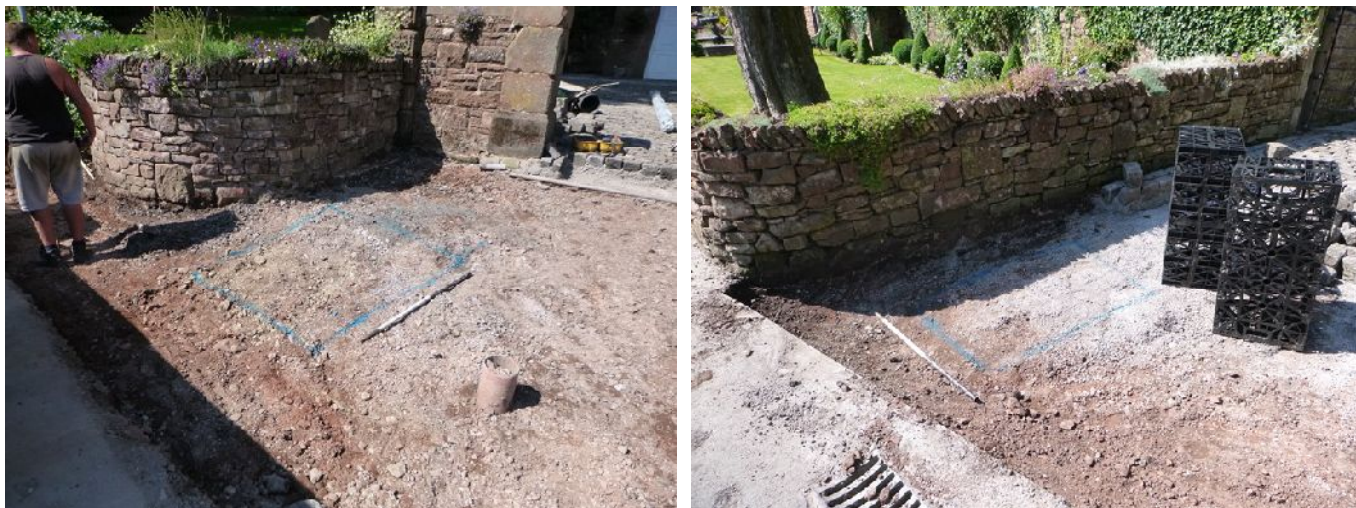
Plate 1 (left): The south pit prior to excavation, viewed from the north-east
