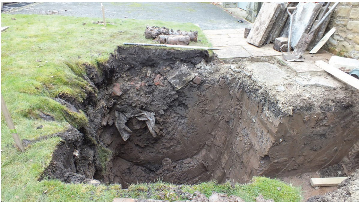
Plate 122: East-facing section of the trench excavated to the south of the barn
