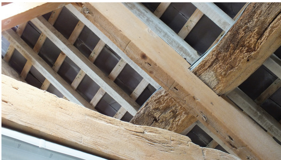
Plate 79: Timber marks on the truss in Room 3
