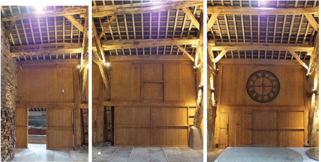
Plate 67 (left): Bay 5, west elevation, Room 2
