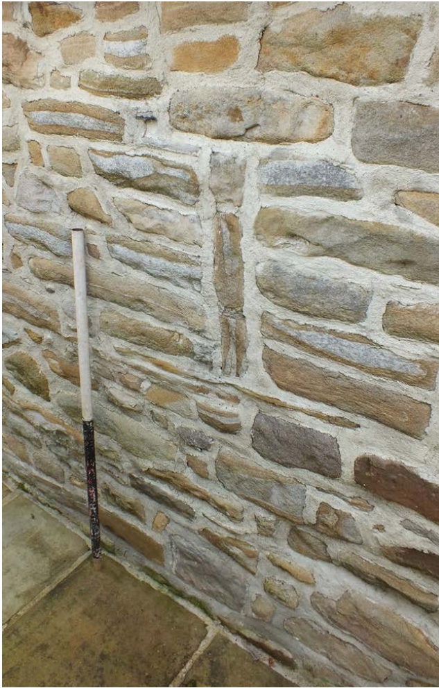
Plate 25 (left): Blocked ventilation slot at the south end of the east external elevation
