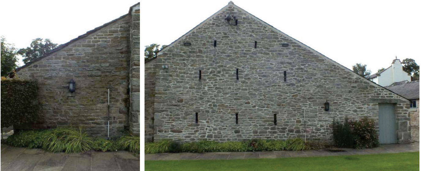
Plate 6 (left): East end of the north external elevation
