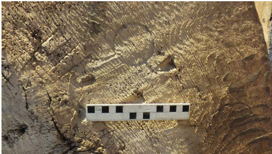
Plate 48: smaller circular mark on the south face of the east side of Truss 3, Room 2
