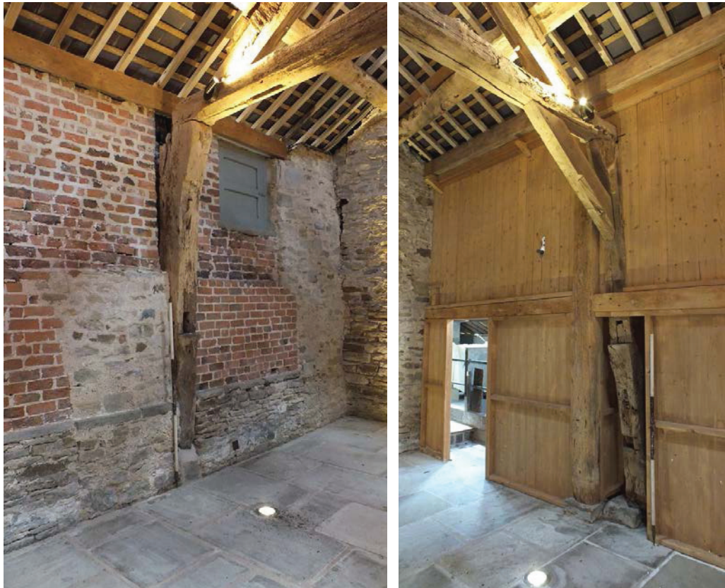
Plate 55 (left): East side of the north face of Truss 5
