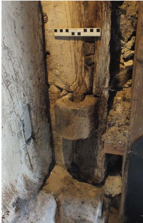
Plate 62: Pivot at the base of the post to the south of Truss 2, Room 2
