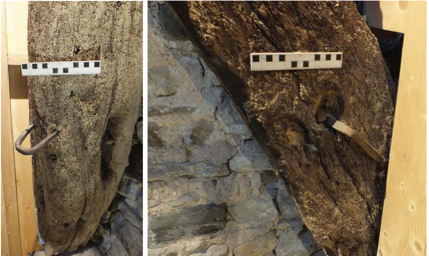
Plate 33 (left): Iron tether at the west end of Truss 1, Room 2
