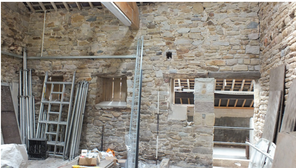
Plate 84: West elevation of Room 3
