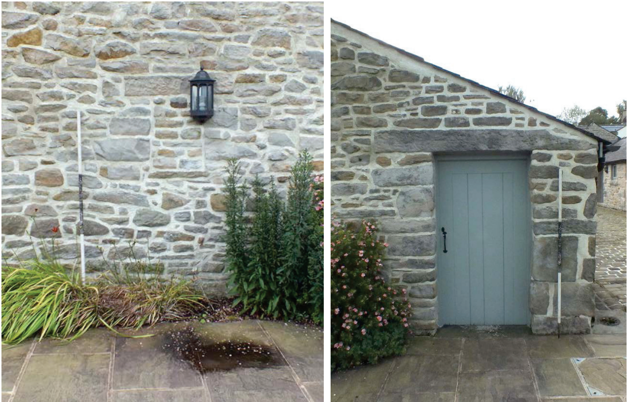
Plate 8 (left): Blocked window in the north external elevation
