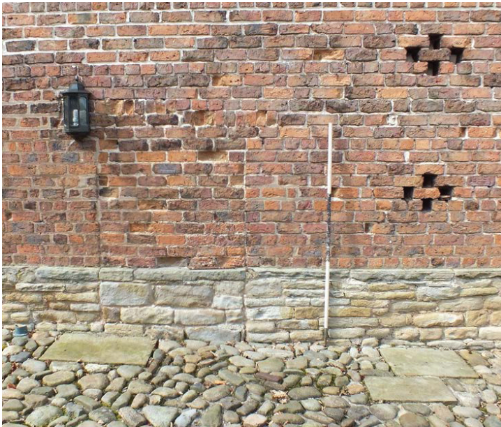
Plate 13 (left): Blocked feature and ventilators in the brick-built section of the east external elevation
