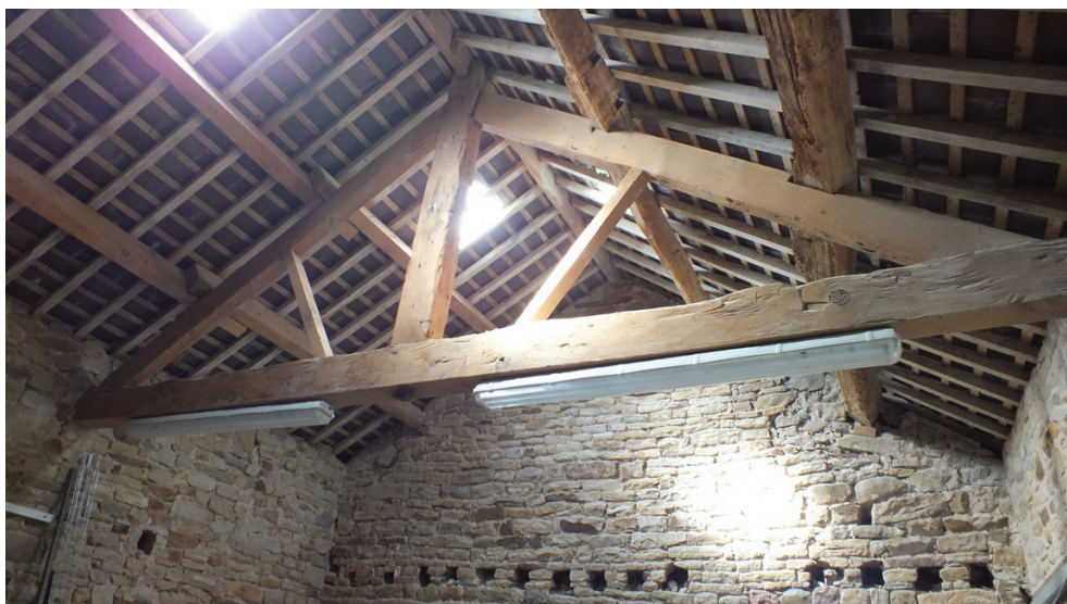
Plate 78: Truss in Room 3
