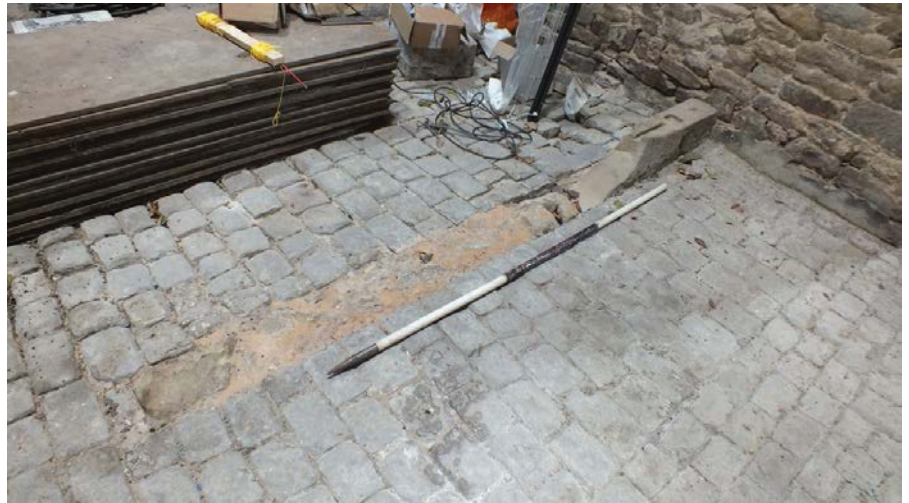
Plate 74 (left): Sett floor in the west side of Room 3 and channel
