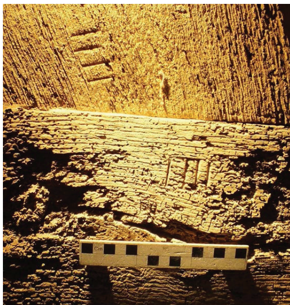
Plate 50 (left): Carpenter's mark 'IIII' on the west side of the north face of Truss 4, Room 2
