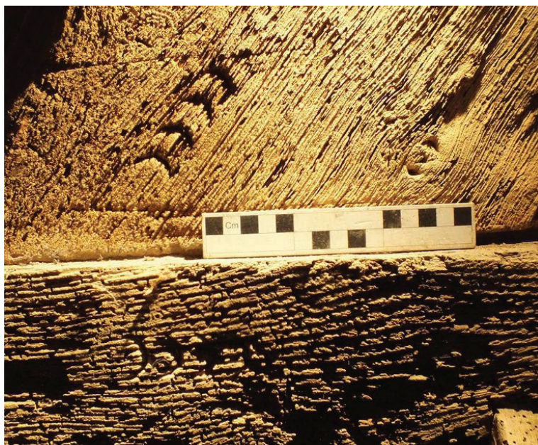
Plate 50 (left): Carpenter's mark 'IIII' on the west side of the north face of Truss 4, Room 2
