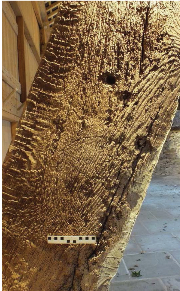
Plate 47 (left): Circle motifs including possible 'daisy wheel' on the south side of the west cruck of Truss 3, Room 2
