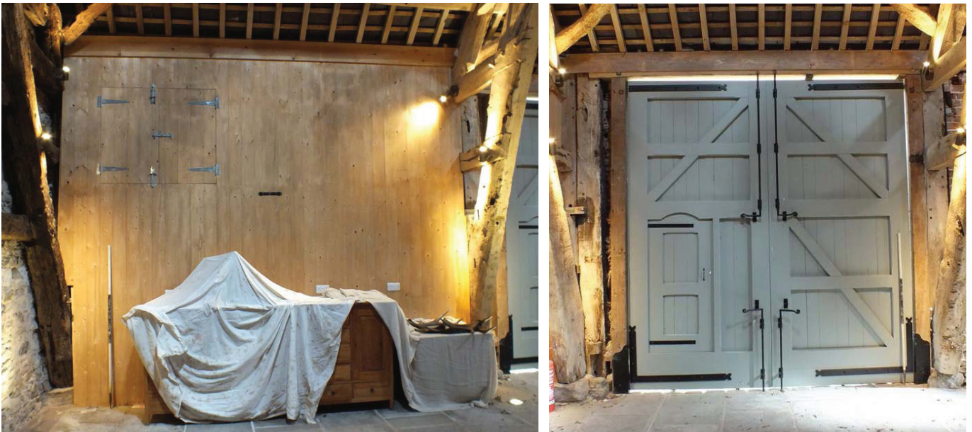
Plate 60 (left): Bay 1, east elevation, Room 2
