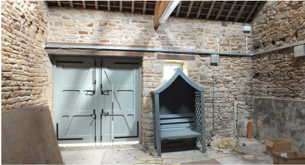
Plate 81: East elevation of Room 3
