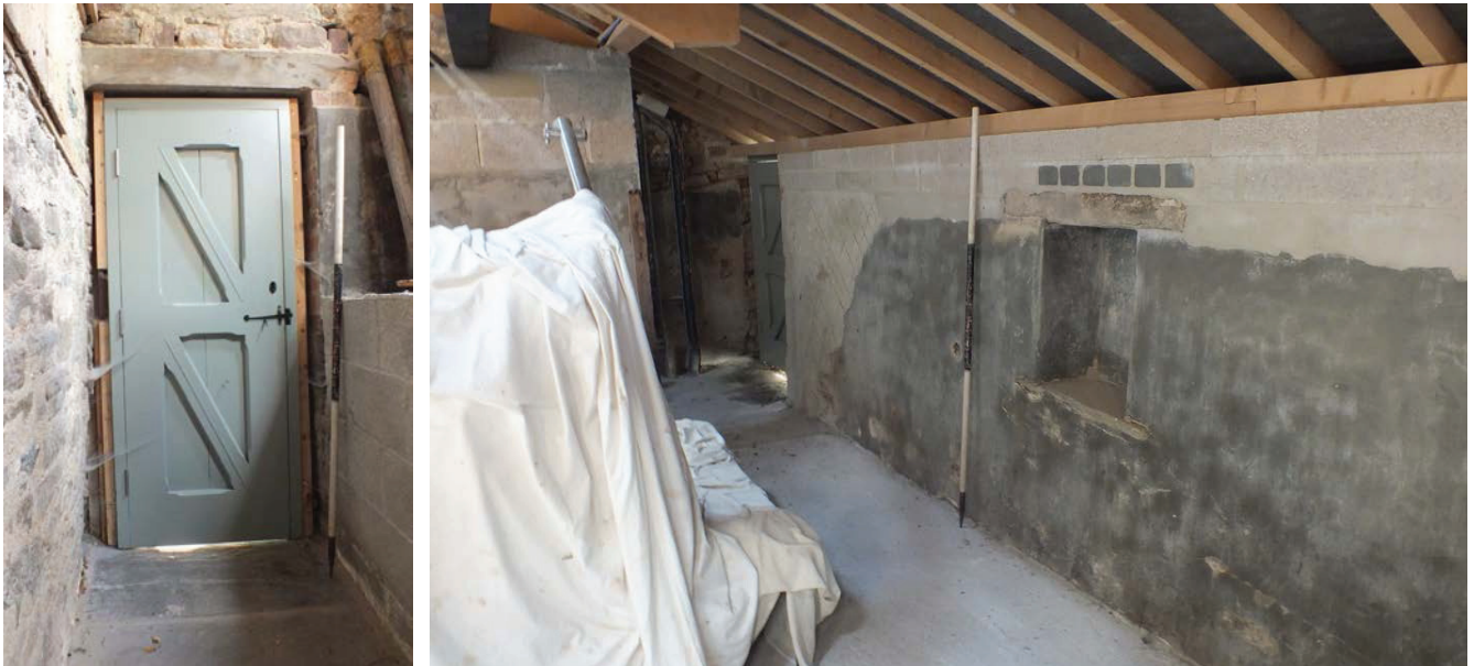
Plate 101 (left): Doorway in the south elevation of Room 4
