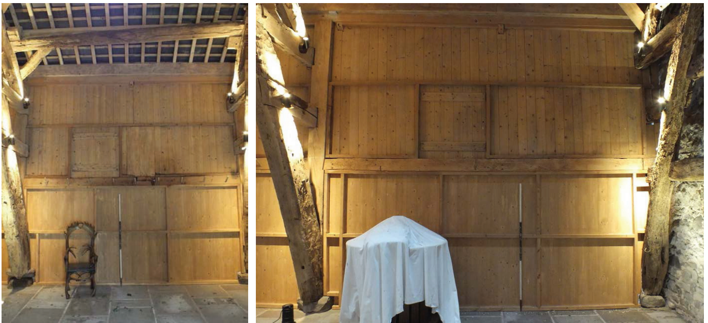
Plate 70 (left): Bay 2, West elevation, Room 2
