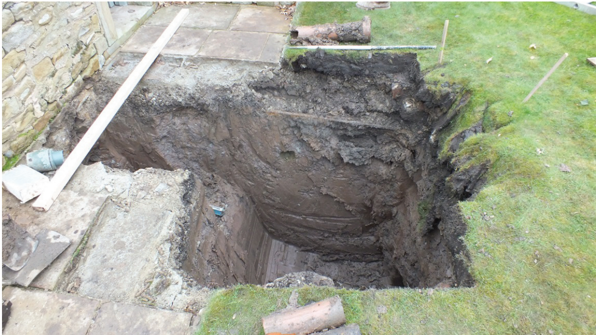
Plate 121: West-facing section of the trench excavated to the south of the barn
