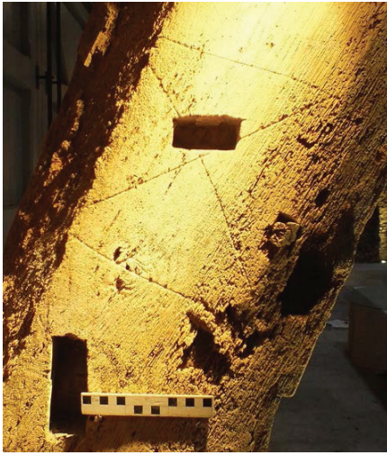
Plate 39 (left): Levelling mark on the east side of the north face of Truss 2, Room 2
