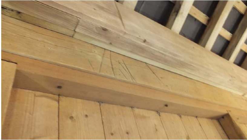
Plate 72 (left): Baltic timber marks in the wall plate at the top of the west elevation, Bay 4, Room 2
