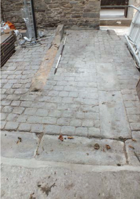
Plate 74 (left): Sett floor in the west side of Room 3 and channel
