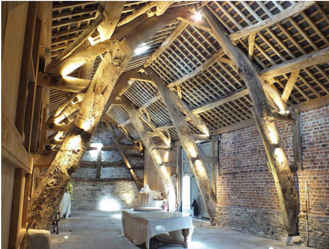
Plate 53: South face of Truss 4
