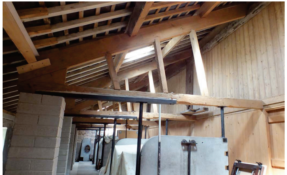
Plate 87 (left): Step down in the north-west corner of Room 4
