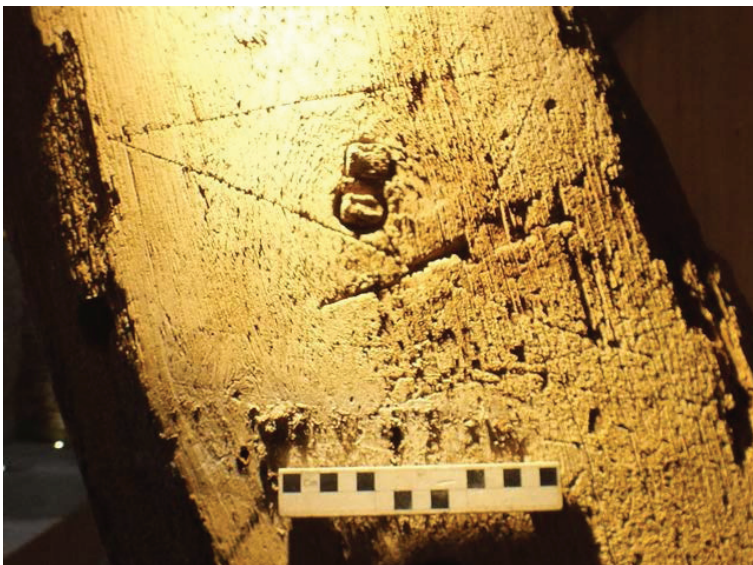
Plate 37 (left): Levelling mark on the west side of the north face of Truss 2, Room 2
