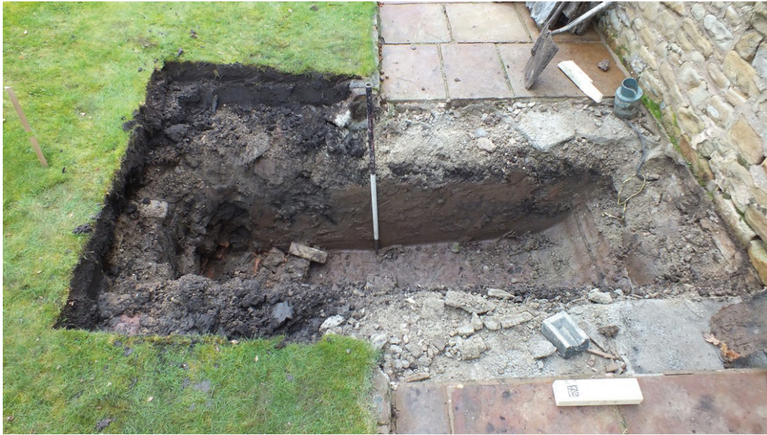
Plate 119: Excavation underway to the south side of the barn
