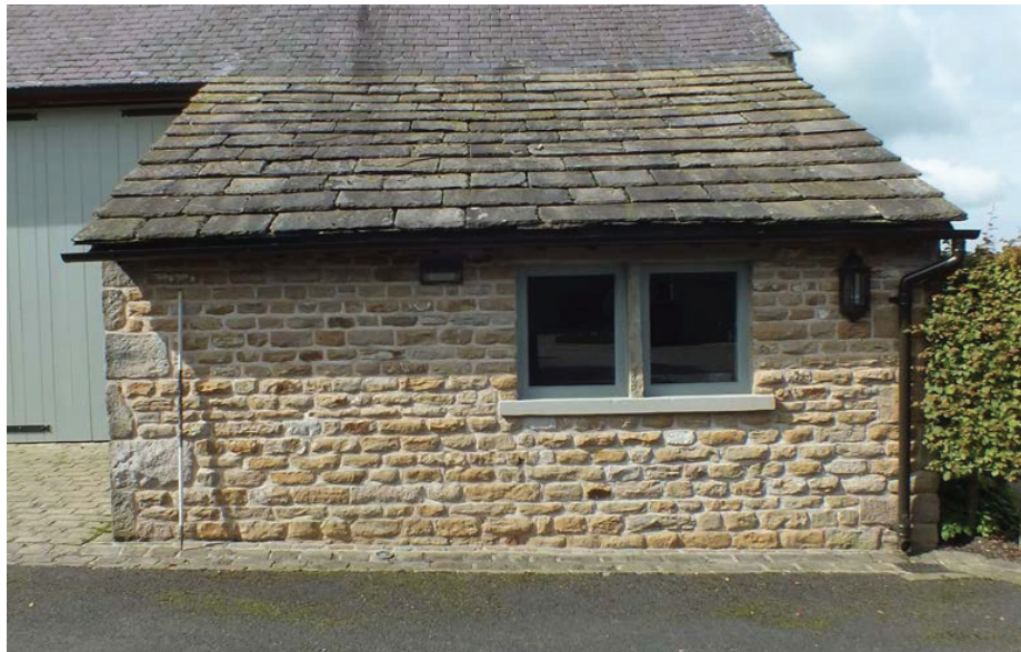
Plate 15: East external elevation of the north-east outshut
