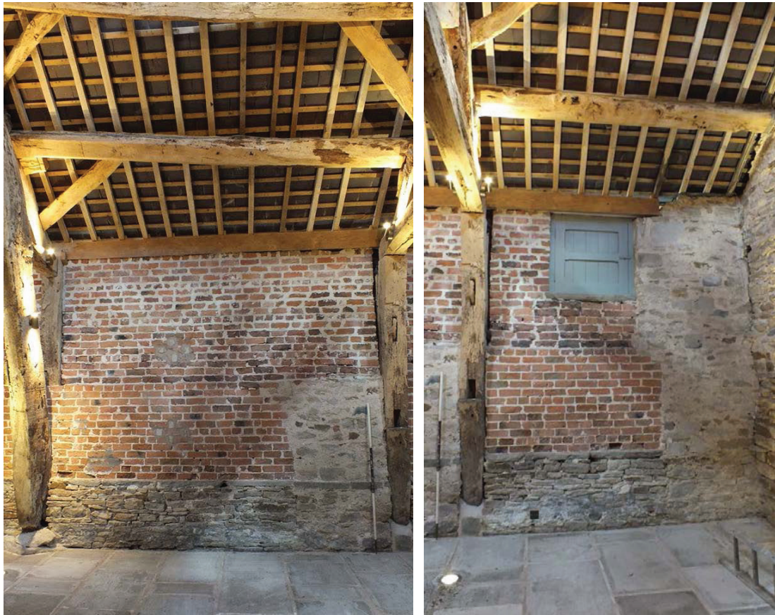
Plate 65 (left): Bay 4, east elevation, Room 2
