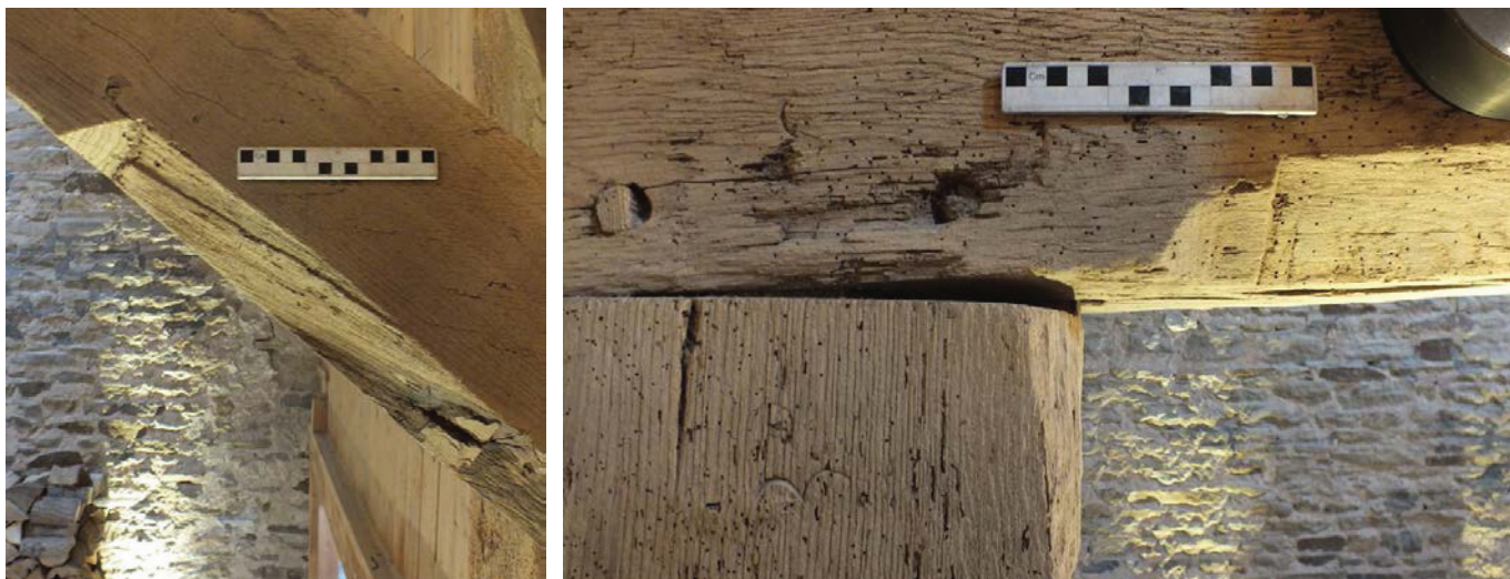
Plate 57 (left): Stop-chamfered brace on the east side of the north face of Truss 5, Room 2
