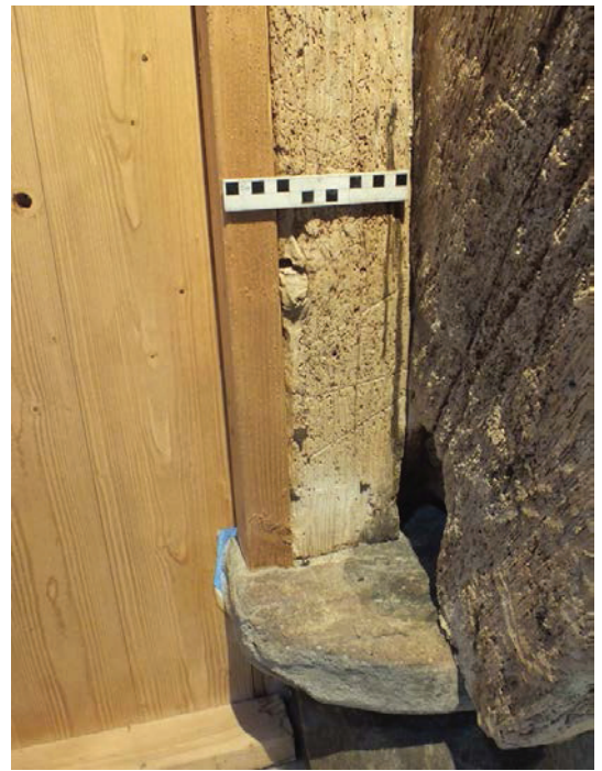
Plate 72 (left): Baltic timber marks in the wall plate at the top of the west elevation, Bay 4, Room 2
