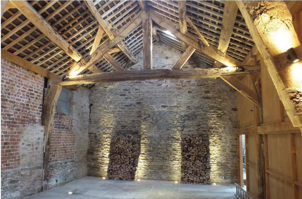
Plate 54: North face of Truss 5
