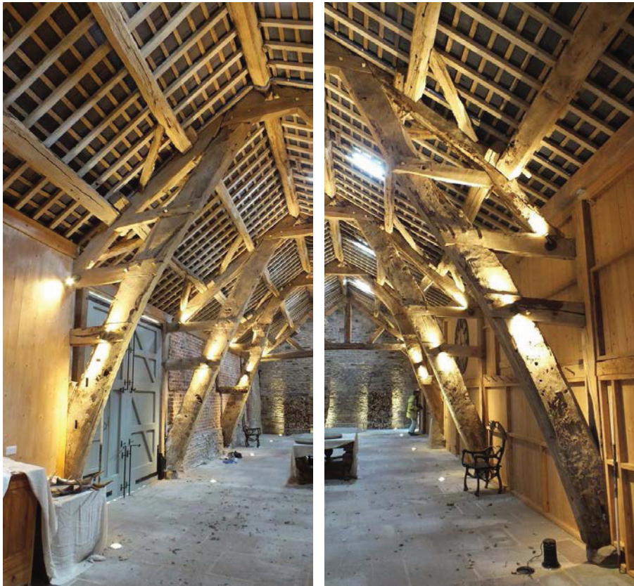
Plate 35 (left): The east side of the north face of Truss 2, Room 2
