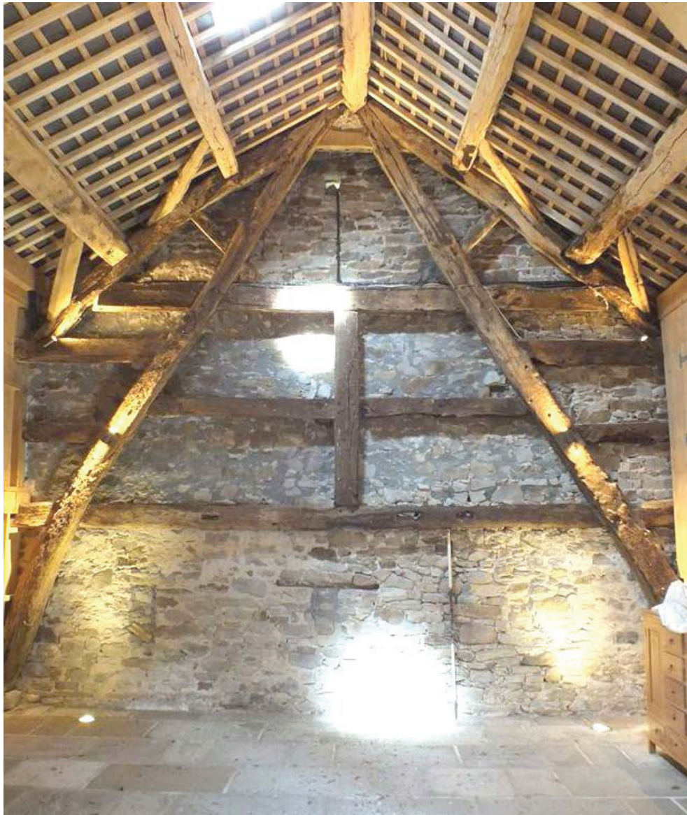
Plate 31: South face of Truss 1, Room 2
