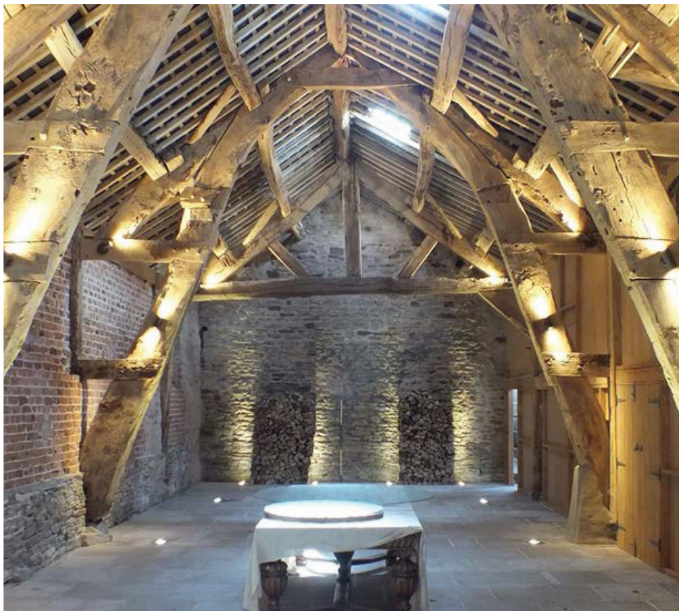
Plate 49: The north face of Truss 4, Room 2
