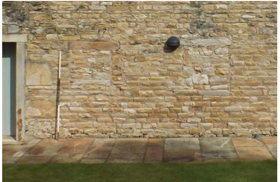
Plate 17 (left): Doorway in the south external elevation
