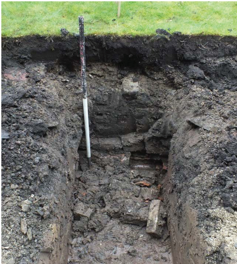
Plate 120: Ceramic drain below setts to the south end of the trench to the south of the barn
