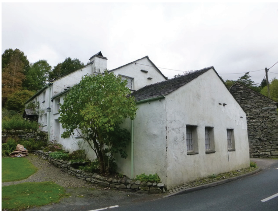
Plate 15: the east external elevation of the house, viewed from the south-east
