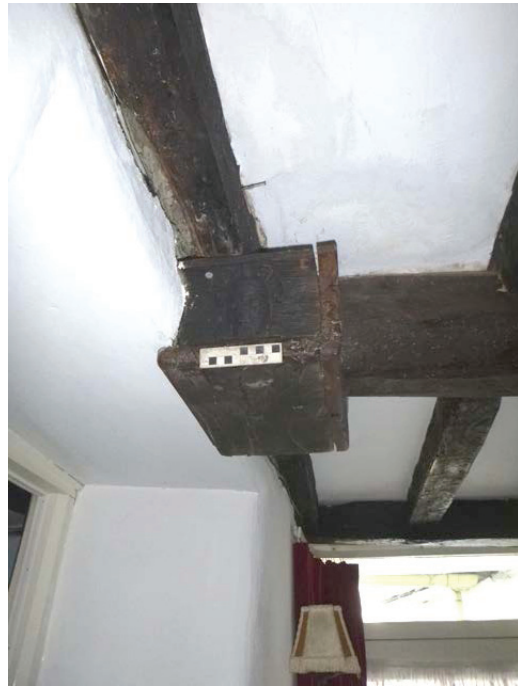
Plate 52 (left): decorated block covering the east end of the beam in Room G9m viewed from the north
