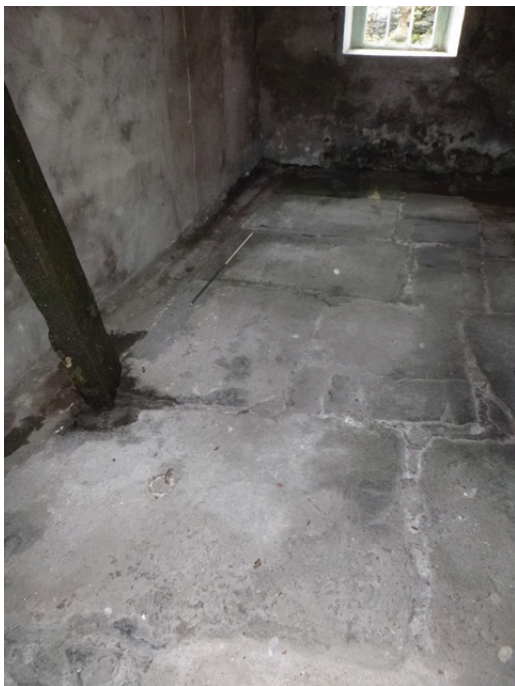
Plate 26 (left): the flag floor and drainage channel along the west side of Room G1, viewed from the north-east
