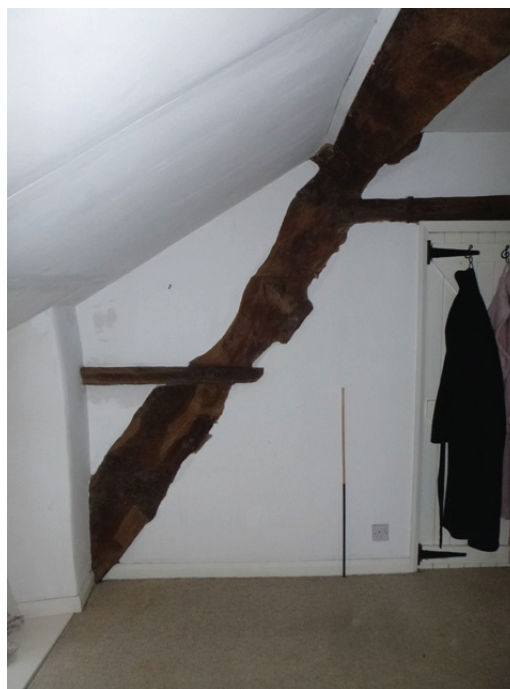
Plate 81 (left): the cruck truss on the east side of Room F10, viewed from the south-west
