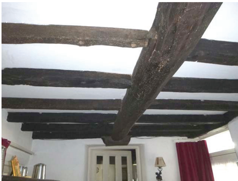
Plate 51: beam and joists in Room G9, viewed from the west
