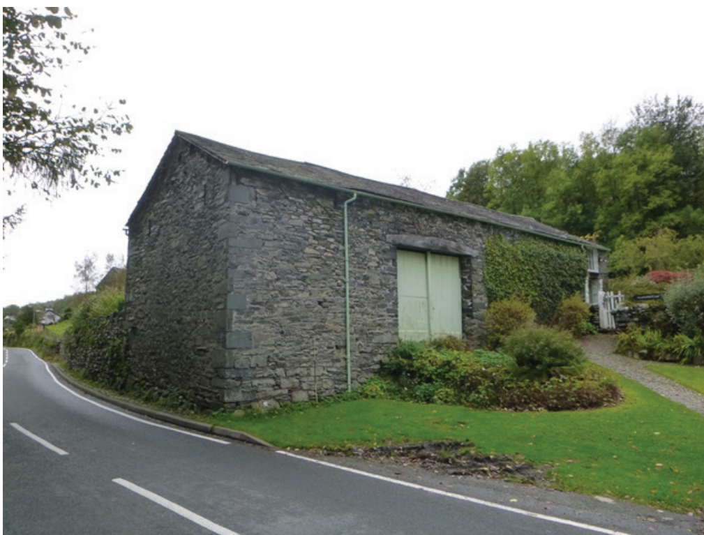
Plate 25: general view of the east and north external elevations of the barn, viewed from the north-east
