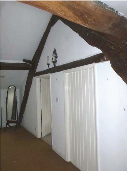
Plate 77 (left): the cruck truss to the west of Room F8, viewed from the south-east
