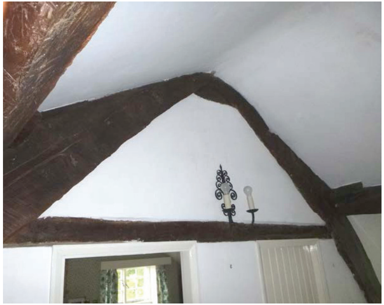
Plate 77 (left): the cruck truss to the west of Room F8, viewed from the south-east
