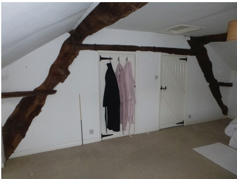
Plate 81 (left): the cruck truss on the east side of Room F10, viewed from the south-west
