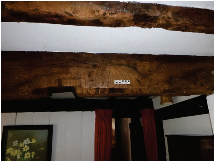
Plate 47 (left): slots in north/south beam in Room G8, viewed from the west
