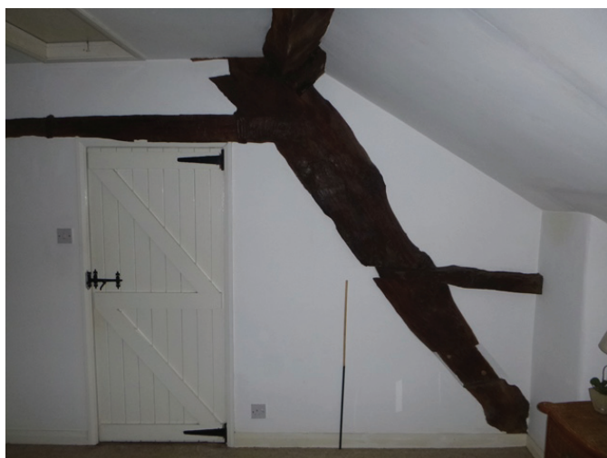
Plate 83 (left): taper marks on the south side of the cruck truss in Room G10, viewed from the west
