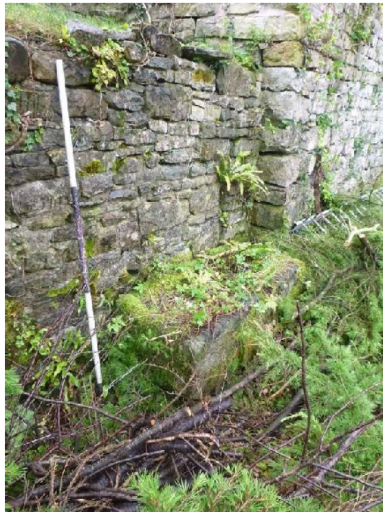
Plate 12: Stone tank or trough on site, viewed from the north-east
