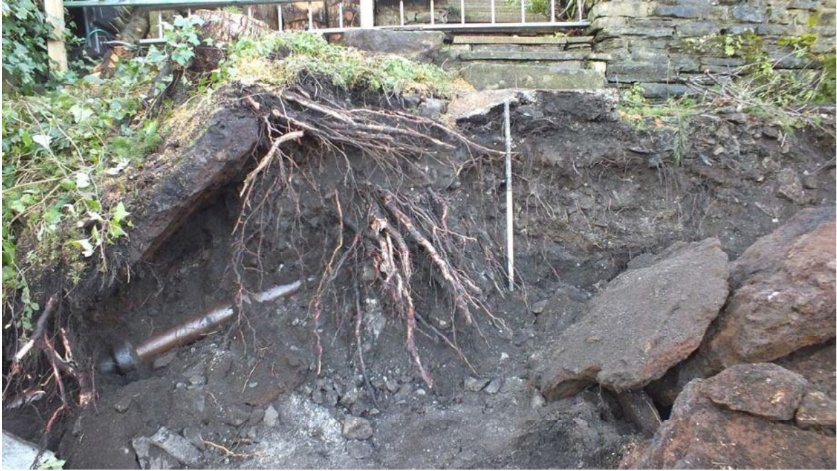
Plate 24: Ceramic drain below the slag heap close to the steps
