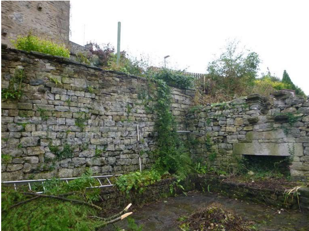
Plate 18: South-west corner of the room on the first floor
