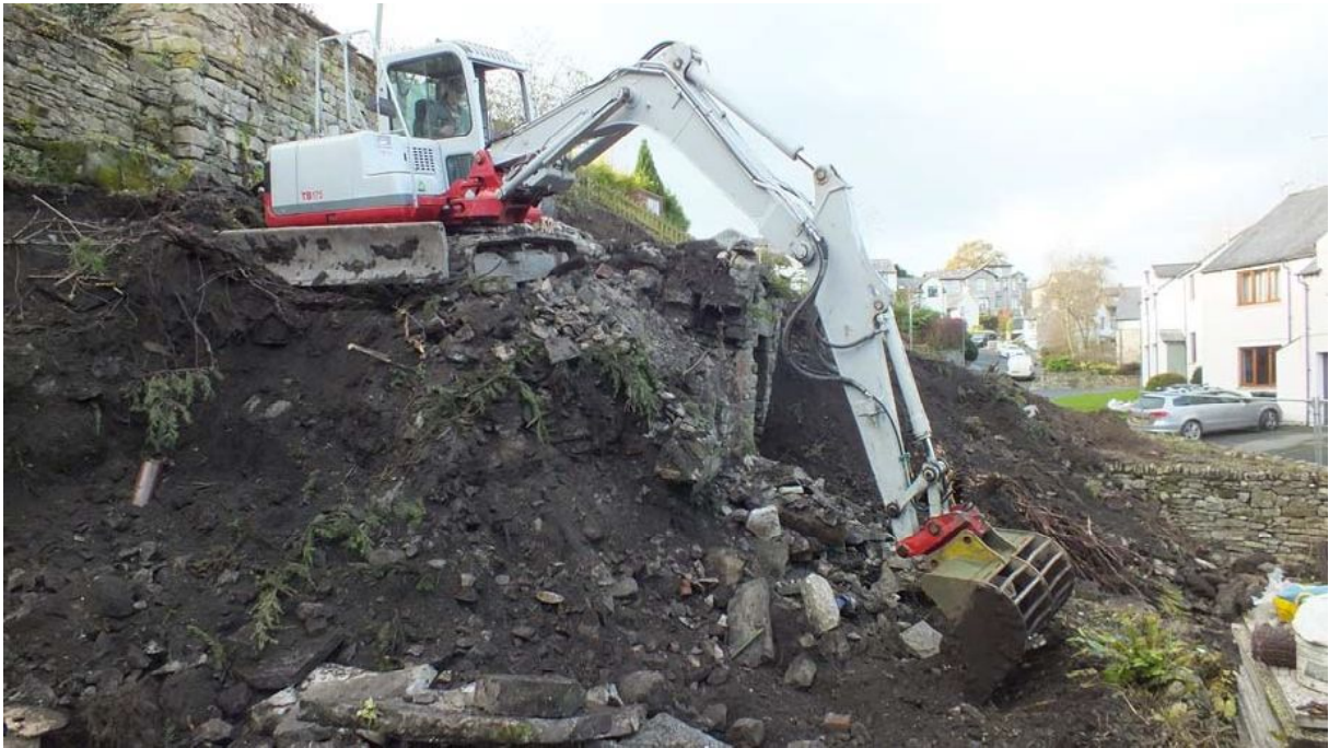
Plate 27: Demolition of the standing building underway
