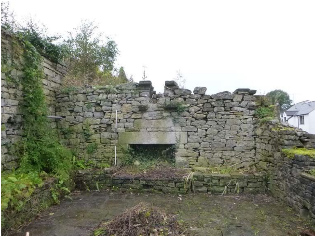
Plate 19: East internal elevation of the room on the first floor
