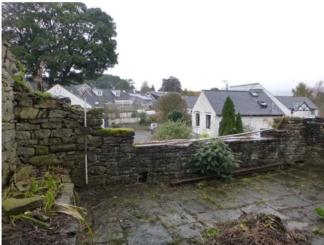
Plate 16: North internal elevation of the room on the first floor
