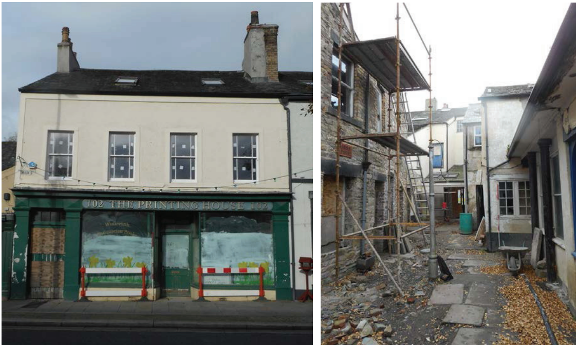
Plate 10 (left): View of 102 Main Street from the south
