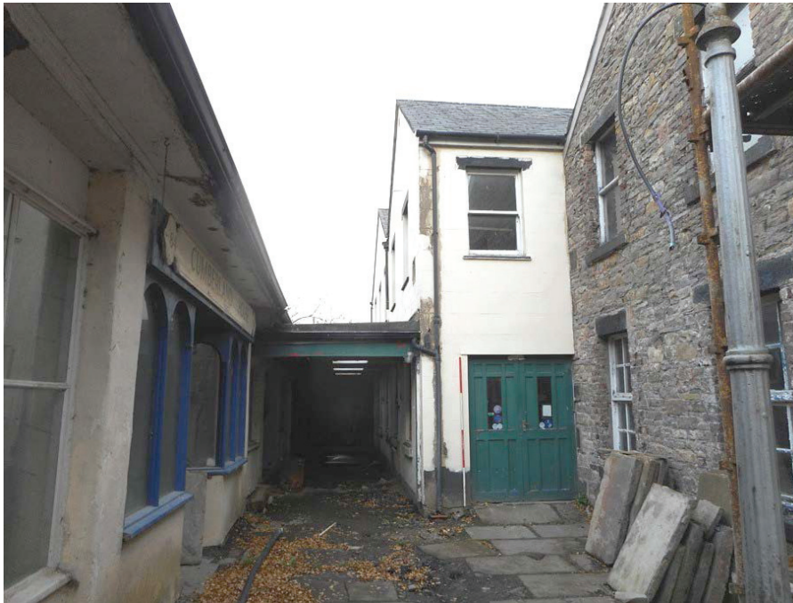
Plate 13: North end of the courtyard, viewed from the south
