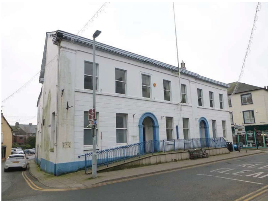
Plate 86: The west external elevation, viewed from the north-west
