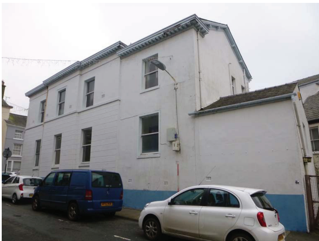
Plate 91: The west end of the south external elevation, viewed from the south-east
