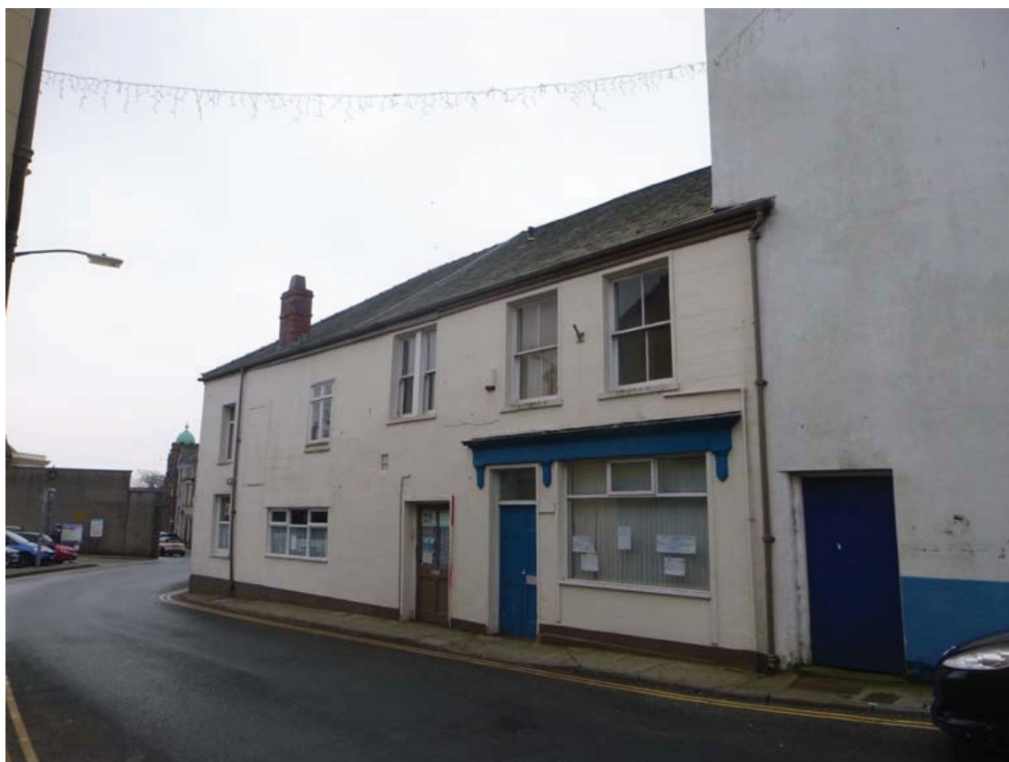
Plate 83: The east end of the north external elevation, viewed from the north-west
