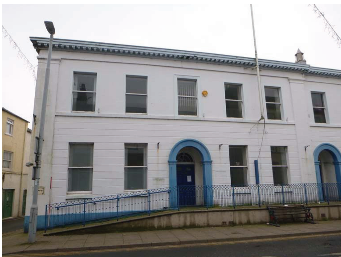
Plate 87: The north end of the west external elevation, viewed from the west
