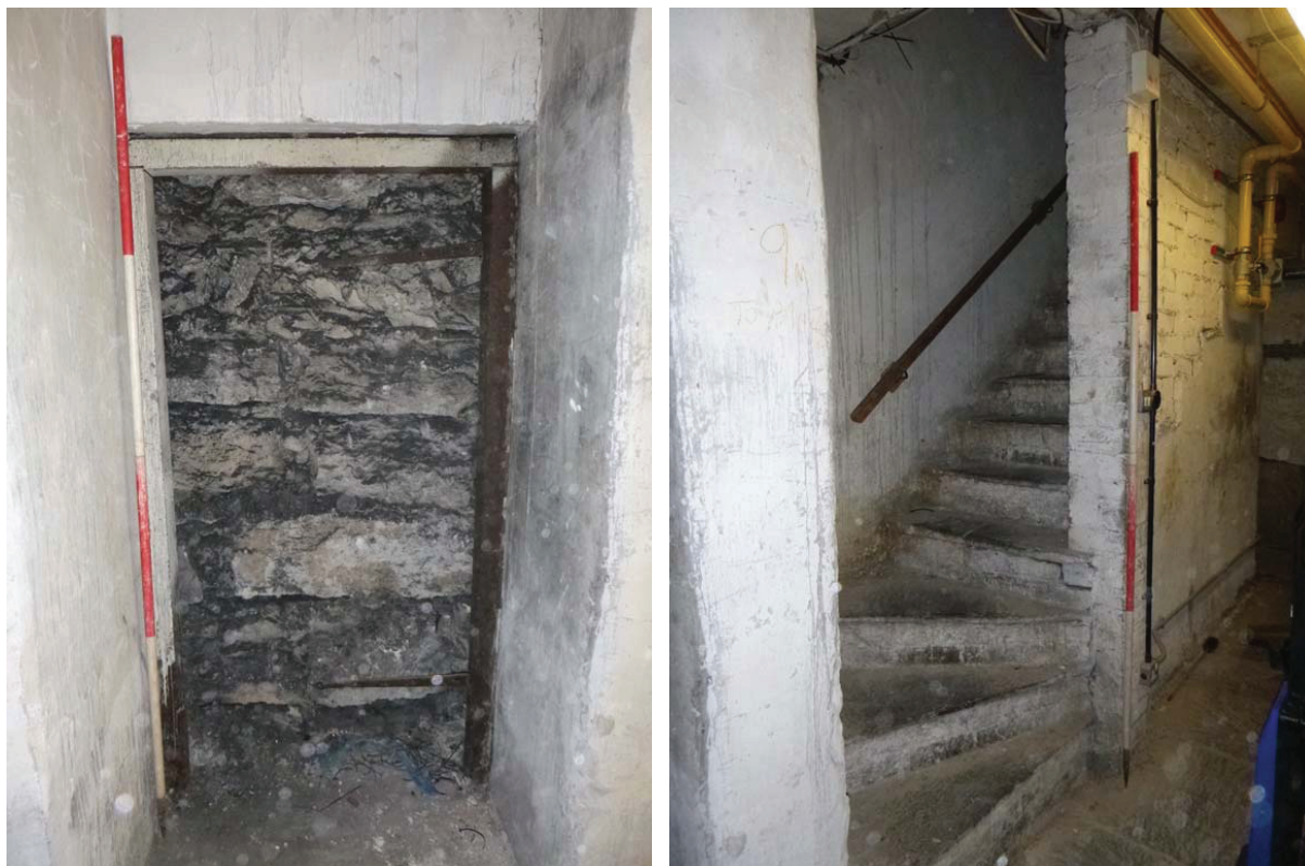
Plate 113 (left): The blocked doorway at the west end of the north elevation of Room B8, viewed from the south
