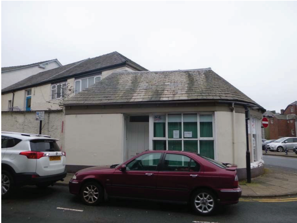
Plate 95: The east end of the south external elevation, viewed from the south
