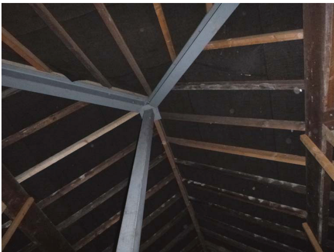
Plate 245 (left): The post and beam structure supporting the roof in Room A11, viewed from below
