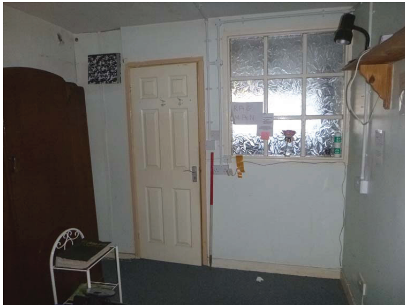
Plate 163: The north elevation of Room G20, viewed from the south
