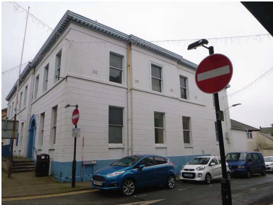
Plate 90: The west end of the south external elevation, viewed from the south-west
