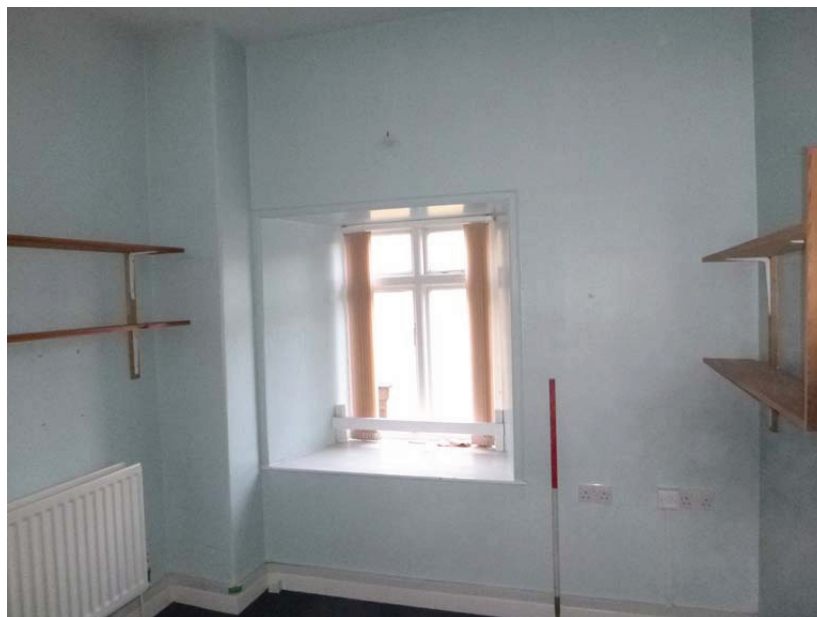
Plate 224: The north elevation of Room F20, viewed from the south-east
