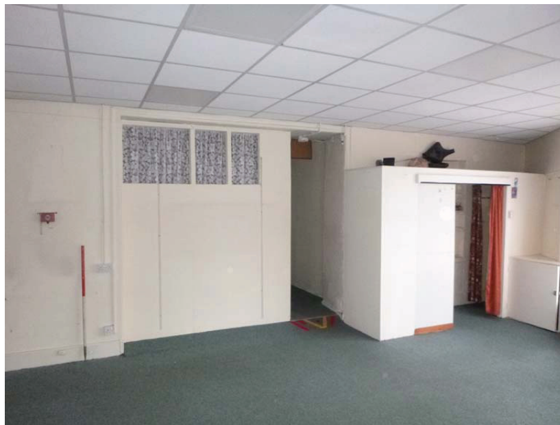
Plate 169: The west elevation of Room G26, viewed from the east
