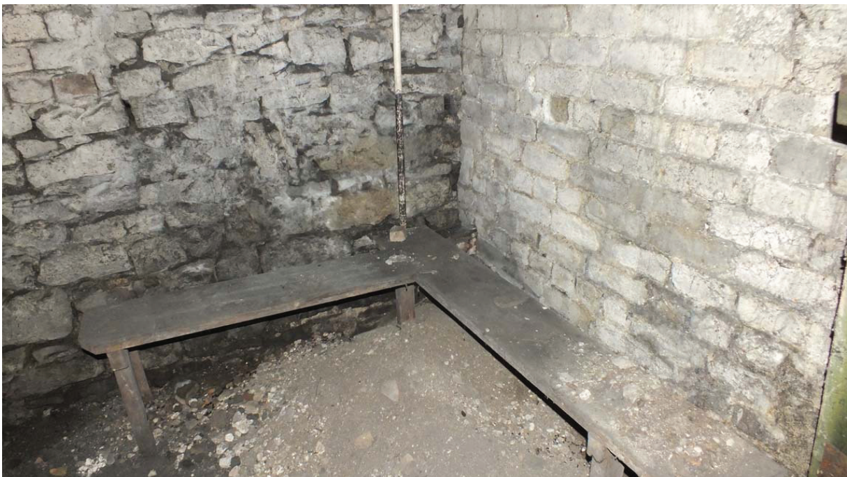
Plate 28: Timber benches in the north-east corner of Cellar B
