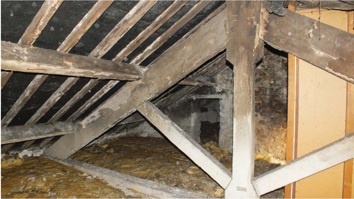
Plate 68: King post truss in the attic above Room F12
