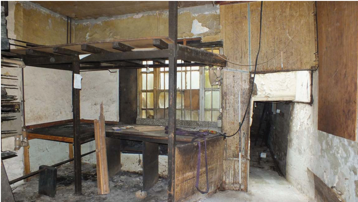
Plate 45: South elevation of Room G7
