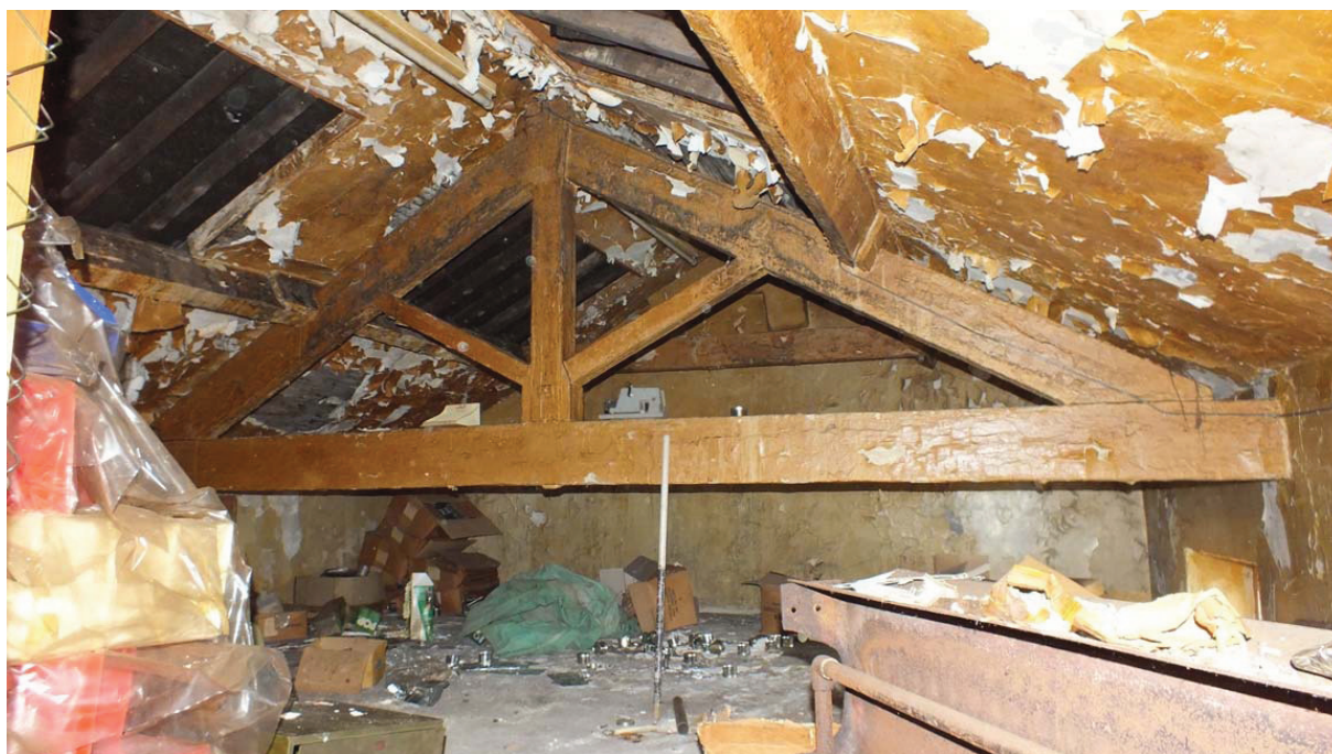
Plate 61: Truss in Room F14a
