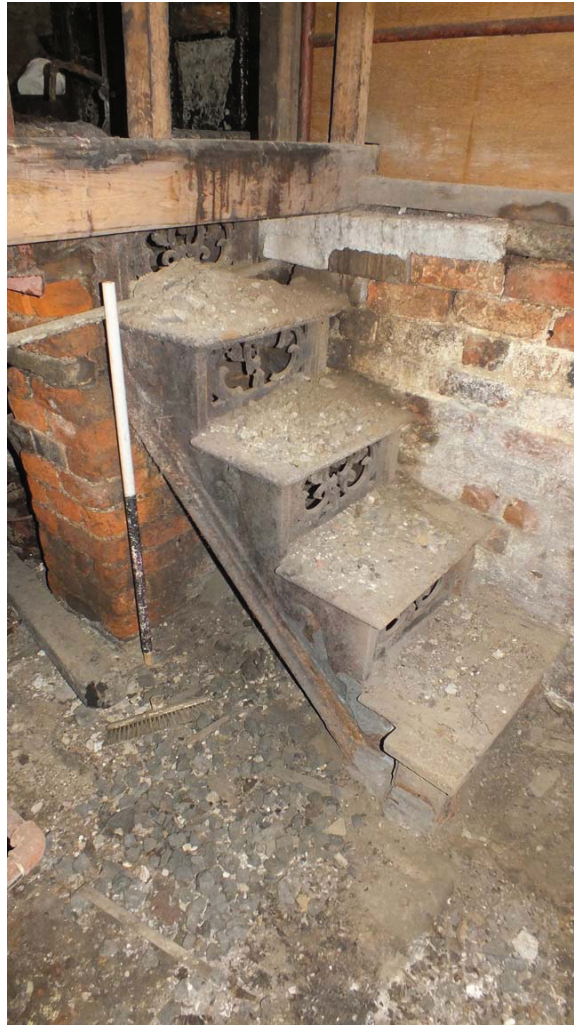
Plate 29: Stairs in cellar C
