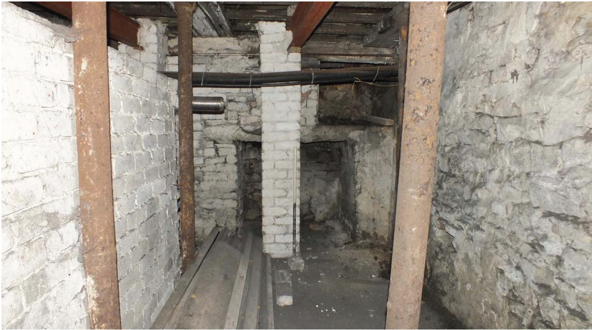
Plate 27: west elevation Cellar B showing columns supporting the ceiling
