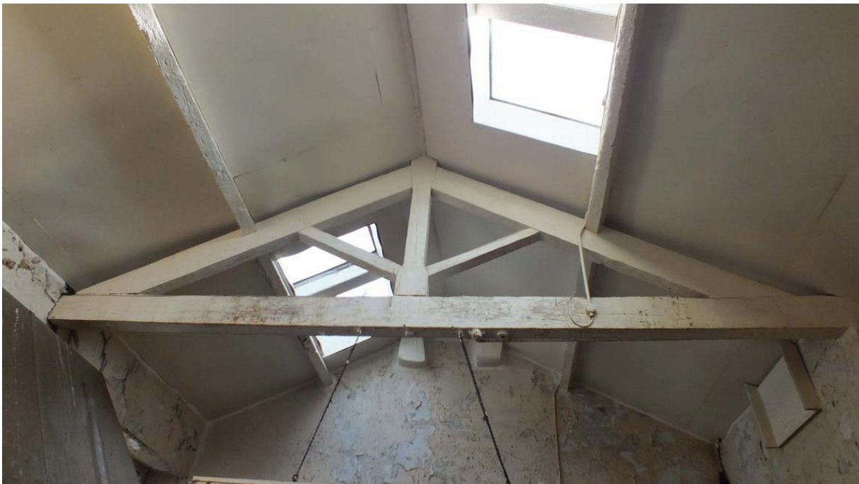
Plate 54: Truss in Room F13
