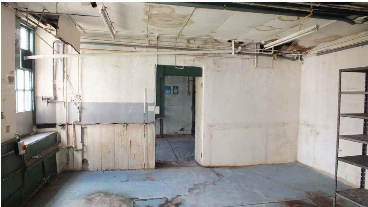
Plate 35: South elevation of Room G3
