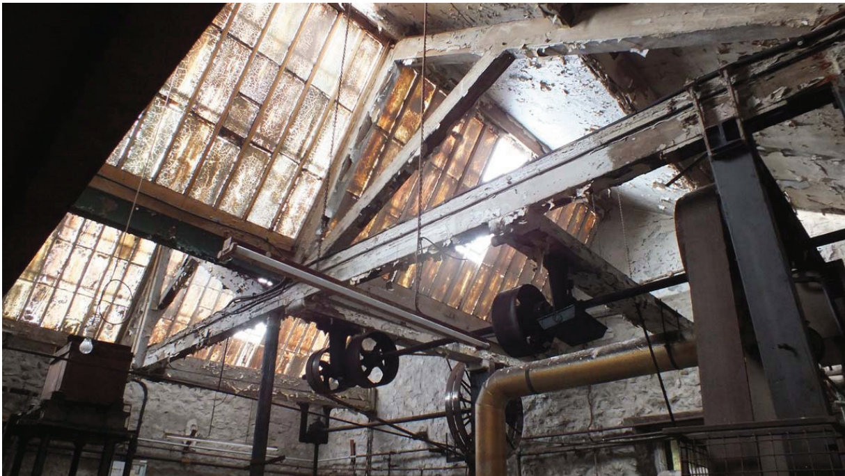
Plate 39: Trusses in Room G6
