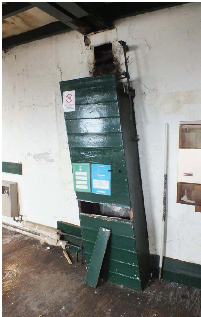
Plate 60: Boxing for former drive belt, west side of Room F14
