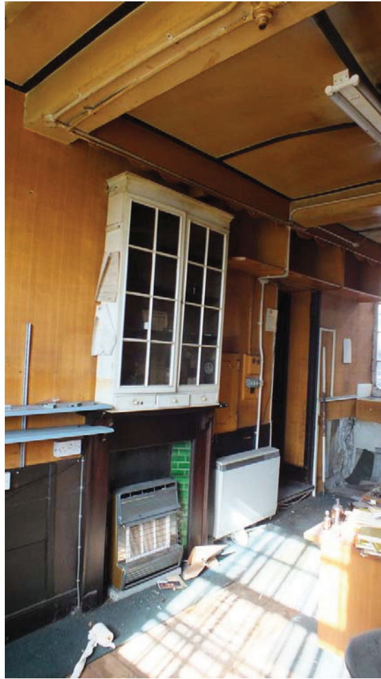
Plate 31: Room G1, west elevation, fireplace and cabinet
