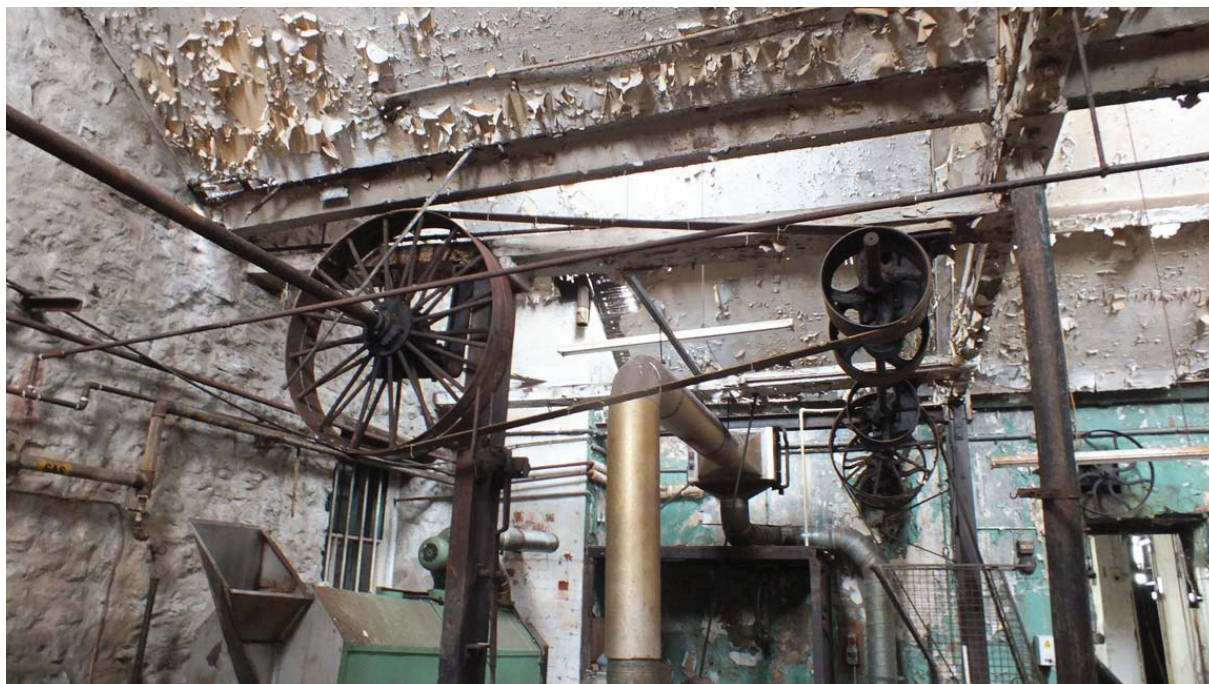
Plate 40: Extant drive shafts and wheels in Room G6
