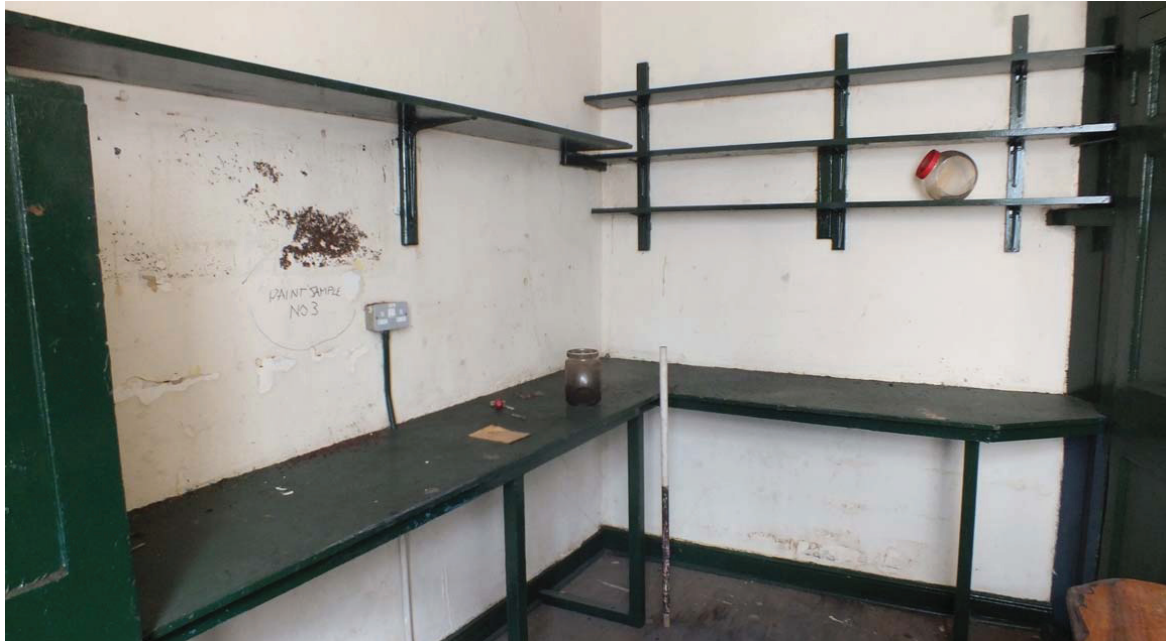
Plate 49: Oblique view of the east and south elevations of Room G10
