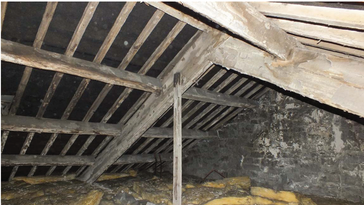
Plate 67: Tie beam truss in the attic above Rooms F17-18
