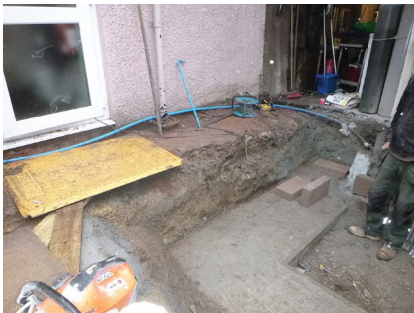
Plate 14: South-facing section in the south-east area of the site
