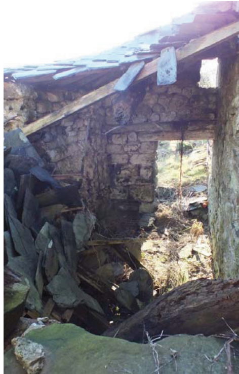
Plate 50: General view of Room G15
