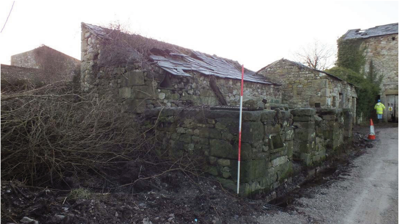
Plate 32: The north external elevation of the north/south block
