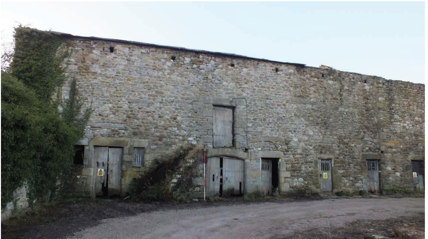
Plate 15: East end of north external elevation of main block
