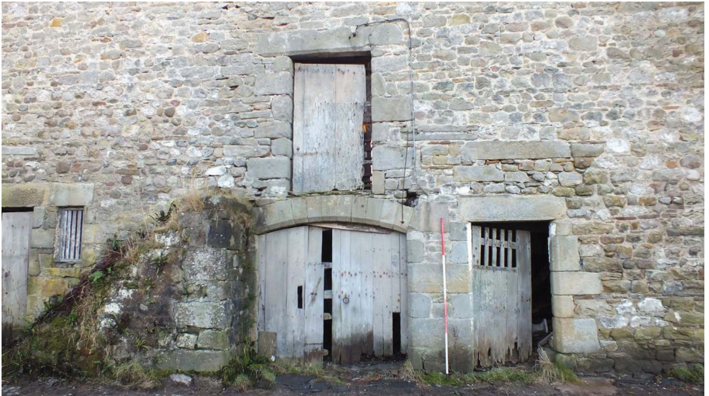
Plate 16: Detail of the wagon doorway and stairs at the east end of the north external elevation of the main block
