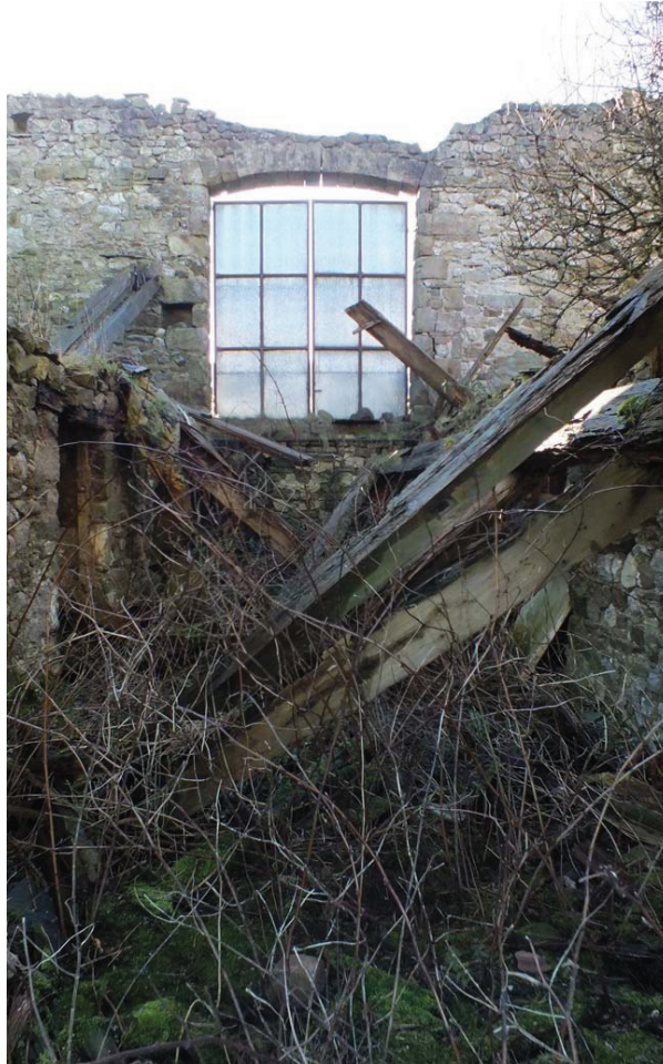
Plate 39: General view of Room G2
