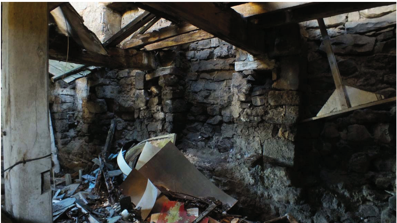
Plate 47: The west elevation of Room G6
