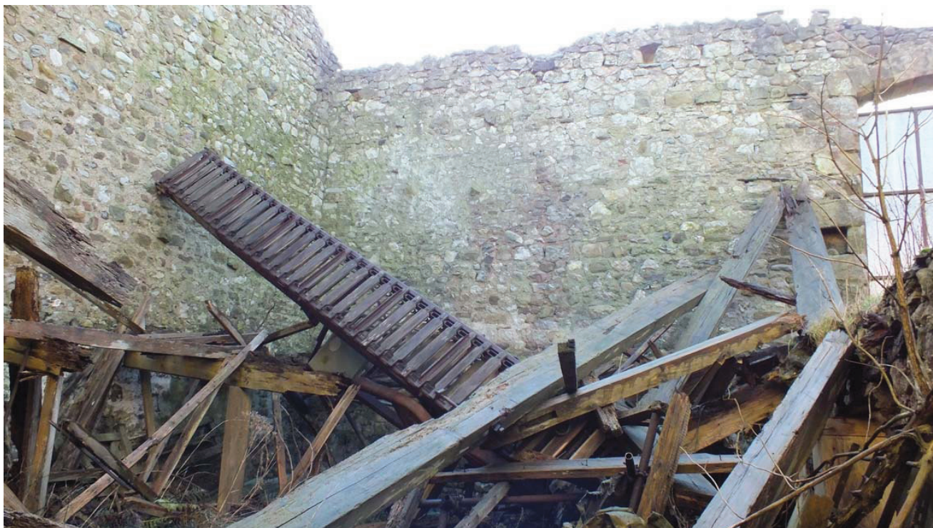
Plate 40: General view of Room G3
