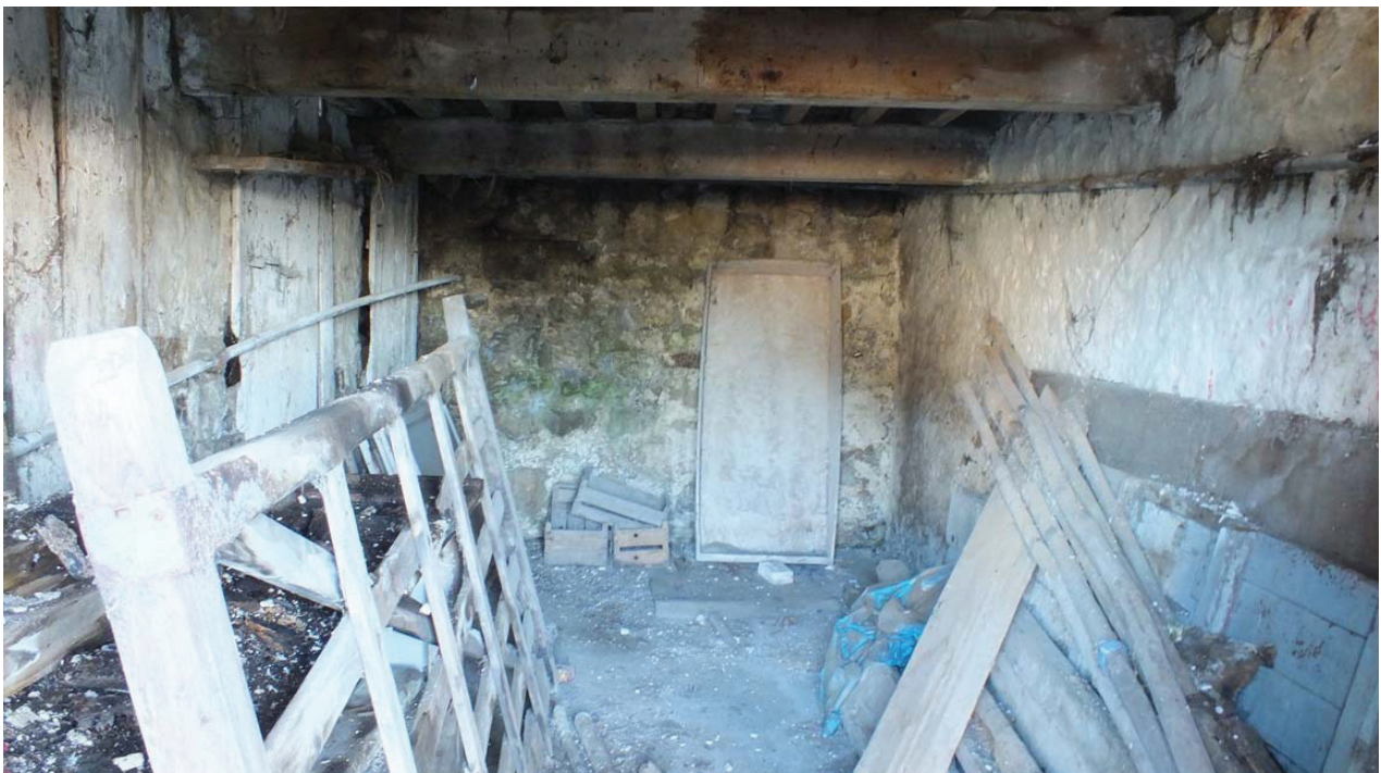
Plate 43: General view of Room G5
