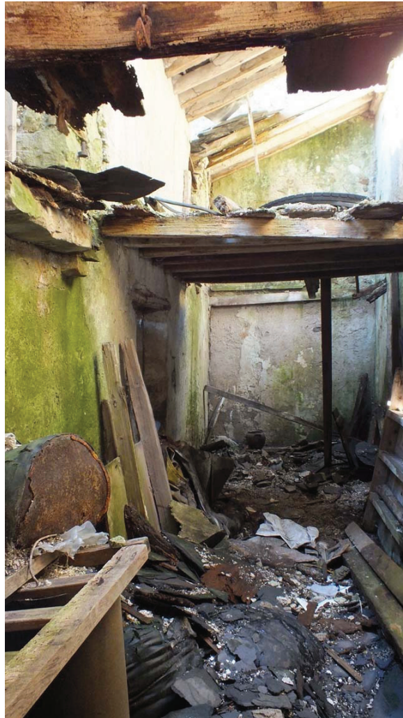
Plate 54: General view of Room F3
