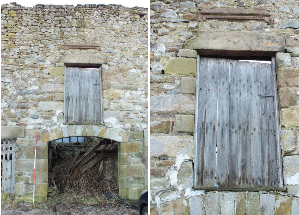
Plate 11: Wagon doorway at west end of north external elevation of main block, with pitching door above
