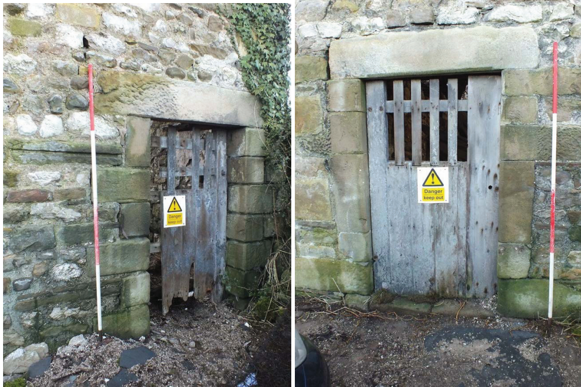
Plate 9 (left): The westernmost door in north external elevation of main block
