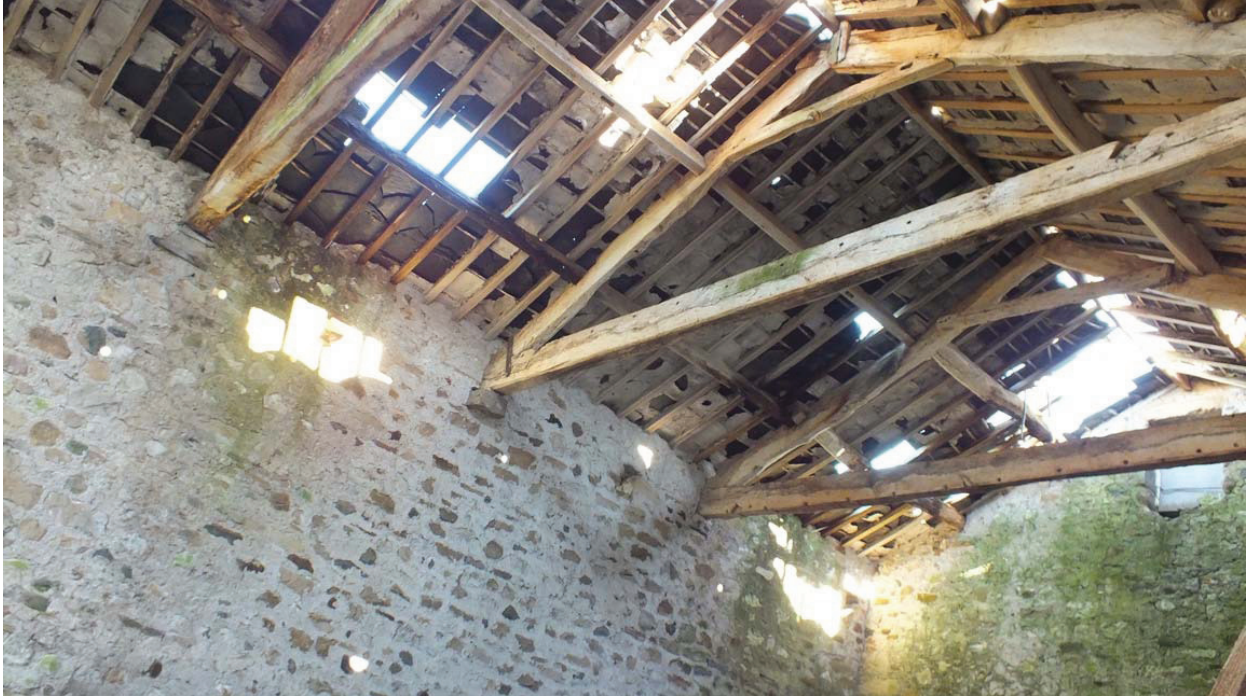
Plate 52: Trusses in Room F2
