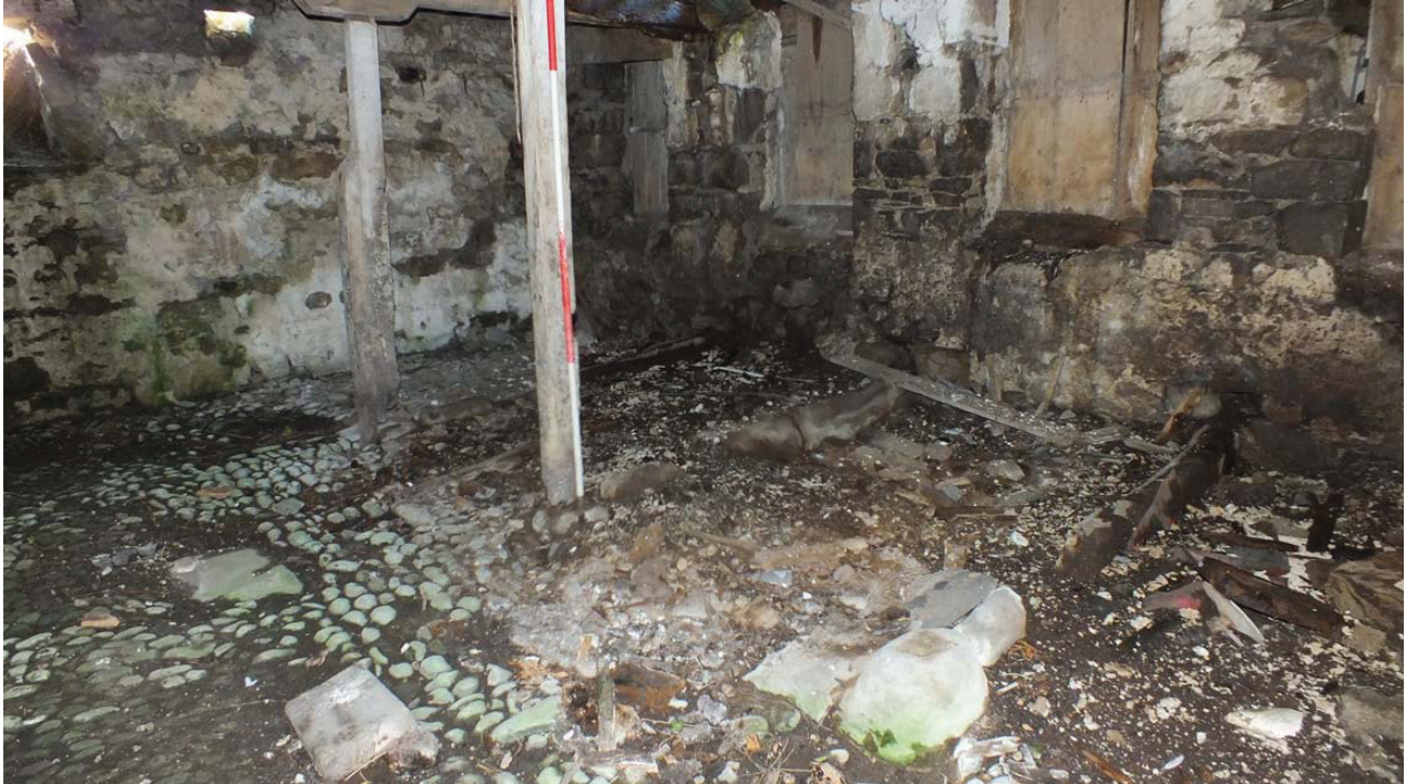
Plate 44: Stall partition bases and cobbled floor on the west side of Room G6
