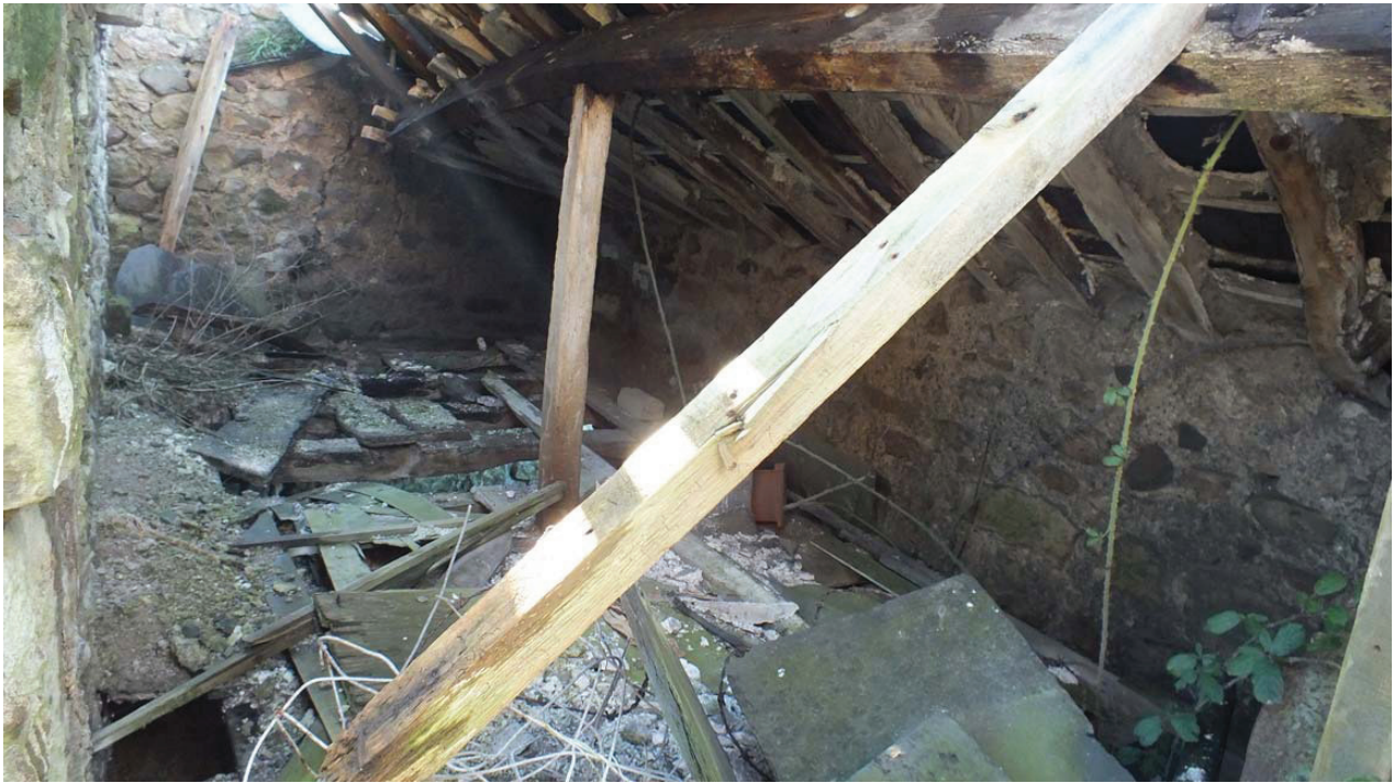
Plate 55: General view of Room F4
