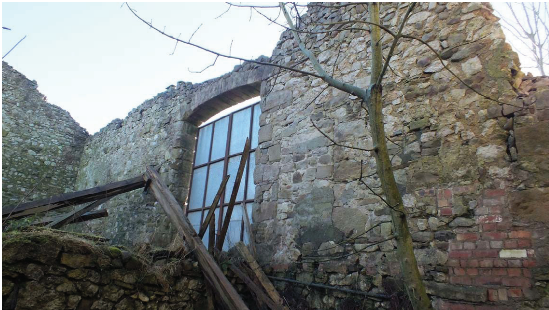
Plate 51: The south internal elevation of Room F1
