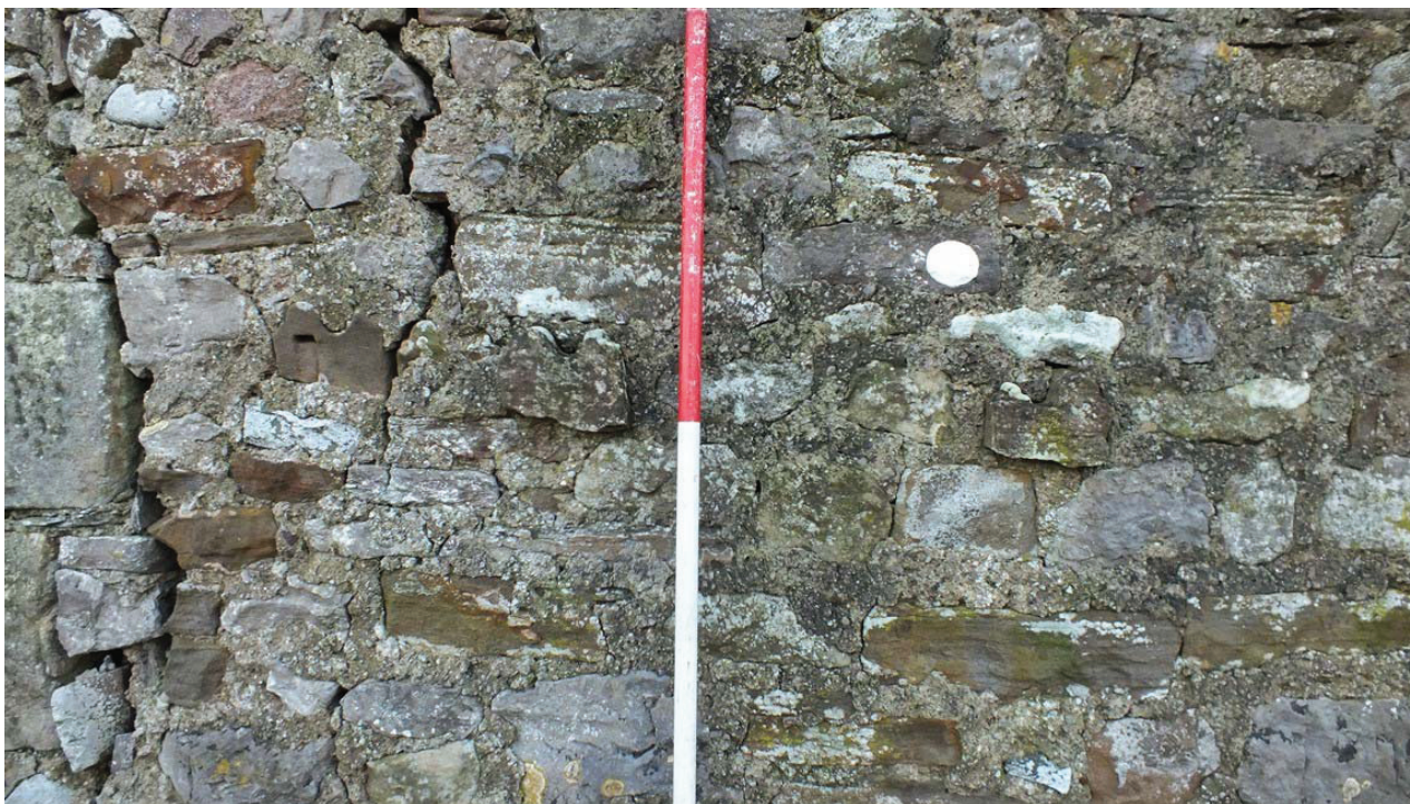
Plate 28: Detail of reused stone in the west external elevation of the main block
