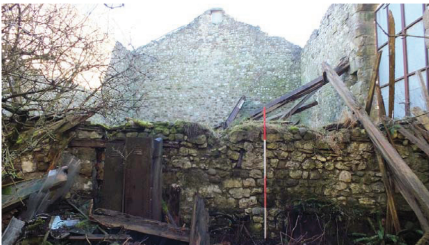
Plate 35 (left): The east internal elevation, Room G1
