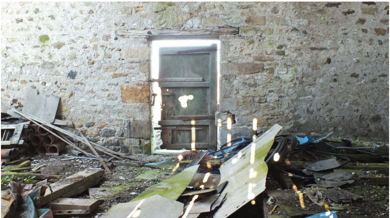
Plate 53: The winnowing door in the north elevation of Room F2
