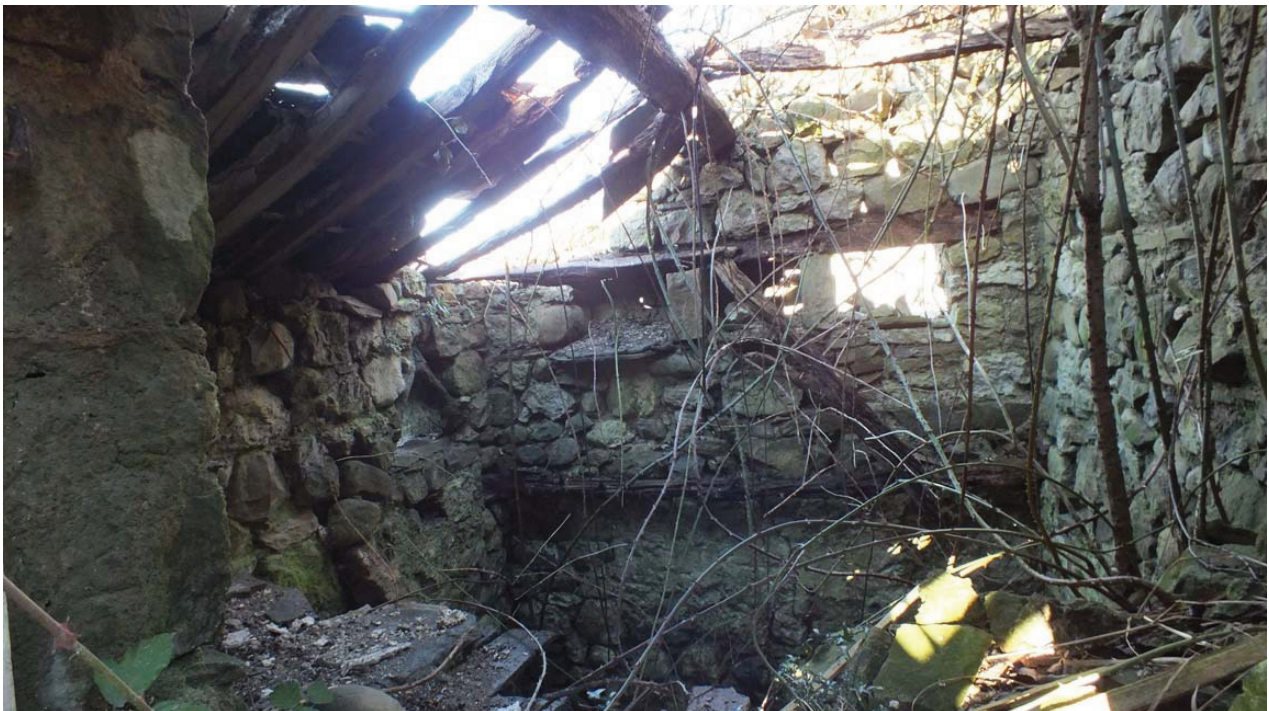
Plate 56: General view of Room F5
