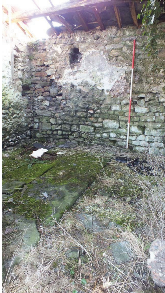
Plate 48: The floor of Room G9 showing the raised floor and channel
