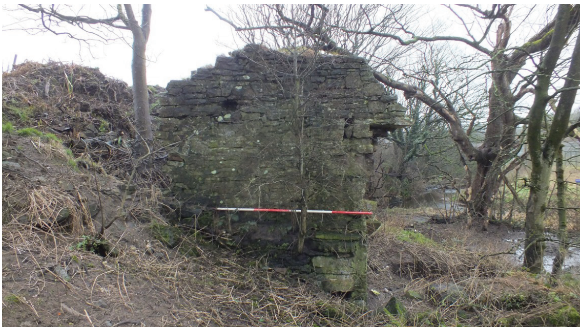
Plate 17: East elevation of Building 2, viewed from the east
