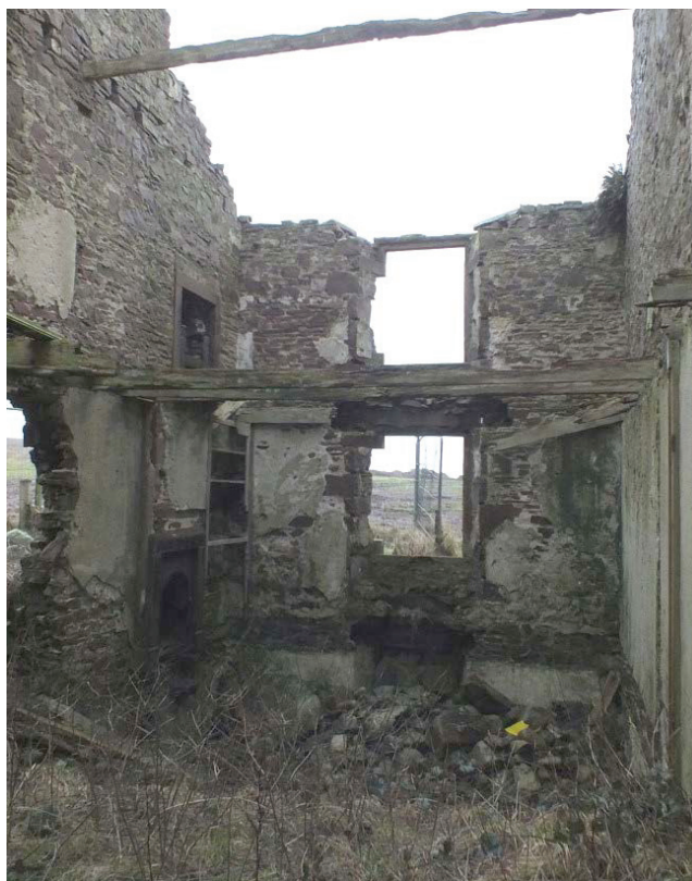
Plate 21: South-west internal elevation of G2, viewed from the north-east
