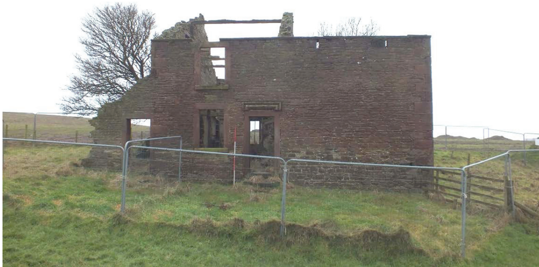
Plate 6: North-east external elevation of Building 1
