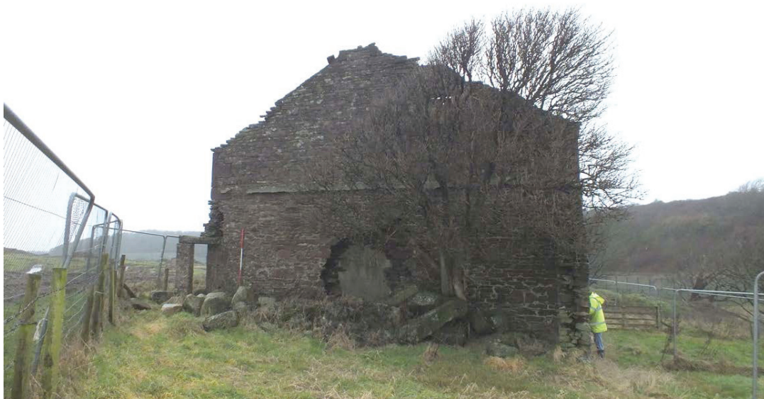
Plate 9: South-east external elevation of Building 1
