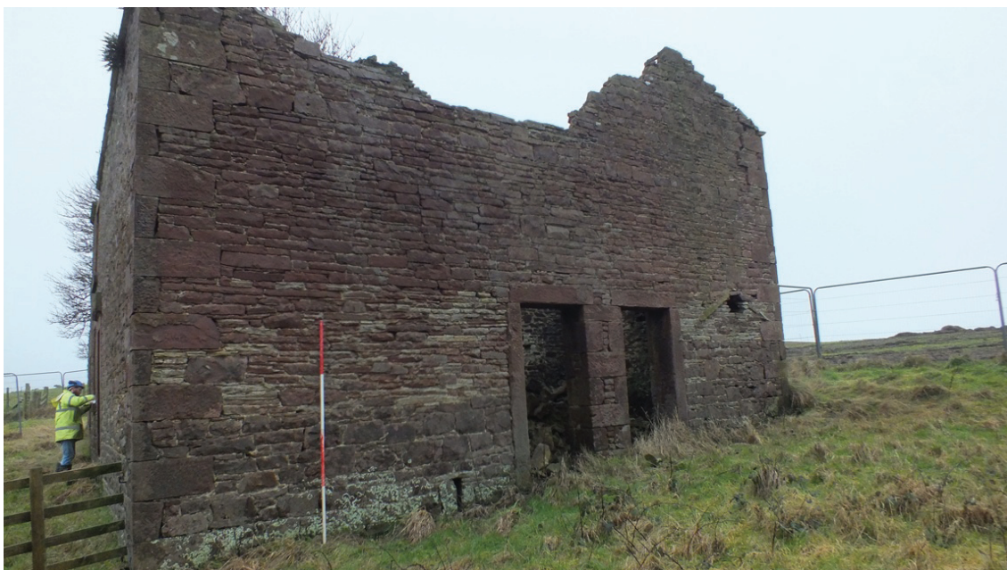
Plate 12: North-west external elevation of Building 1, viewed from the north
