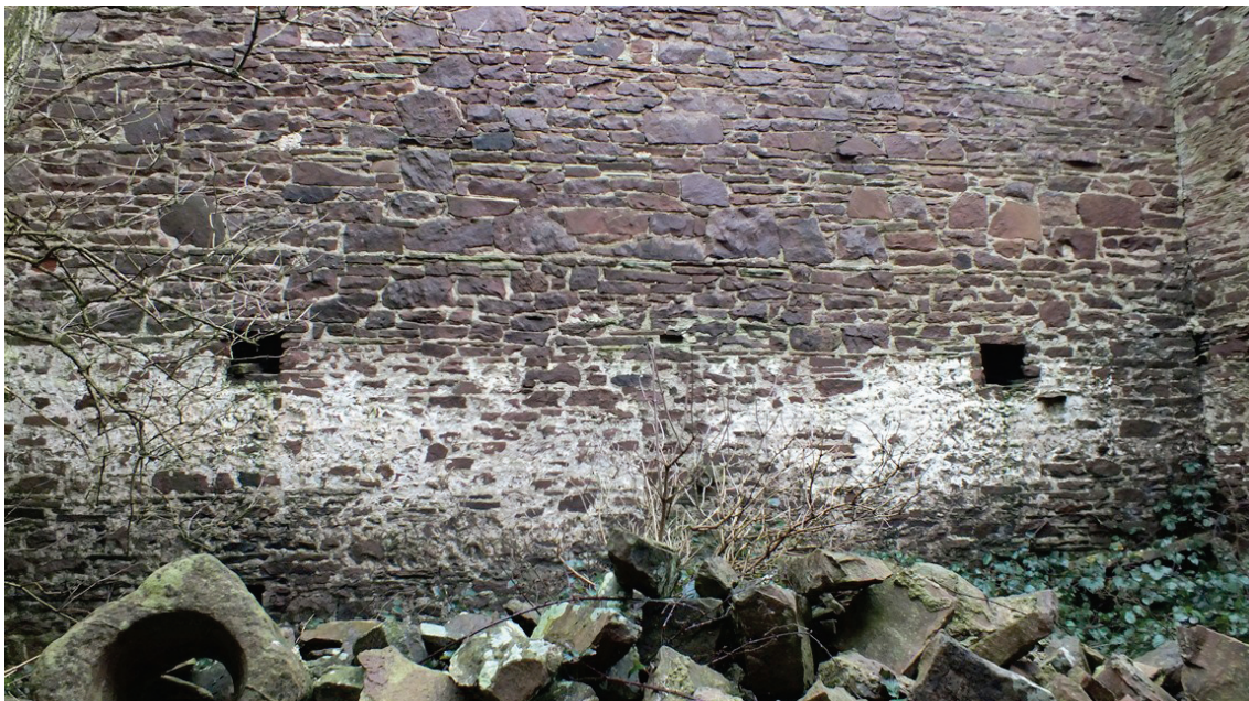
Plate 25: South-east internal elevation of G3, viewed from the north-west
