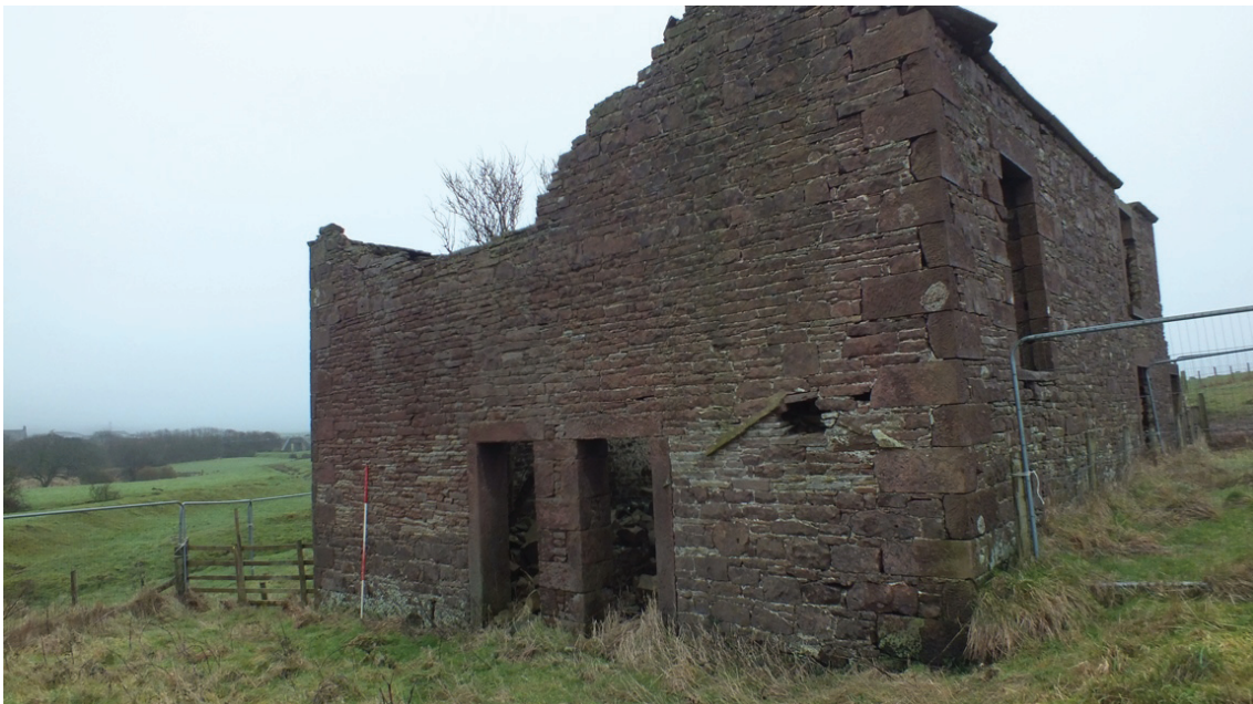
Plate 11: North-west external elevation of Building 1, viewed from the west
