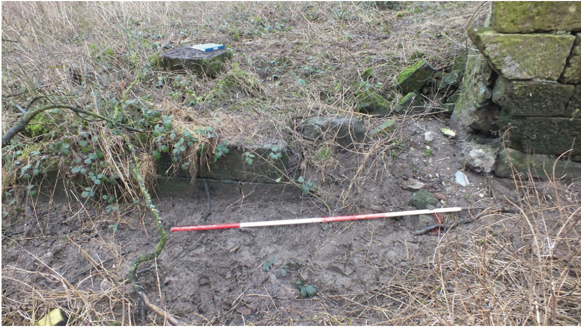
Plate 15: North end of the west elevation of Building 2 and the west wall of the wheel pit, viewed from the west
