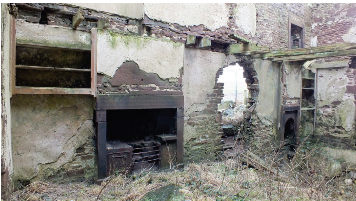
Plate 22: South-east internal elevation of G2, viewed from the north-west
