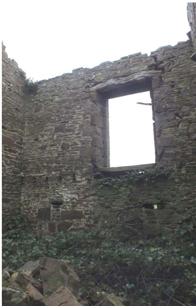
Plate 26: South-west internal elevation of G3, viewed from the north
