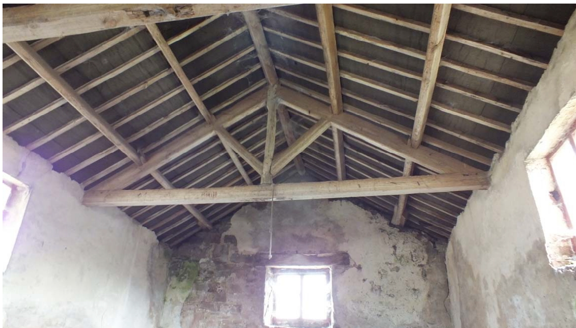
Plate 14: Eastern truss, viewed from the west
