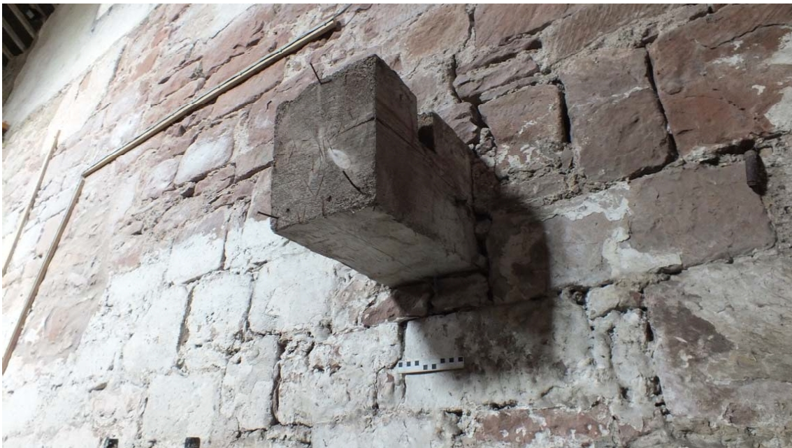
Plate 17: Remains of early beam projecting from the north internal elevation, viewed from the south-east
