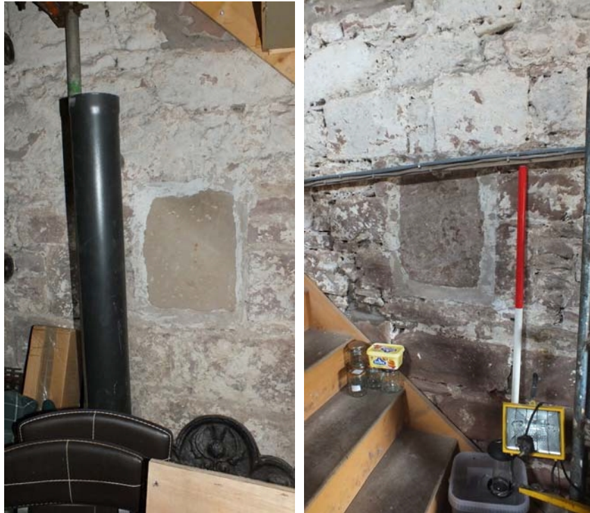
Plate 15 (left): Aperture blocked with a single slab on the west side of the ground floor of the north internal elevation, viewed from the south
