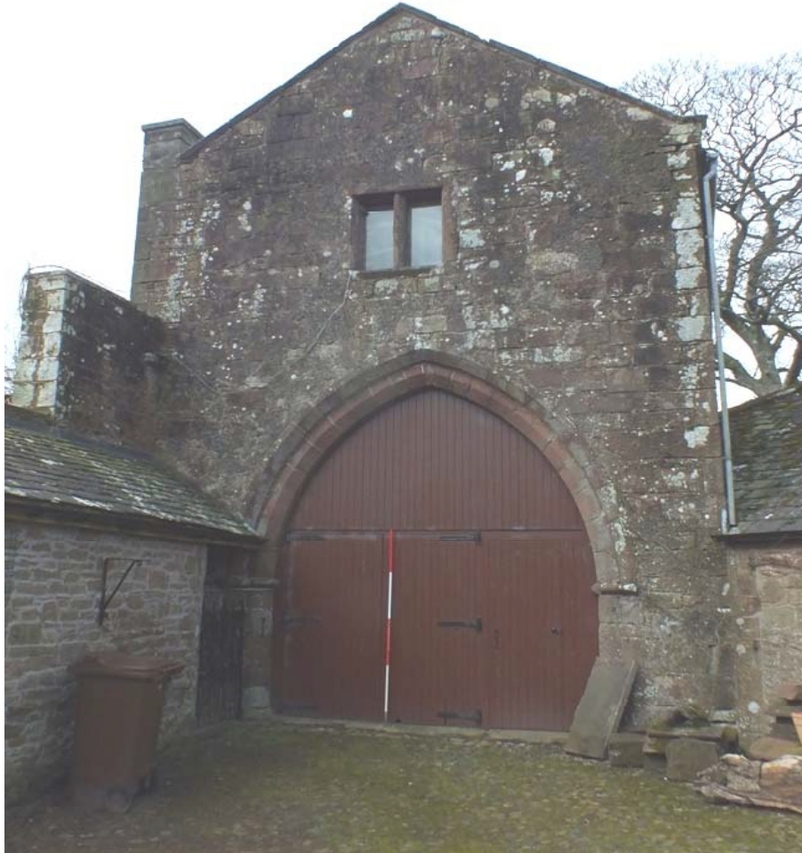
Plate 10: General view of the east external elevation, viewed from the east
