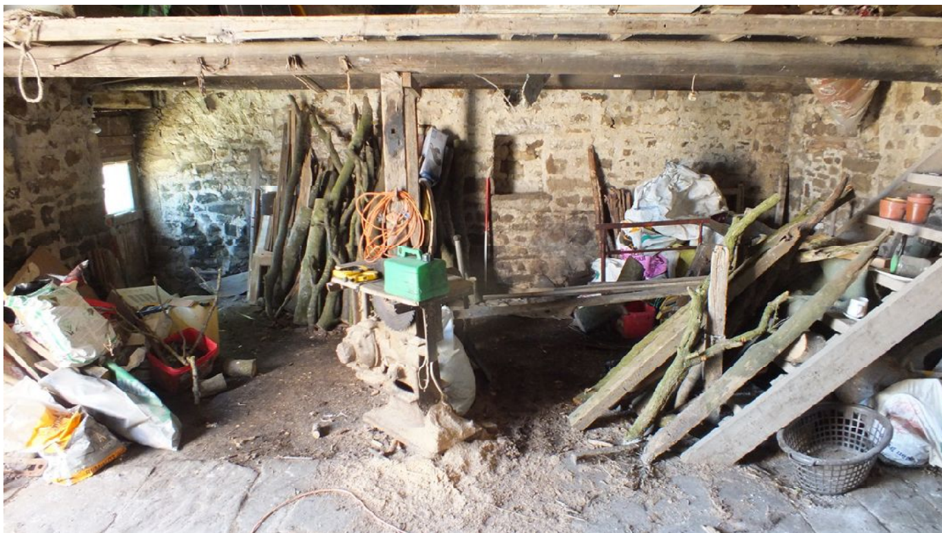
Plate 67: The south-east internal elevation of Barn 3 at ground floor level
