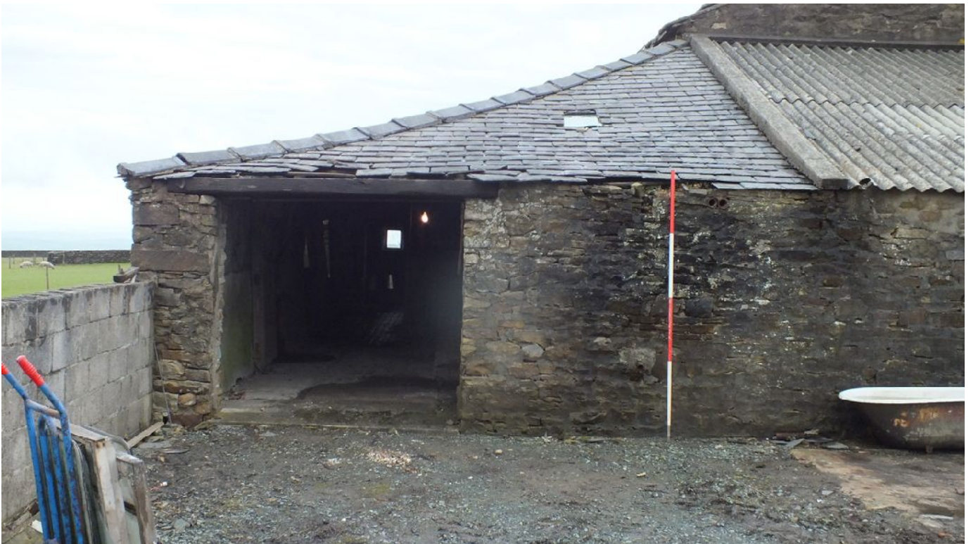
Plate 14: South-east external elevation of Barn 1
