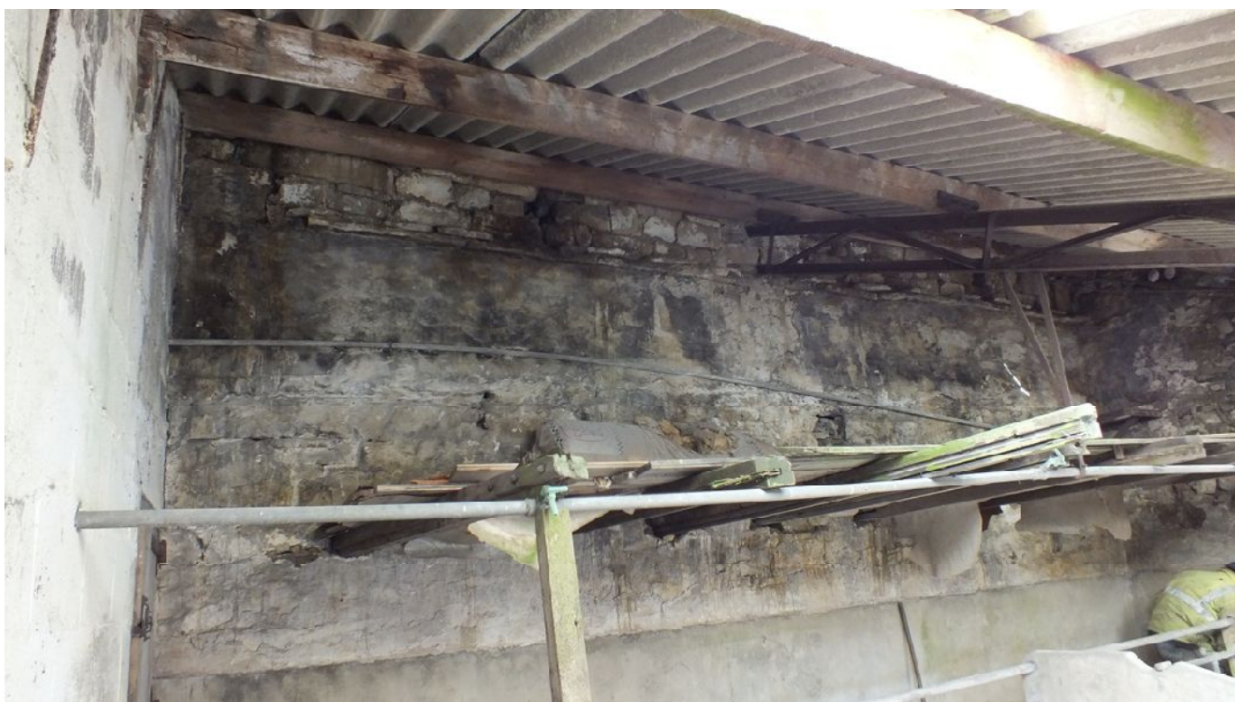
Plate 47: Hayloft and throughstones in the north-west internal elevation of Barn 2
