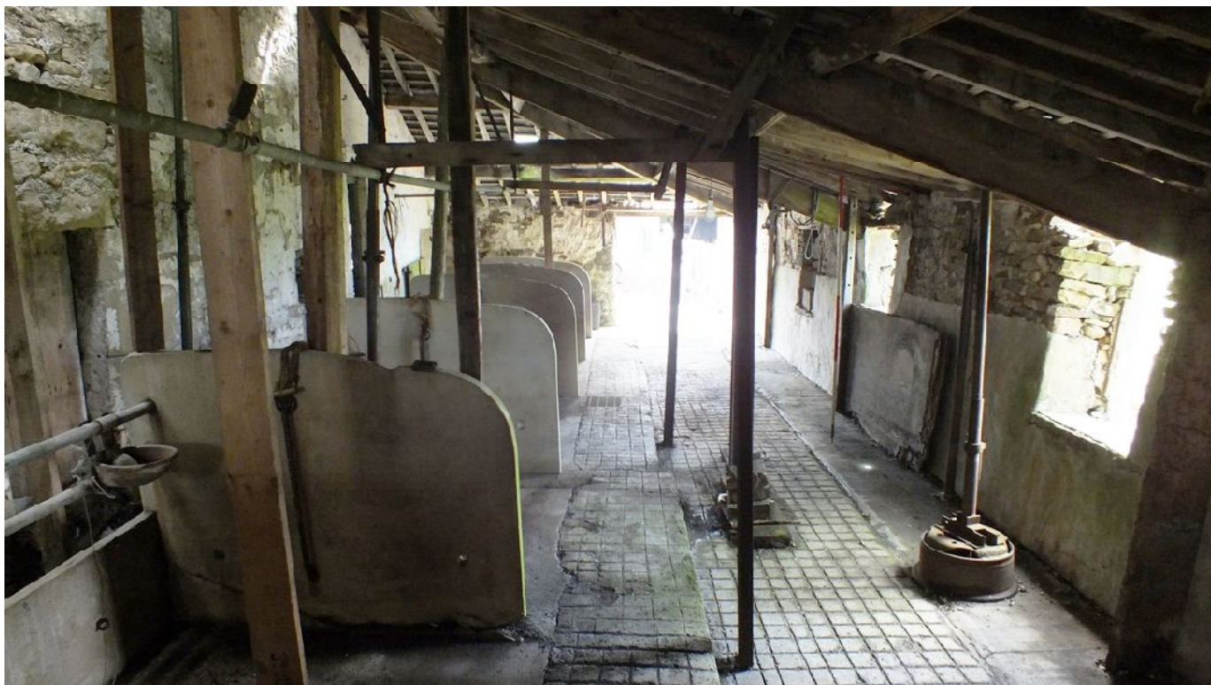
Plate 42: General view of Barn 1 from the north-west end
