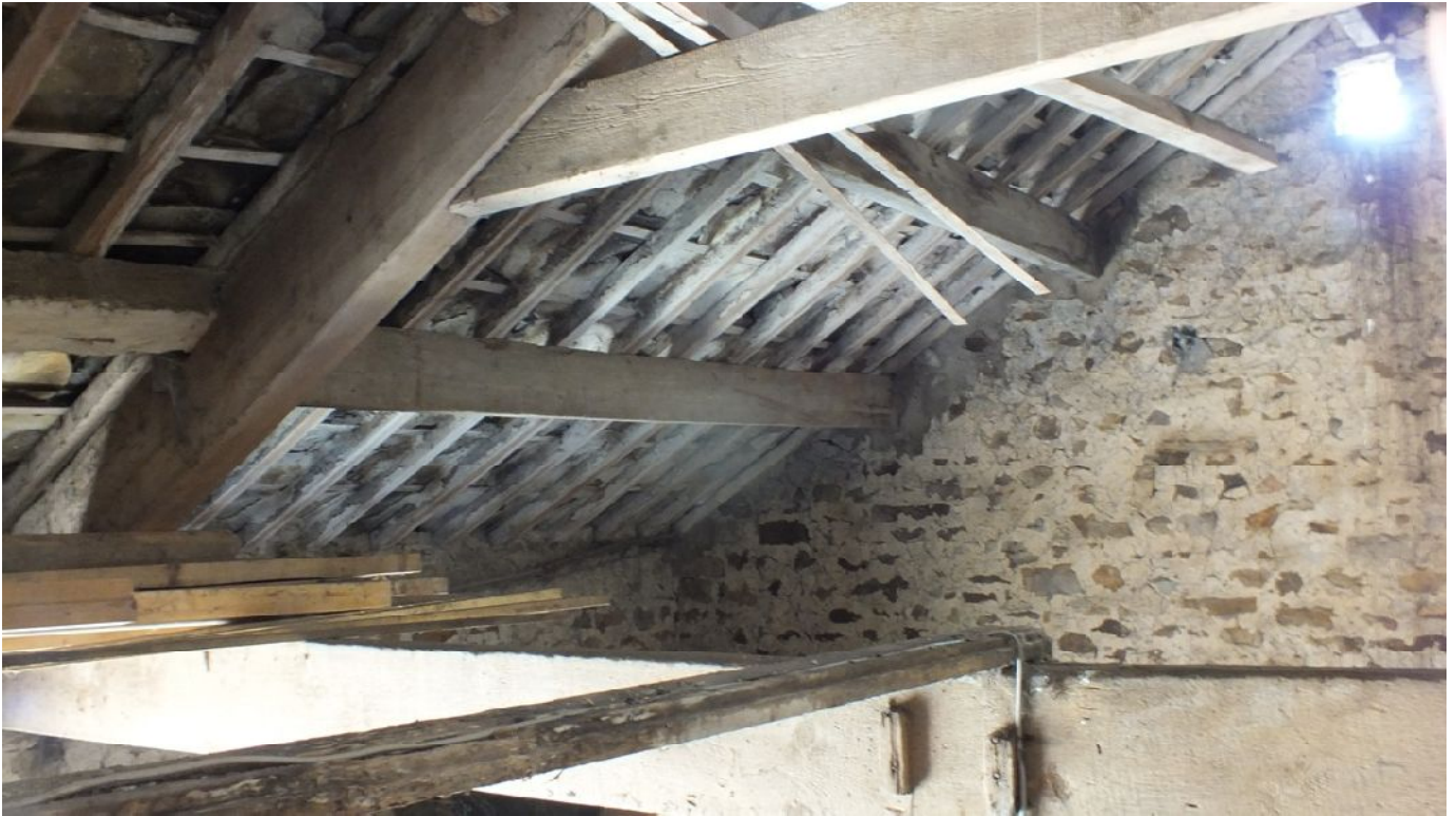
Plate 55: Replacement purlins at the south-east end of Barn 3
