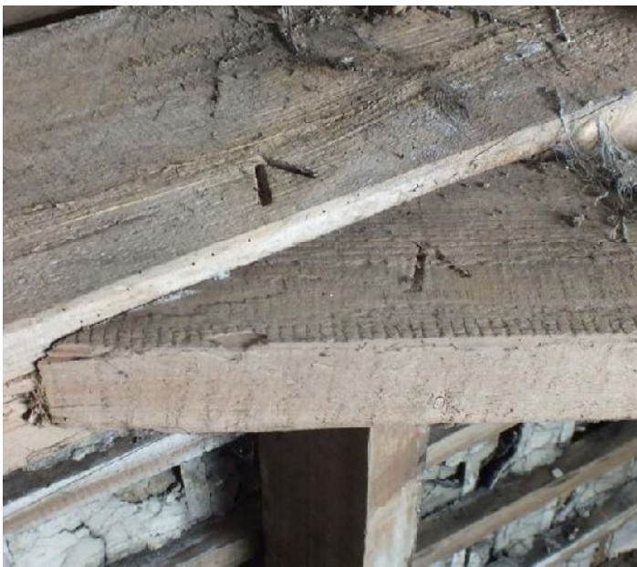
Plate 56 (left): Carpenter's mark on the north-west truss in Barn 3
