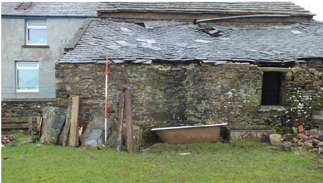
Plate 18: North-west end of the south-west external elevation
