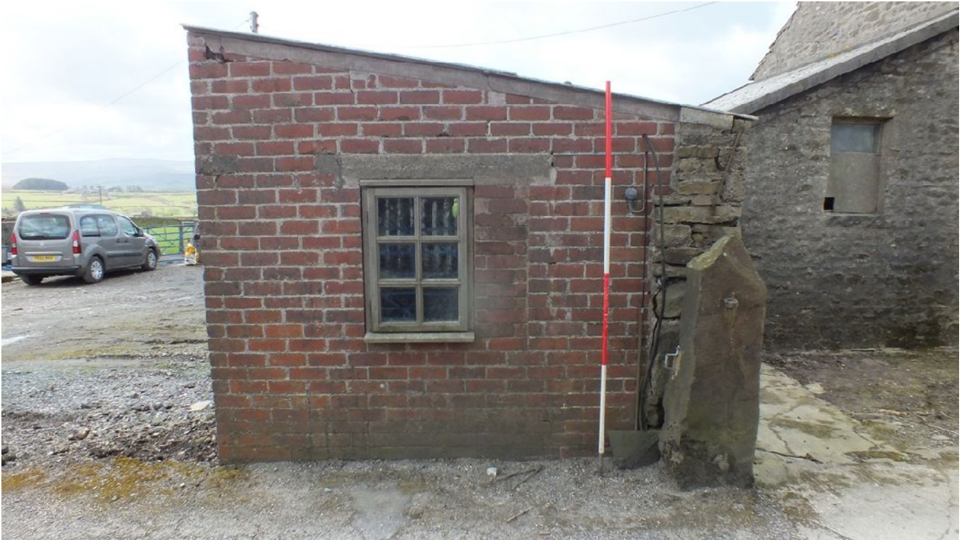
Plate 10: North-east external elevation of the outshut
