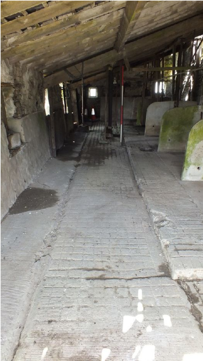
Plate 26 (left): Gridded concrete in the dung channel along the south-west side of Barn 1
