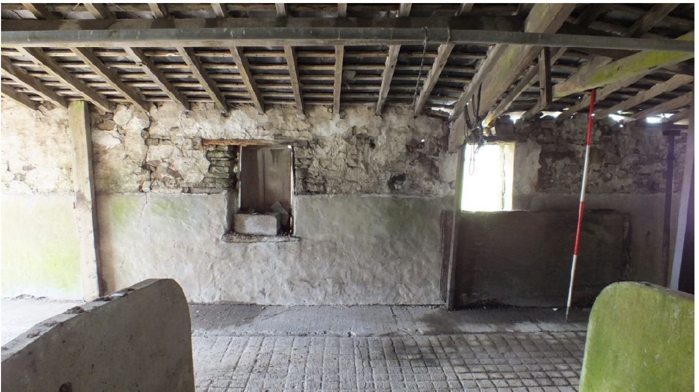
Plate 41: South-east end of the south-west internal elevation of Barn 1
