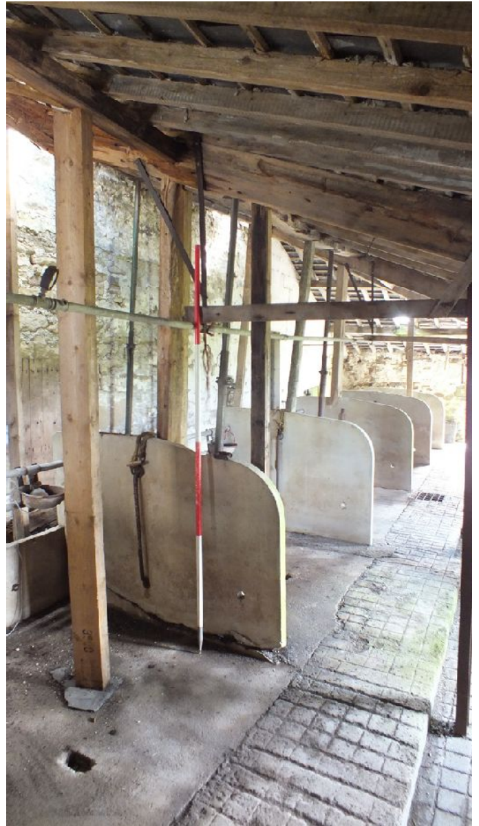
Plate 26 (left): Gridded concrete in the dung channel along the south-west side of Barn 1
