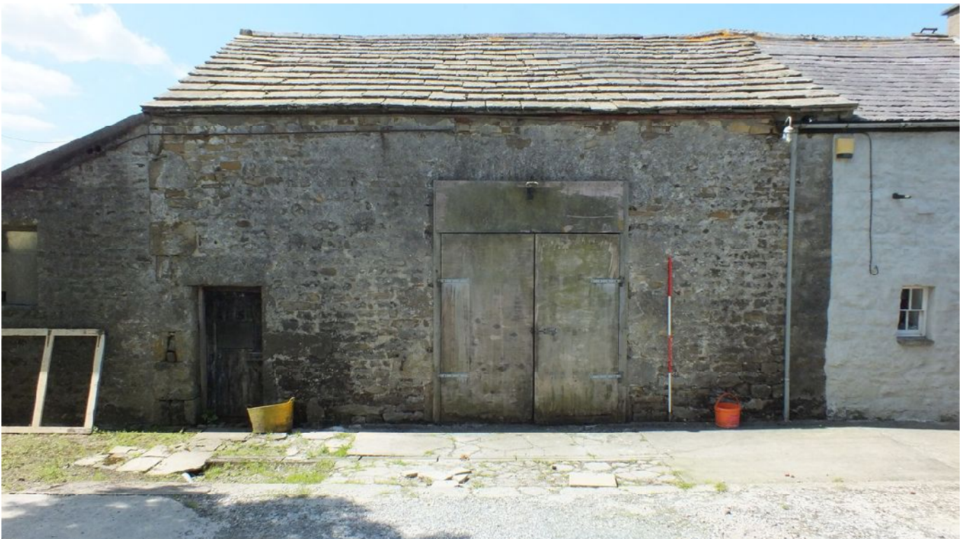
Plate 11: The north-east external elevation of Barn 3
