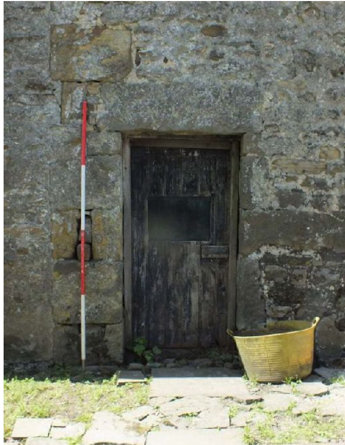
Plate 12: South-east doorway in the north-east external elevation of Barn 3
