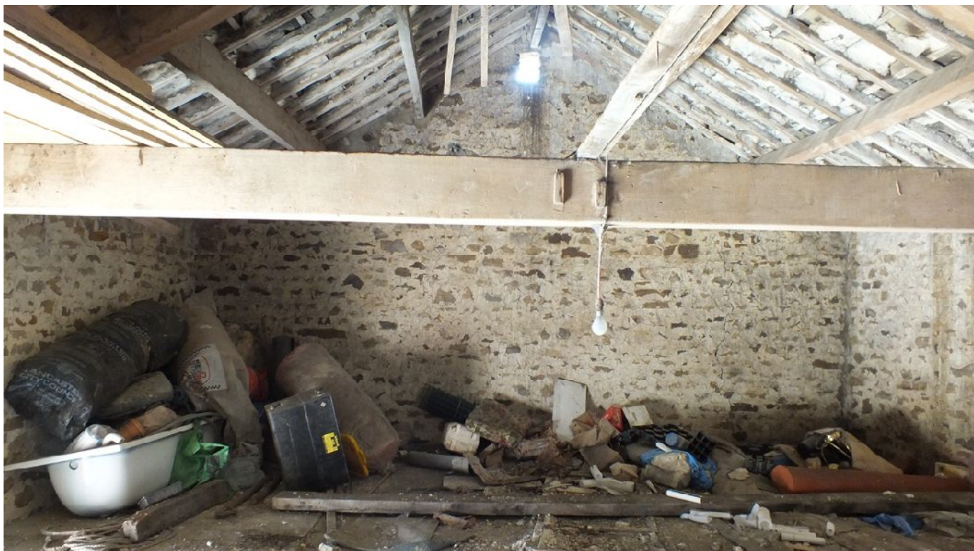
Plate 70: The south-east internal elevation of Barn 3 at the upper floor level
