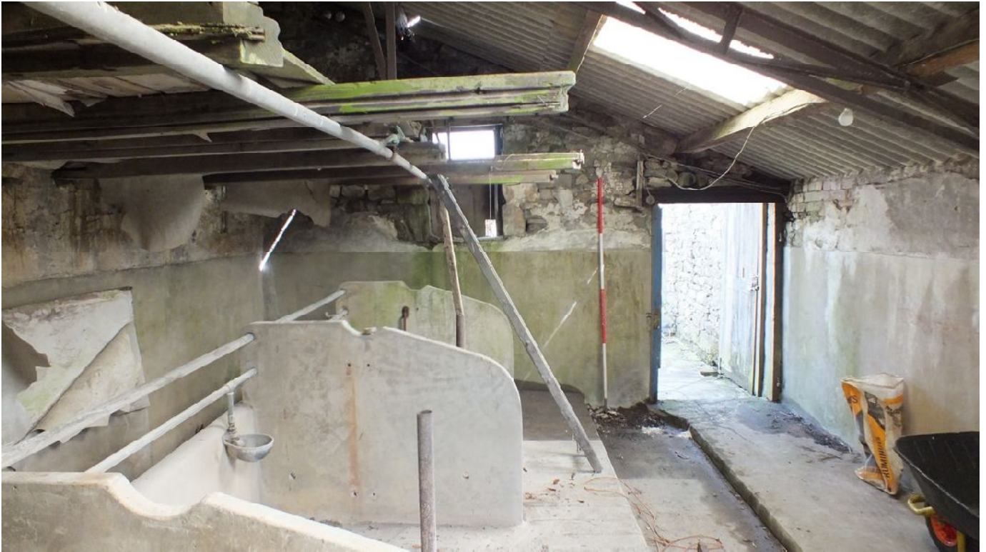
Plate 48: North-east internal elevation of Barn 2
