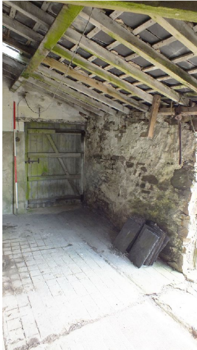
Plate 39: North-east side of the south-east internal elevation of Barn 1
