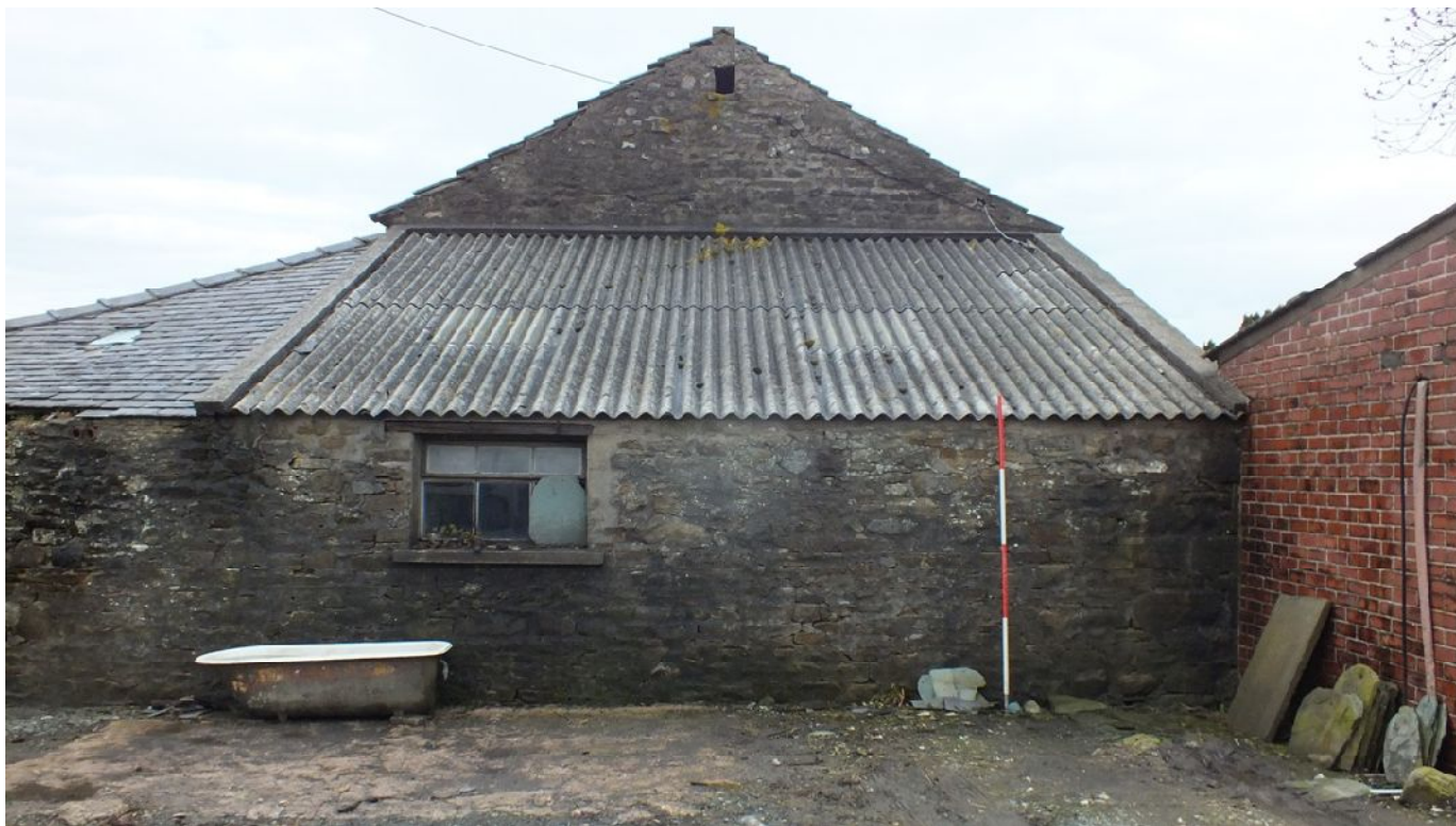
Plate 15: South-east external elevation of Barn 2
