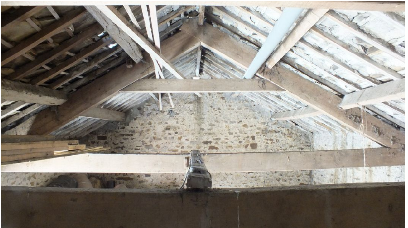
Plate 52: The south-east truss in Barn 3
