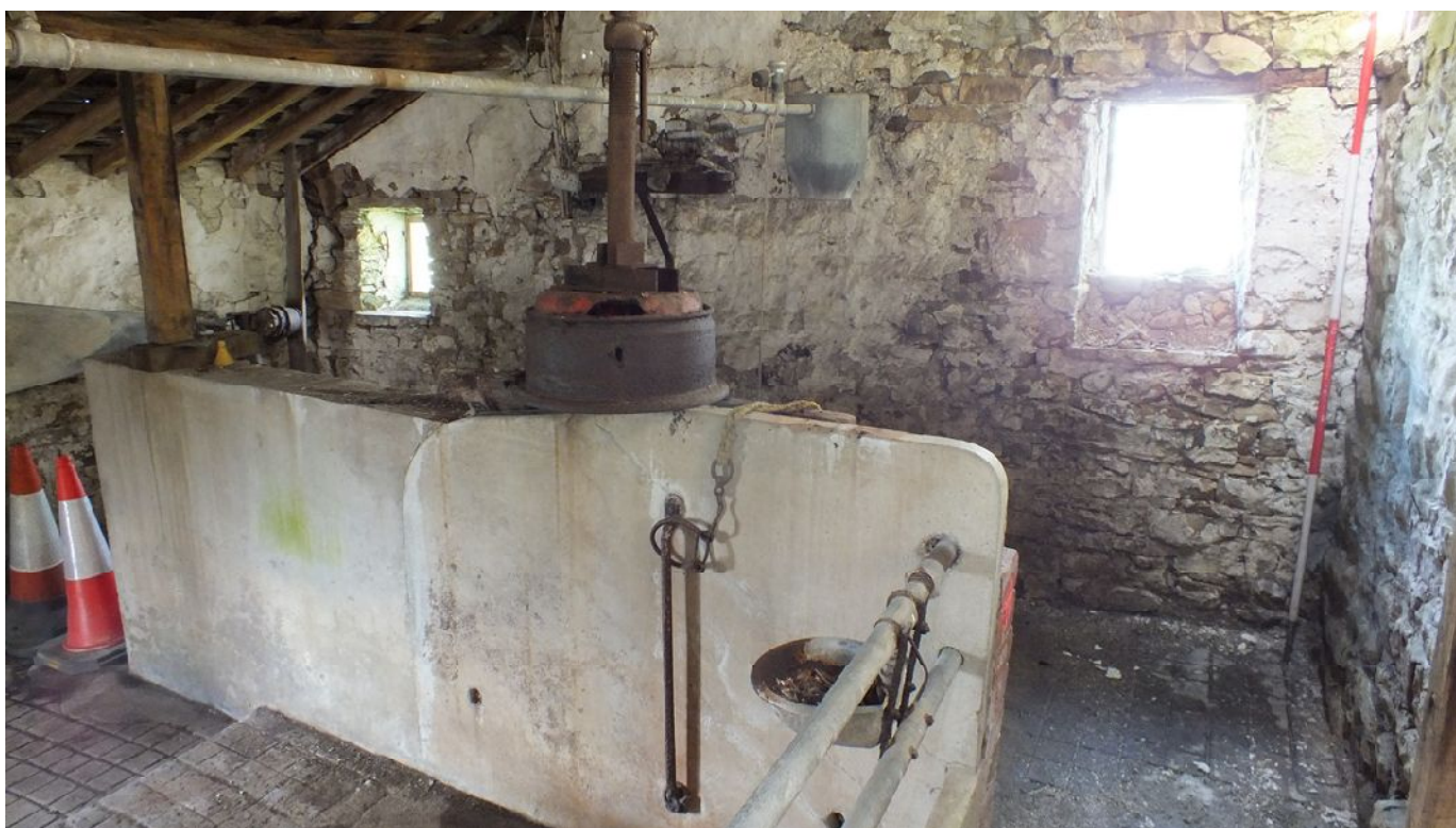
Plate 29: North-west internal elevation of Barn 1
