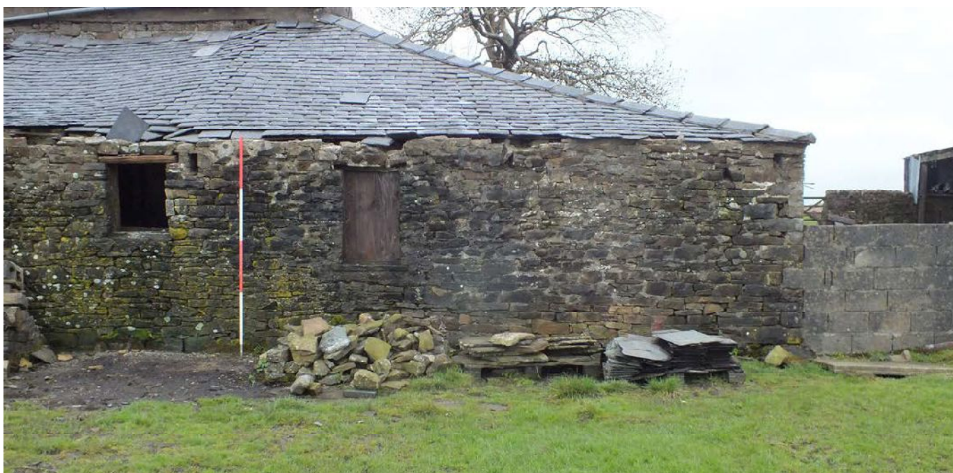
Plate 20: South-east end of the south-west external elevation
