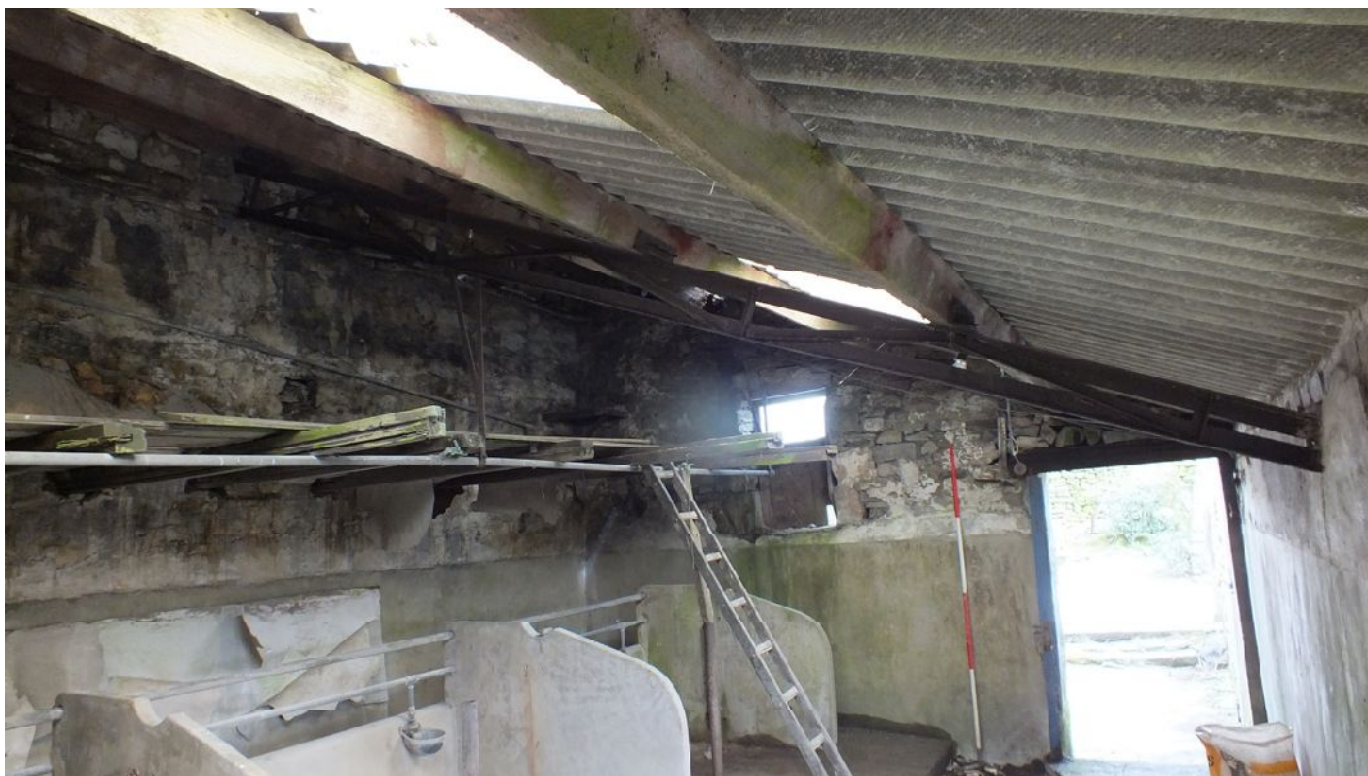
Plate 43: South-west side of the metal beam support in Barn 2
