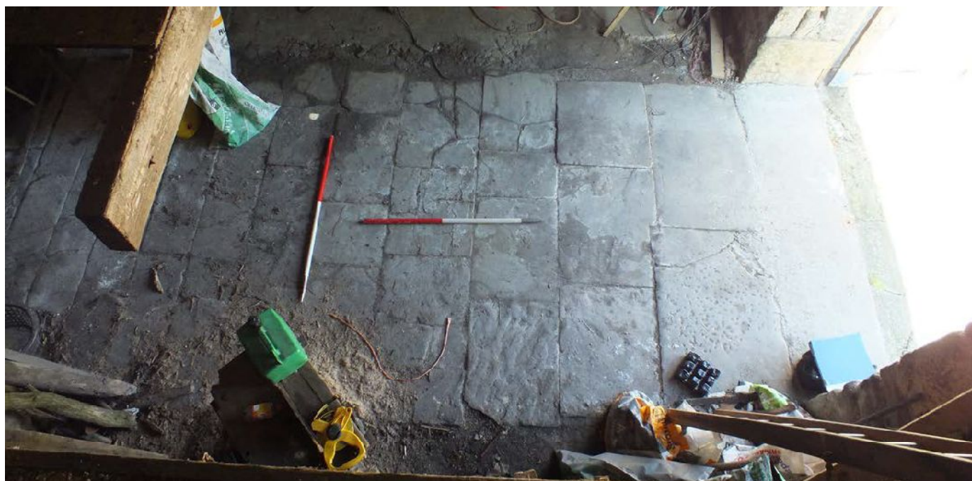
Plate 59: Stone threshing floor in Barn 3, viewed from above
