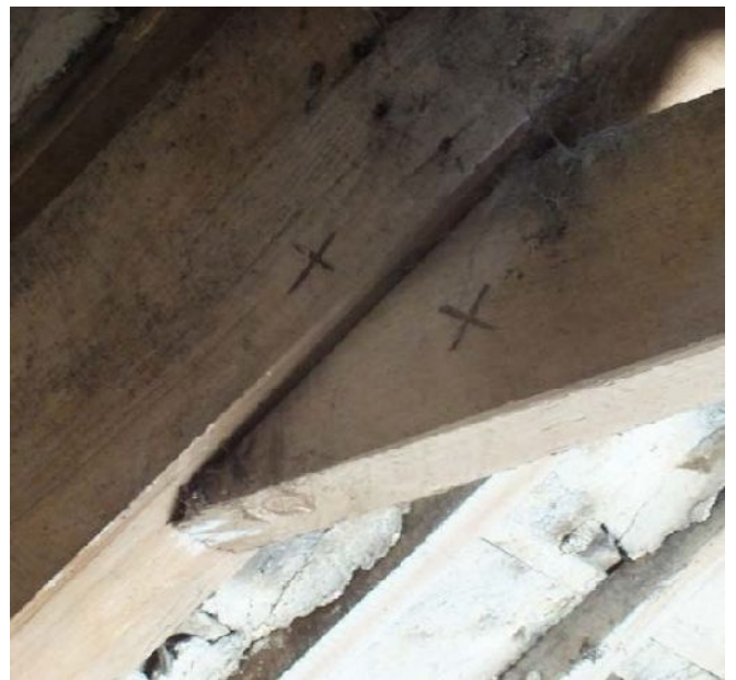
Plate 56 (left): Carpenter's mark on the north-west truss in Barn 3
