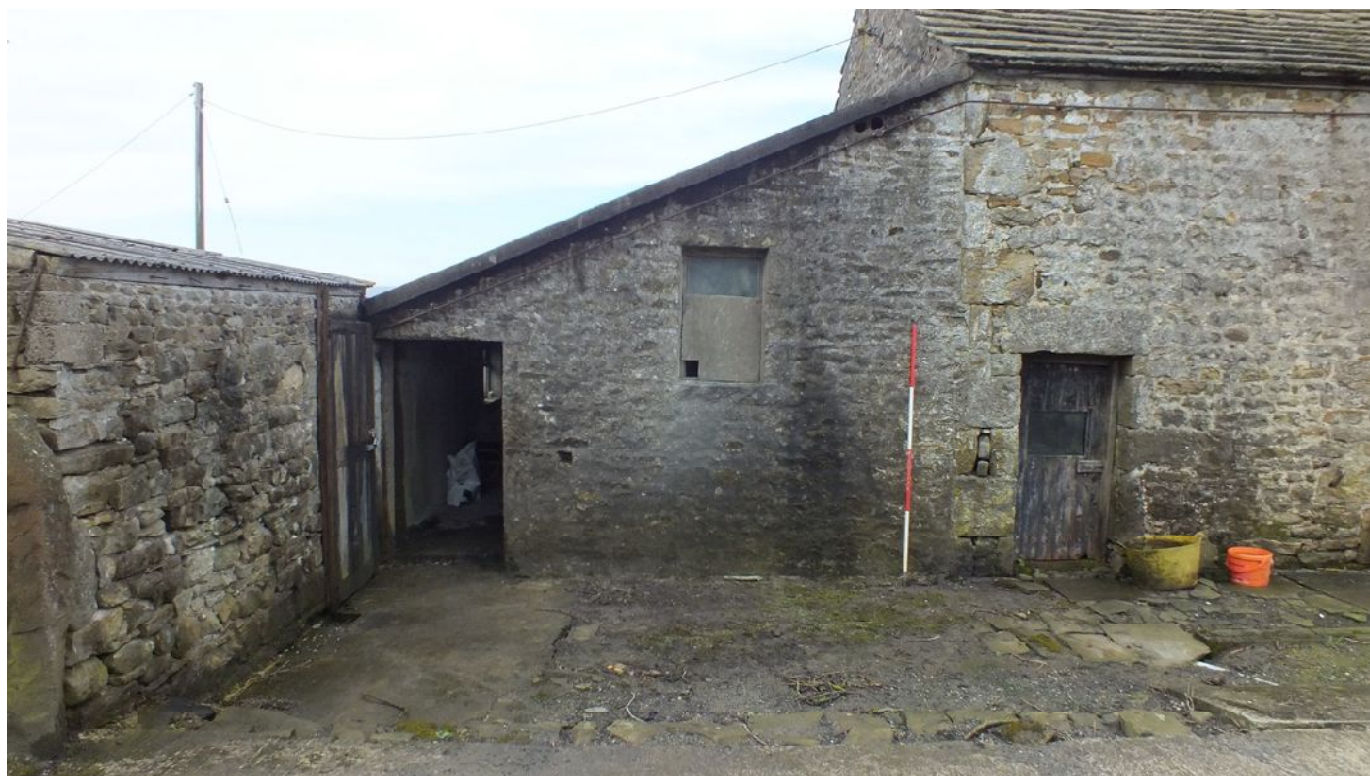
Plate 8: North-east external elevation (Barn 2)
