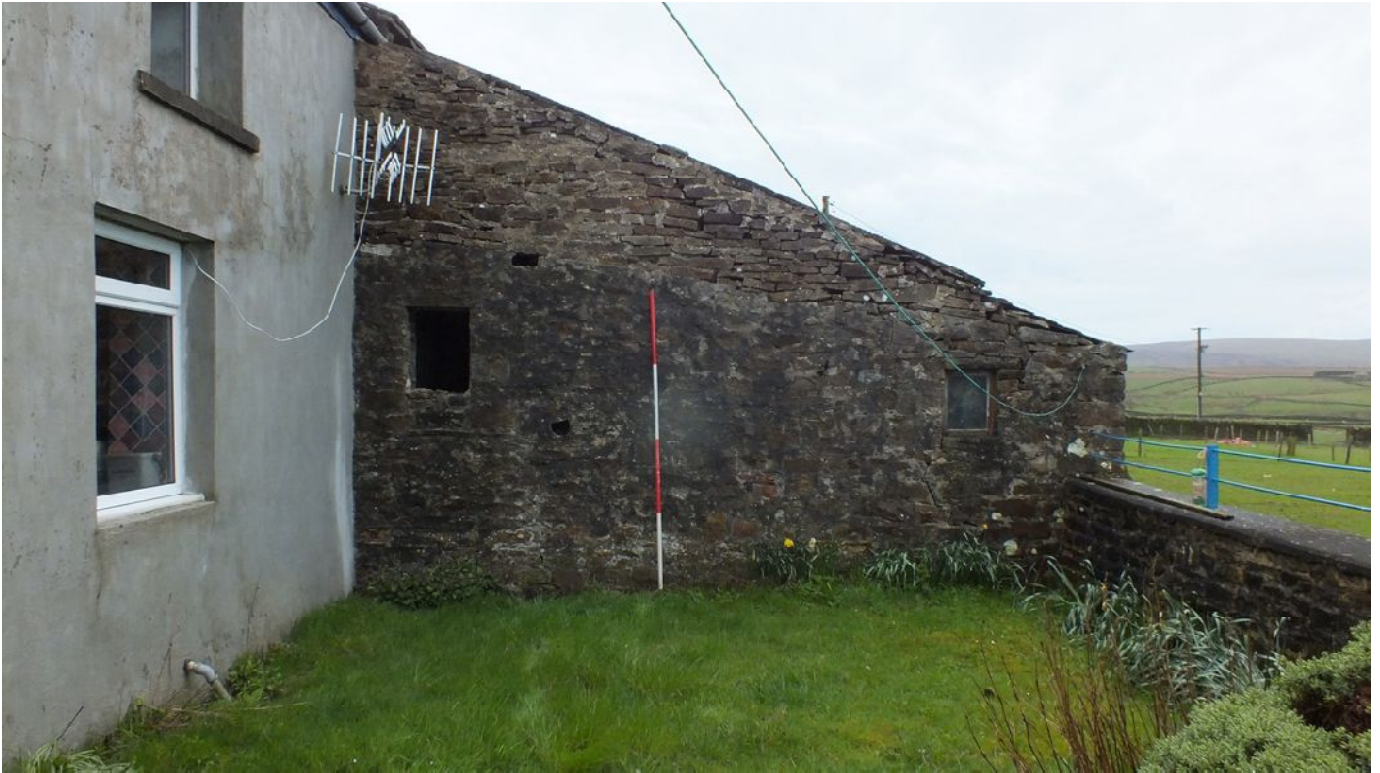
Plate 24: North-west external elevation of Barn 1
