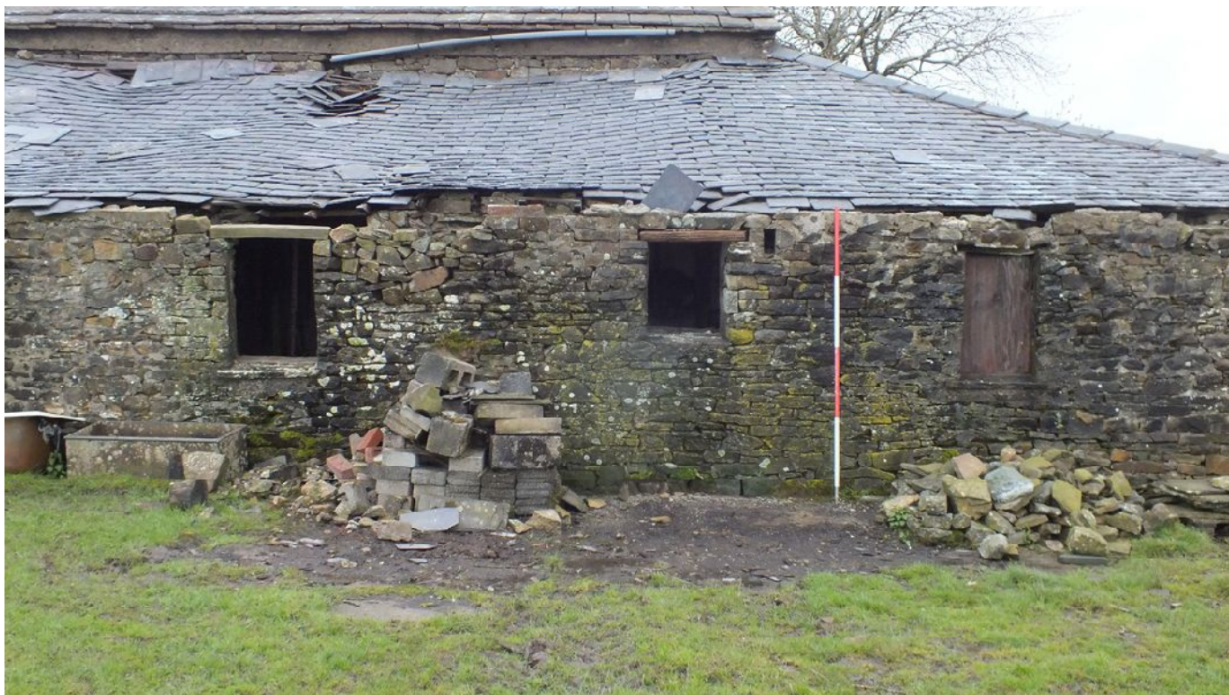
Plate 19: Centre of the south-west external elevation
