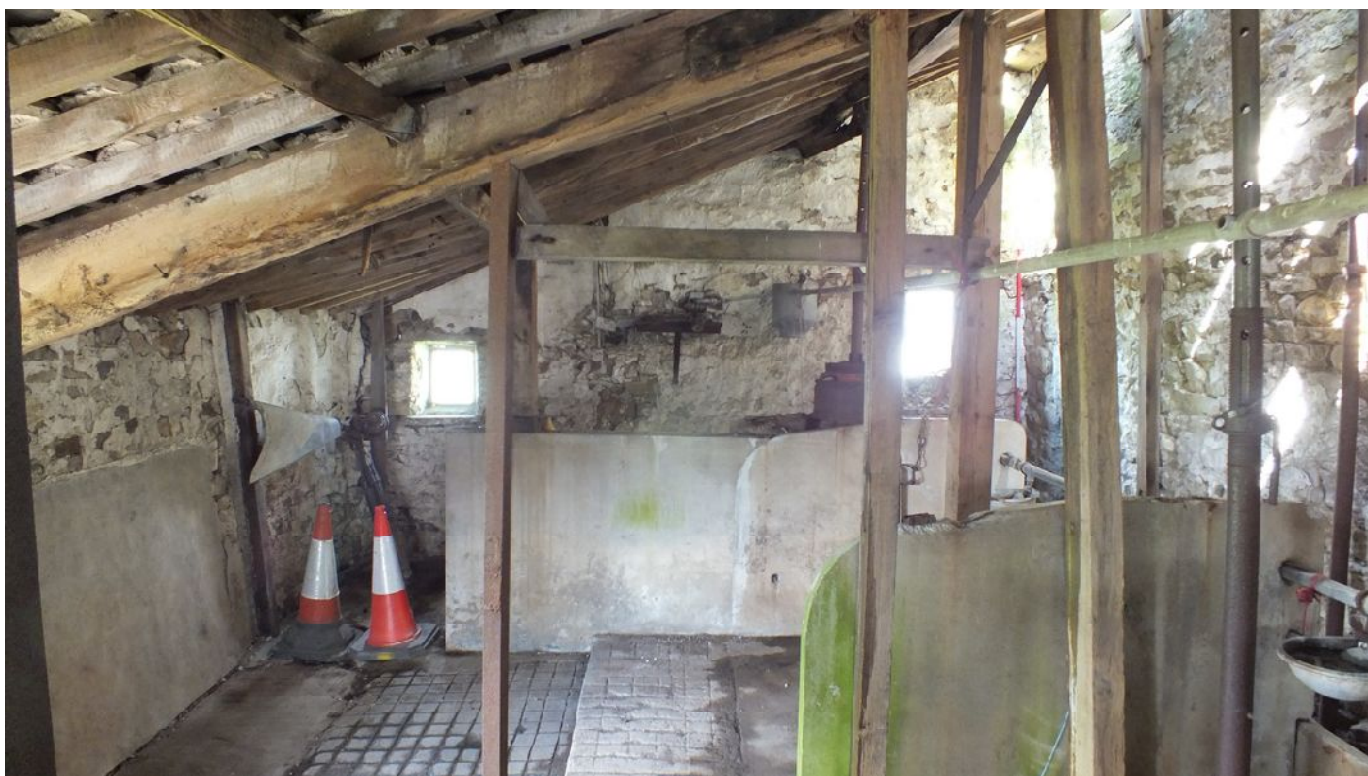
Plate 28: Low redbrick partition wall at the north-west end of Barn 1
