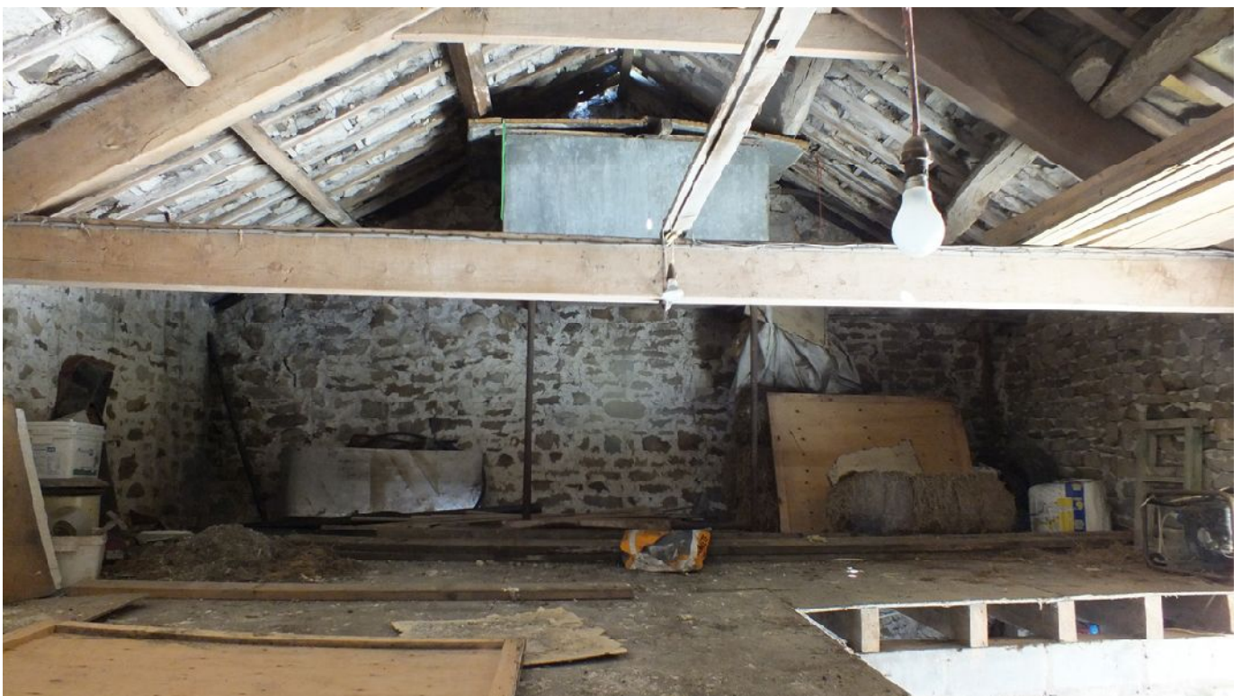
Plate 62: The north-west internal elevation of Barn 3 at the upper floor level
