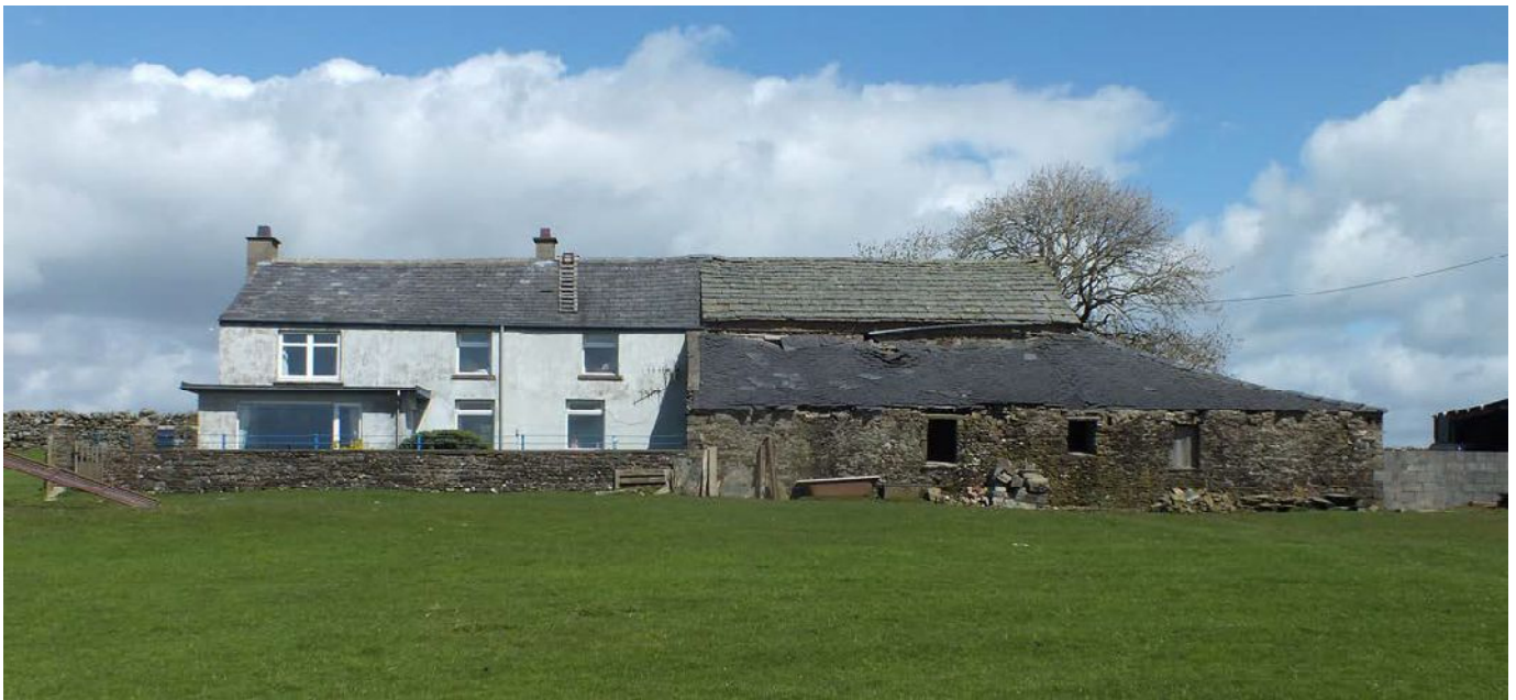
Plate 6: General view of the barns and house from the south-west
