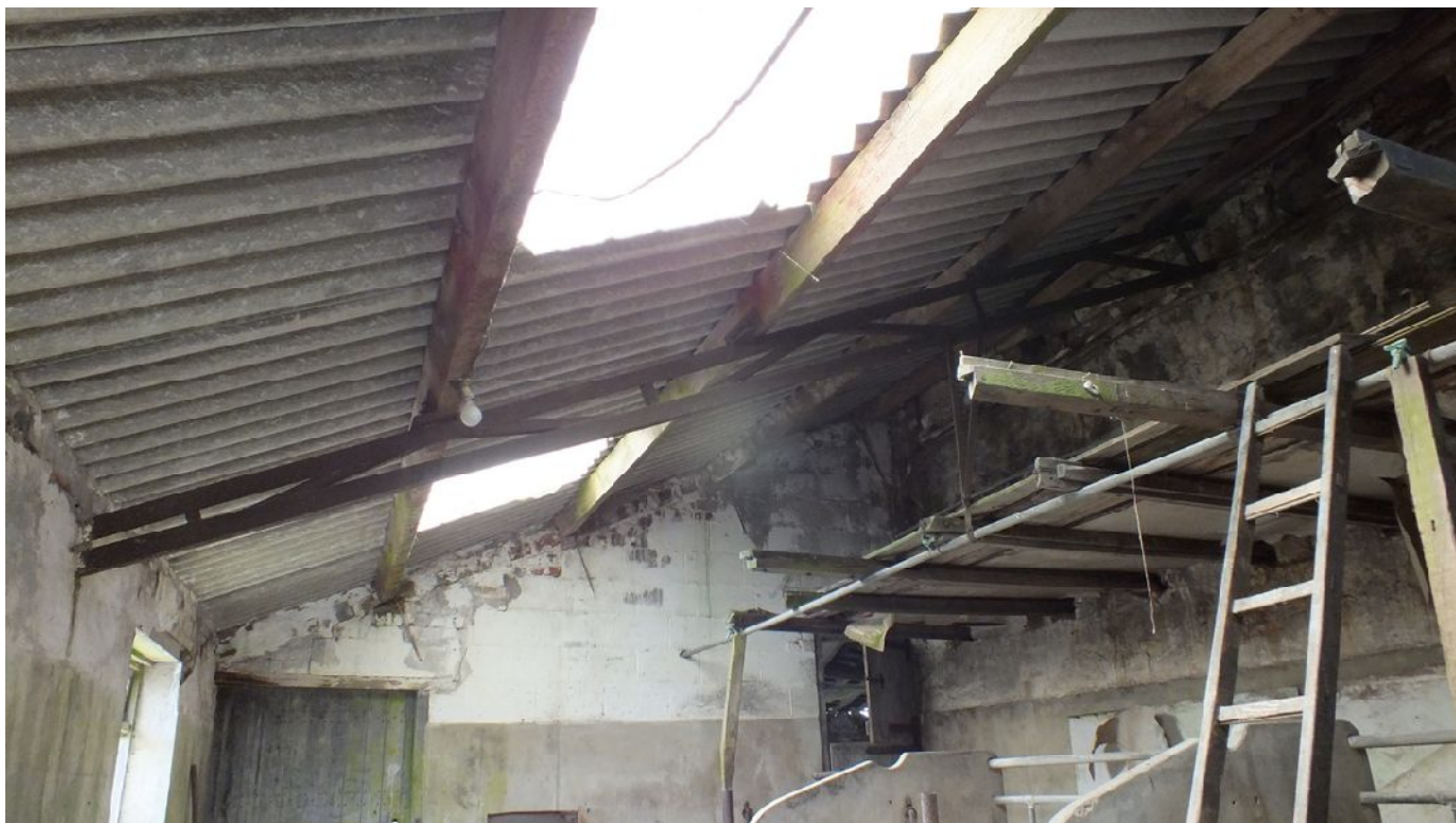
Plate 44: North-east side of the metal beam support in Barn 2
