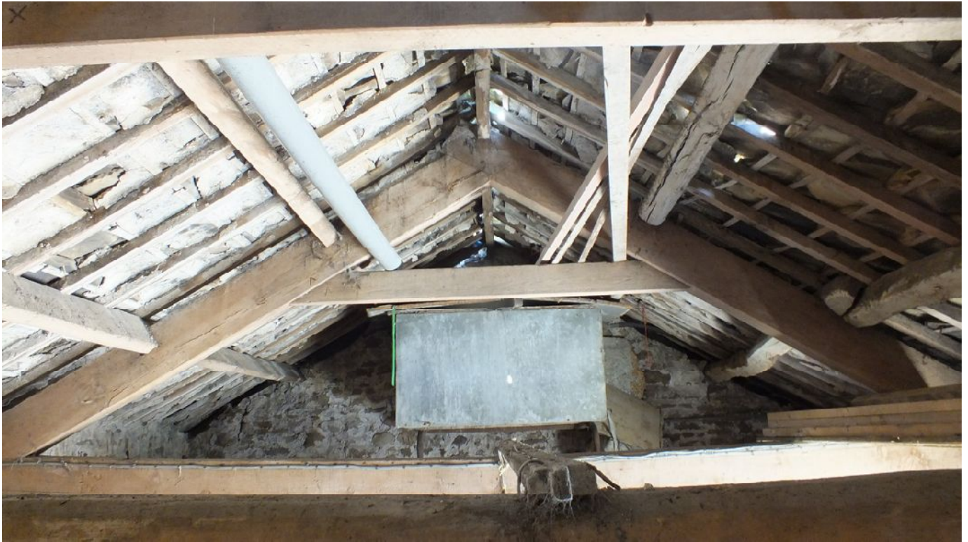
Plate 51: The north-west truss in Barn 3
