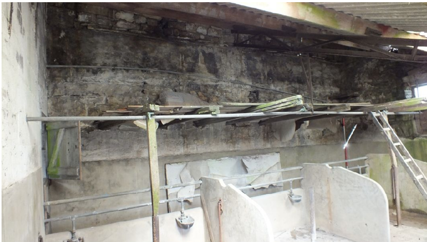
Plate 46: North-west internal elevation of Barn 2
