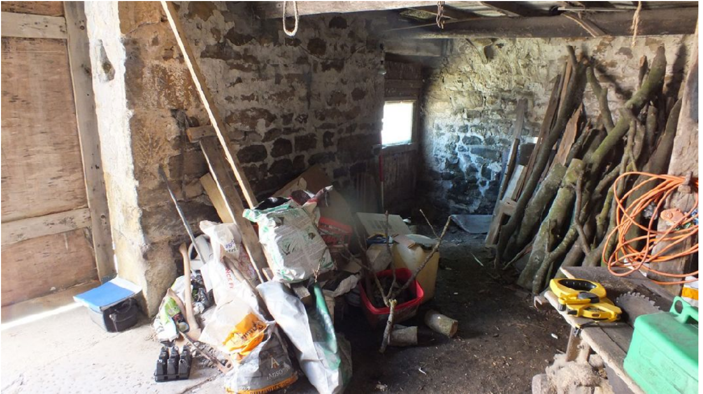
Plate 64: The south-east end of the north-east internal elevation of Barn 3 at ground floor level
