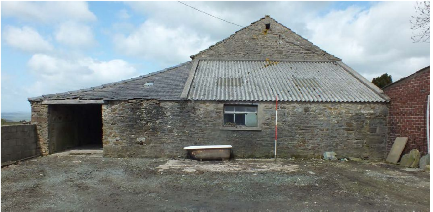
Plate 13: South-east external elevations of the barns
