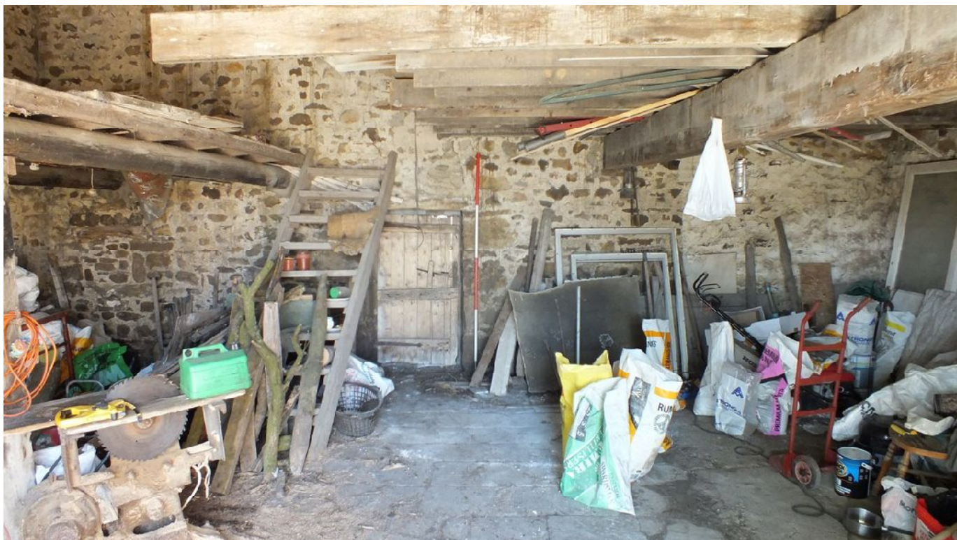
Plate 71: The south-west internal elevation of Barn 3 at ground floor level
