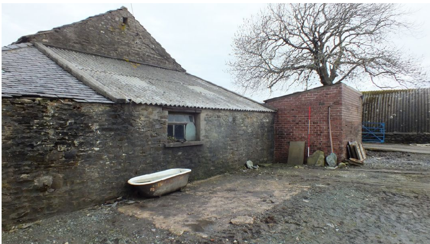
Plate 16: Outshut against the south-east external elevation of Barn 2
