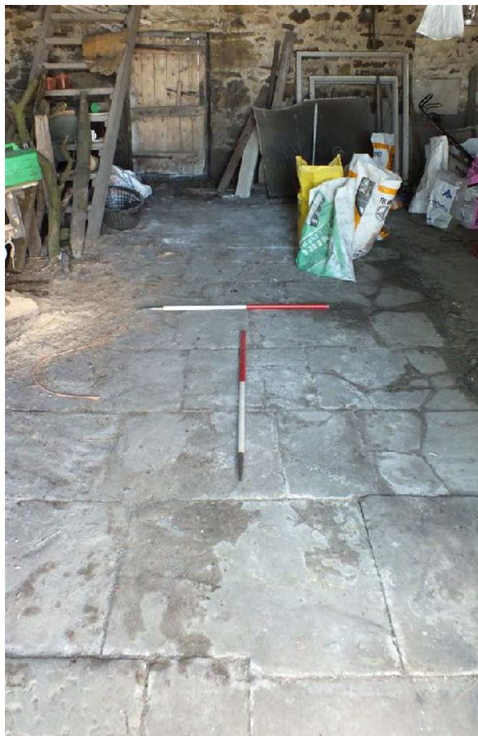
Plate 58: Stone threshing floor in Barn 3
