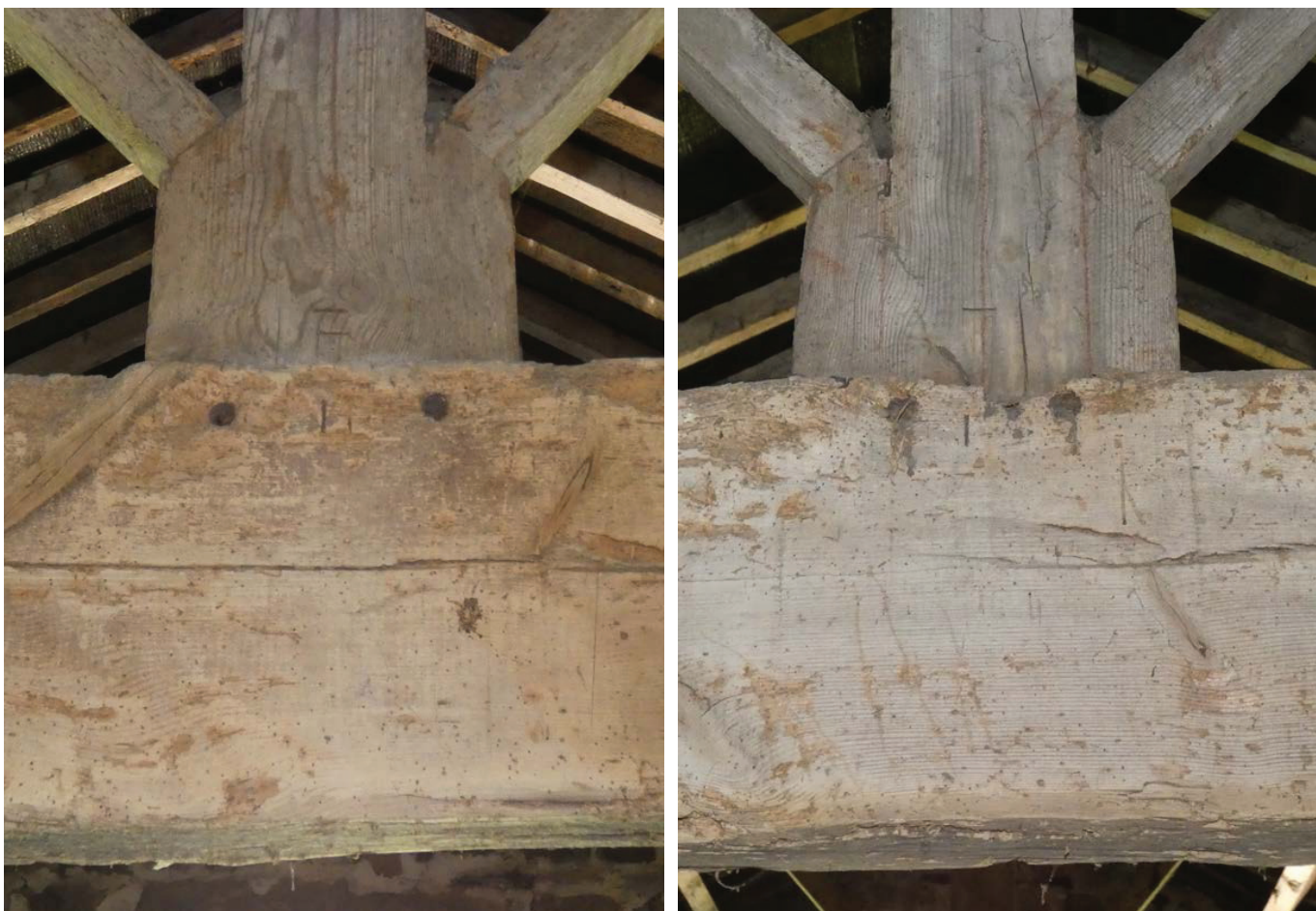
Plate 54 (left): 'll' marked on the south-west face of the north-east truss in F1
