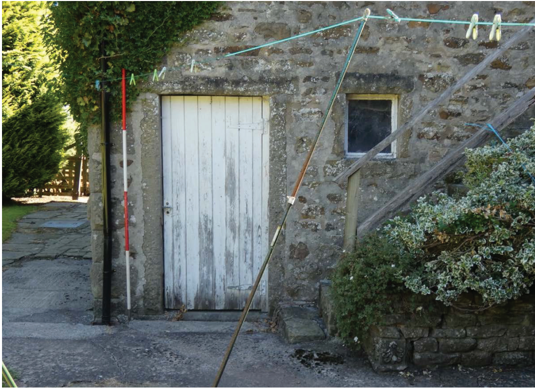
Plate 19: North-west end of the south-west external elevation at ground floor level
