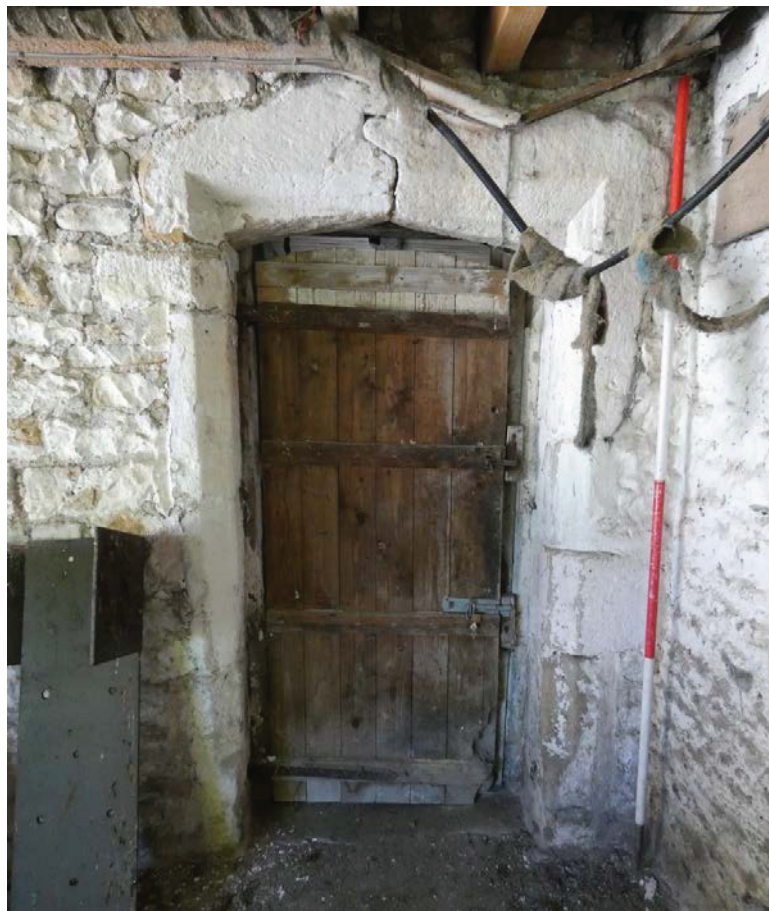
Plate 38: Detail of the early door surround in G3
