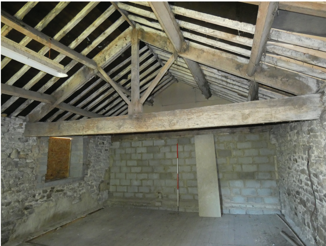
Plate 50: North-east face of the south-west truss in F1
