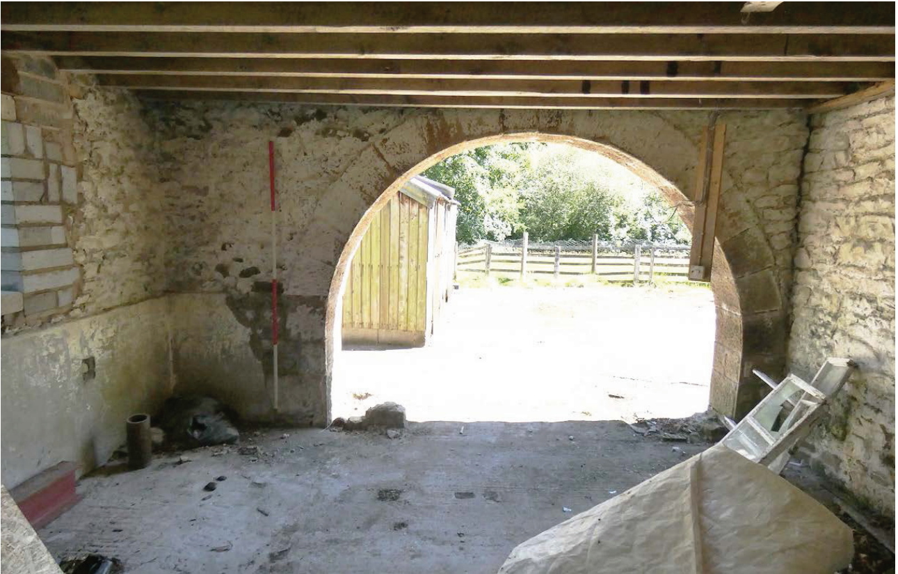
Plate 35: North-east elevation of G3
