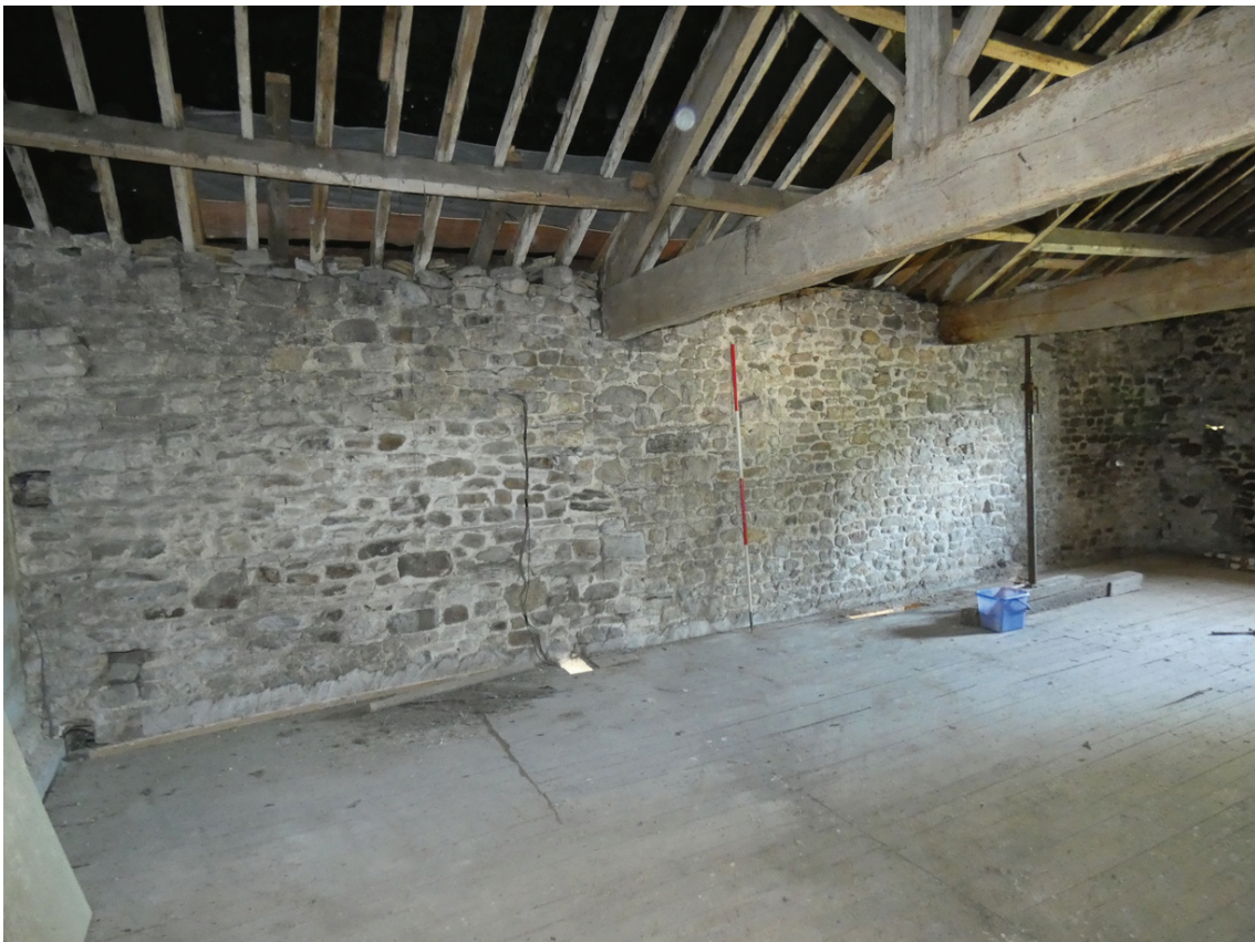
Plate 60: North-west elevation of F1
