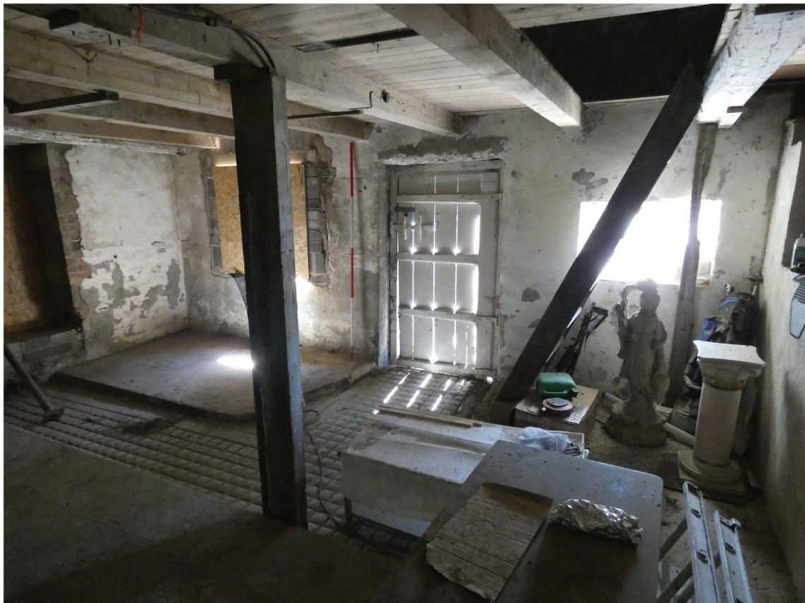
Plate 33: South-east elevation of G2
