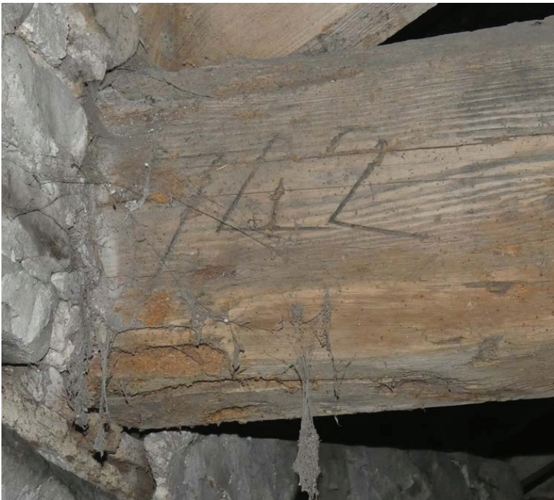
Plate 52 (left): '742' marked on the north-east face of the north-east truss in F1
