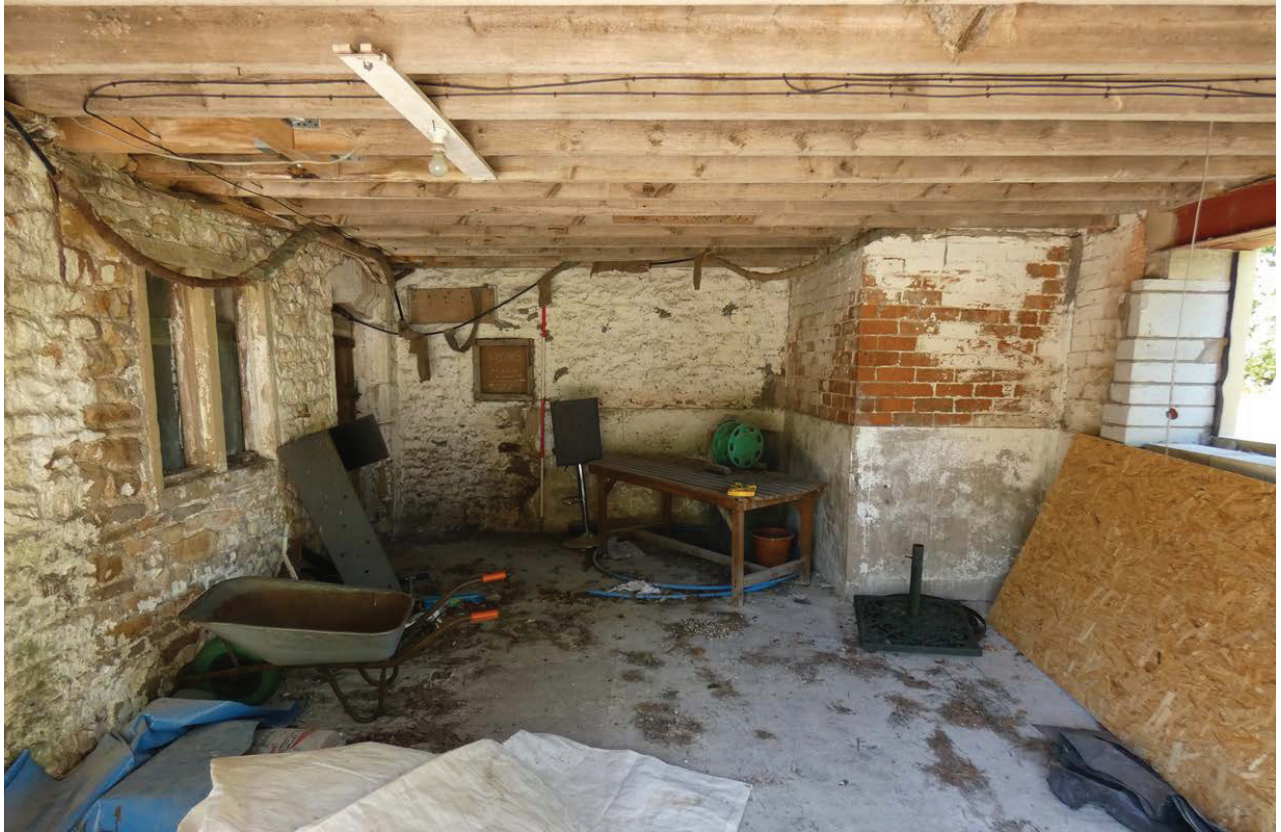
Plate 39: General view of the south-west end of G3
