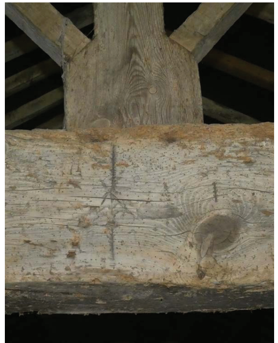
Plate 52 (left): '742' marked on the north-east face of the north-east truss in F1
