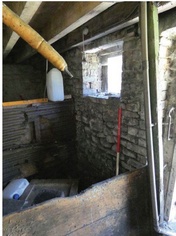
Plate 49: Window in the south-west elevation of G4
