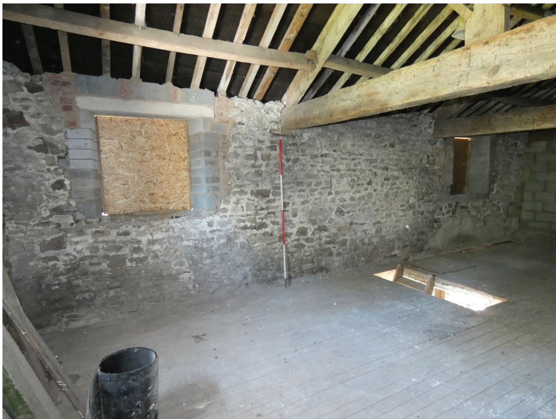
Plate 57: North-east end of the south-east elevation of F1
