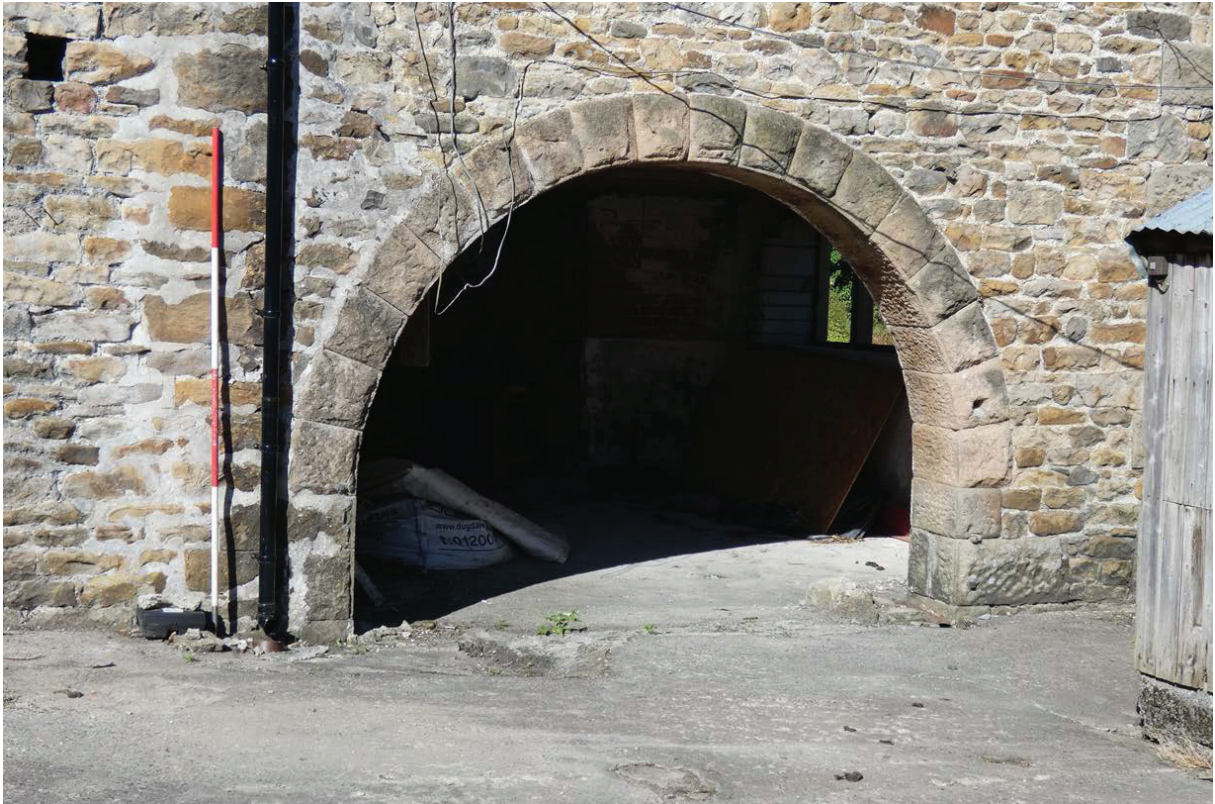
Plate 12: Archway at the north-west end of the north-east external elevation
