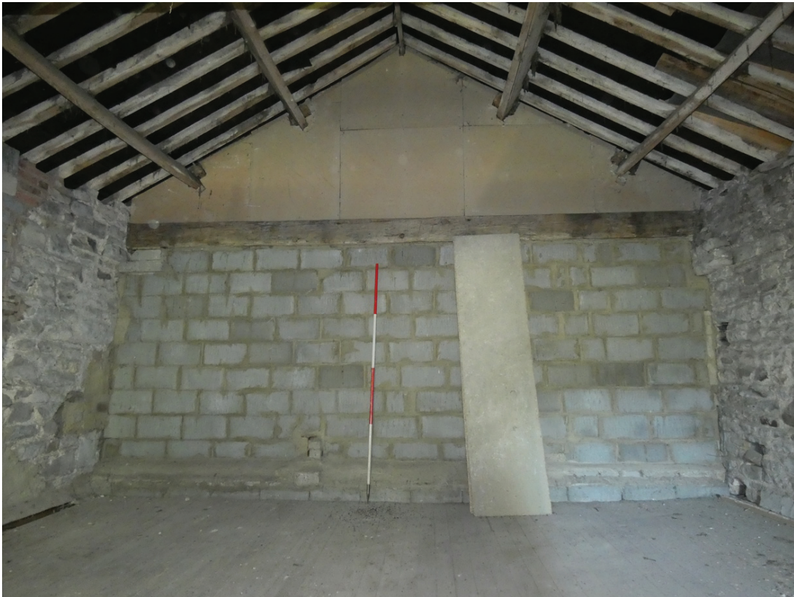
Plate 59: South-west elevation of F1
