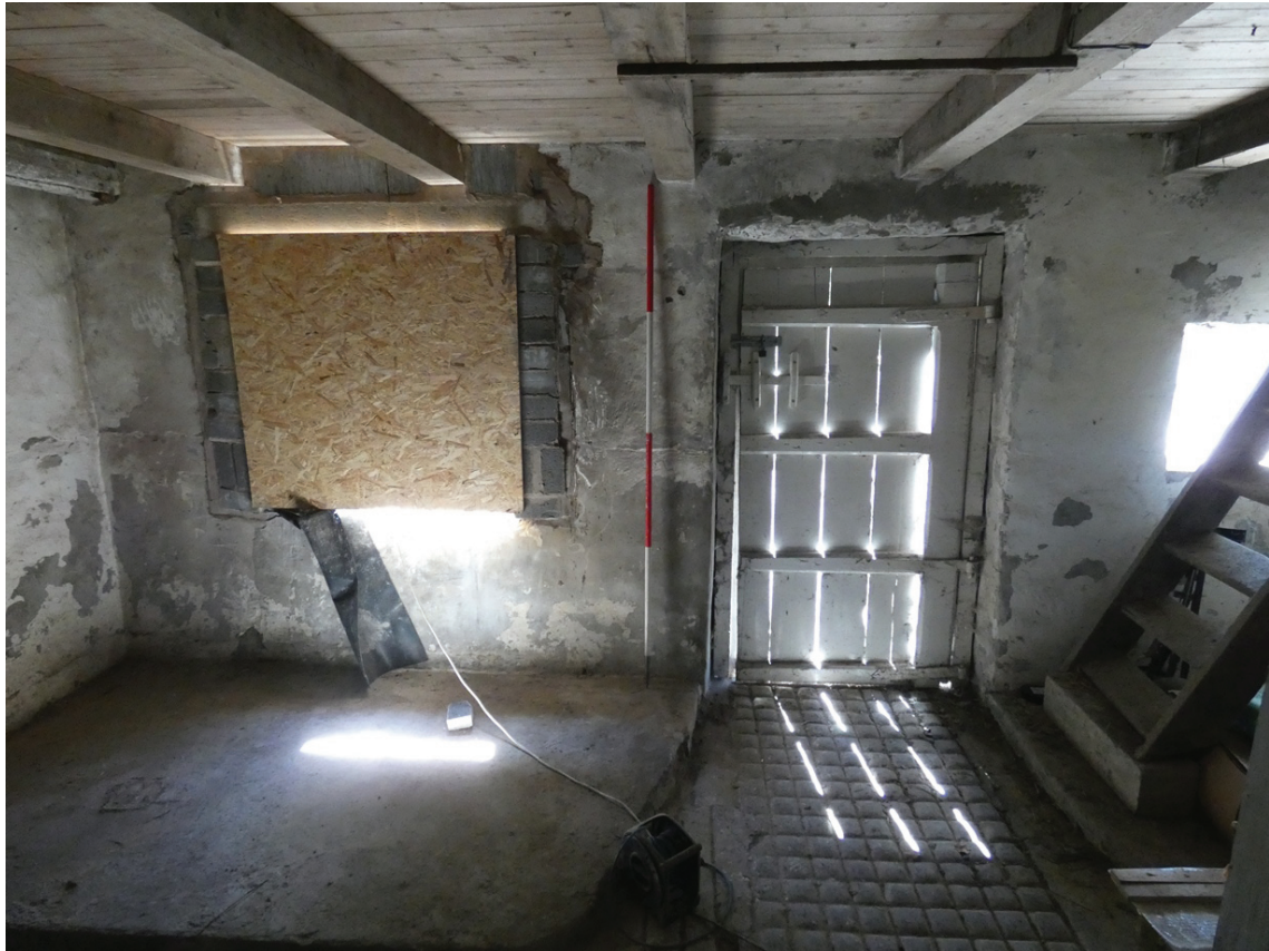
Plate 32: North-east end of the south-east elevation of G2
