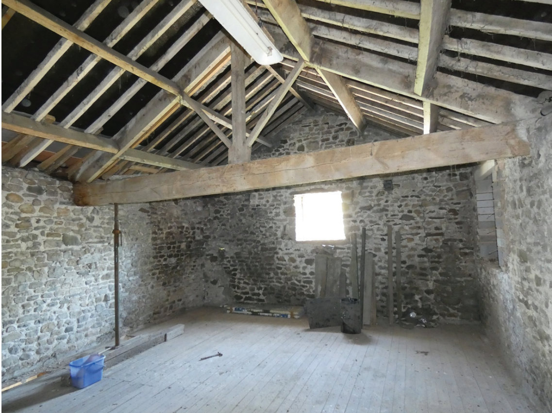
Plate 51: South-west face of the north-east truss in F1
