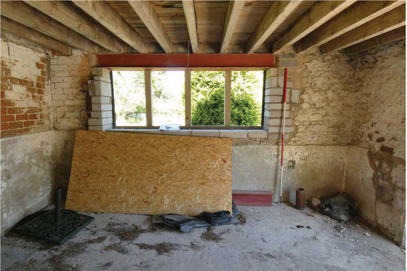
Plate 41: Window inserted in the north-east end of the north-west elevation of G3
