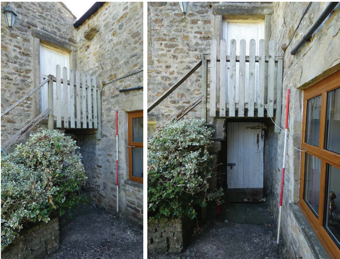
Plate 20 (left): Steps to the first floor at
