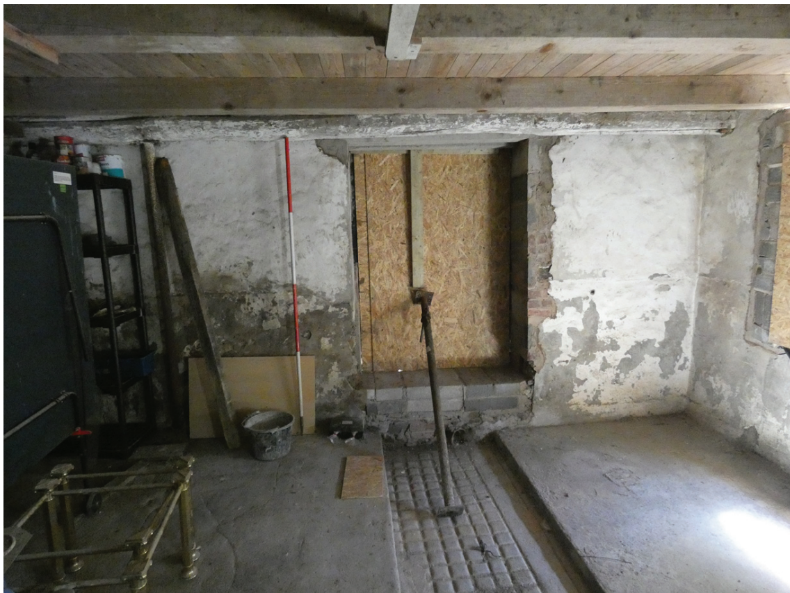
Plate 31: Recently inserted doorway in the north-east elevation of G2
