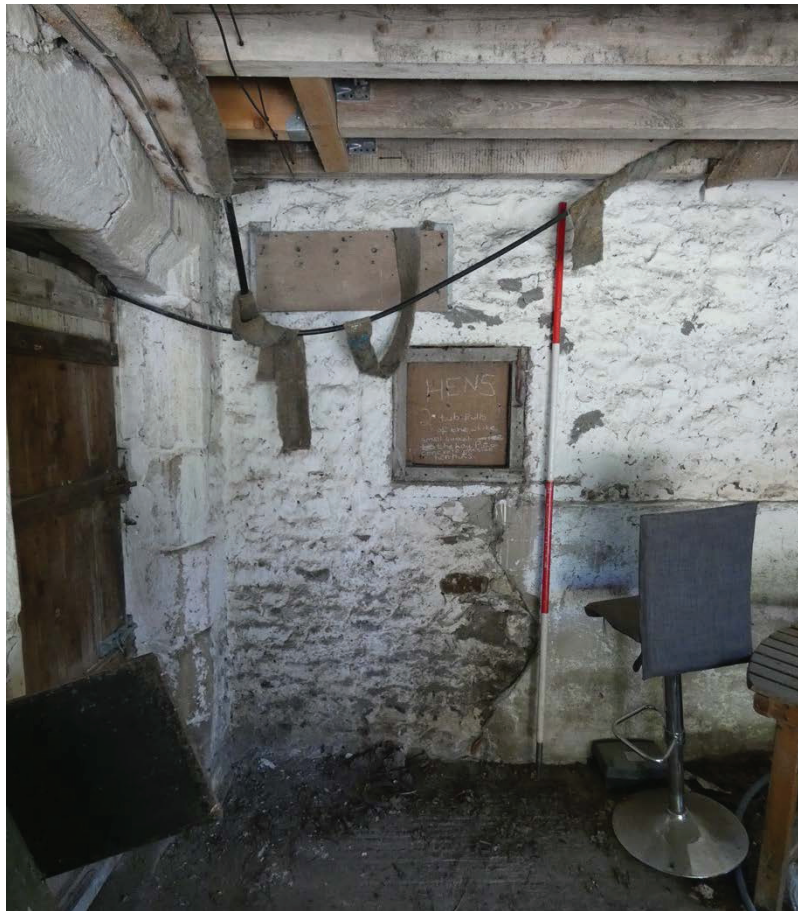
Plate 40: Window in the south-west elevation of G3
