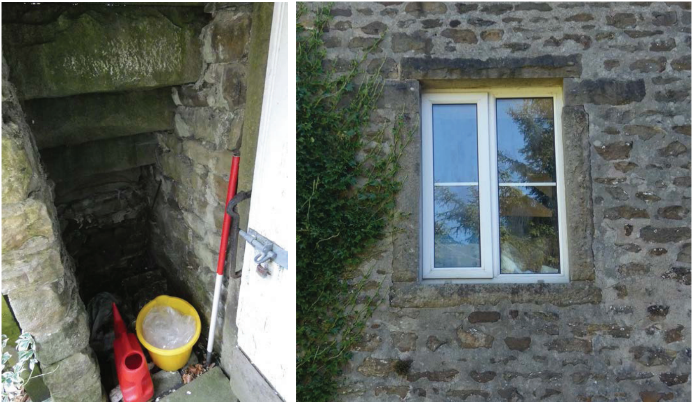
Plate 22: Area below the stairs on the south-west elevation
