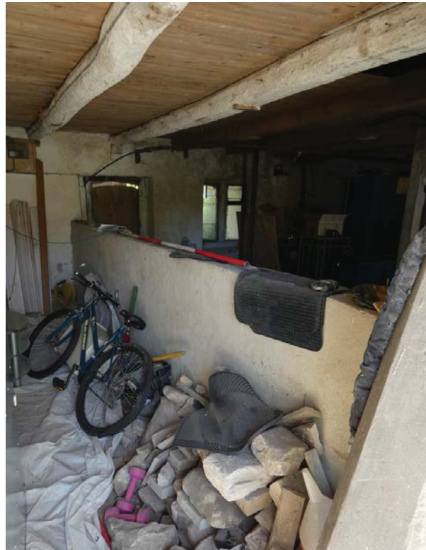
Plate 27: Low partition wall between G1 and G2
