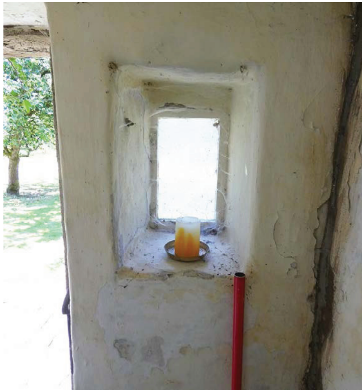
Plate 44: Window in the north-west elevation of G3a
