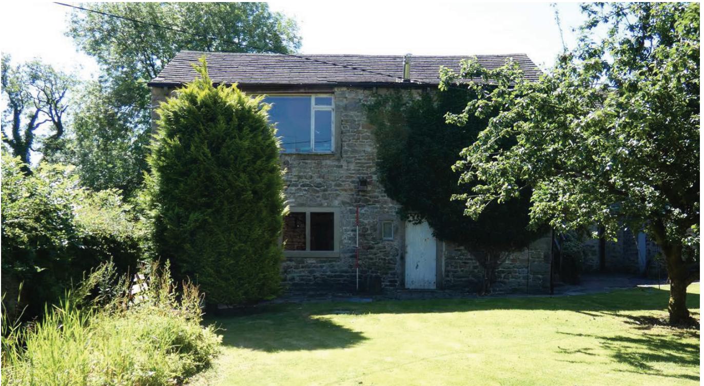
Plate 15: North-west external elevation
