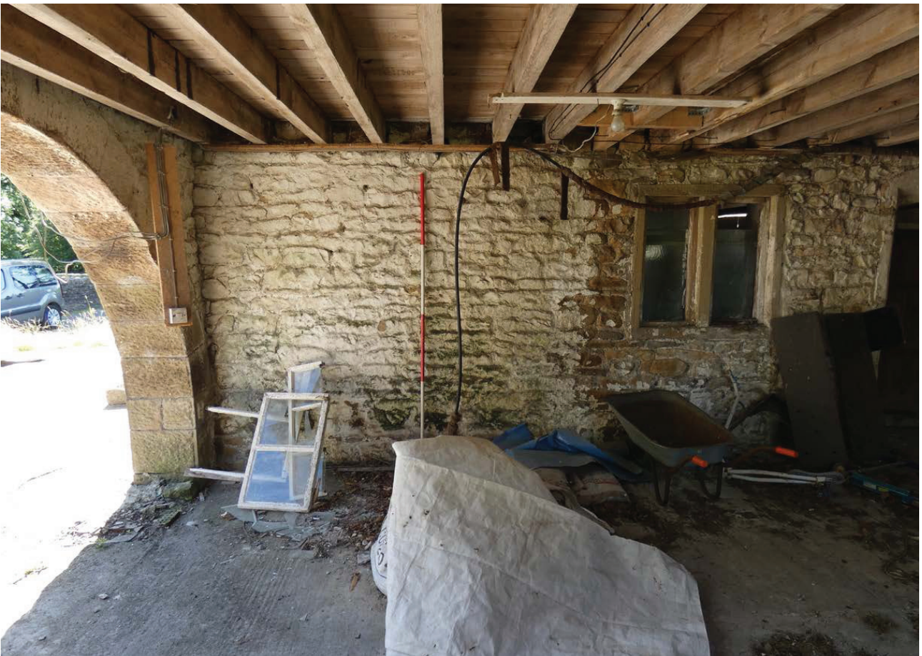
Plate 36: North-east end of the south-east elevation of G3
