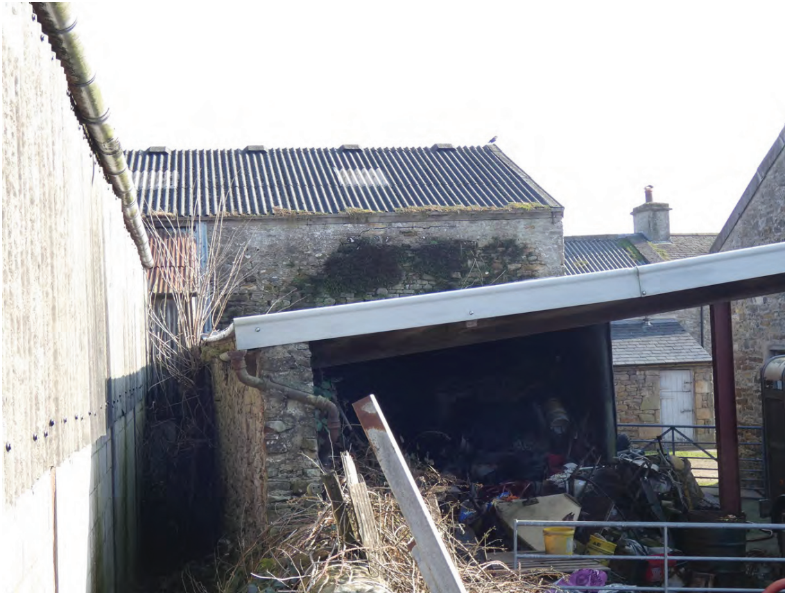
Plate 17: The north-east end of the north-west external elevation
