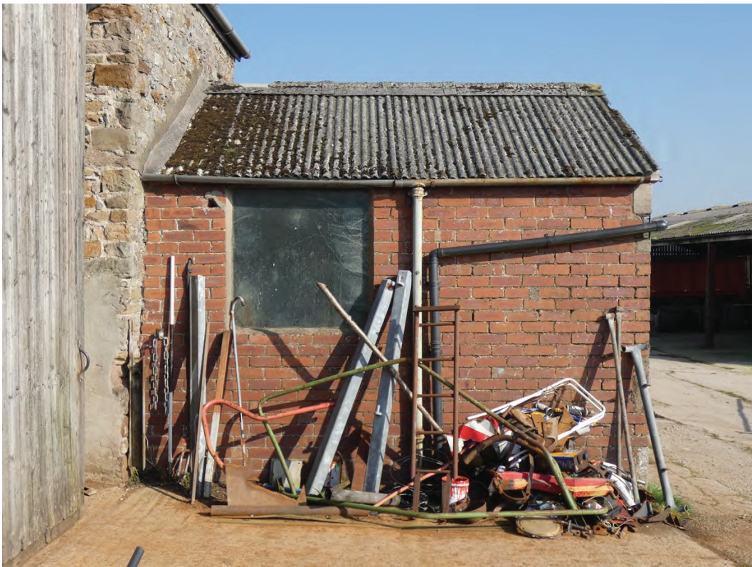
Plate 14 (right): The return to the south-east of the south-east external elevation, viewed from the south-west
