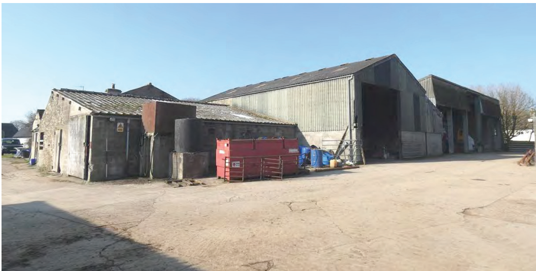
Plate 12: The north-east external elevation viewed from the east showing the modern extension to the north-west
