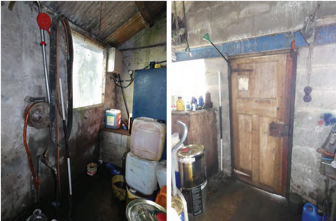
Plate 24 (right): Window in the south-west elevation of Room G3, viewed from the east
