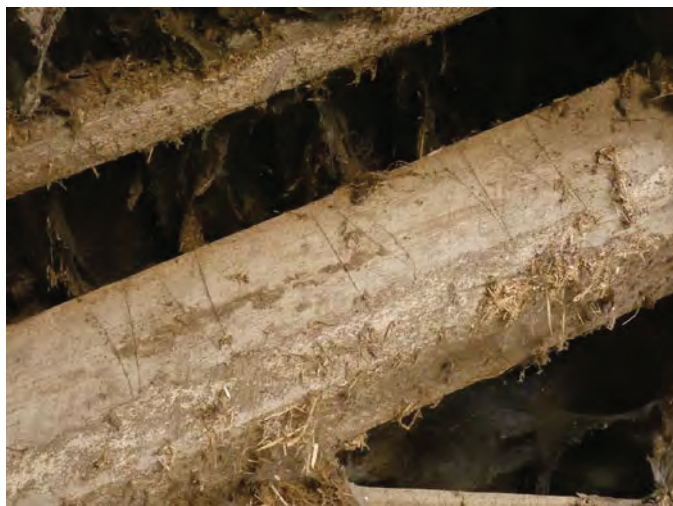
Plate 31 (left): Carpenter's mark 'III' on south-east truss in Room G4, viewed from the south-east
