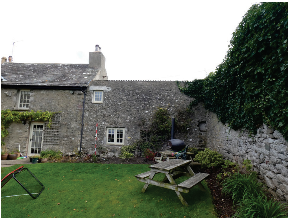
Plate 18: General view of the south-west external elevation, viewed from the south-west
