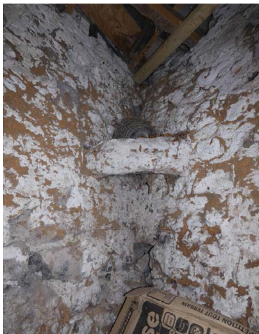
Plate 27: Stone 'lintel' across the south corner of Room 1, viewed from the north
