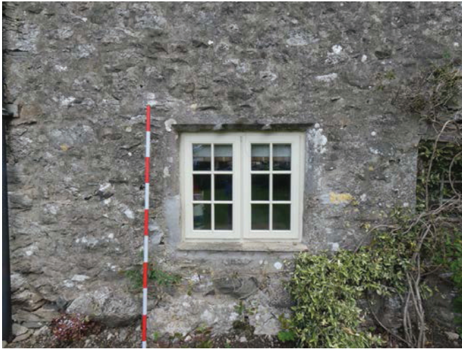
Plate 22 (left): North-west window retaining elements of a stone mullion in the south-west external elevation, viewed from the south-west
