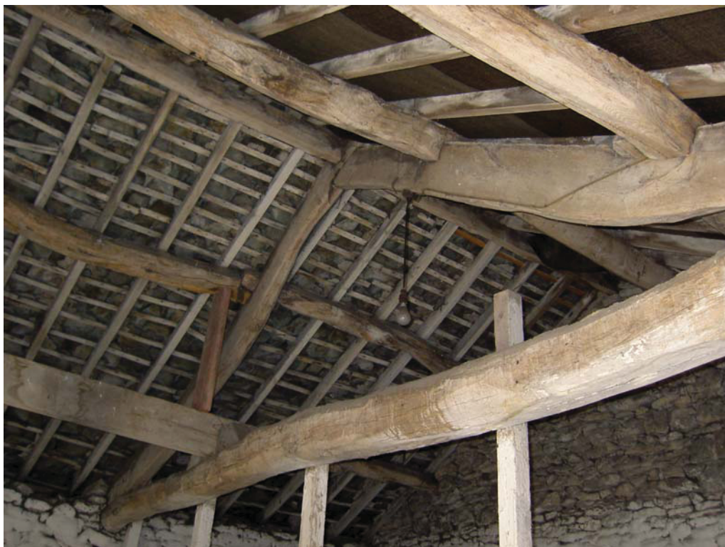
Plate 16: Truss and inserted beam with supports in stable
