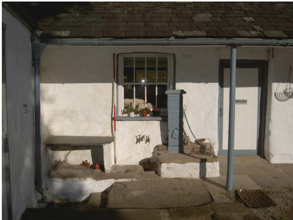
Plate 6: Detail of the pump and associated trough
