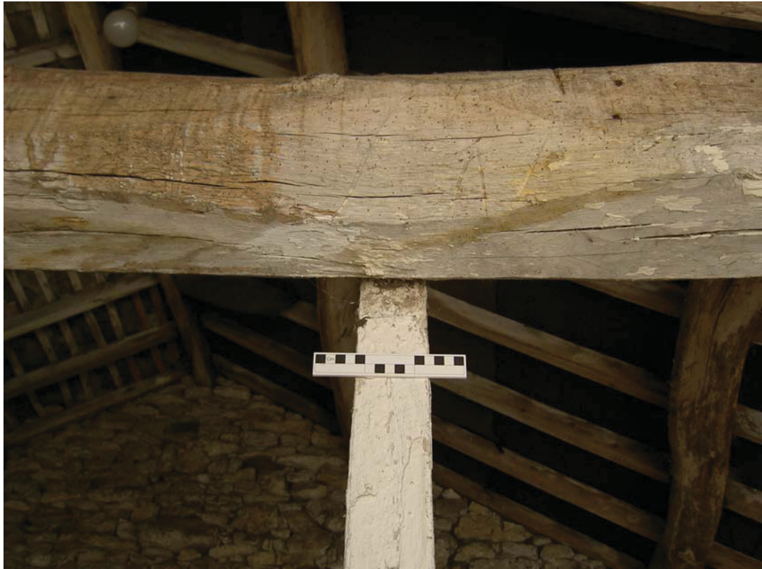
Plate 17: Baltic timber marks in west face of tie beam in stable
