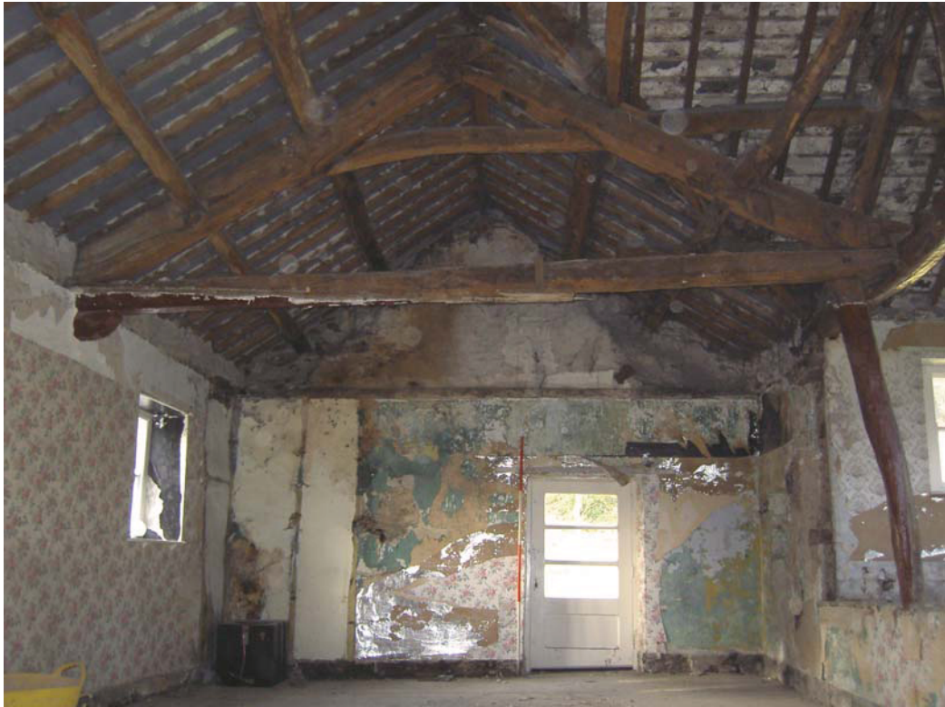
Plate 37: The western truss and west elevation in F1 showing the raised gable and the post supporting the north end of the truss
