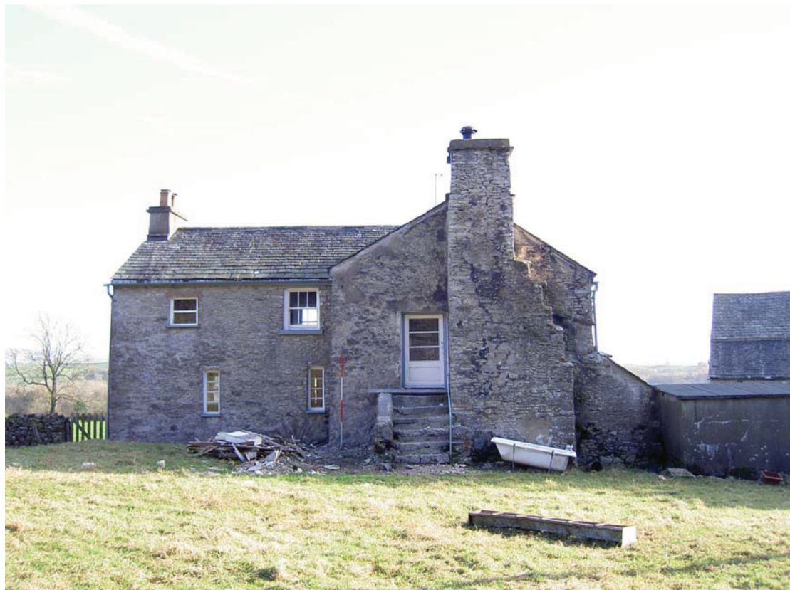
Plate 14: West external elevations of the farmhouse and northern extension
