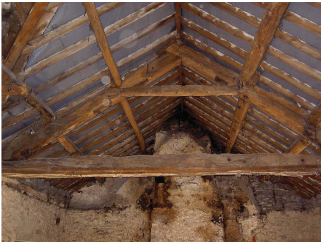
Plate 34: West face of eastern truss, F1
