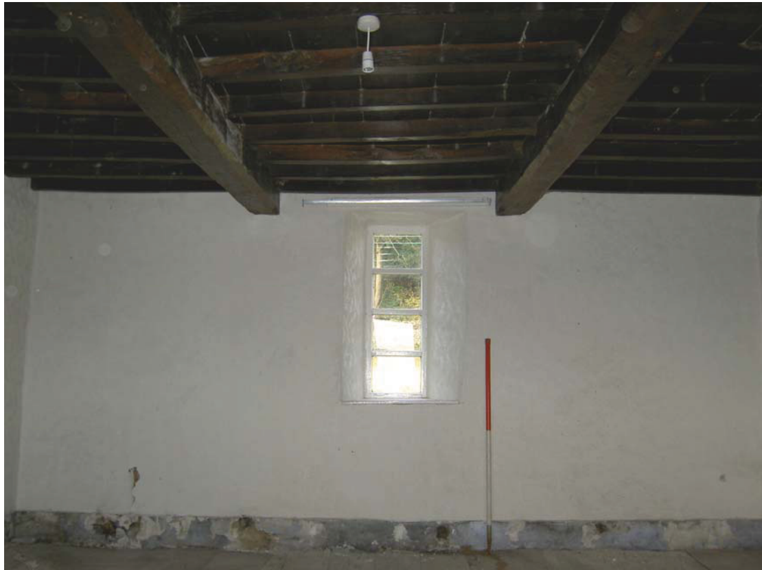
Plate 31: Ceiling and west elevation, G3
