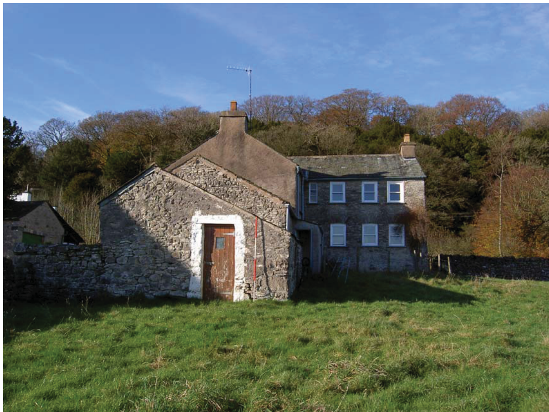
Plate 10: East external elevations of the outbuildings
