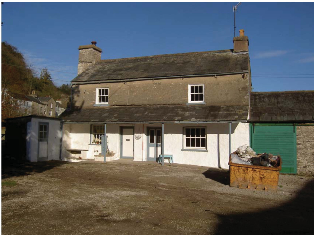
Plate 4: Front (south) external elevation of the farmhouse
