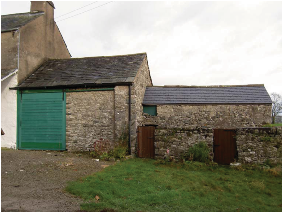
Plate 7: South (front) external elevation of the stable and pig sties
