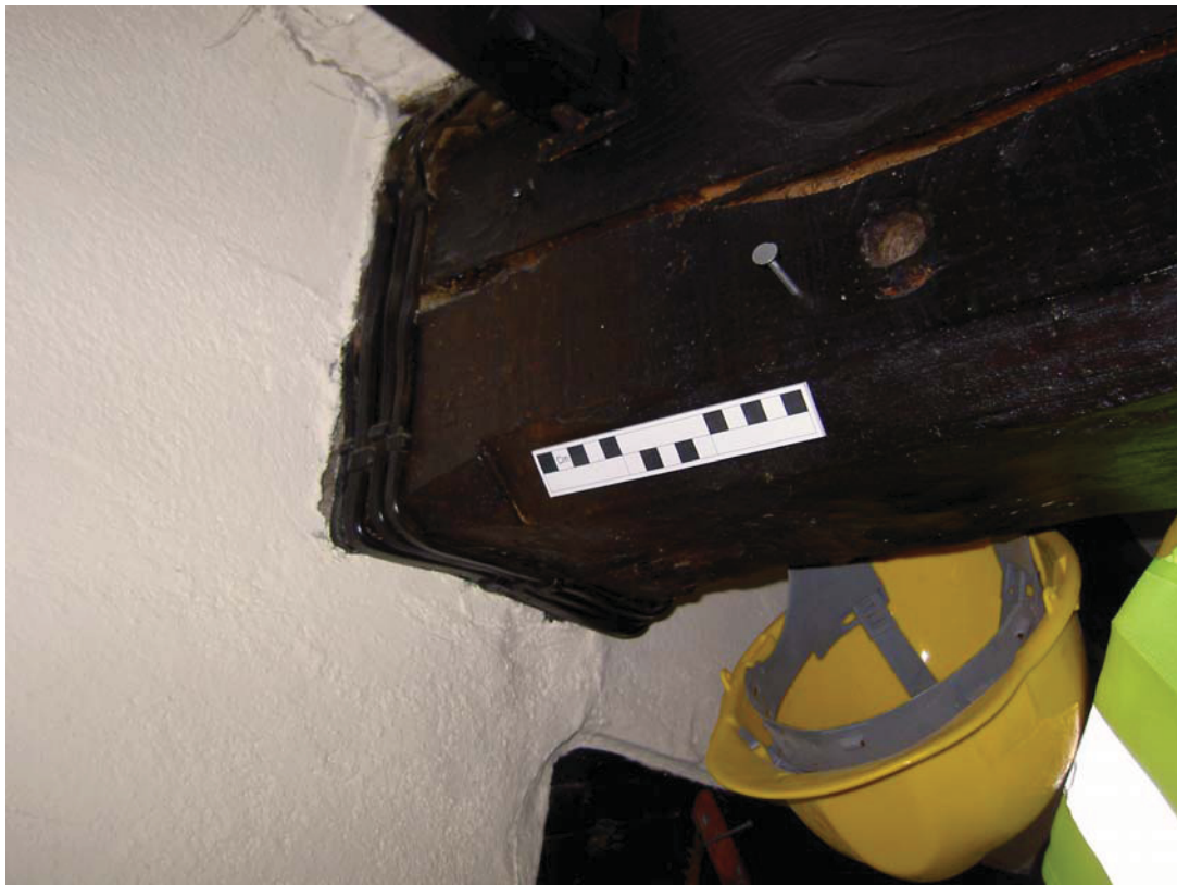
Plate 22: Detail of stop chamfer, north end of westernmost beam, G1
