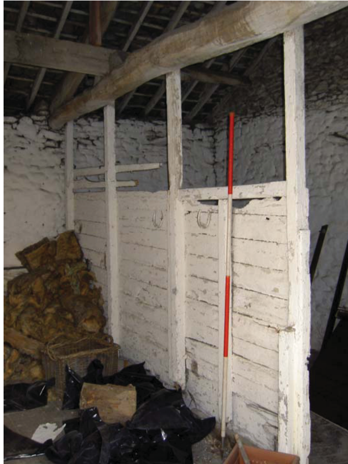
Plate 15: Timber partition wall in the stable
