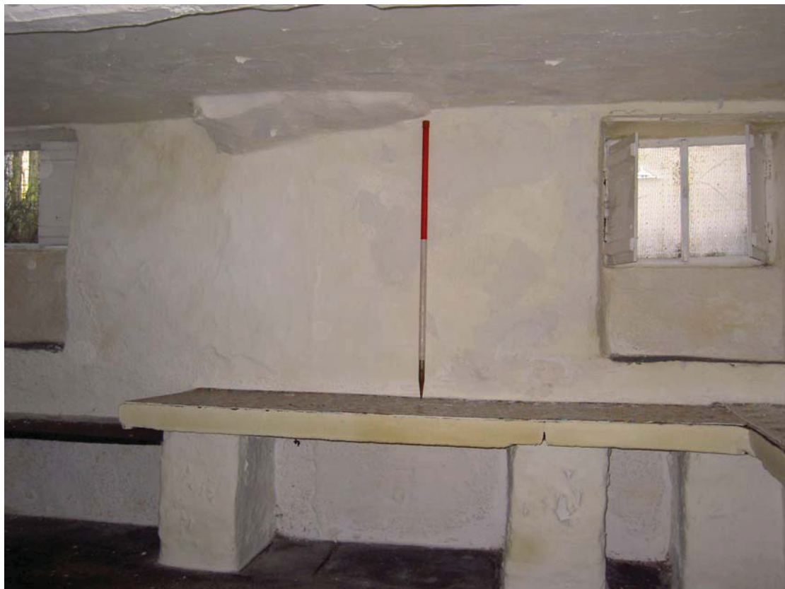
Plate 18: North side of C1 showing slate bench and shuttered window
