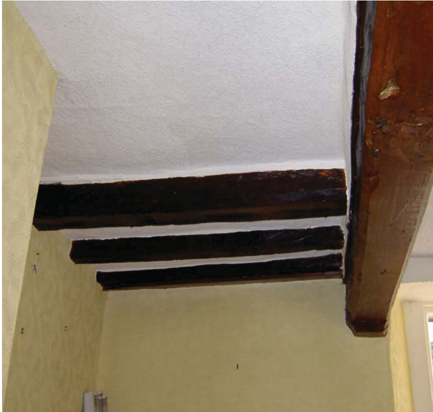
Plate 29: Beams in south-east corner of G2 indicating position of smoke hood
