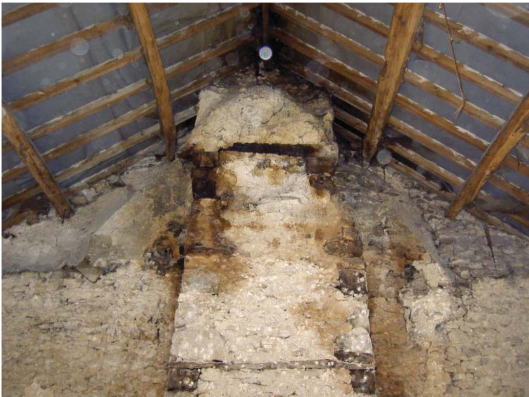
Plate 36: The east elevation in F1 showing the original corbelled chimney, inserted chimney breast, and raised roof line
