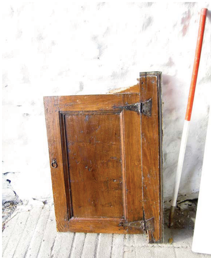
Plate 40: Loose door with early strap hinges in the stable
