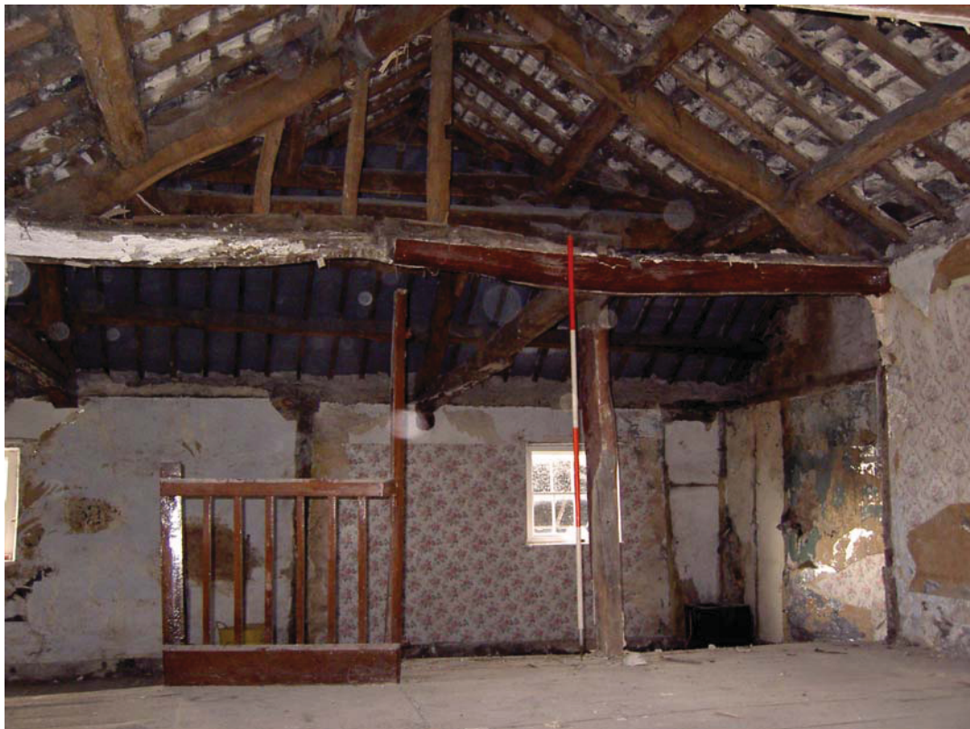
Plate 38: The southern truss in F2 showing the post supporting the western truss in F1, the banister, and the posts forming stud partition walling between the tie beam and principal rafters
