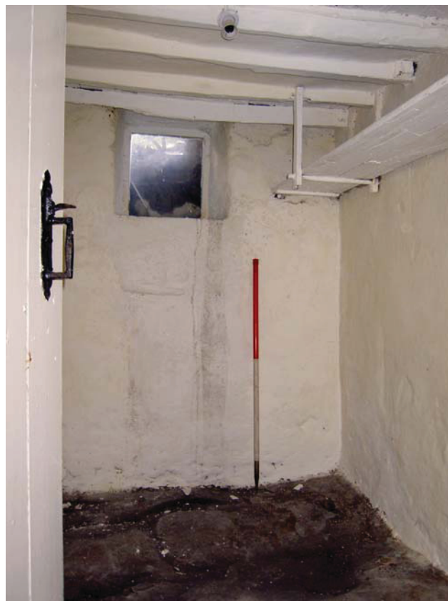
Plate 20: West side of C2 showing bedrock floor and shelf along north wall
