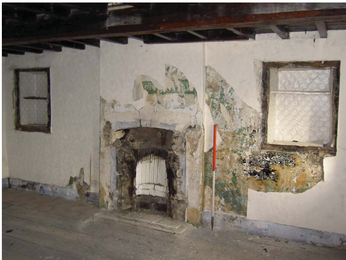
Plate 32: Fireplace and flanking cupboards, north end of G3
