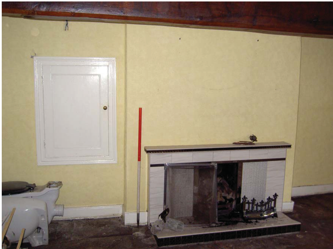
Plate 30: Modern fireplace and spice cupboard, east side of G2
