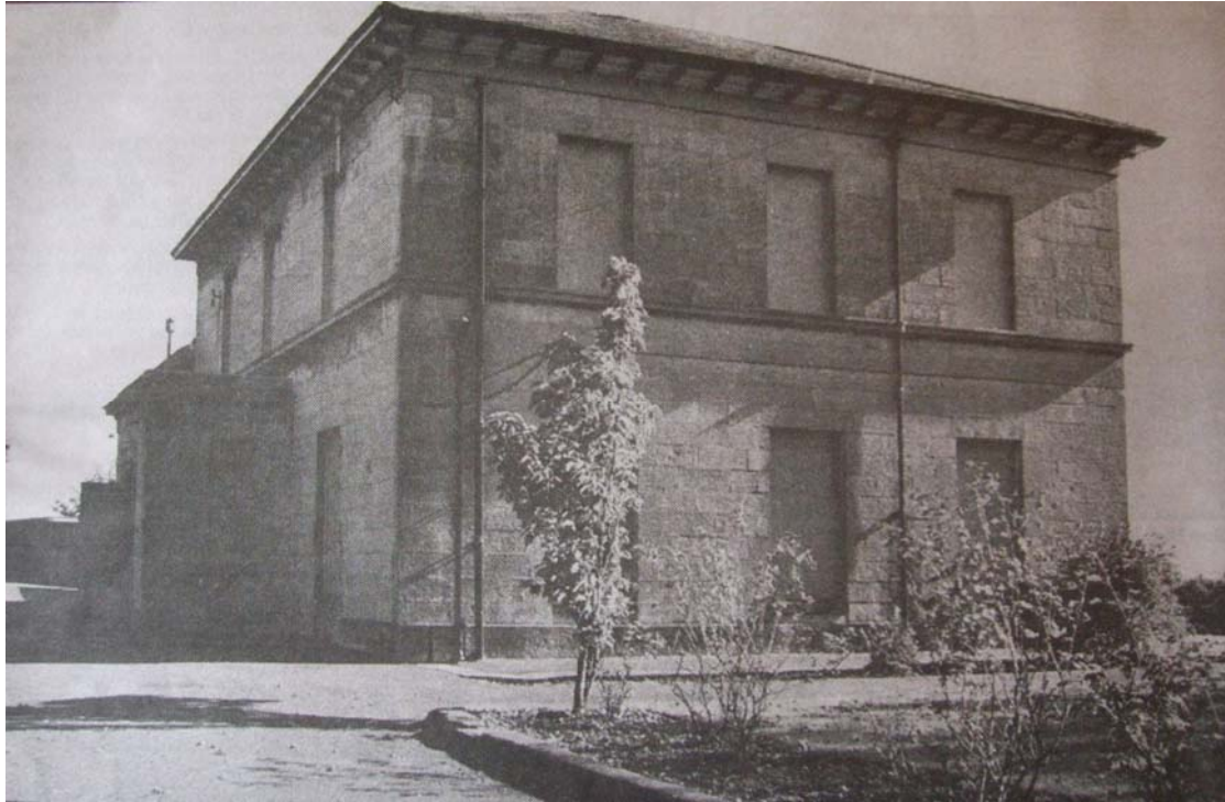
Plate 39: View of Ford House boarded up in 1998 to prevent vandalism (from Horne 1998a)
