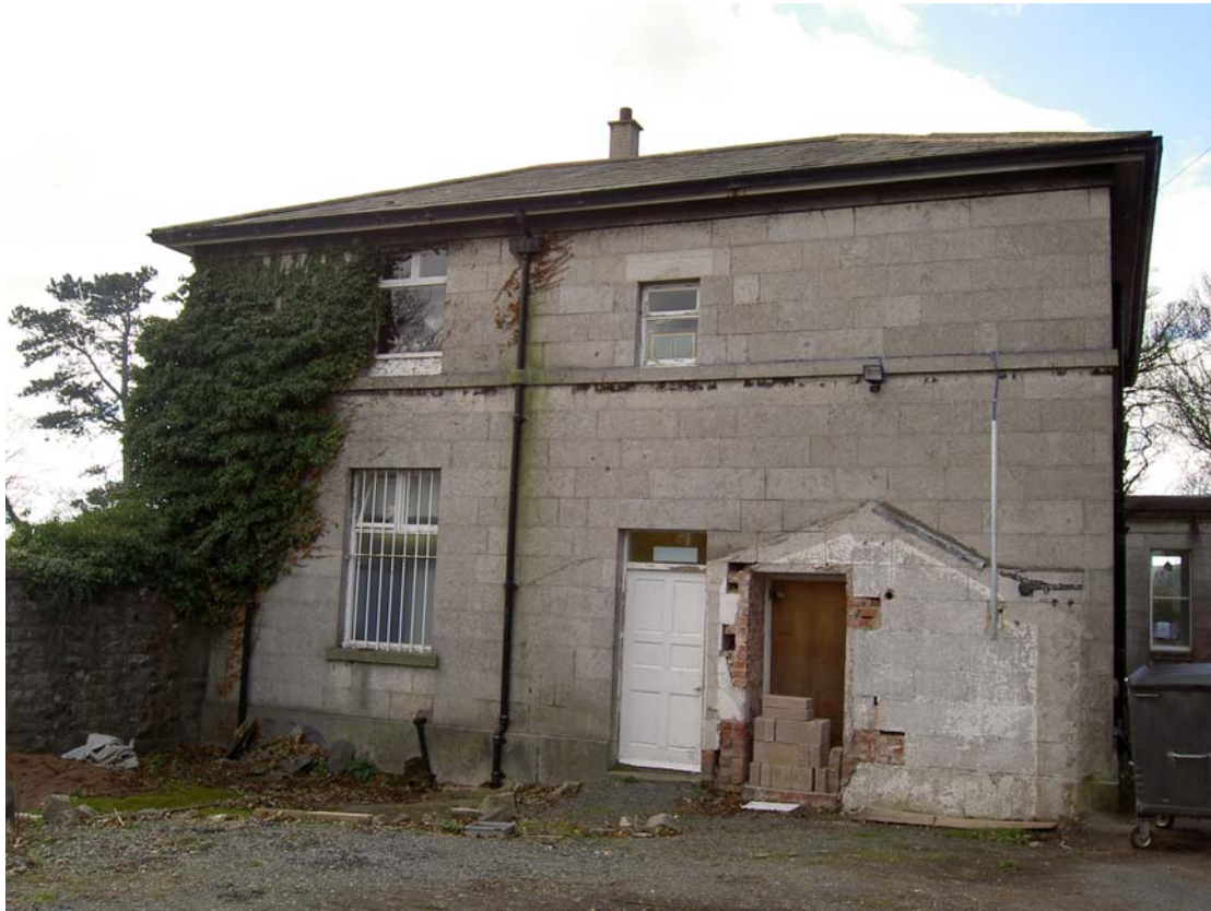
Plate 52: Scar of outshut on north-east side of house
