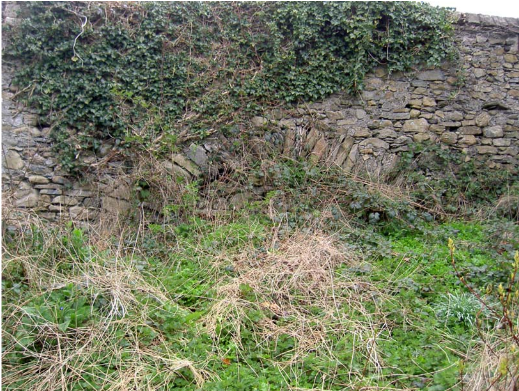
Plate 46: Possible bee alcove (Alcove 2) built into the boundary wall
