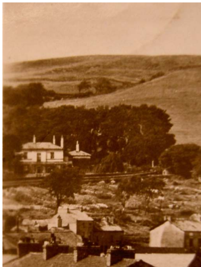
Plate 30: Detail from a photograph of c1920 showing the south-east elevation of the house with its veranda (from collection of Bernard and Elizabeth Ellis)
