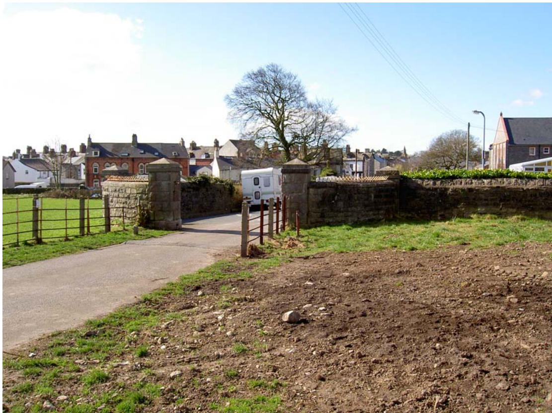
Plate 43: View of the main gate and associated fences
