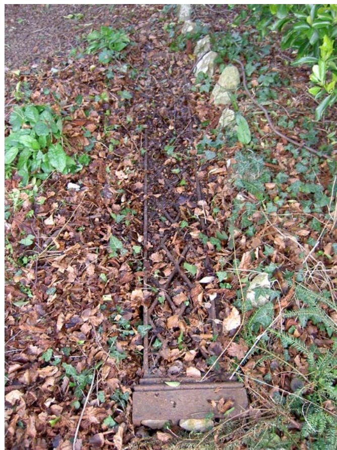
Plate 47: Remains of part of the iron veranda
