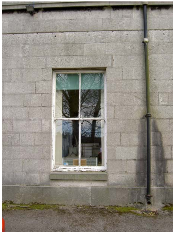
Plate 51: Remodelled window in the south-west elevation of the house
