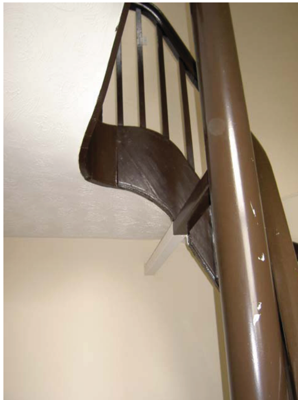
Plate 14: Horizontal bar cutting through the inner fascia of the stair well on the first floor
