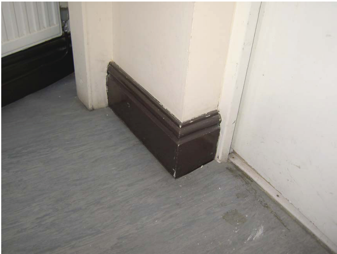
Plate 16: Modern ogee-moulded skirting board on the first floor
