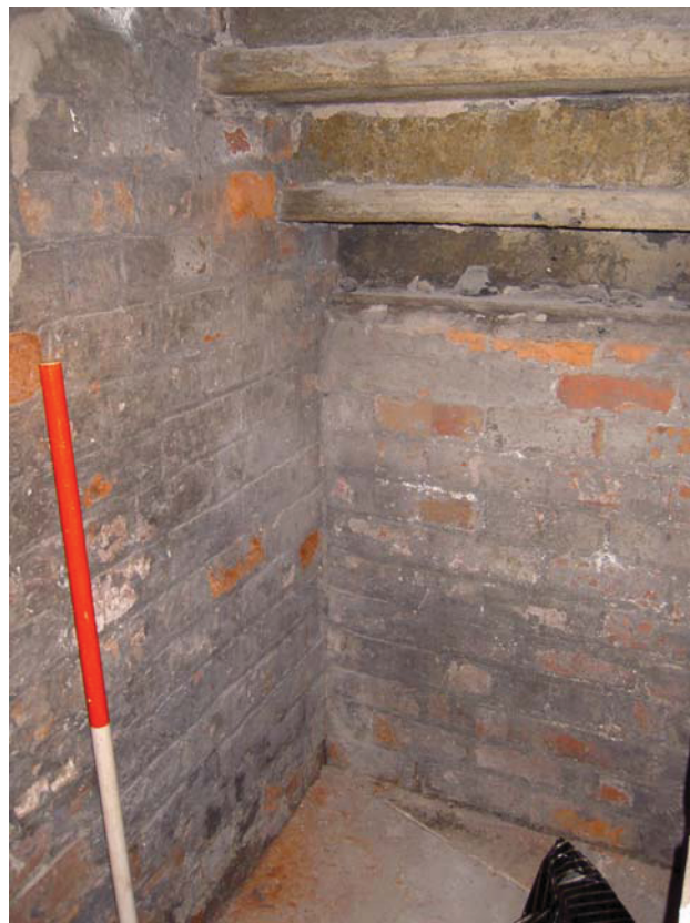
Plate 23: Brickwork beneath the basement steps
