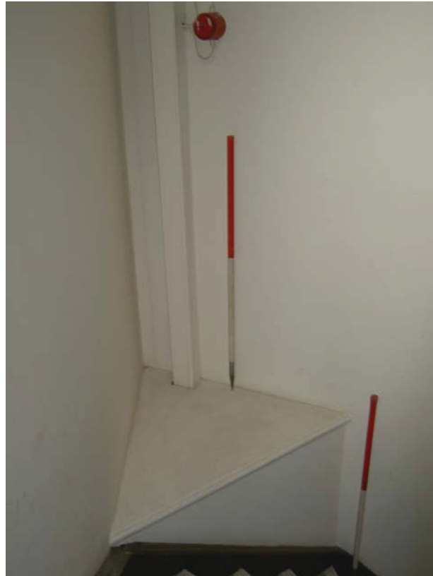
Plate 20: Moulded shelf on the ground floor
