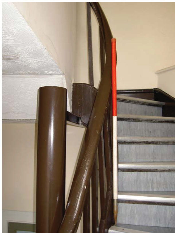
Plate 8: The top of the inserted metal post between the second and third floors
