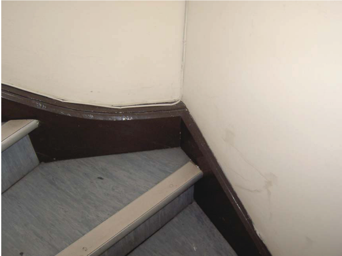
Plate 15: Original chamfered skirting board on the first floor
