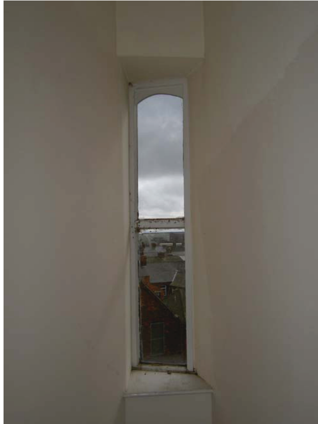
Plate 7: The south-east window on the third floor
