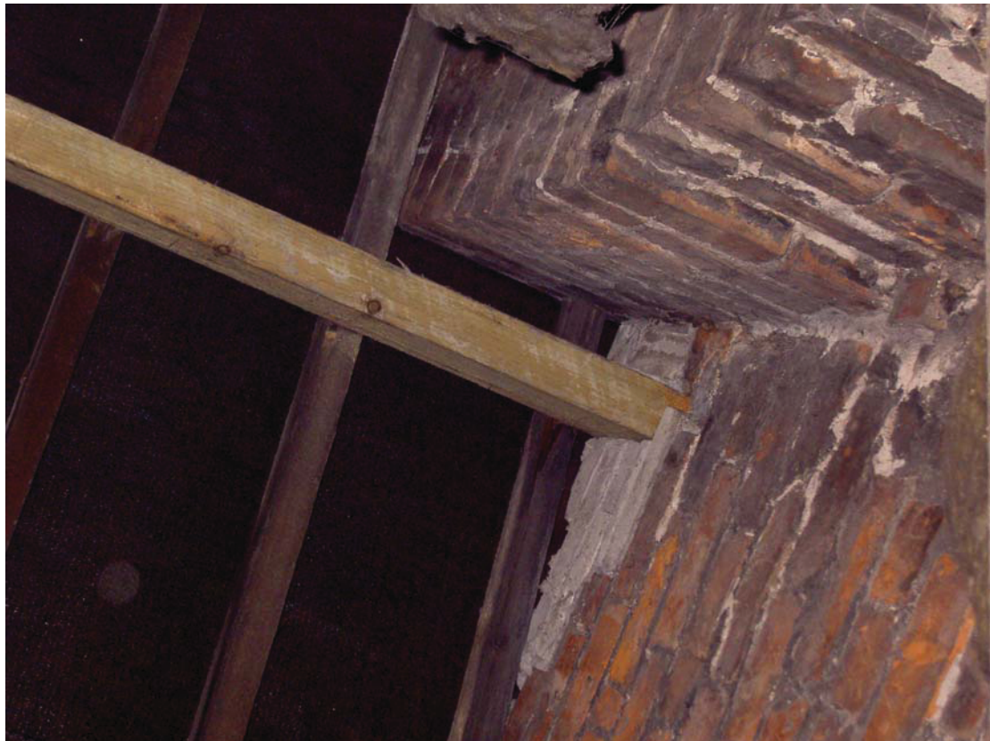
Plate 6: View inside the roof space showing the original brickwork and beam
