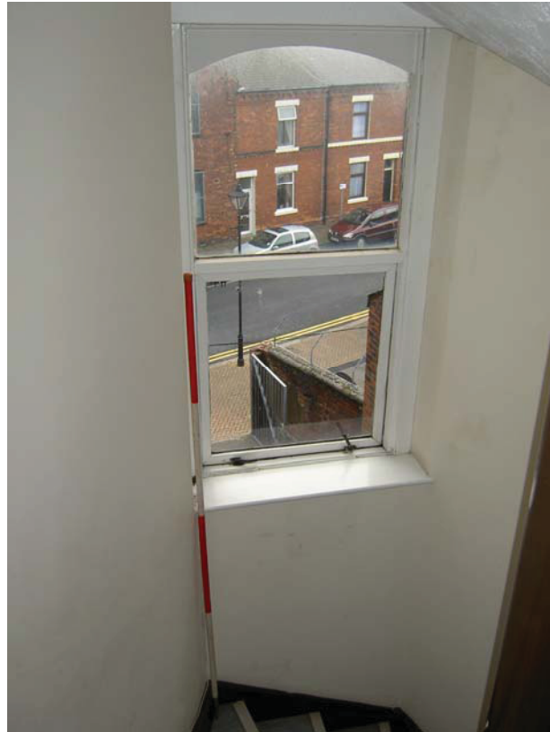
Plate 13: Window in the south side of the first floor
