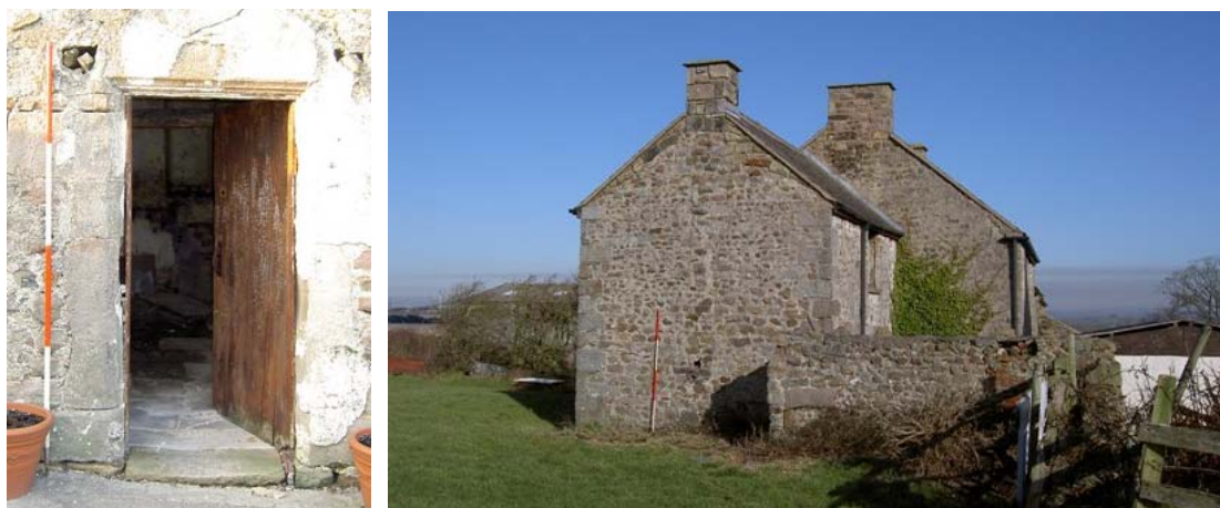
Plate 22: Detail of front door within the south elevation
