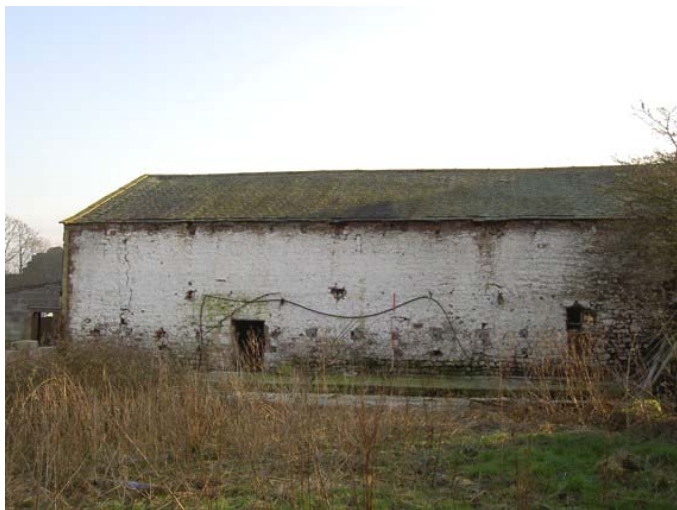
Plate 15: North elevation of the barn
