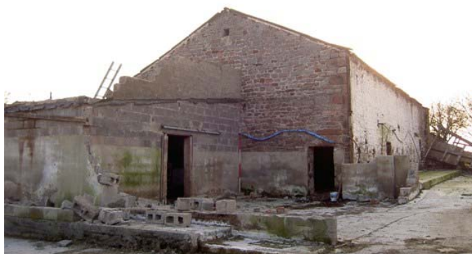
Plate 17: East gable and the remains of attached modern buildings
