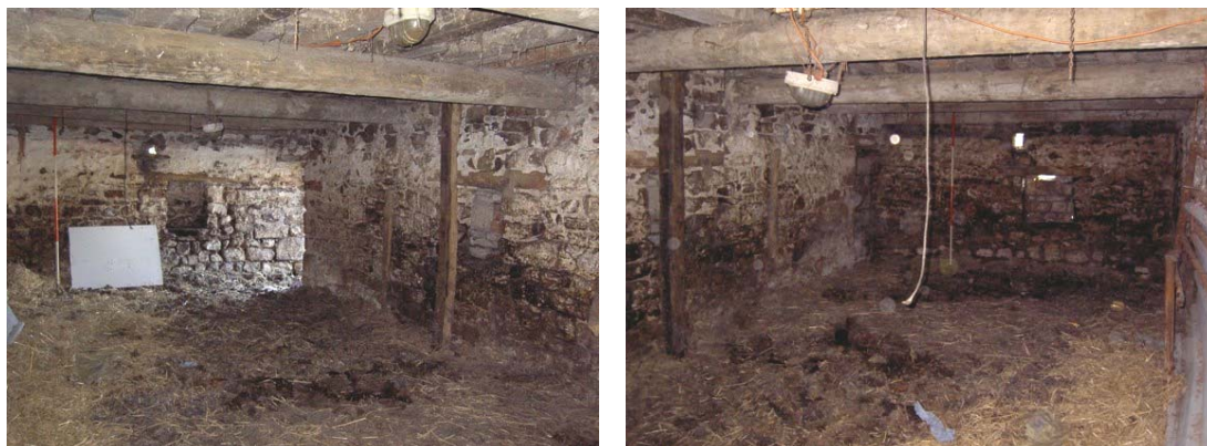
Plate 26: North-east corner of the shippon at the east end of the barn, showing the alcove in the north wall
