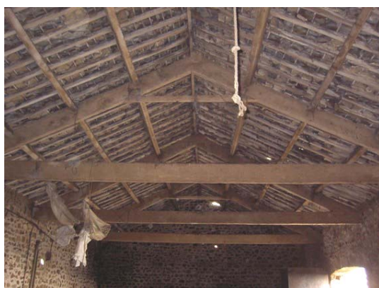
Plate 24: West faces of the trusses within the barn
