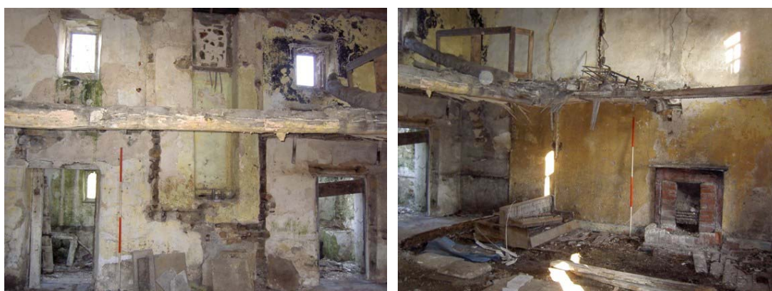
Plate 29: North internal elevation of the house
