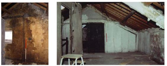
Plate 29: Partition and ceiling scars, second floor east rooms
