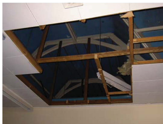
Plate 38: (right) Truss above Room 10, as visible from Room 4
