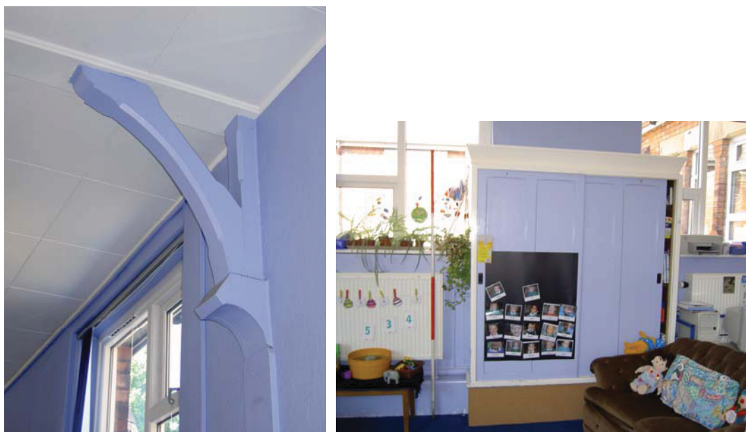
Plate 48: (left) Bracket from the roof truss in Room 18
