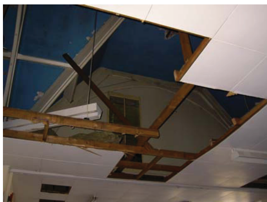
Plate 37: (left) Truss visible in Room 4
