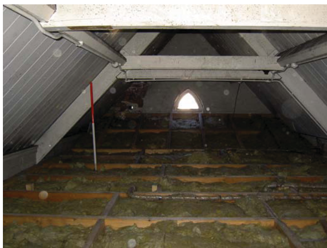
Plate 39: Roof space above Rooms 7 and 8
