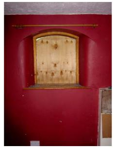
Plate 46: (left) Converted doorway in the south-west elevation of Room G12
