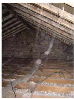
Plate 63: (left) King-post truss above Room F12b showing brick chimney stack to north-east
