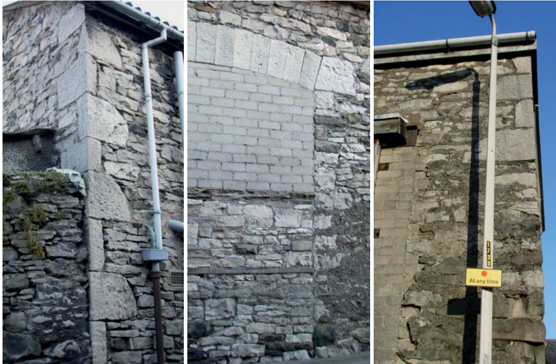
Plates 22-24: Details of the limestone quoin and doorway arches on Cross Lane
