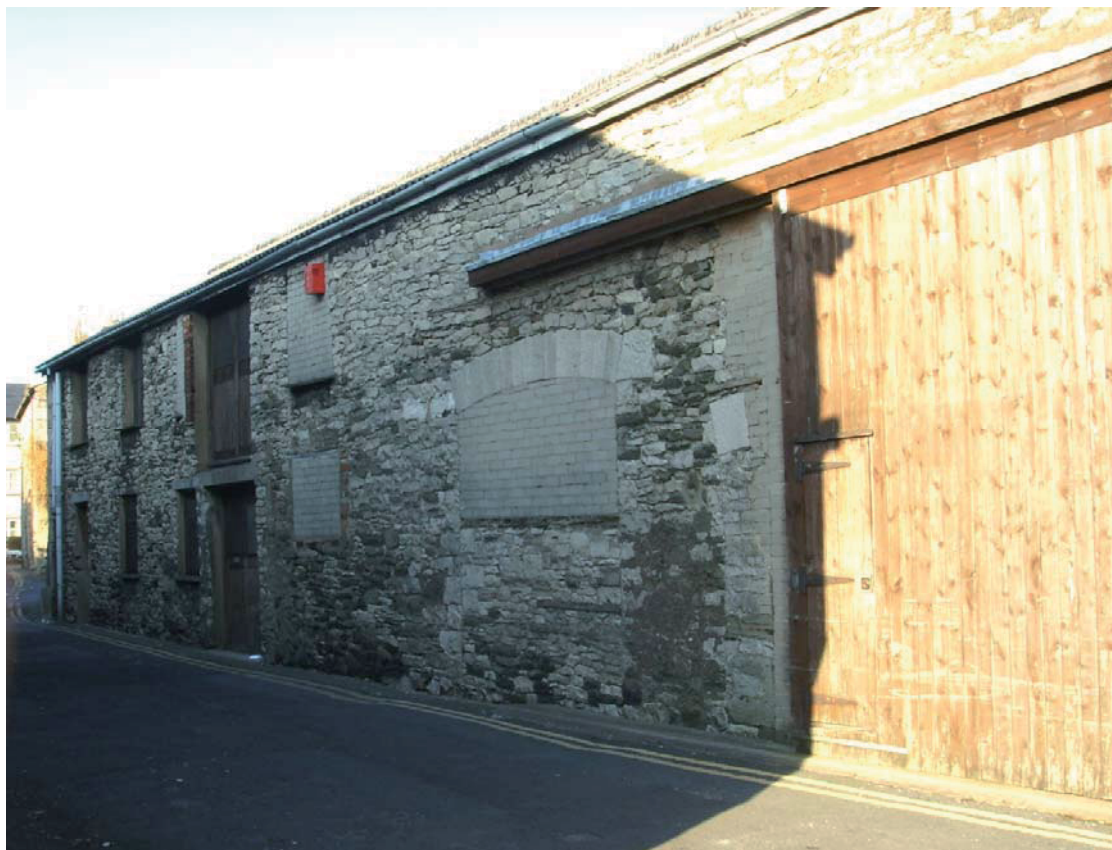
Plate 21: View of the main standing building on Cross Lane, facing north
