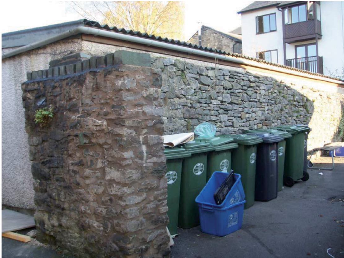
Plate 20: Rear view of the garages to be demolished, facing east
