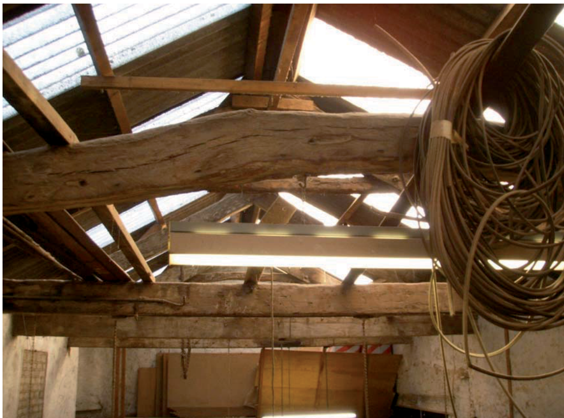
Plate 28: Possible original 18 th century roof trusses in Workshop 1
