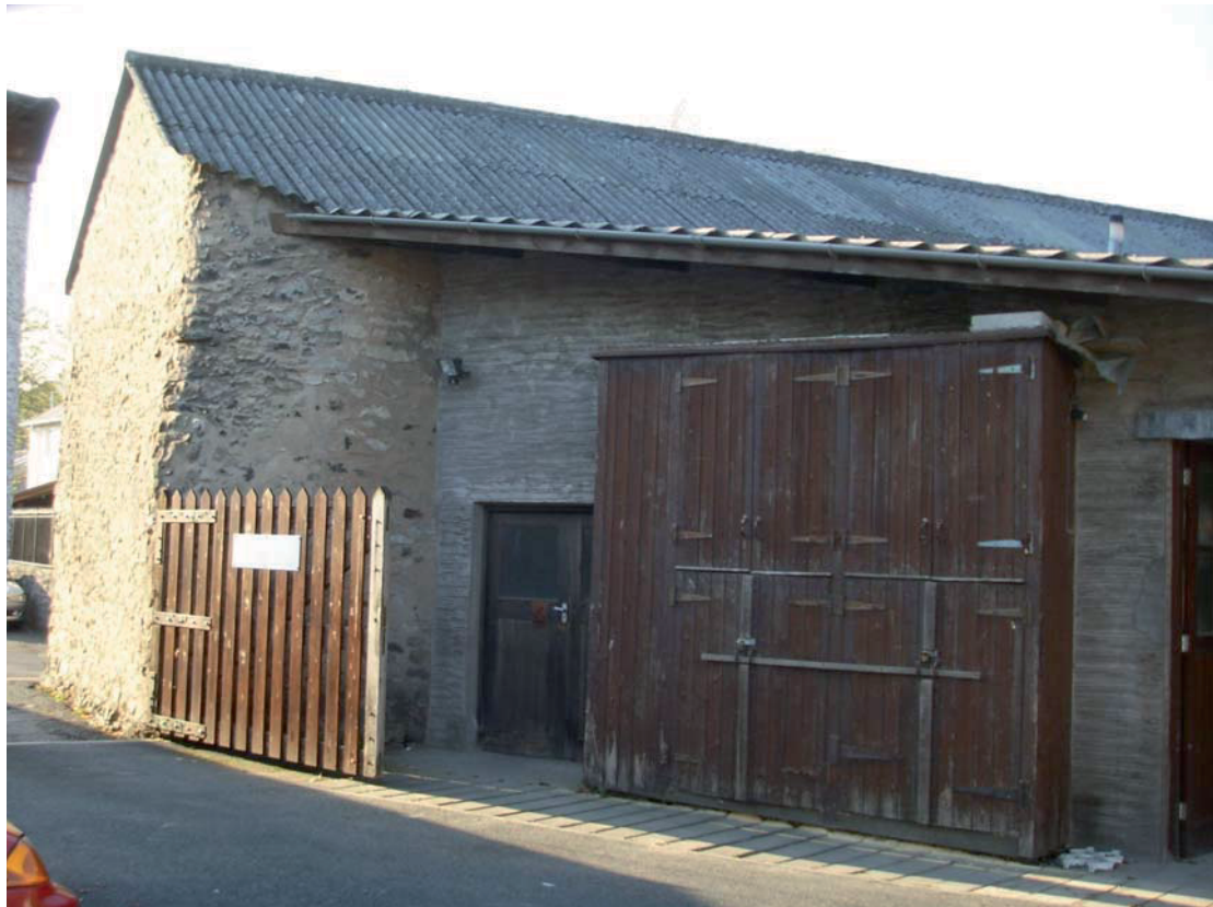
Plate 27: The south elevation of the standing buildings
