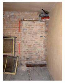
Plate 55: (left) First floor, Room 1, iron strap attached below window in north-east elevation
