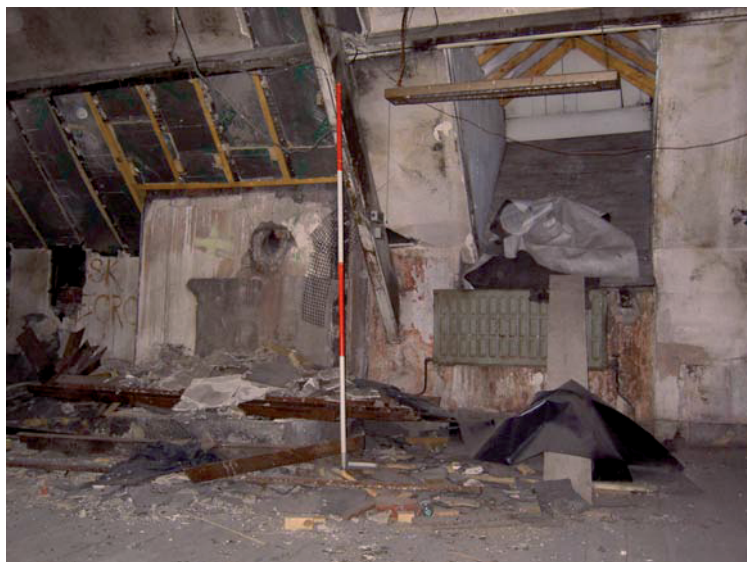
Plate 84: (above) Attic Room 2a, roof structure detail, looking south-east
