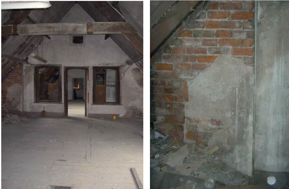
Plate 86: (left) Attic Room 2a, south-east elevation
