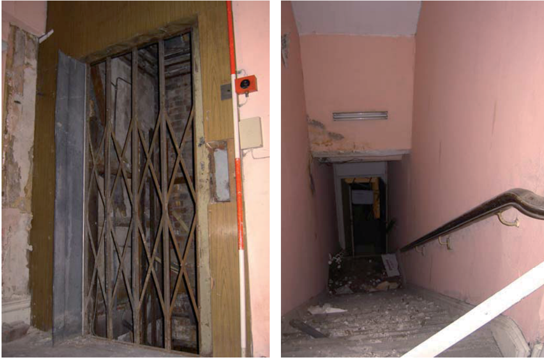
Plate 70: (left) Second floor, elevator shaft, from the west
