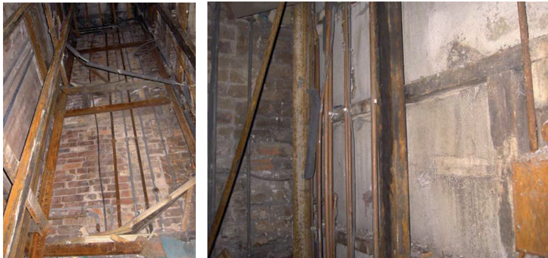
Plate 58: (left) Elevator shaft, first floor level, south-east elevation, looking upwards
