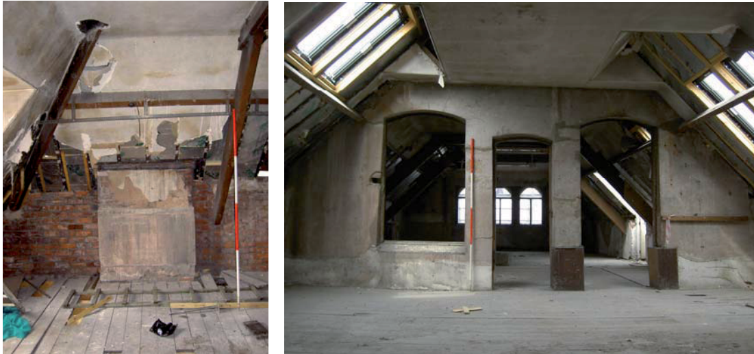
Plate 82: (left) Attic Room 1b, blocked chimney breast on south-west elevation
