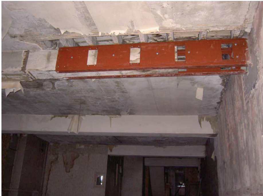
Plate 64: Detail of beam repair, Second floor Room 2
