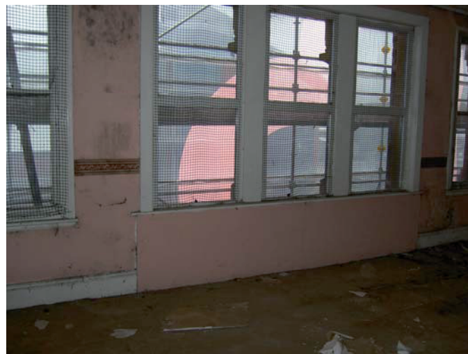
Plate 63: Second floor Room 1, north-west elevation
