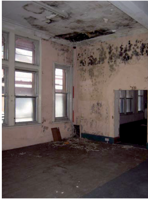
Plate 52: (left) First floor Room 1, north corner showing part of the window
