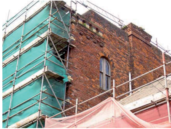
Plate 19: Part of the north-east elevation, viewed from High Street
