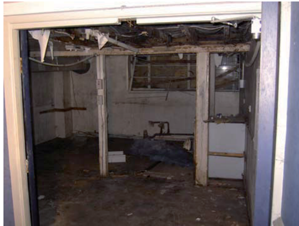
Plate 37: Ground floor Room 2a, south-east elevation
