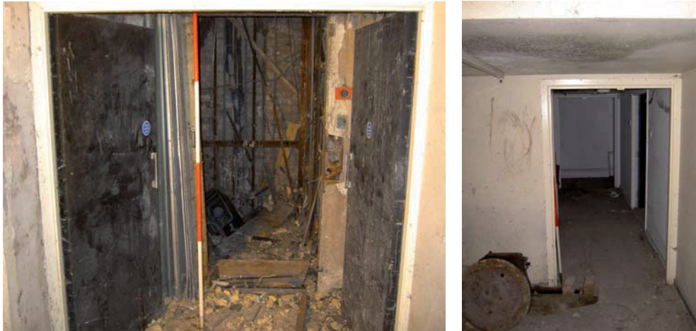
Plate 41: (left) Room S3, elevator shaft, looking south-east
