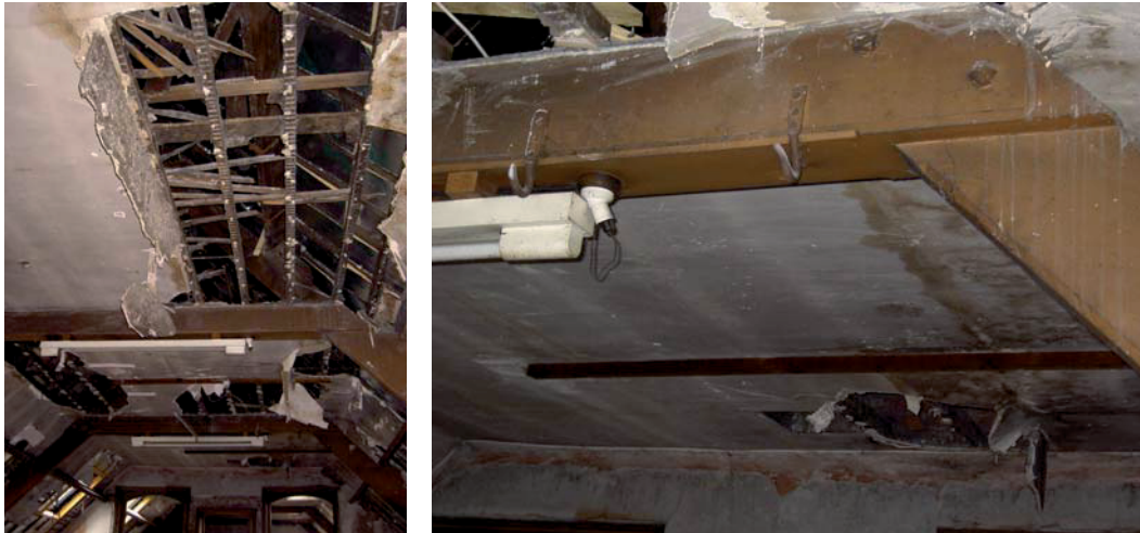
Plate 72: (left) View of ceiling structure in attic Room 1a
