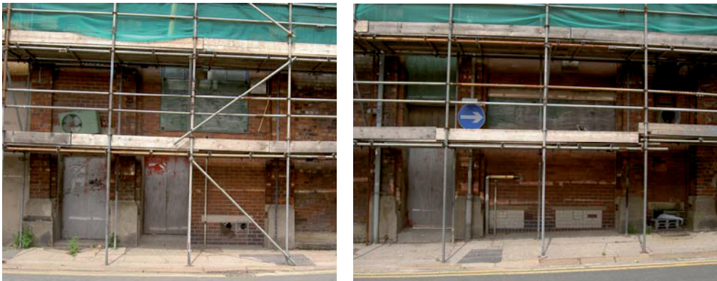
Plate 21: (left) Rear (south-east) elevation ground floor, south-west half
