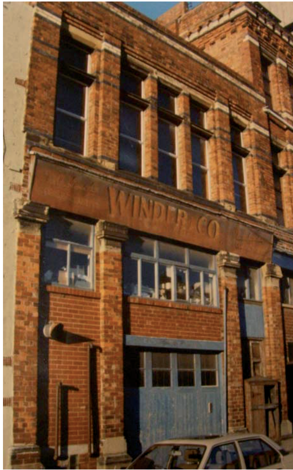
Plate 16: A view of the rear of 102 Abbey Road in 1991, just showing the original crenellated brickwork extending round No. 104 in the top right corner
