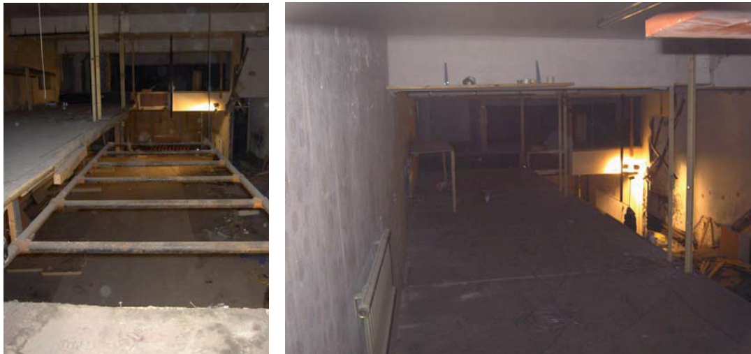
Plate 46: (right) Mezzanine floor, looking north-west
