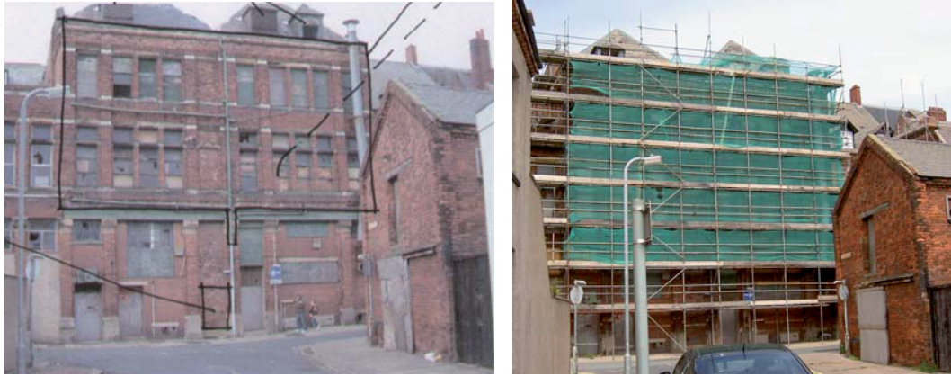
Plate 23: (left) Rear (south-east) elevation, as it appeared prior to the erection of scaffolding
