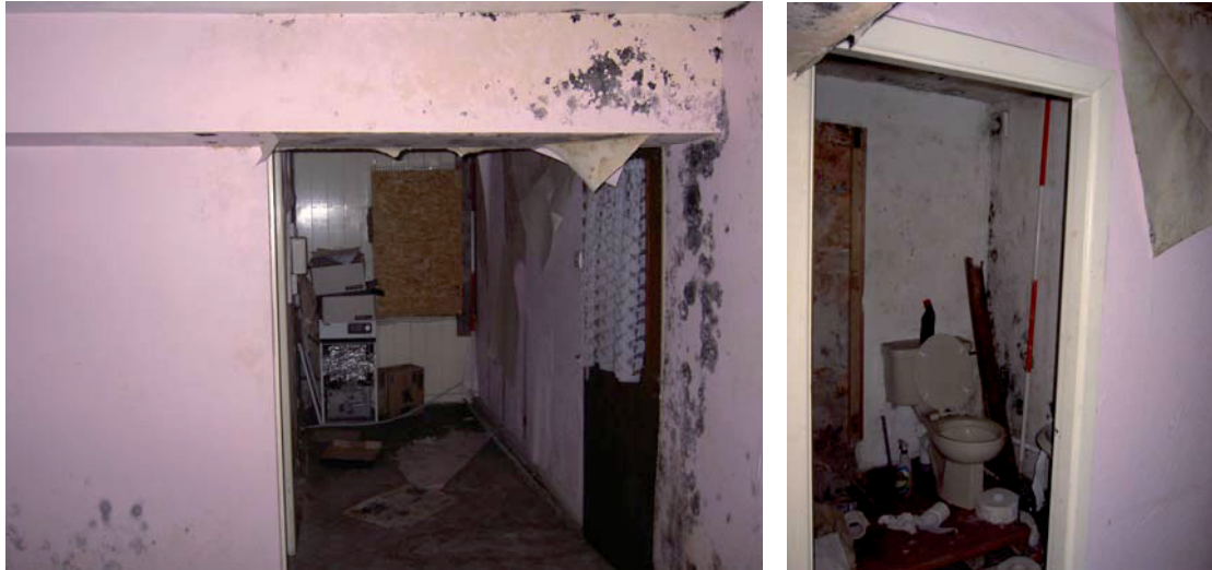
Plate 48: (left) Mezzanine room M3, south-east elevation
