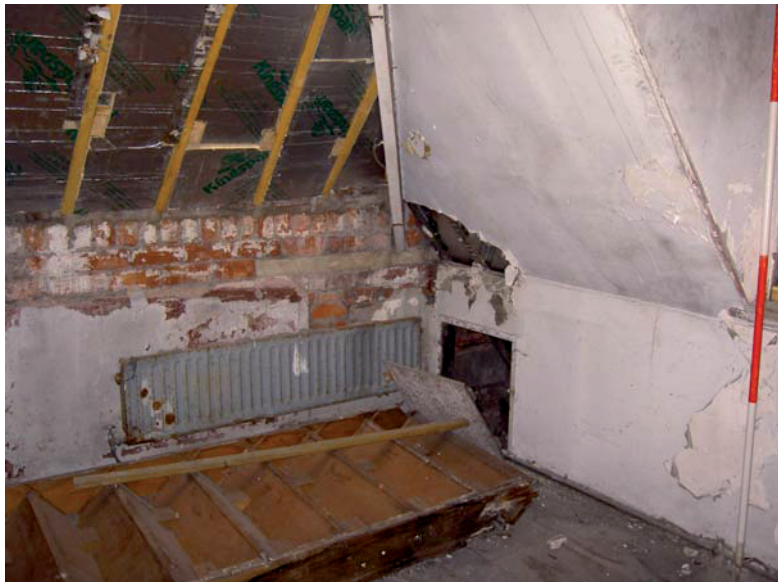
Plate 92: (above) Attic Room 2b, north-west elevation
