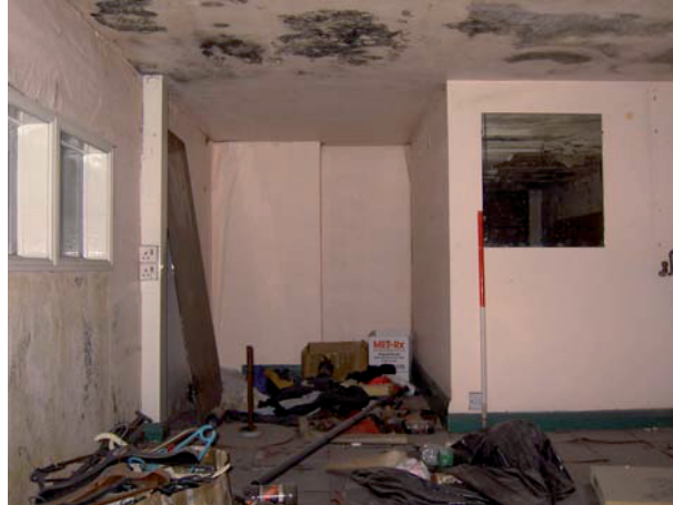
Plate 53: First floor mezzanine room, north-east elevation
