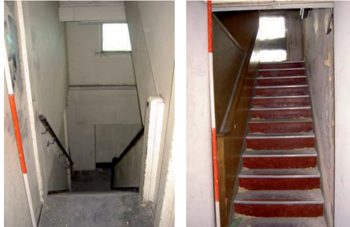
Plate 56: (left) East main stairs, looking south-east to ground floor/first floor landing
