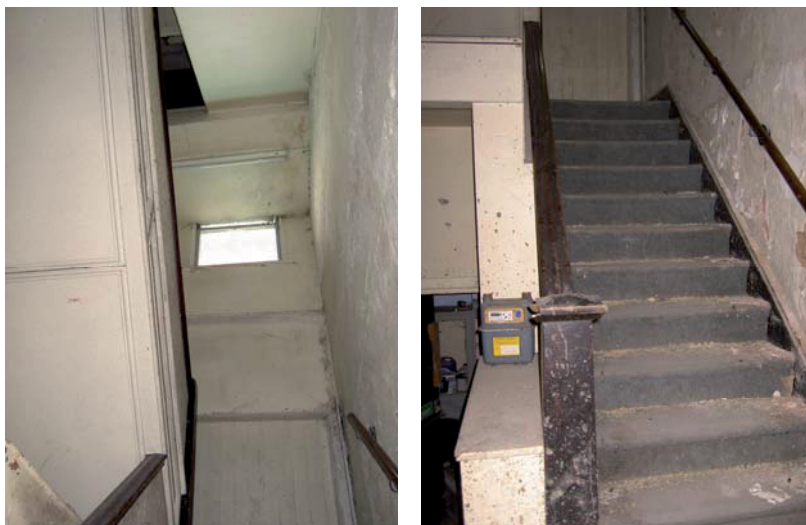
Plate 43: (left) East main stairs south-east elevation
