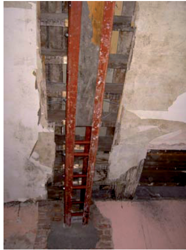
Plate 60: Detail of beam repair in Second floor Room 1
