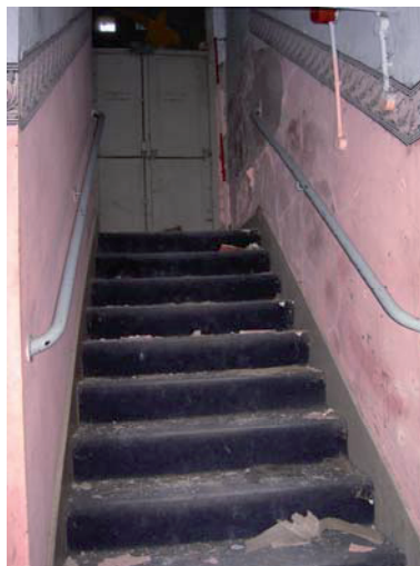
Plate 34: Basement, stairs, looking south-east up to the basement/ground floor landing
