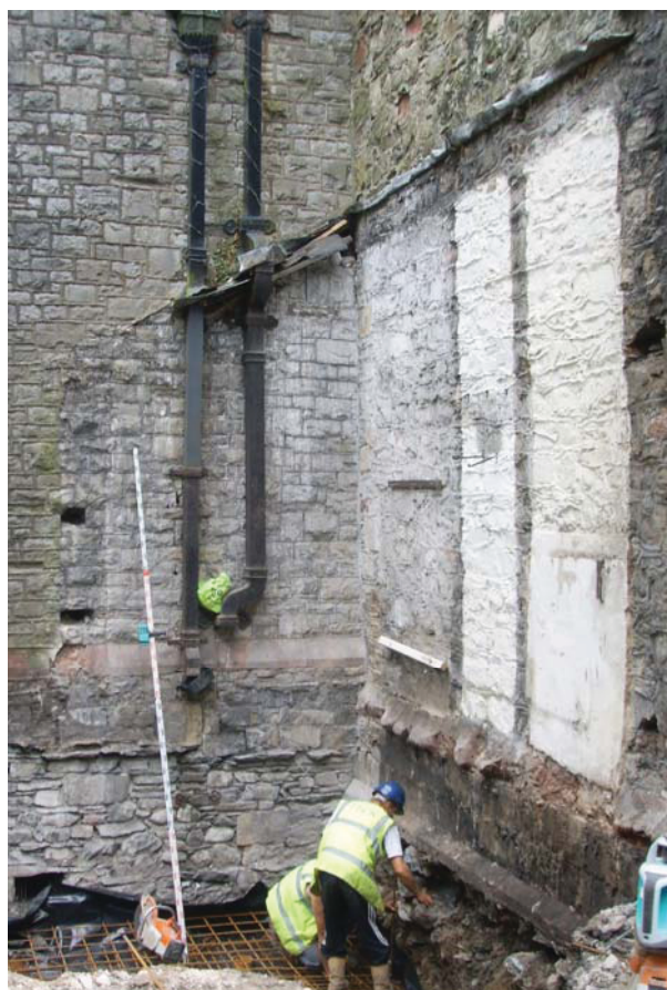
Plate 4: Working shot showing outline of demolished outbuilding
