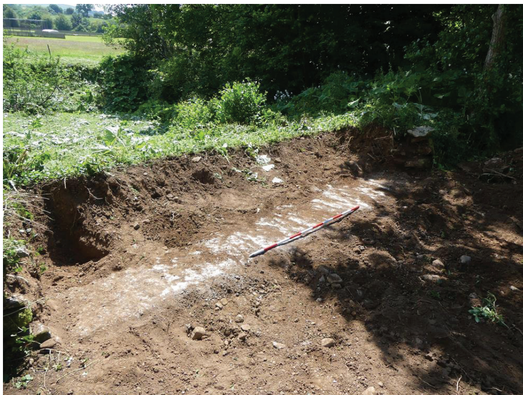
Plate 18: Concrete footing 103 fully exposed, viewed from the north
